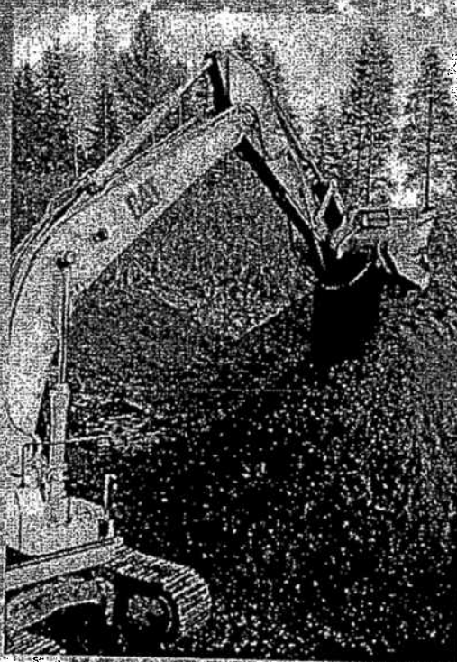
10. Stabilization of clay and contaminated soil
