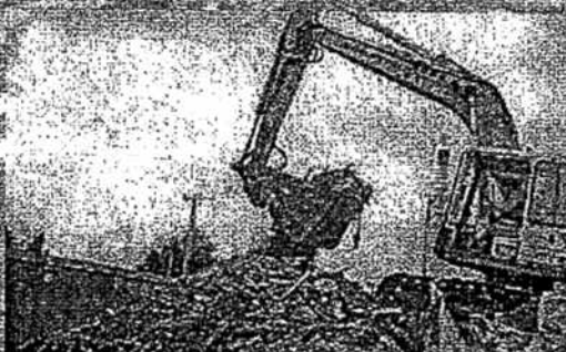
5. Construction waste and contaminated soil can be screened and crushed.
