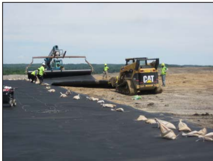
Flexible membrane liner (FML) being deployed at a landfill to control odors.
