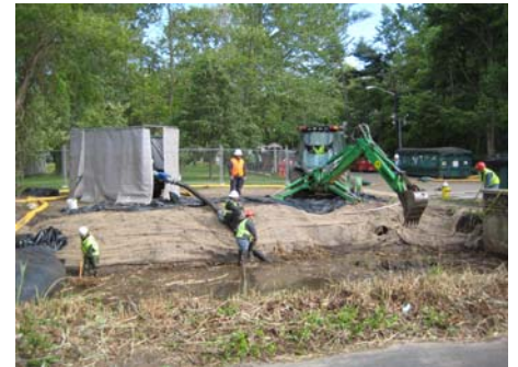
Erosion mat placed on the bank of Old Mill Creek.
