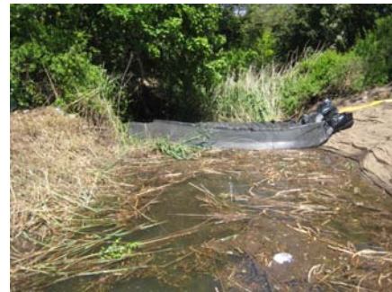
Aqua dams were placed in Old Mill Creek to re-route water from west to east overland through pipes.
