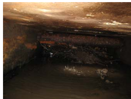
A water main was discovered in the culvert under Barnum Avenue.
