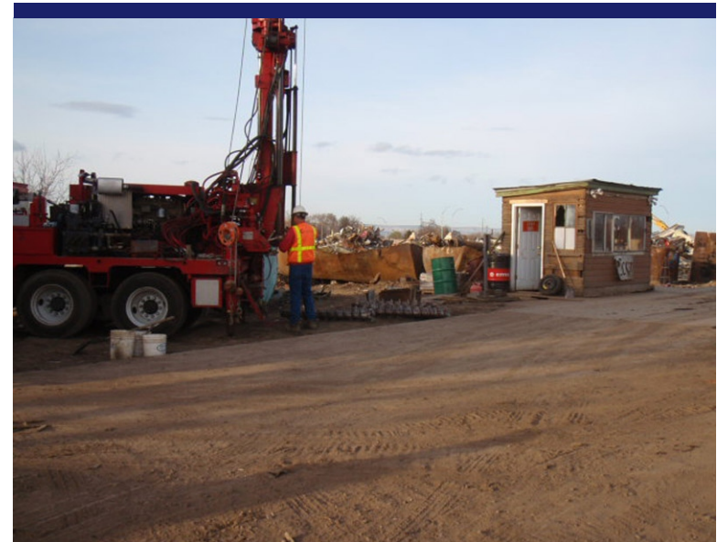
Photo 4 Set-up for MW-1 installation.
