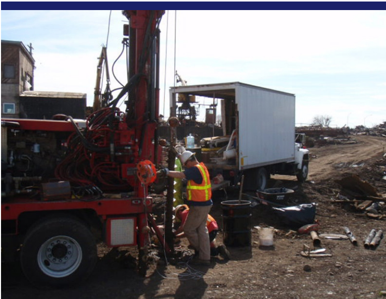
Photo 3 Drilling MW-3 with Cascade Drilling Company.
