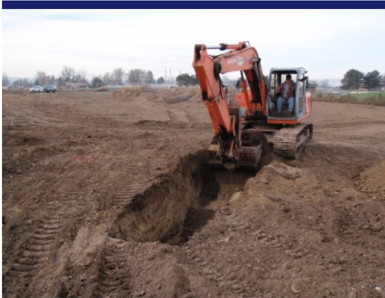
Photo 5 Excavating Test Pit 1.
