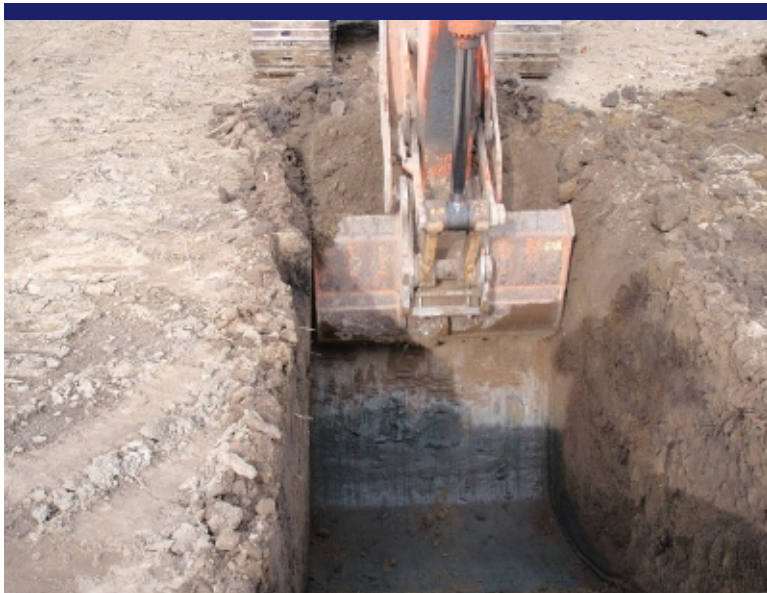
Photo 11 Starting to dig Test Pit 4. Encountering thick clay.
