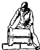
Laying on Top Half Conduit
