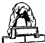
Setting on Bottom Half Conduit
