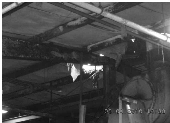
A leaky roof on the Pickens Plating building could allow rain to reach open acid vats and cause a chemical reaction that would release dangerous fumes.
