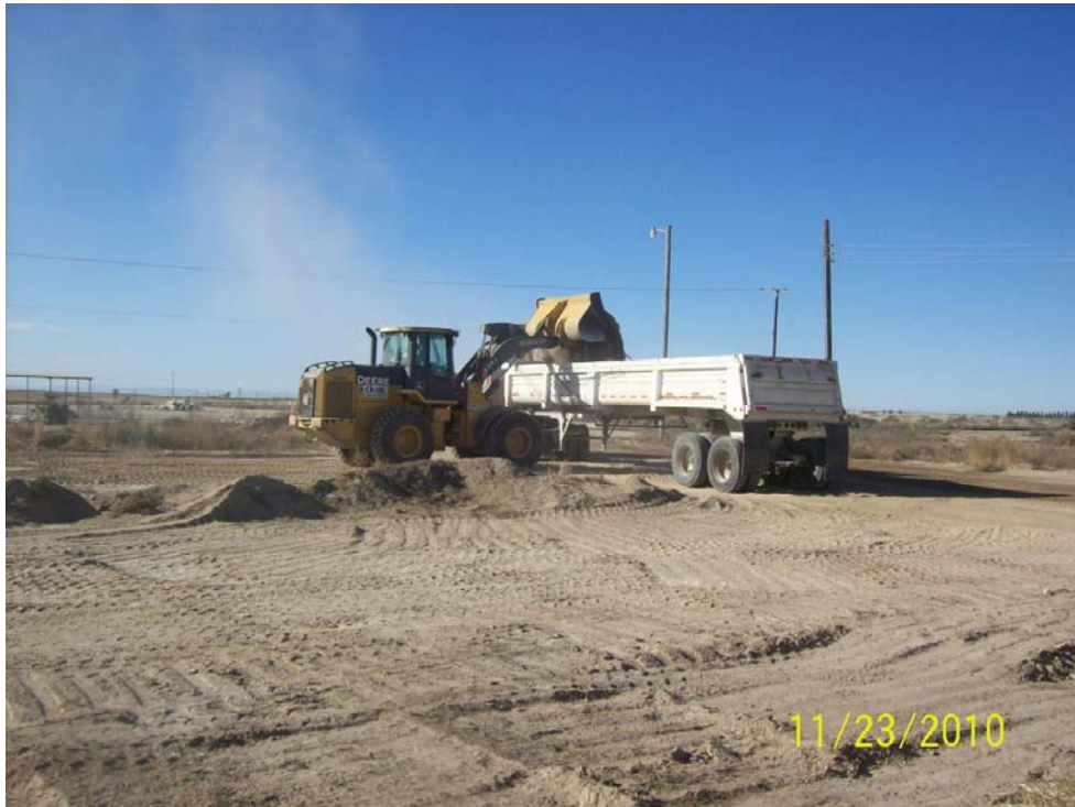
ERRS operator loading a truck with non-hazardous soil from Area B to be transported to Charter Waste Landfill in Odessa, TX (103_2482)
