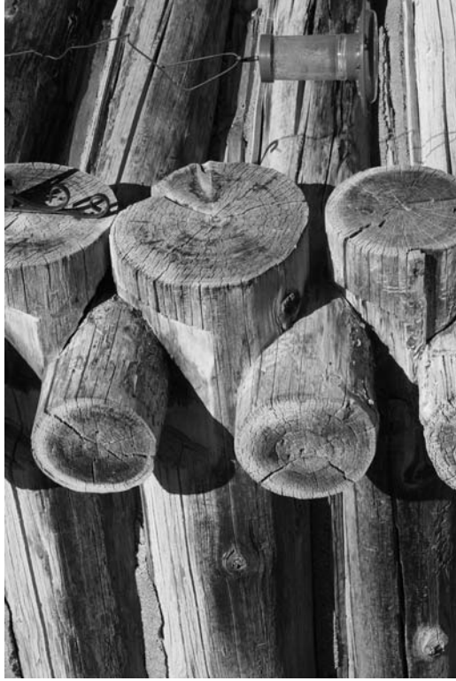
View of V-notched logs, detail taken 9/9/2009
