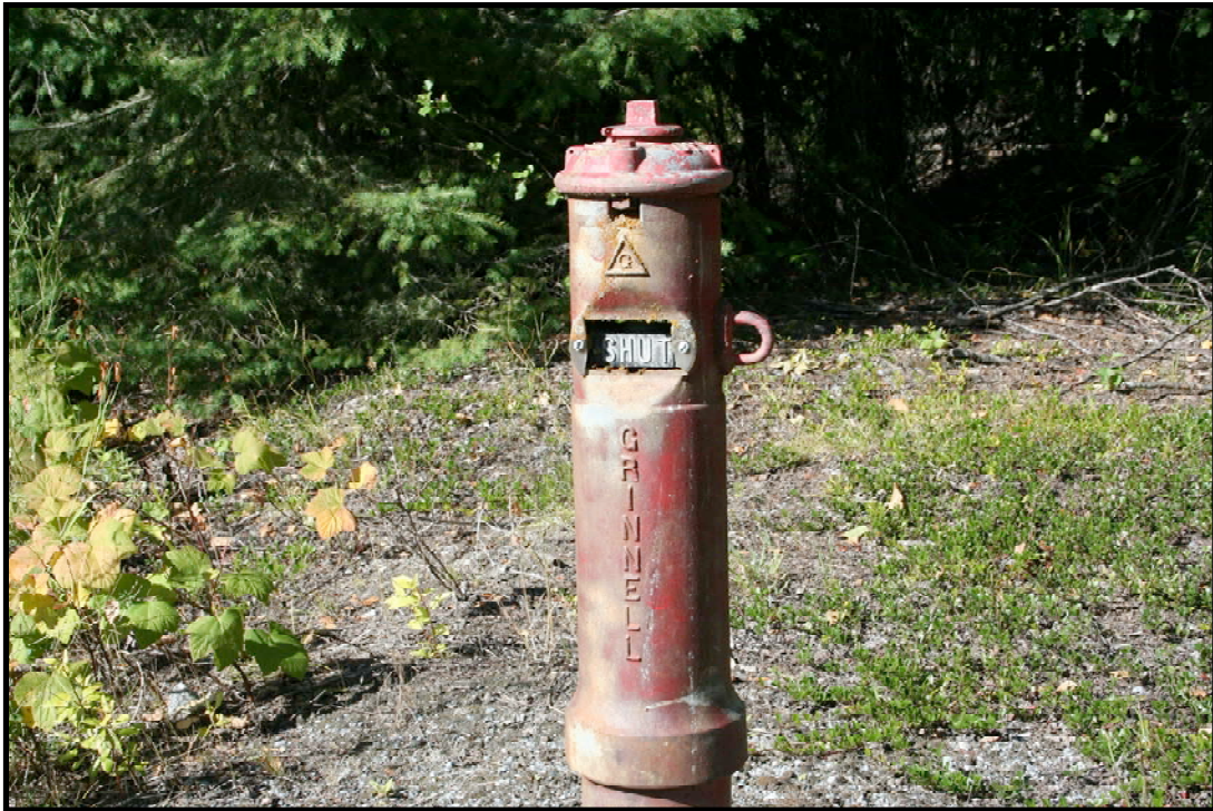
Figure 10. Sluice valve spigot control, view to the southeast.
