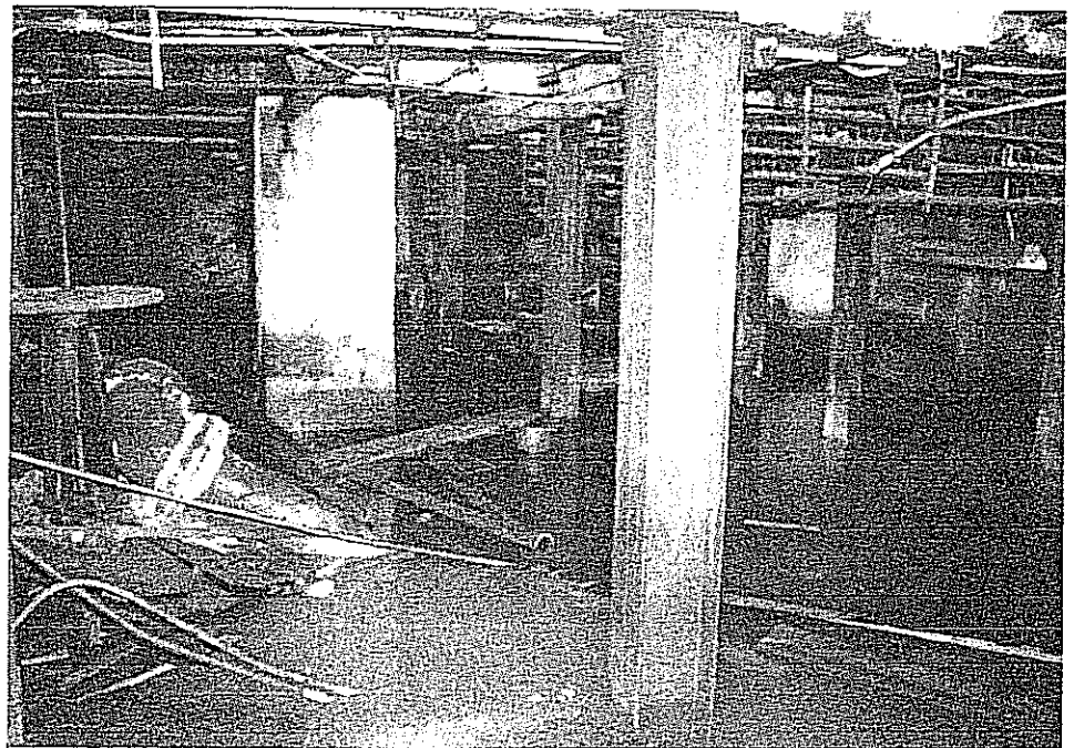
FLOODED LOWER LEVEL OF POWER PLANT BUILDING
