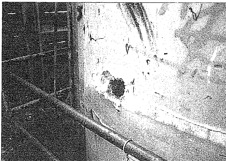
POSSIBLE ASBESTOS CONTAINING INSULATION AROUND SMOKE STACK SOUTH END OF POWER PLANT BUILDING
