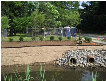
View of the restored area with jute mat used as erosion control.
