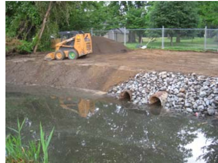
Outfall pipes, found in the center of Old Mill Creek, were reattached during the Landscape Restoration activities.
