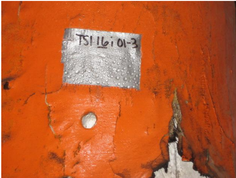
Tsi16i-01-3_16 inch Orange Boiler Wrapped Piping
