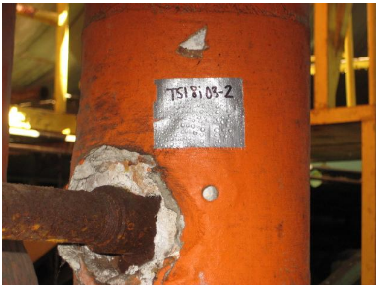
Tsi8i-03-2_8 inch Orange Boiler Wrapped Piping
