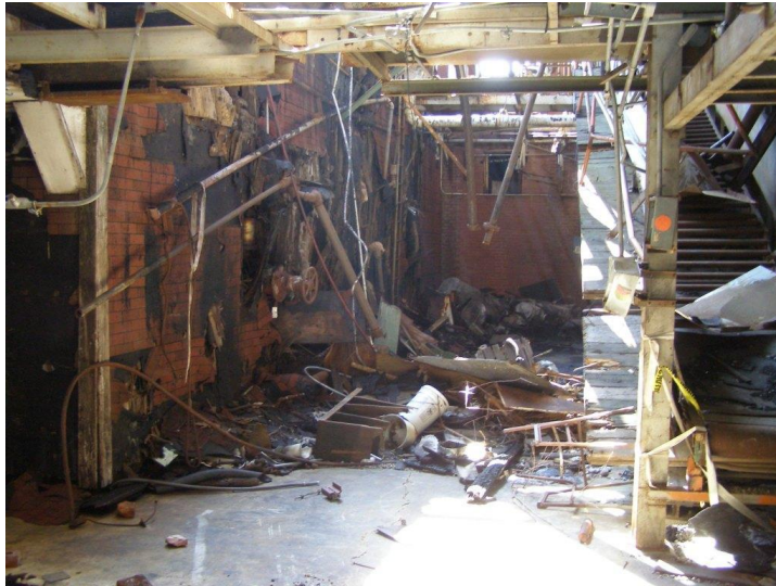
Photo 4. Collapsed Conveyor Belt and Breezeway Area (Figure 1, Area 7)
