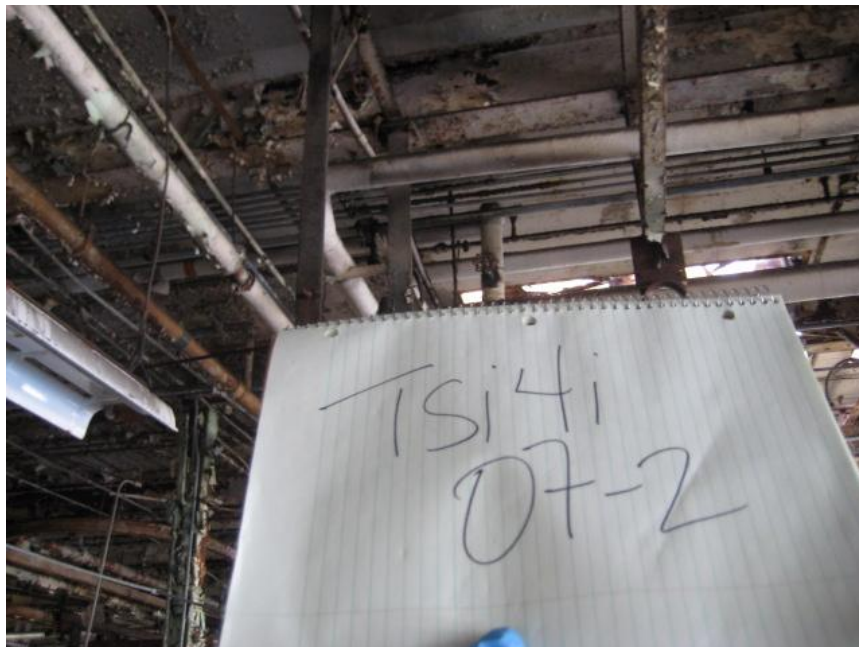
Tsi4i-07-2_4 inch White Wrapped Piping-Green Band
