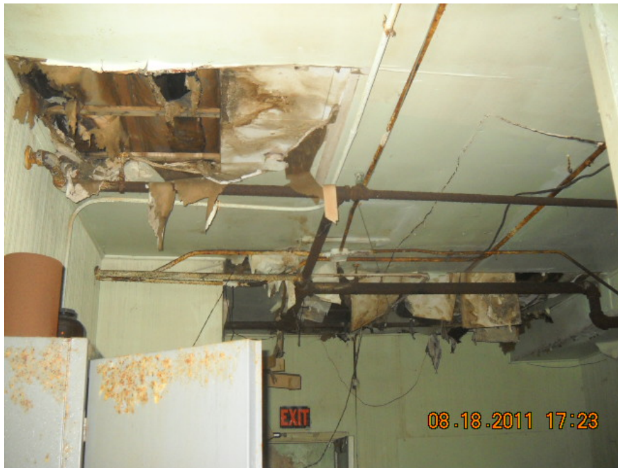
Site: Lyndon Street Drum Site Photograph No.: 8 Direction: West Subject: Deteriorating roof and ceiling in Room A
