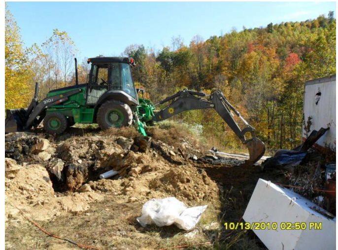
Figure 5 Contaminated soil excavation.
