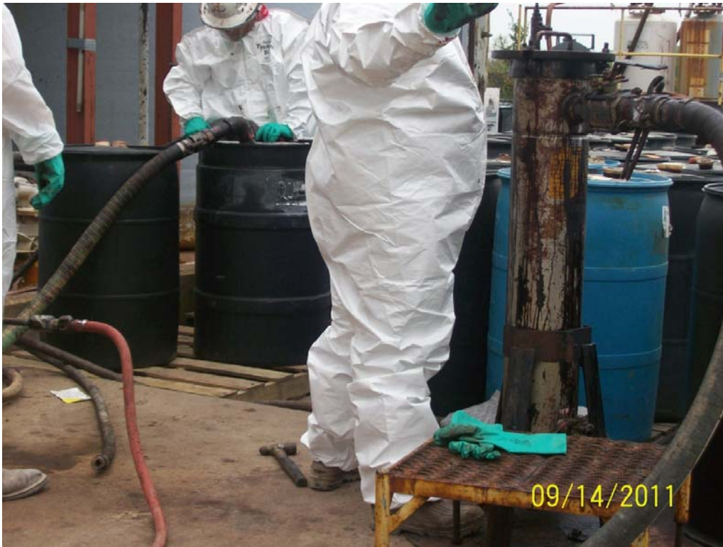
Filtration of bromobenzene, using a 50-micron filter (Photo# 103_3356).
