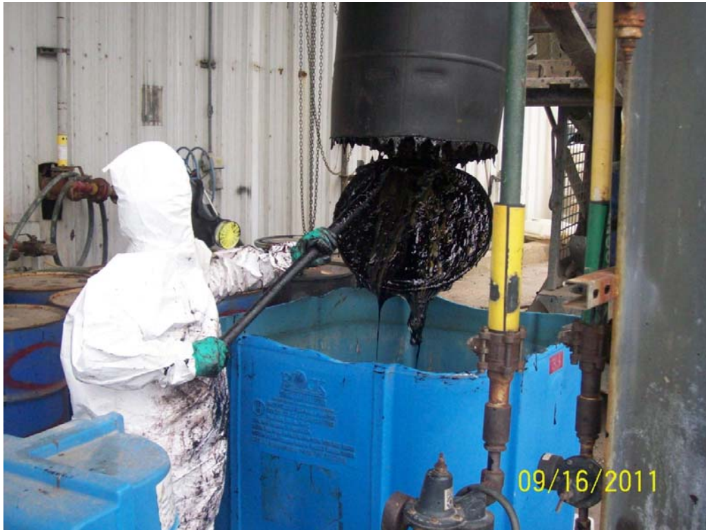
Consolidation of DBFB/dibromotoluene mix (sludge) into totes (Photo# 103_3365).
