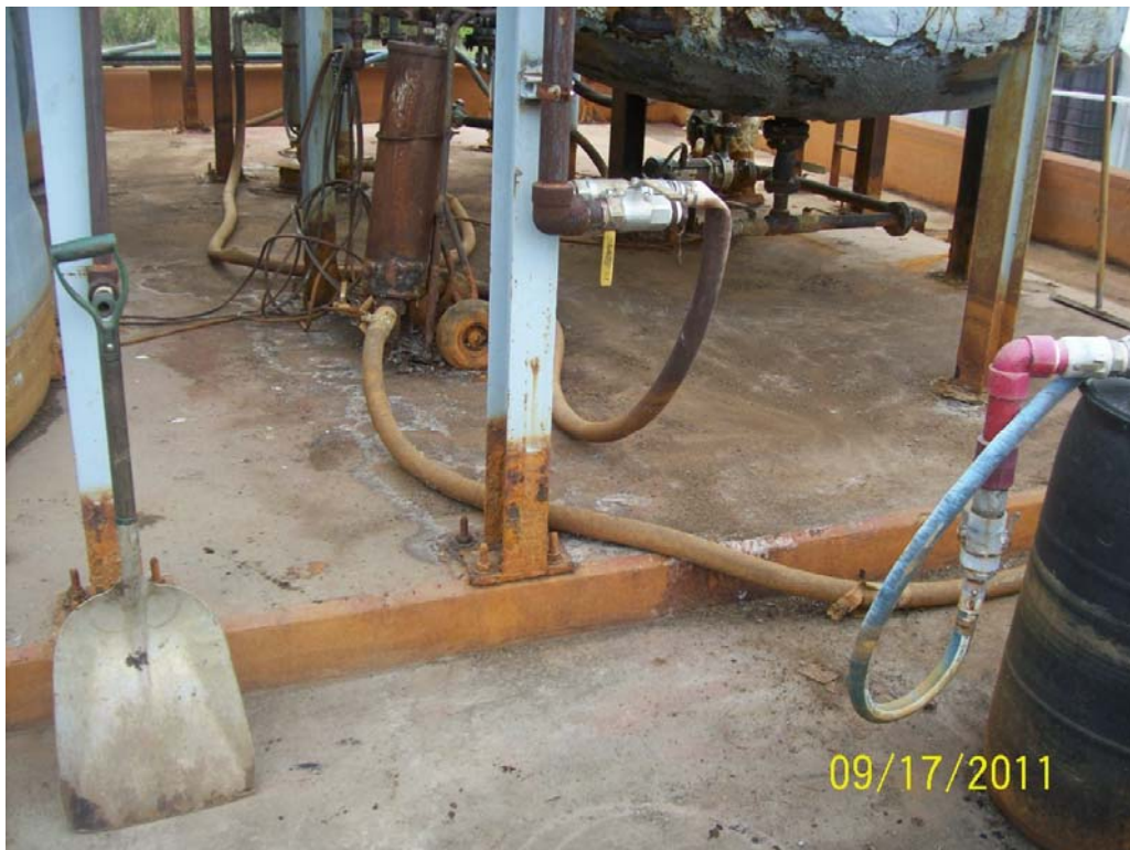
Decontaminated New Tank Farm secondary containment (Photo# 103_3376).
