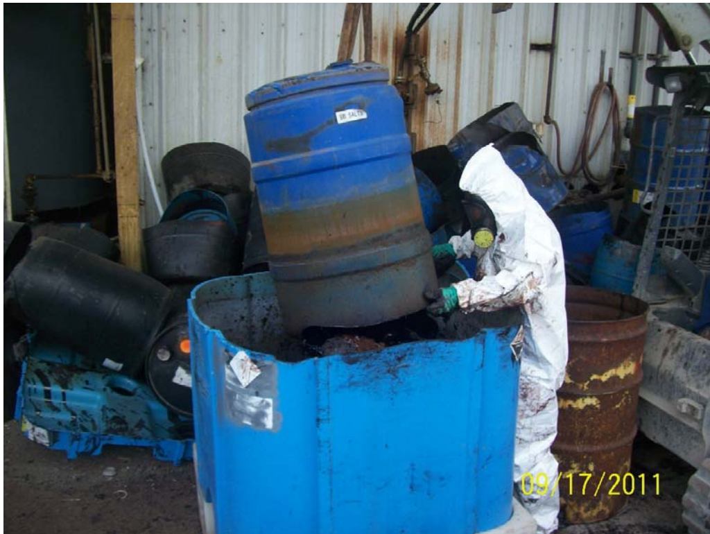
Sludge consolidation (Photo# 103_3369).
