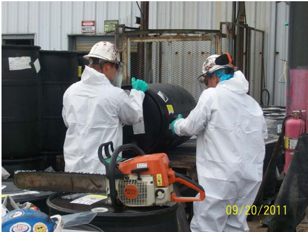
Resizing emptied drums for disposal shipment (Photo# 103_3388).
