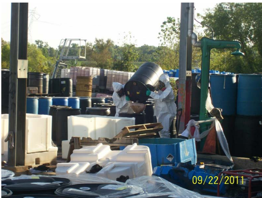
Drum consolidation (Photo# 103_3408).
