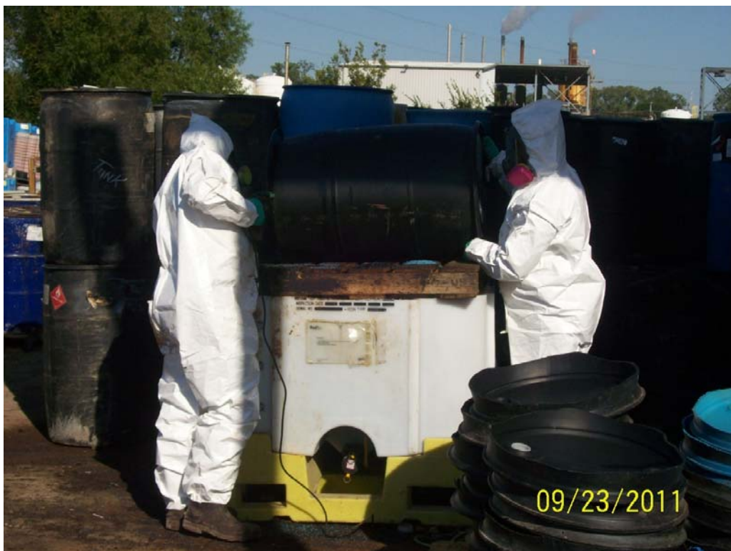
Resizing emptied drums (Photo# 103_3427).
