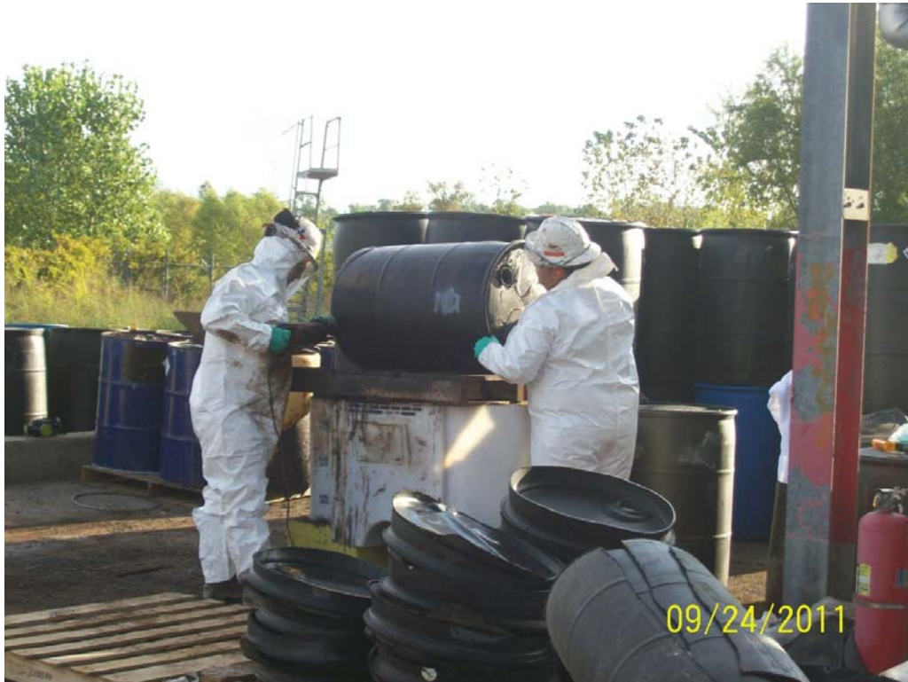
Resizing emptied drums (Photo# 103_3435).
