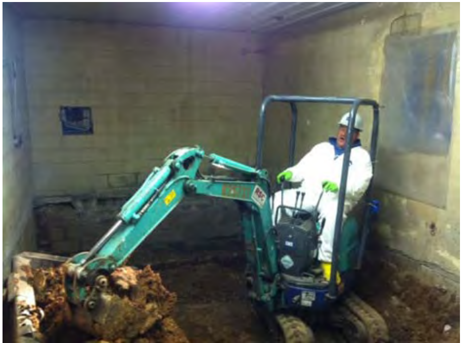
An EPA contractor uses a mini-excavator inside the small room at Sandies that once housed the dry cleaning operation.
