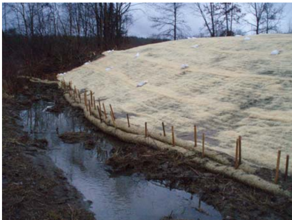
Coconut mat—Erosion control
