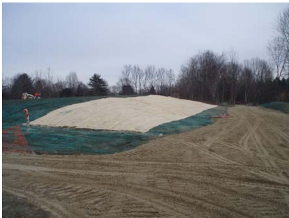
Coconut mat—Erosion control
