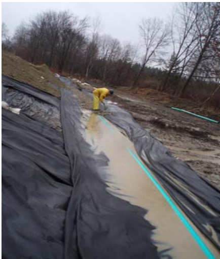
Curtain drain installation
