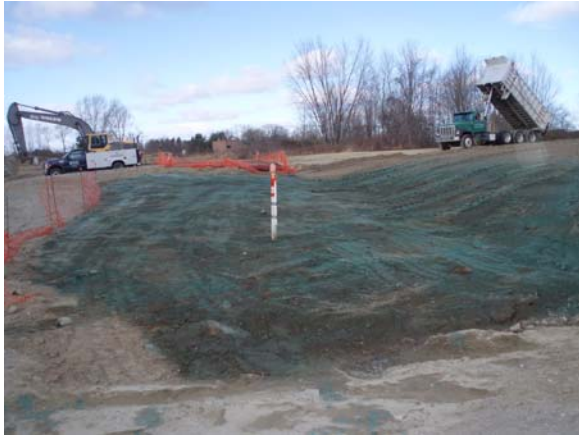
Gas pipeline hydro-seeded
