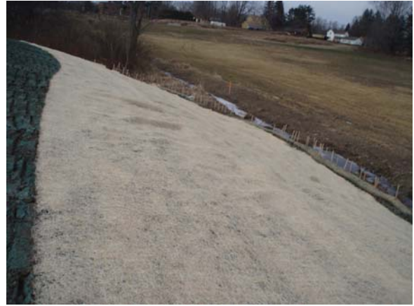
Gas pipeline hydro-seeded
