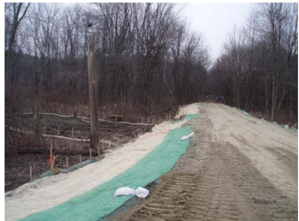
Coconut mat—Erosion control
