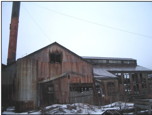
Figure 7: No. 5 Reverberatory Furnace Building (located in the center of the photo), south side, showing failed windows and intact south roof
