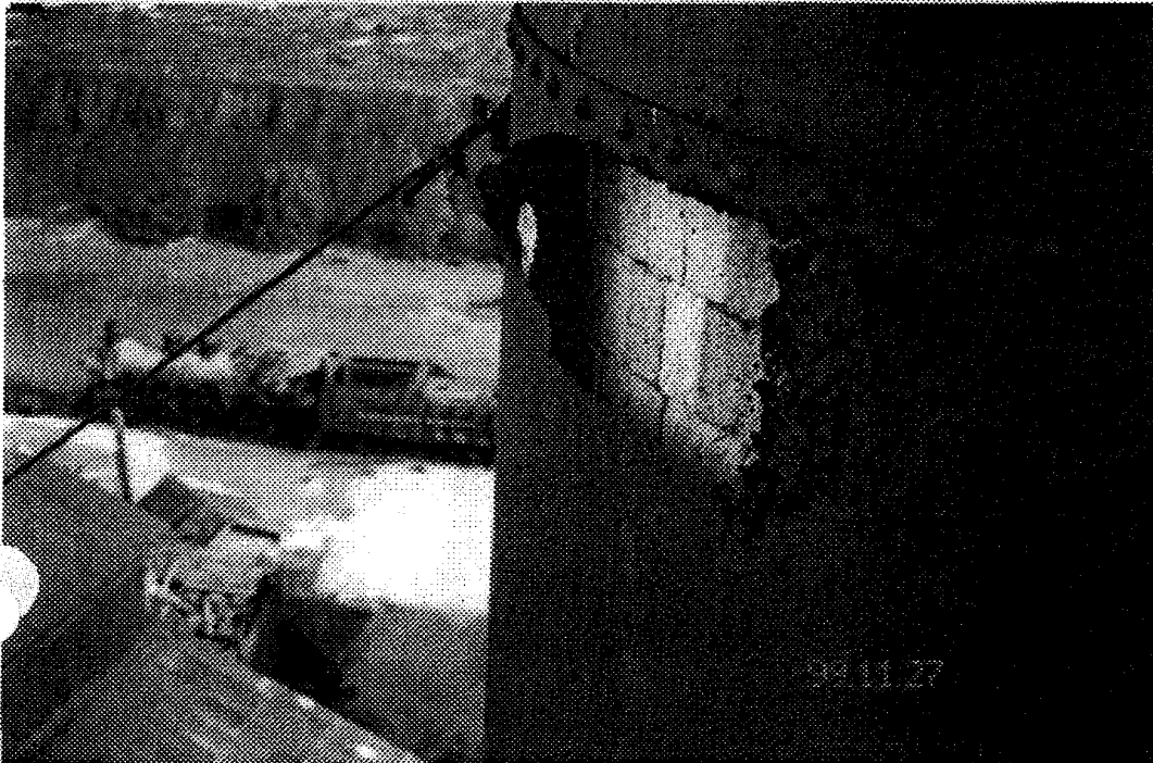
Photo # 6: Hole in steel plate noted \pm 15' below top of stack, west quadrant.
