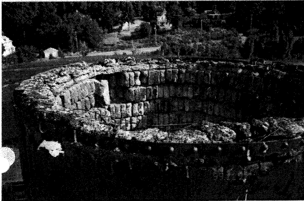
Photo # 1: View of lining brickwork at top of stack.
