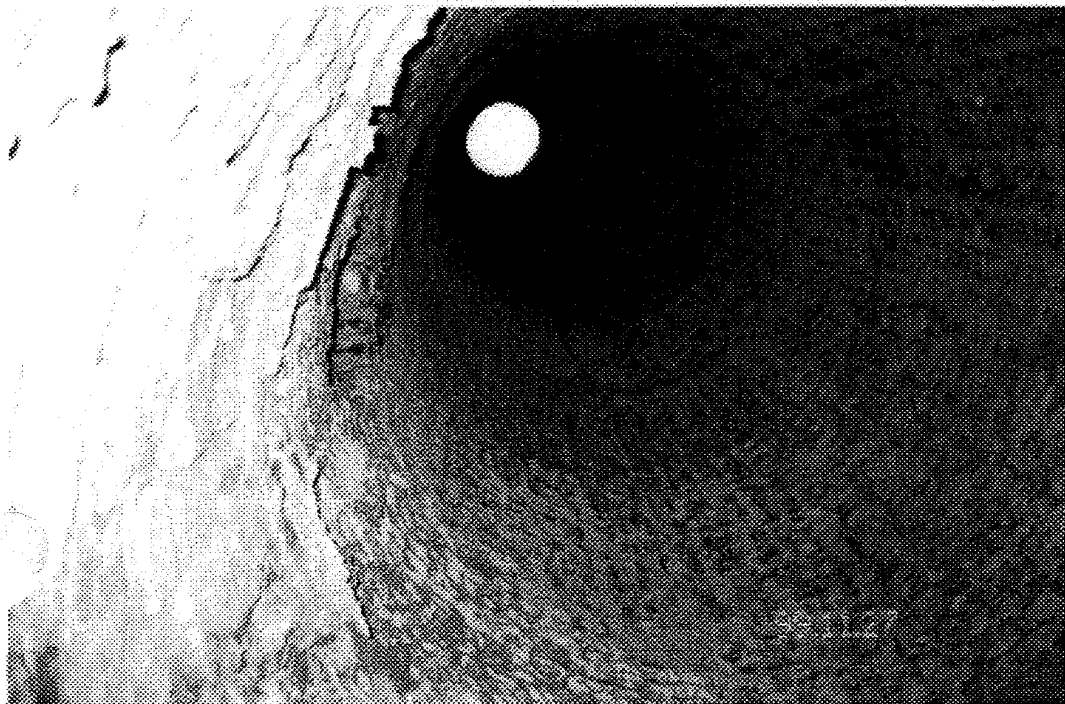
Photo # 3: View looking up lining brickwork from base of stack.
