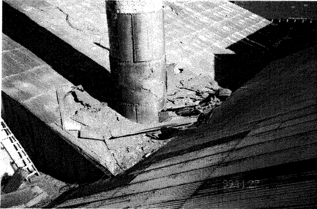
Photo #12: View of stack at roof elevation. Note steel debris laying on roof.
