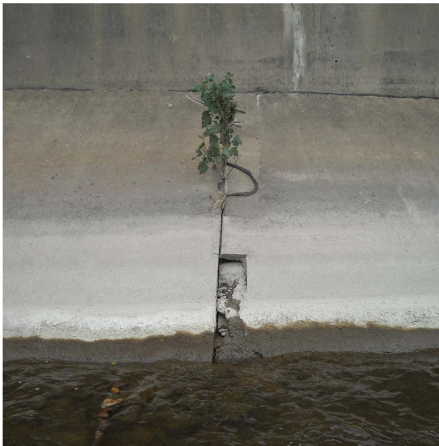
Compromised concrete paving joint (pictured above) leaking oily sheen
