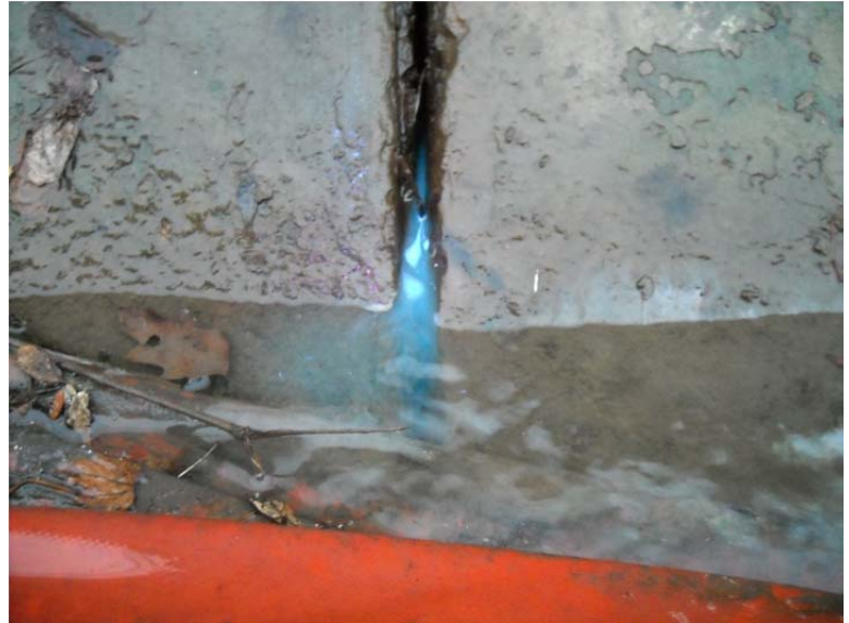
Compromised concrete paving joint (located west of joint pictured above) leaking oily sheen. Fluoresced under UV spotlight.
