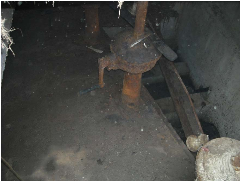
Hand cranks associated with sanitary sewer valves located below
