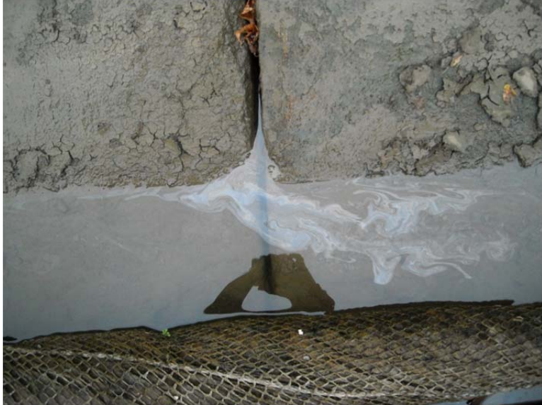
Compromised concrete paving joint (pictured above) leaking oily sheen
