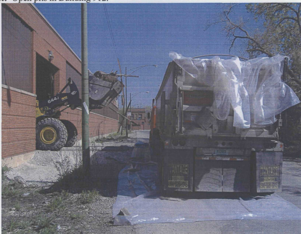
Site: Ingersoll Photo Number: 10 Direction: North Subject: ERRS loading debris from Building 1014 into lined truck for disposal.
