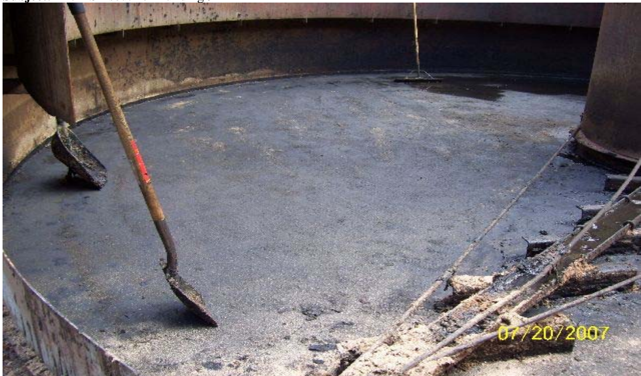
Site: Ingersoll Removal Site Photo Number: 35 Direction: East Subject: The AST south of Building 914 after sludge removal by ERRS
