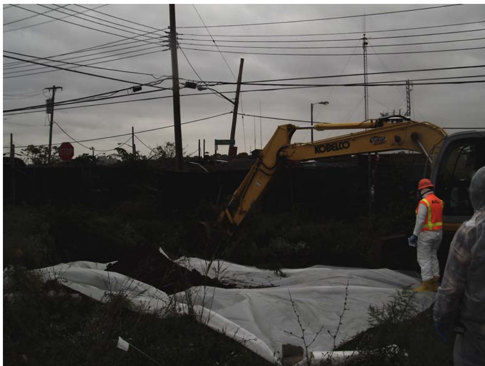
Photograph 1. 4 October 2010. Backhoe excavating Test Pit ZA-1.
