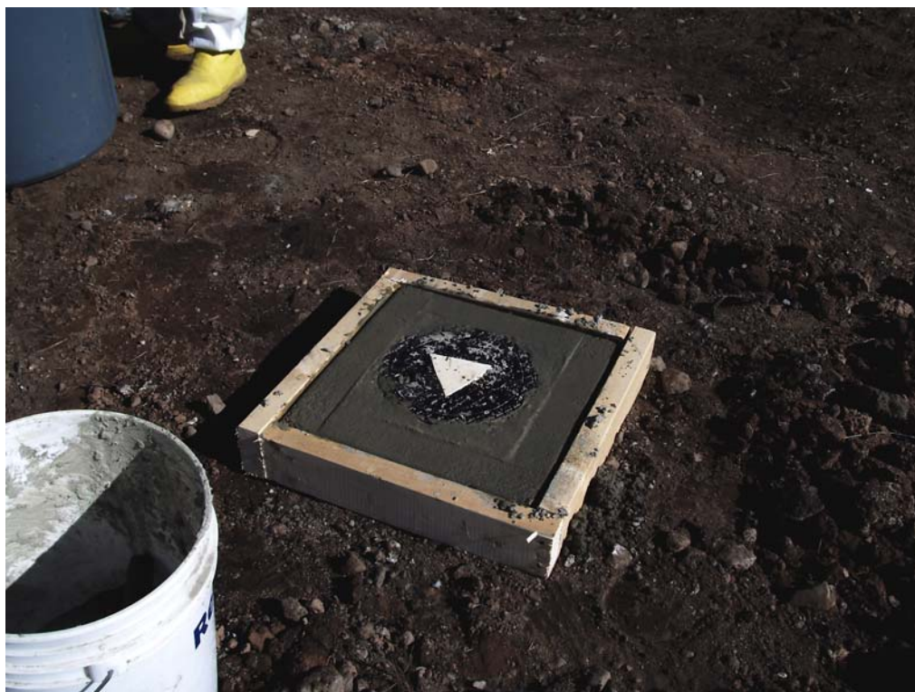
Photograph 6. 8 October 2010. Completion of well PO-1.
