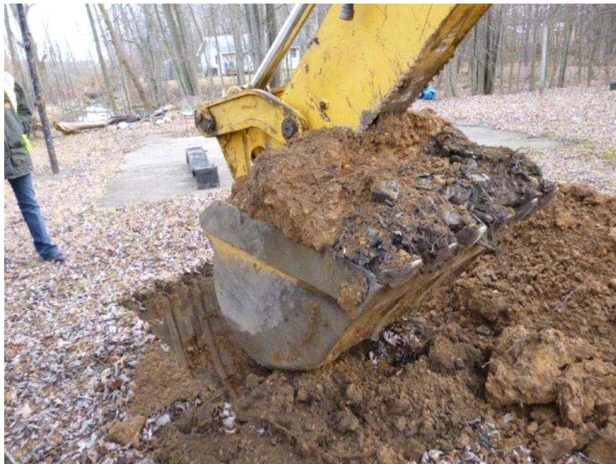
Photograph No.: 6 Photographer: Naren Babu Orientation: Northeast TDD Number: TO-01-11-11-0028 Contract: EP-S5-10-10, OTIE Date: 12/20/2011 Site Name & Location: Lovers Lane Site, Kent County, Michigan. Subject: View of broken lead-acid battery casings and soil in the bucket excavated from Test Pit #2.
