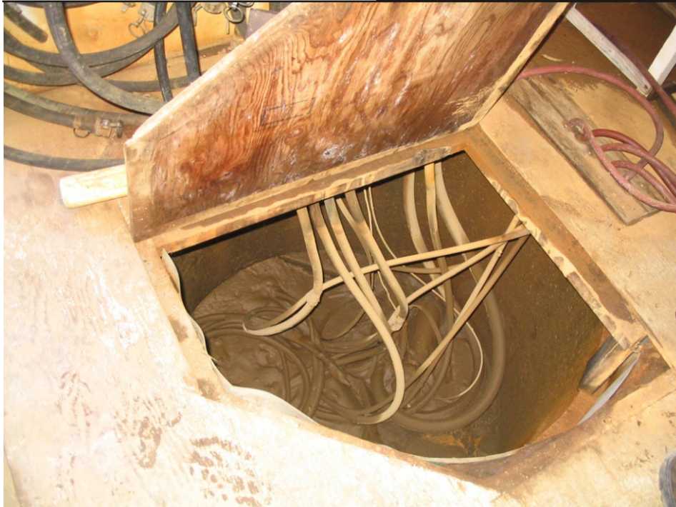
Photo 14 Plumbing sump underneath treatment shed. Direction: Northeast
