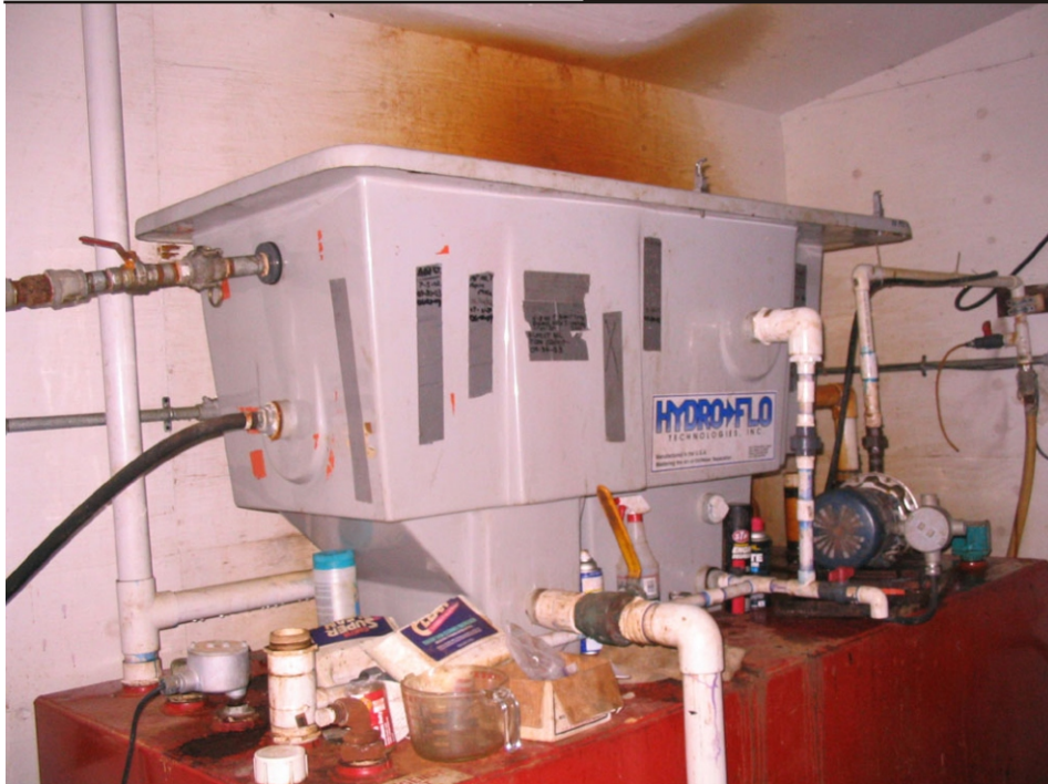
Photo 12 Oil / water separator inside treatment shed. Direction: Southeast
