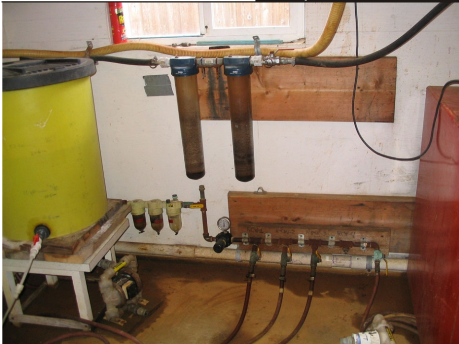
Photo 16 Chlorine injection (yellow tank) and compressed air distribution system for groundwater recovery pumps. Direction: East
