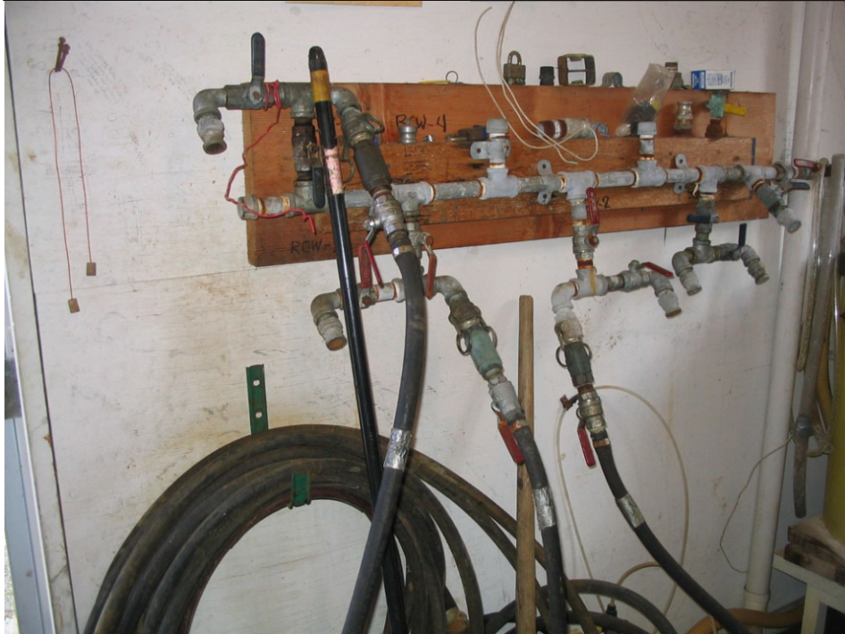
Photo 15 Manifold for groundwater influent from recovery wells. Direction: Northeast
