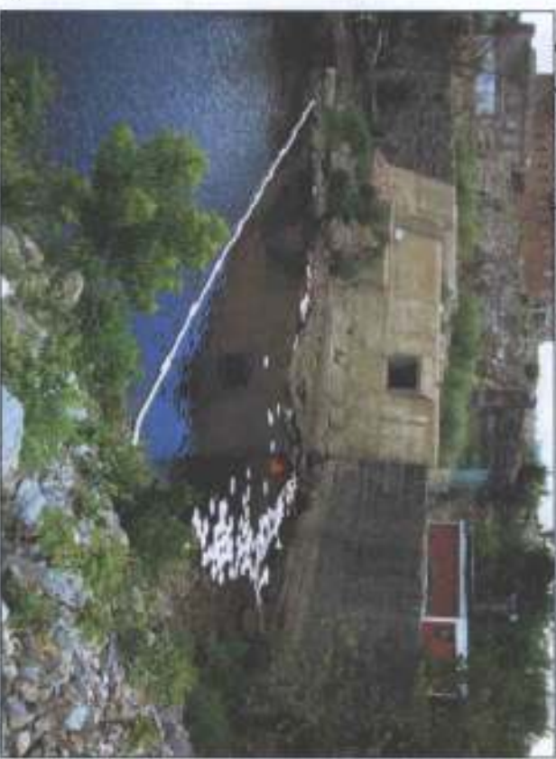
15. Wed, 7/13/11: EPI worker power hot-washing the rocks and retaining wall with the freed oil caught by the sorbent pads and boom.
