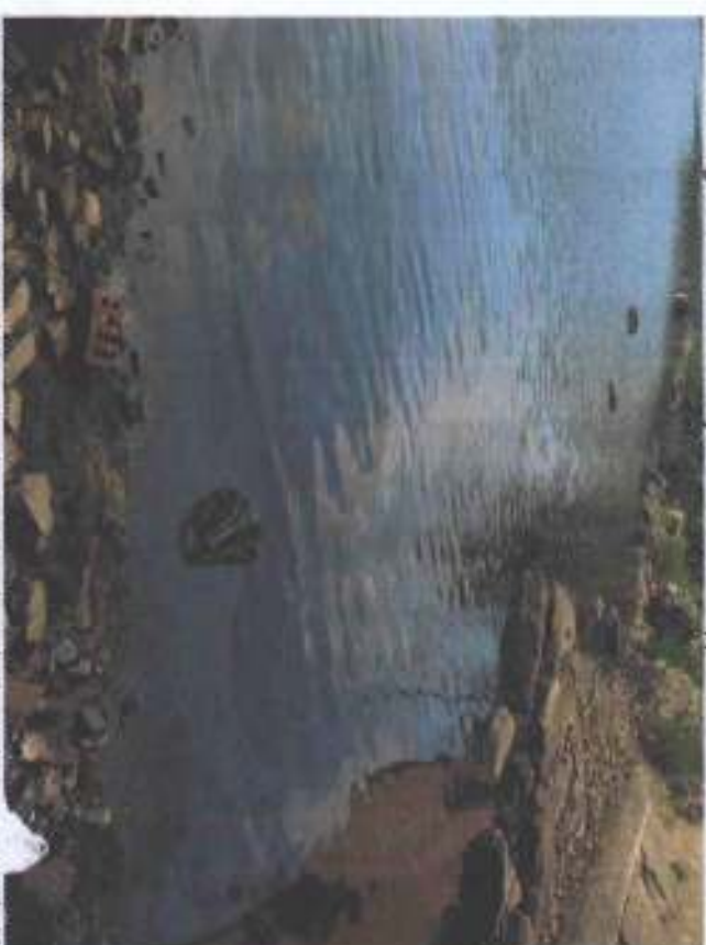
3. Tues. 7/12/11: the 1.5' high smear (bathtub ring) of black oil up the side of the retaining wall from fluctuating water level. A 15" clay drain outlet is at upper left.
