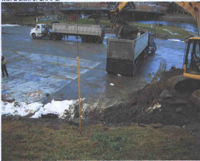
42. oil contaminated soil for transport to CPRC Group in Scarborough, ME..
