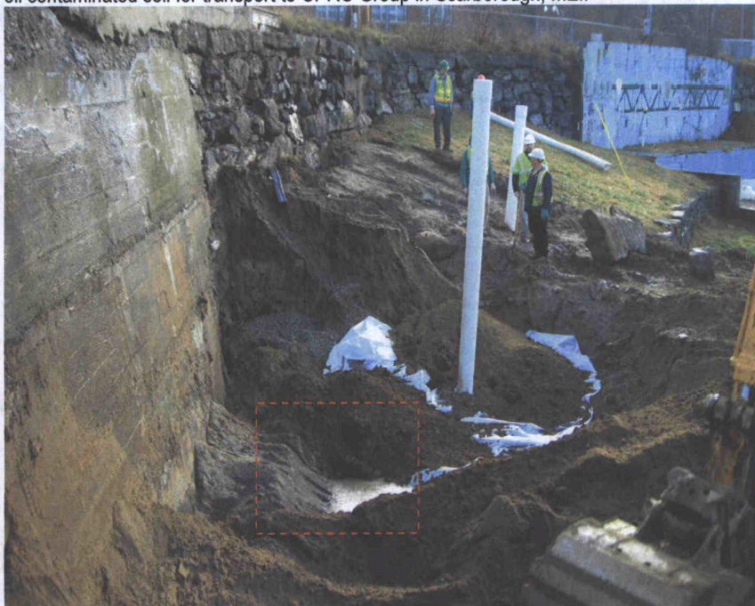
43. and MW-1 with Mill Street at the left and the CMP substation building in the far background. The SE end of TP-11 lies open; the concrete cradle for the former UST is within the dashed box. In the background the blue concrete platform is part of the former Columbia Mill building. The crushed stone around MW-2 is covered with poly and is being covered by sand clean fill.
