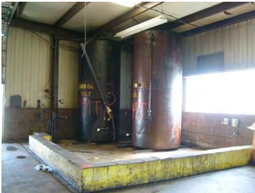
Photo No. 8: View of the two 1,750-gallon used oil ASTs located in the storage area.
