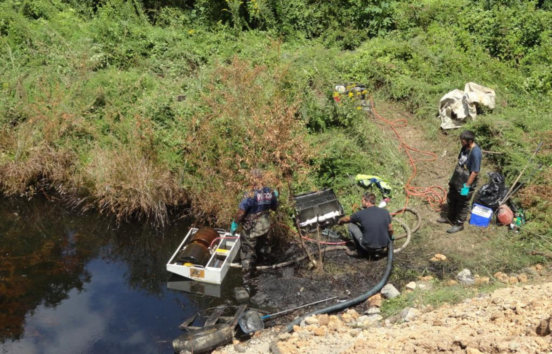
Photo of skimming operations at the eastern end of the retention pond. The retention pond runs east to west along the northern eastern portion of the property.
