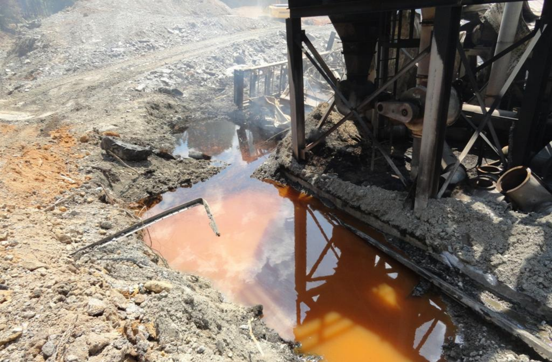
Collection Point 2 at the rear of the facility structure. Water is orange in color with oil weeping from the southern wall of the pit.
