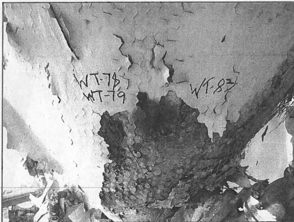
Water Treatment Plant – Exterior ACM Hot Water Storage Tank TSI
