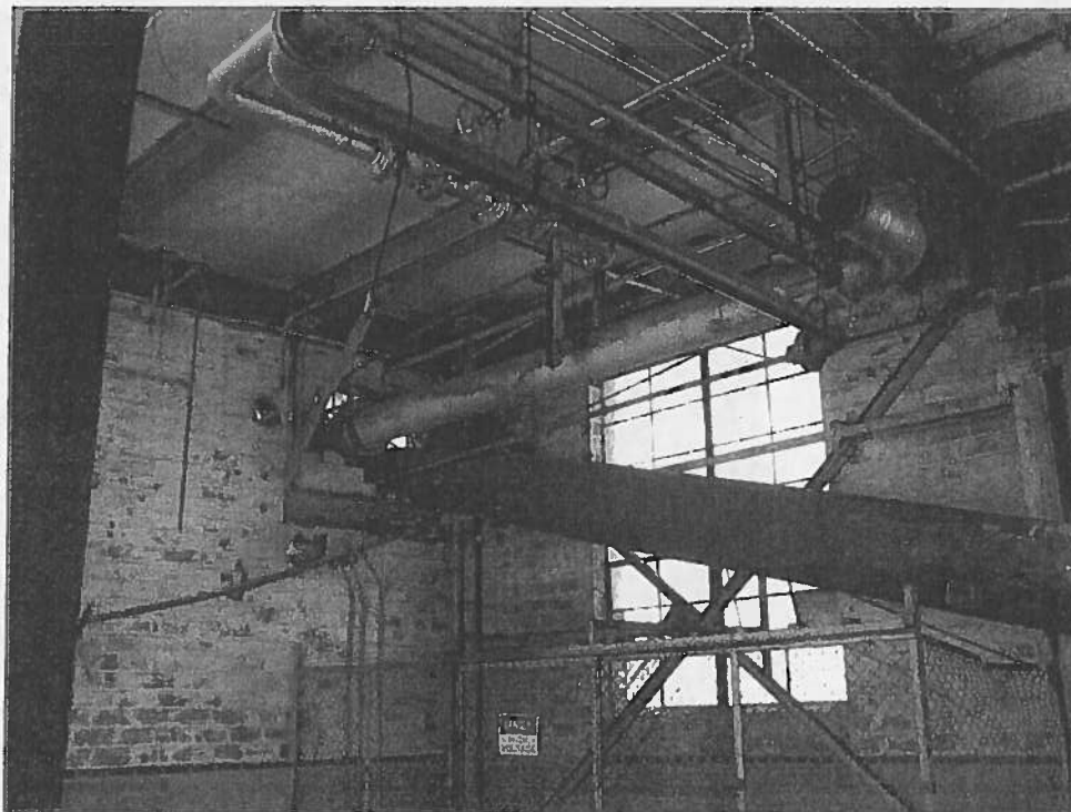
Pump Room Ground Level – Northwest View of ACM Pipe Insulation
