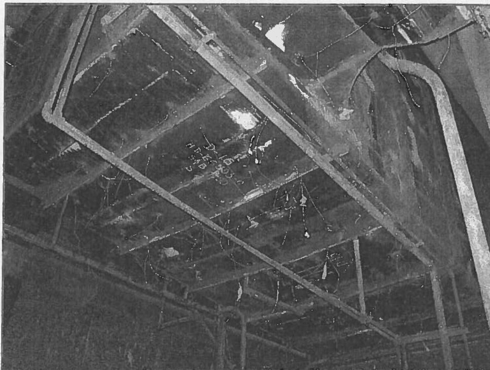
Boiler Room Operating Floor – Air Heater Duct ACM TSI Debris
