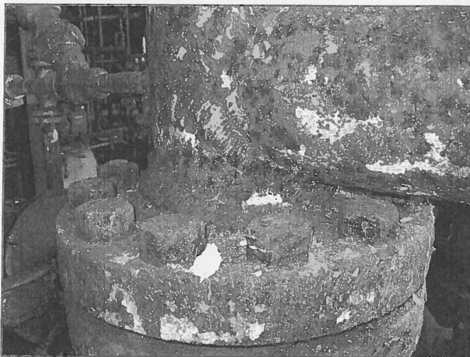
Boiler Room Operating Floor – Steam Header ACM TSI Debris
