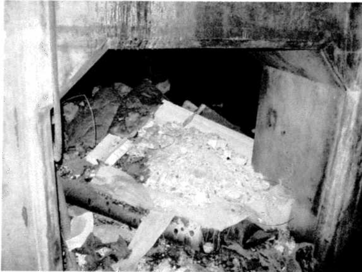
7495-31 In the turbine building basement under the north turbine room. The raised platform for the pit has asbestos debris piled under it. Sample # 159 was taken in this location.
