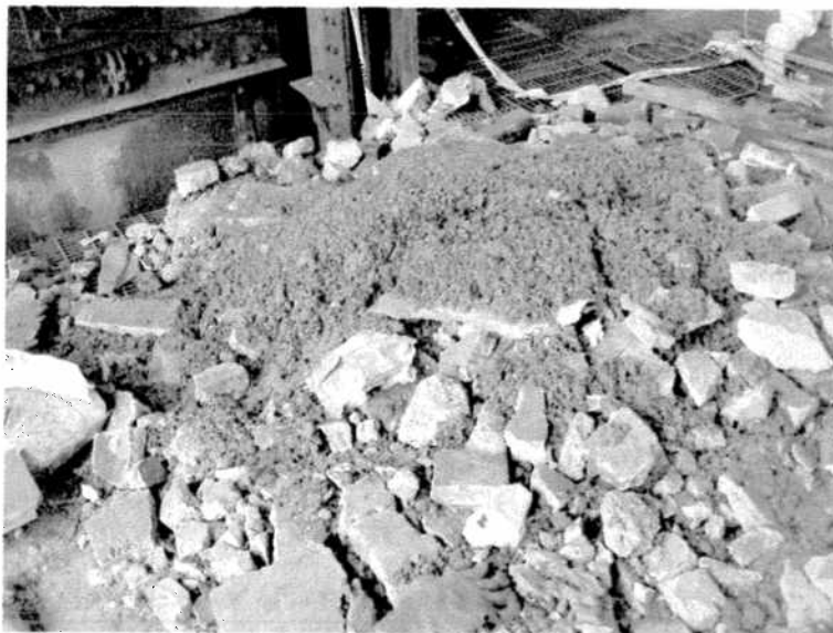
7495-16 In the boiler building near boiler #2 on the east side showing asbestos containing debris pile.
