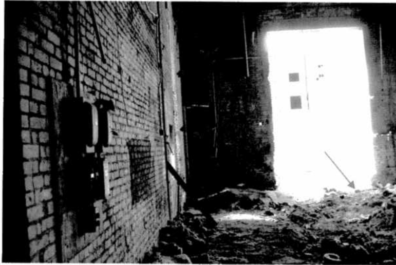
7495-03 After entering and climbing the stairs to the main floor looking south toward a former roll-up door which is missing leaving the floor open to the outside environment. Notice the asbestos containing debris on the floor.
