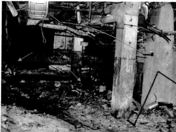
7495-28 The basement of the turbine building looking south from the north wall of the main room. The floor is completely covered with asbestos containing debris from piping above. Several piles of debris have asbestos stickers in them.
