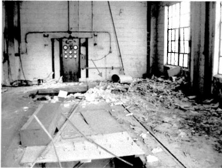
7495-09 Looking west from the north turbine room roll-up door . Notice the asbestos contaminated debris field in the picture. The half covered open pit has allowed some material to fall to the basement also hiding hidden open holes to the floor below.
