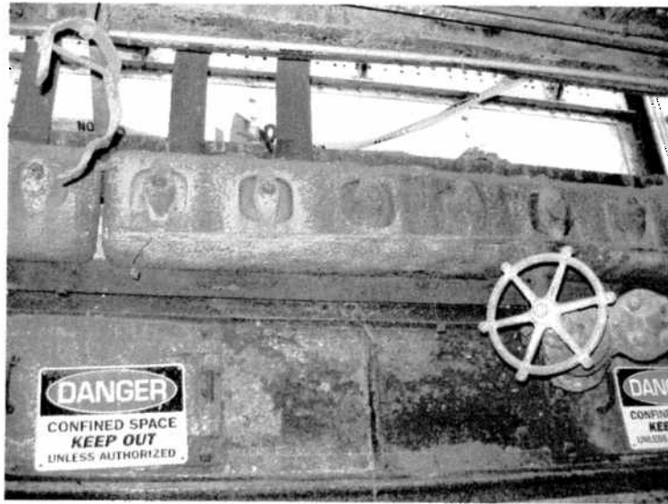
7495-25 In the basement of the Boiler building looking at the Boiler #1 base. Ports are missing asbestos insulation present on boiler #2.
