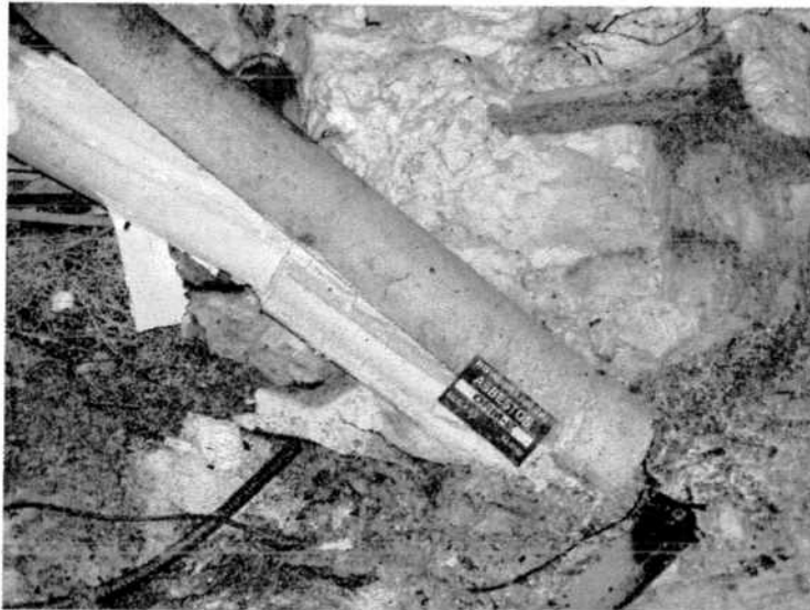
7495-32 This is another picture of debris on the floor of the turbine building basement clearly showing an asbestos label still on the insulation.
