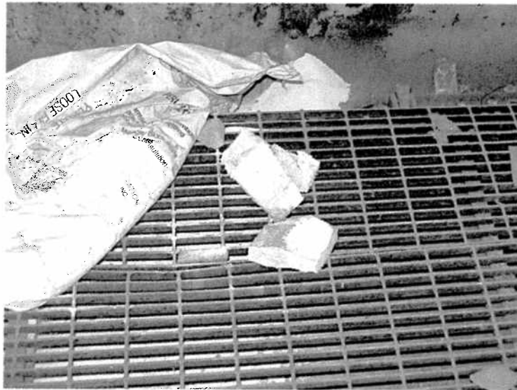
7495-13 In the boiler building by the boiler #2 on the north side asbestos insulation from the wrapped pipes above has fallen down.
