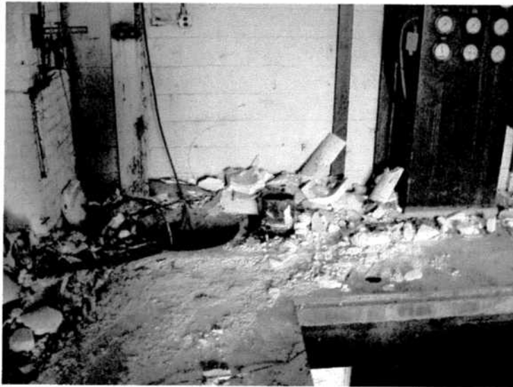
7495-11 Looking east on the south side of the pit in the north room of the turbine building on the main floor. The debris pile is asbestos containing waste material.
