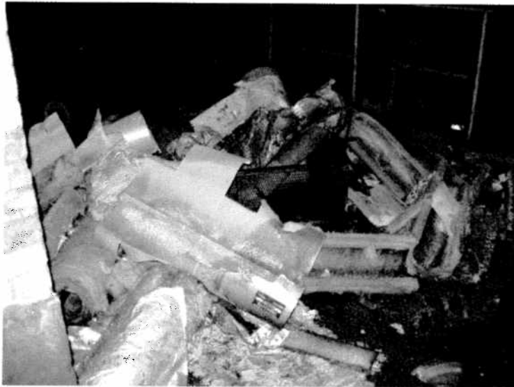
7495-33 This is another debris pile in the turbine building basement with a mix of insulation materials some of which are asbestos containing.
