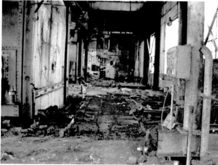
7495-05 On the main floor of the boiler building looking east. Notice the damaged grating on the floor. There are numerous open holes and damaged grating throughout floor area.
