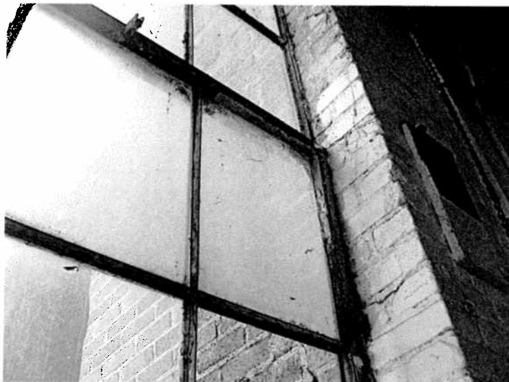
7495-35 This is a picture of the window putty in the turbine building main floor main room. The window putty sample # 136 is asbestos containing and damaged.
