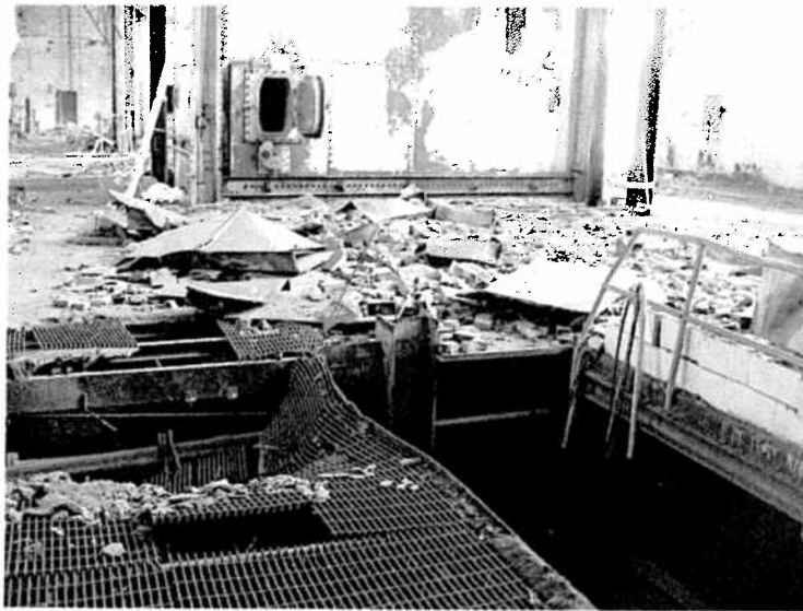
7495-37 This picture shows a closer look at some of the damaged grating within the boiler buildings main floor area.
