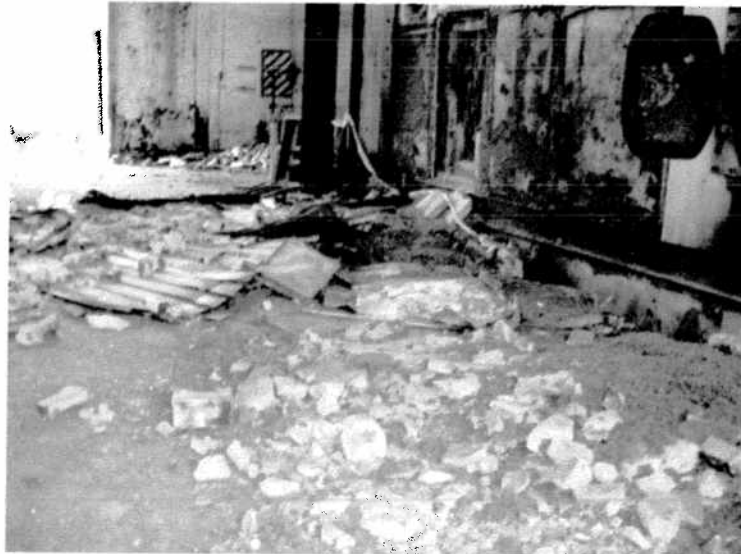
7495-18 On the main floor in the boiler building the piles of debris are positive for asbestos.
