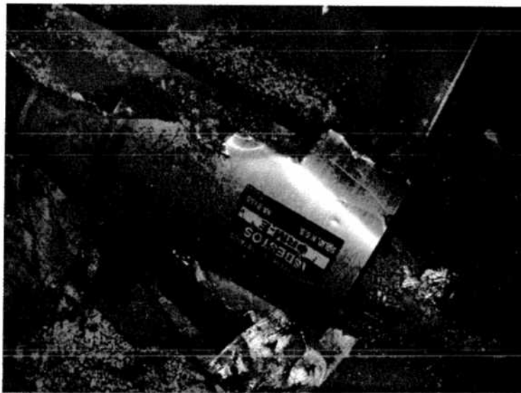
7495-34 This is a close-up of the picture 7495-31 showing another asbestos label on insulating materials that was torn off.
