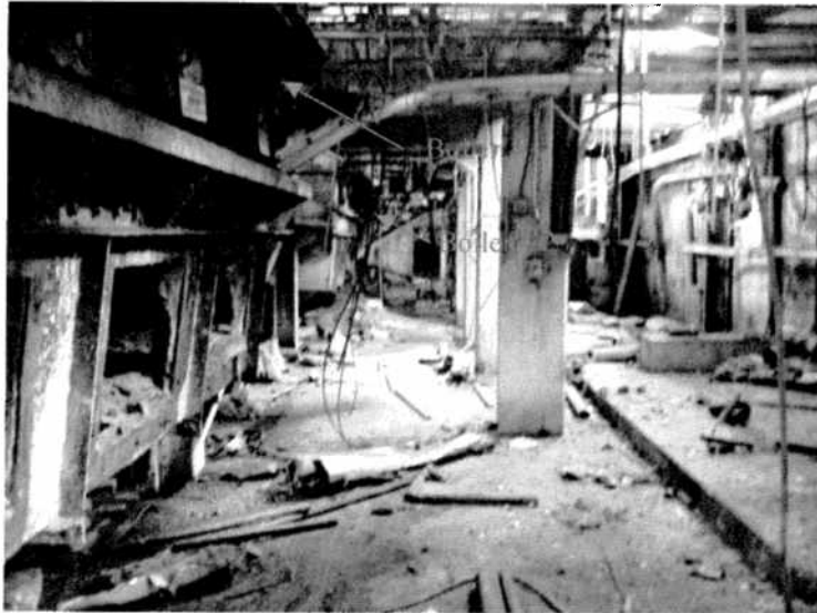
7495-19 In the basement of the boiler building looking west on the north side. The boiler drums insulation is asbestos containing and is still installed on boiler #2 and the asbestos is exposed and damaged.. In boiler #1 the panels are off and the asbestos is missing.
