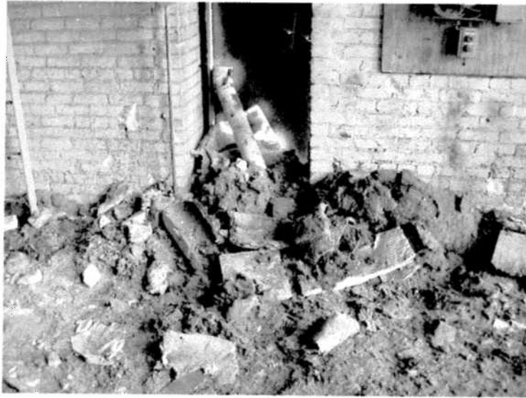
7495-17 On the main floor in the boiler building where samples 102 & 103 in the debris pile were taken and are positive for asbestos.
