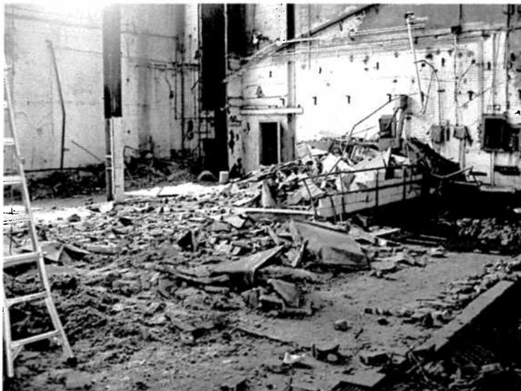
7495-07 On the main floor looking south west. More asbestos contaminated debris west of Boiler number 2.
