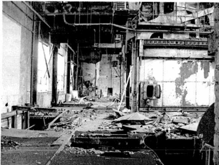
7495-06 On the main floor looking west. Notice the damaged grating on the floor. There are numerous open holes and damaged grating throughout floor area.
