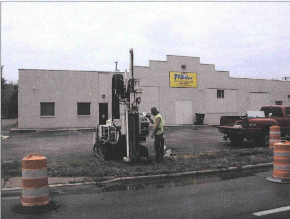
Photo 6: Installation of soil gas probes using a GeoProbe unit
