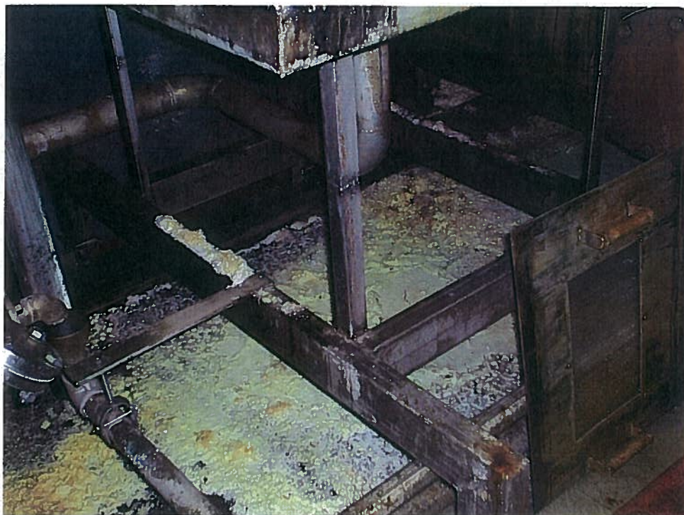
Photograph 9: Composite sample location 5 (BM-SW-05), crystal-like material located inside the process line.
