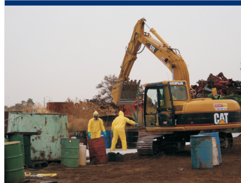
Photo 24 ERRS finding and consolidating drums on visqueen.
