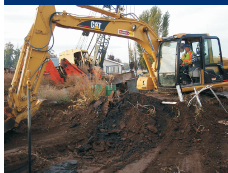
Photo 48 Excavating lead contaminated soil.
