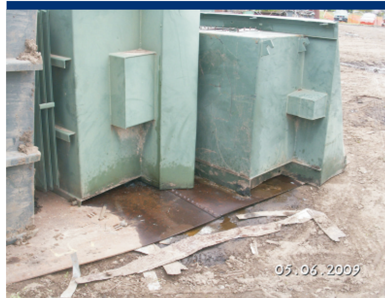
Photo 17 Leaking transformers.
