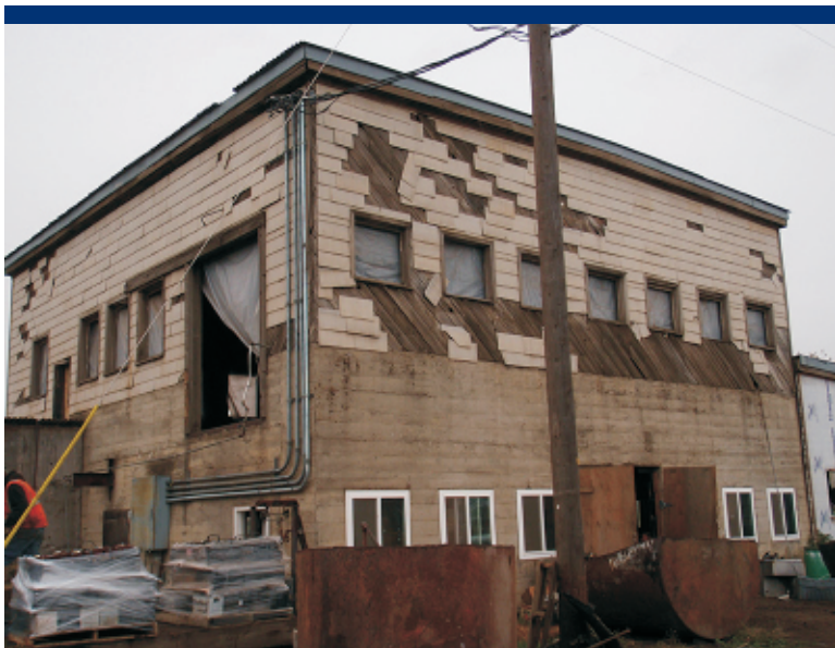
Photo 33 Shop building with ACM siding.
