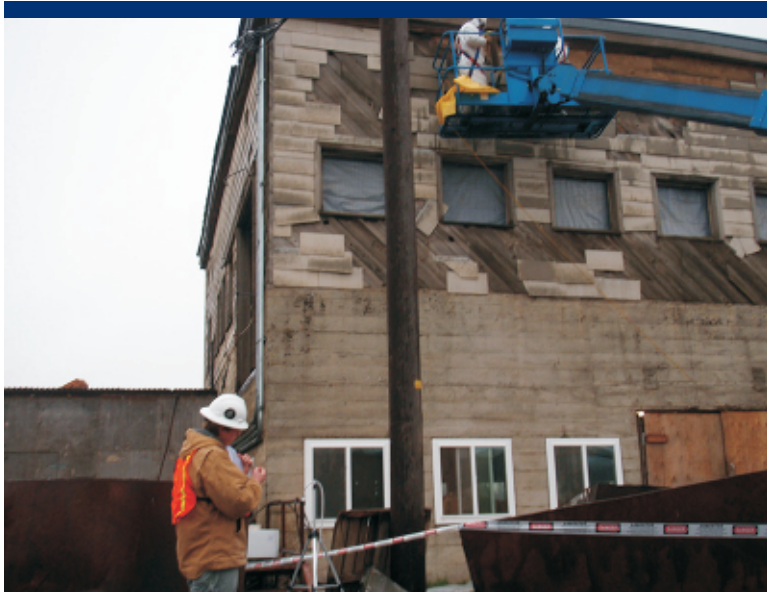
Photo 35 Asbestos abatement crew removing ACM siding from shop building.
