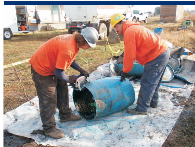
Photo 30 ERRS cutting up drums for disposal.
