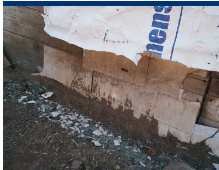
Photo 14 Friable ACM on the ground at the shop building.
