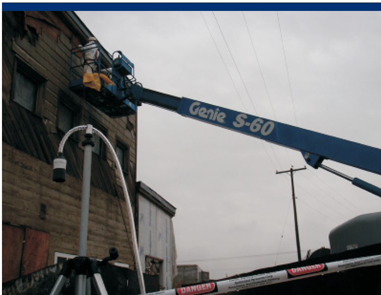
Photo 37 Asbestos abatement crew removing ACM siding from shop building.
