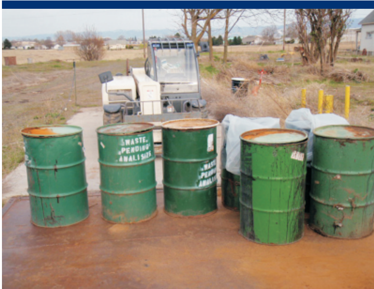
Photo 59 Drums staged on the scale for overpacking.
