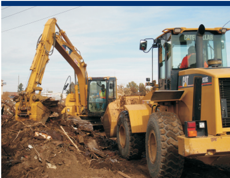
Photo 41 Placing ACM in the loader for transportation to the roll off containers.
