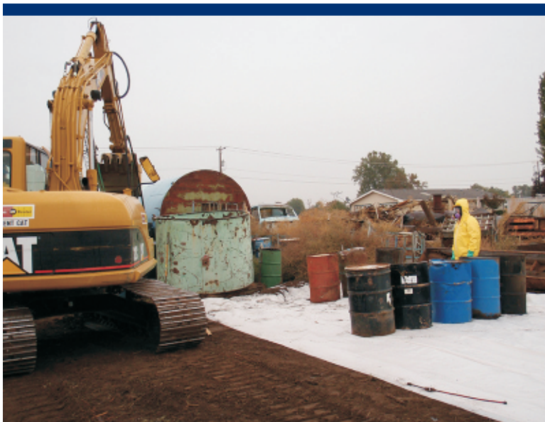
Photo 25 ERRS finding and consolidating drums on visqueen.
