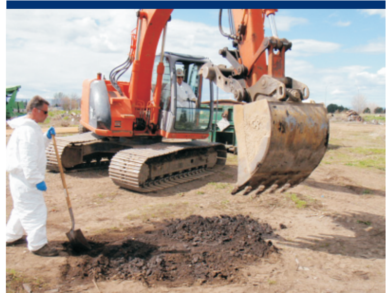
Photo 71 Excavating stained soil near the shop building.
