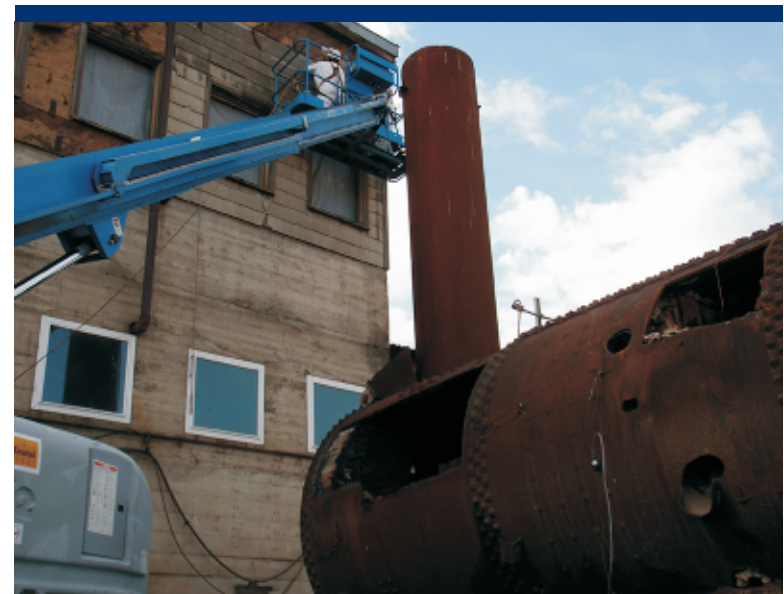
Photo 38 Asbestos abatement crew removing ACM siding from shop building.
