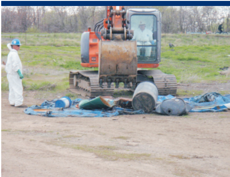
Photo 68 ERRS crushing empty drums prior to disposal.
