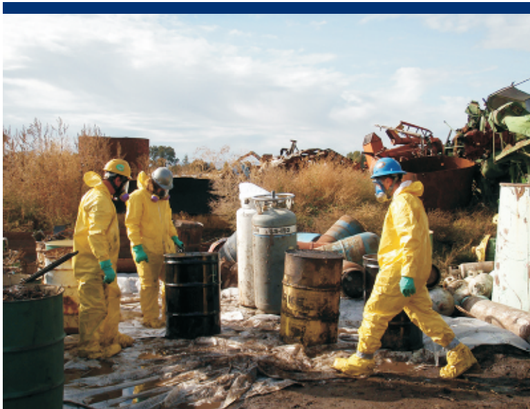
Photo 29 ERRS consolidating like materials in drums.
