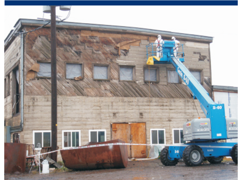
Photo 36 Asbestos abatement crew removing ACM siding from shop building.
