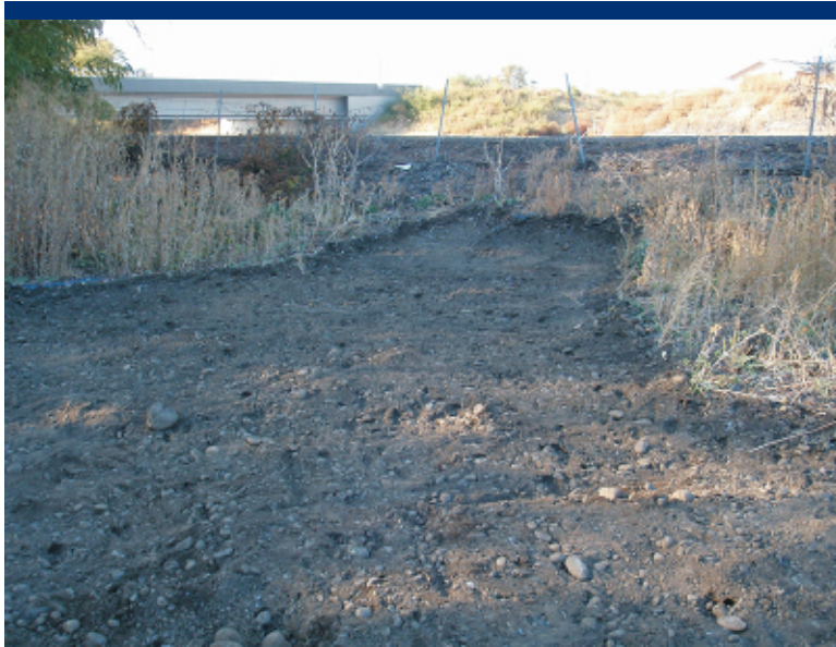
Photo 51 Excavation of surface soil at the swale.
