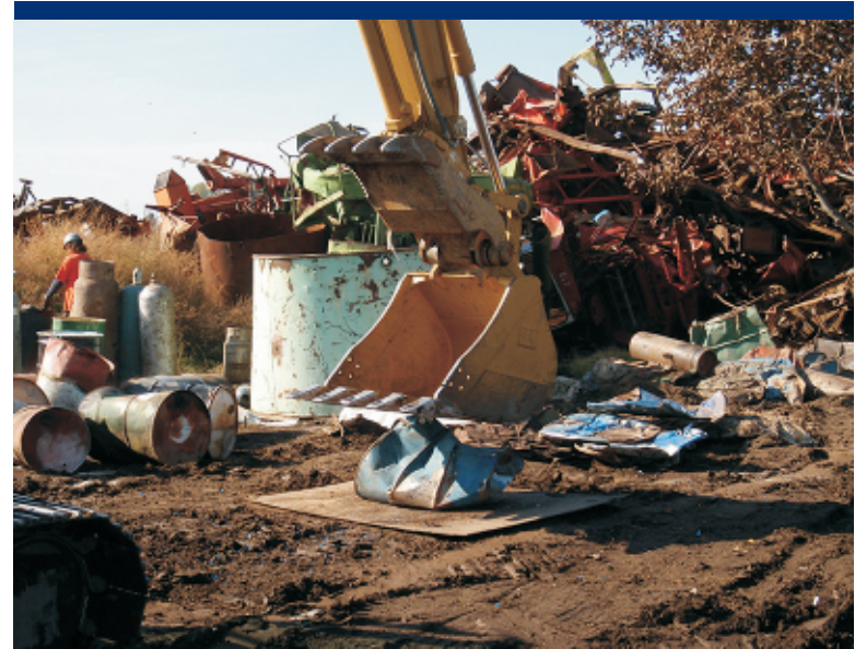
Photo 32 ERRS crushing drums for disposal.
