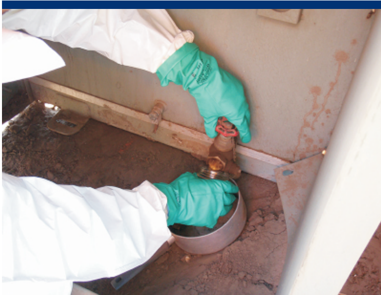
Photo 19 Sampling transformer oil.
