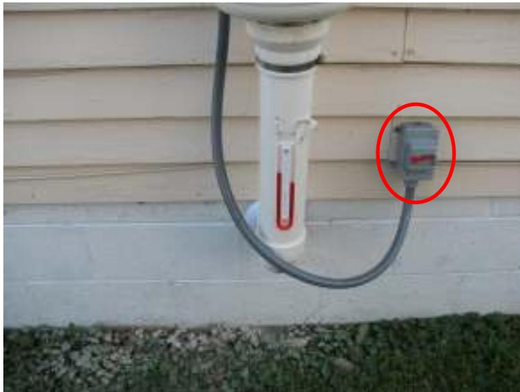
Close-up of the “On/Off” switch located on the exterior of the building. The system is designed to run in the “On” position at all times to ensure it is effective.
