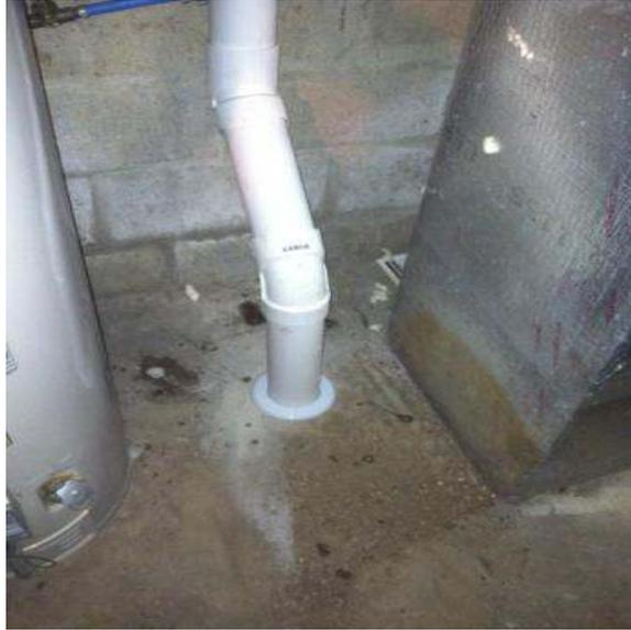
The sub-slab vapor extraction points. PVC piping extends below the concrete slab or crawlspace liner. PVC piping extends upward to an overhead piping system routed to an “in-line” fan located on the exterior of the building.
