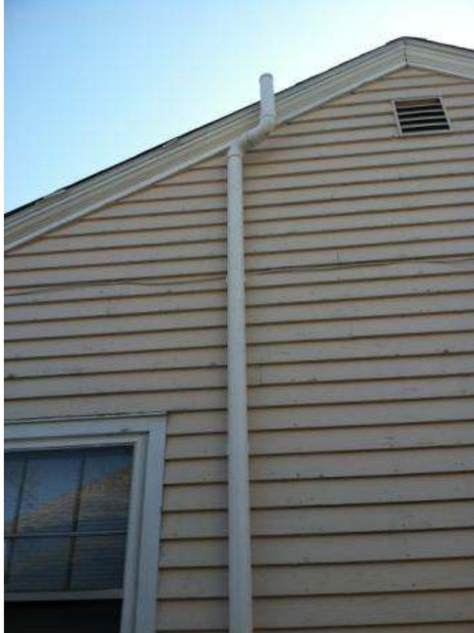
The effluent vent (exhaust) for the system. The vapors are vented above the roof of your building. The vent pipe must be clear of obstructions at all times. This includes caps and covers.
