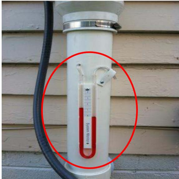
Photo showing the “U-Tube” manometer (vacuum pressure gauge). The U-Tube will display a reading greater than zero (0 inches of water column) on the side where the poly tubing is located when the system is operating effectively.
