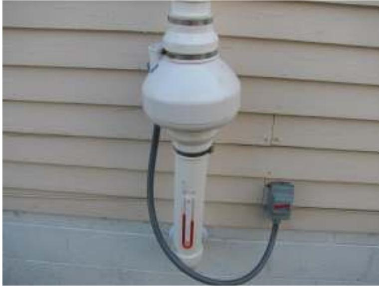
Fan portion of the vapor mitigation system. The fan creates a vacuum under the concrete slab floor or crawlspace. The vacuum draws vapors from under your home and into a PVC pipe system that is vented above the structure. The fan must be “On” and running 24 hours per day to ensure that it is operating effectively.
