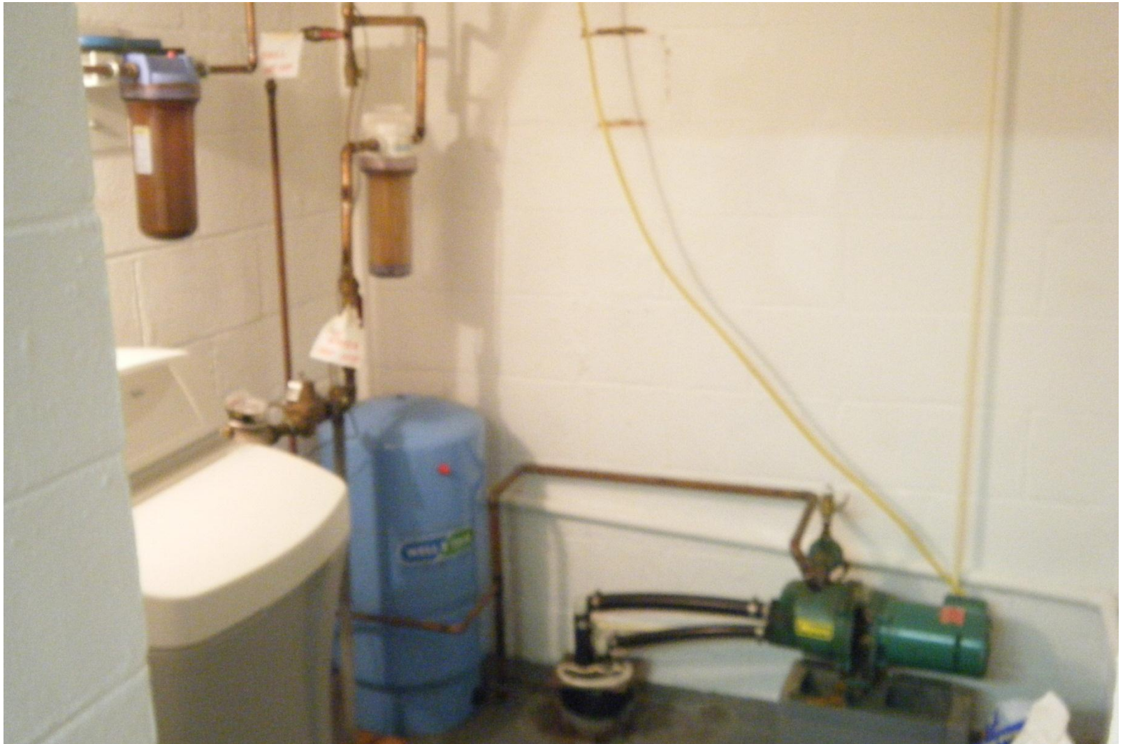
Photograph 13: Well water system in basement: location GW10
