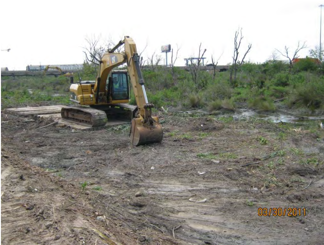
Photo 4 – Clearing surface grasses in the west cell in preparation for deploying geotextile and geomembrane.
