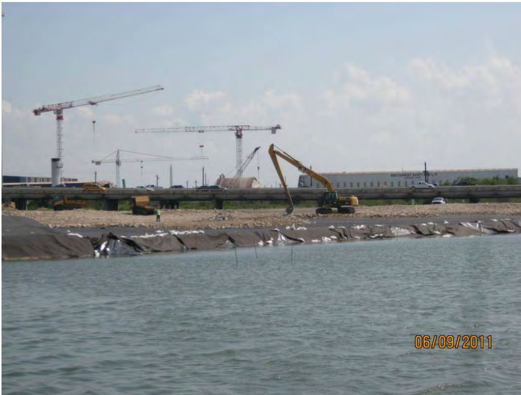
Photo 1 – Placing Armor Cap B/C rock in the Western Cell.
