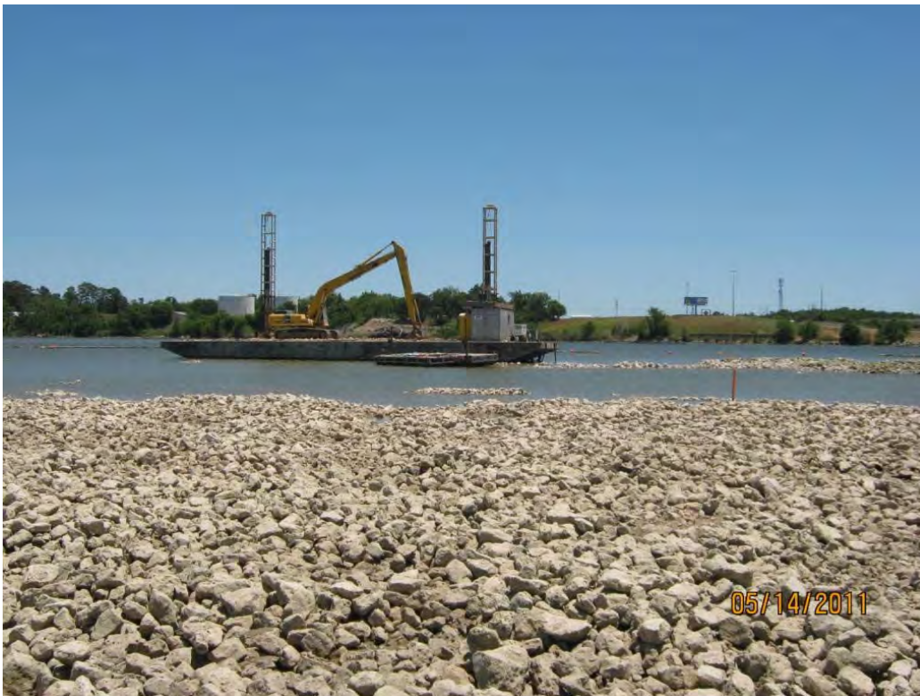
Photo 5 – Armor Cap C rock above the water surface in the Eastern Cell during a low tide caused by north winds.
