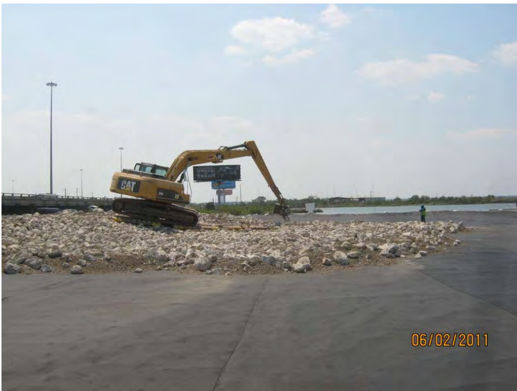
Photo 6 – Long-reach excavator placing Armor Cap B/C rock in the Western Cell.
