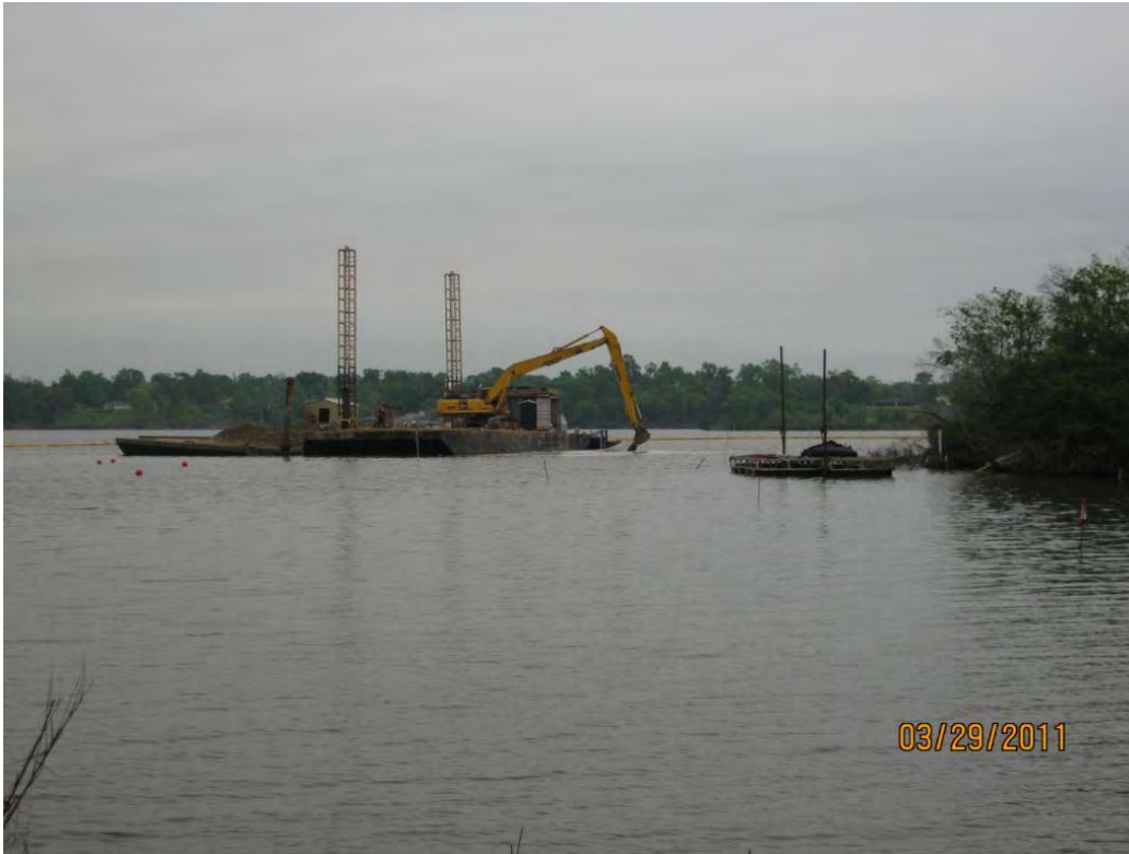
Photo 2 – Water-based operations placing Armor Cap A rock in the northwestern area.
