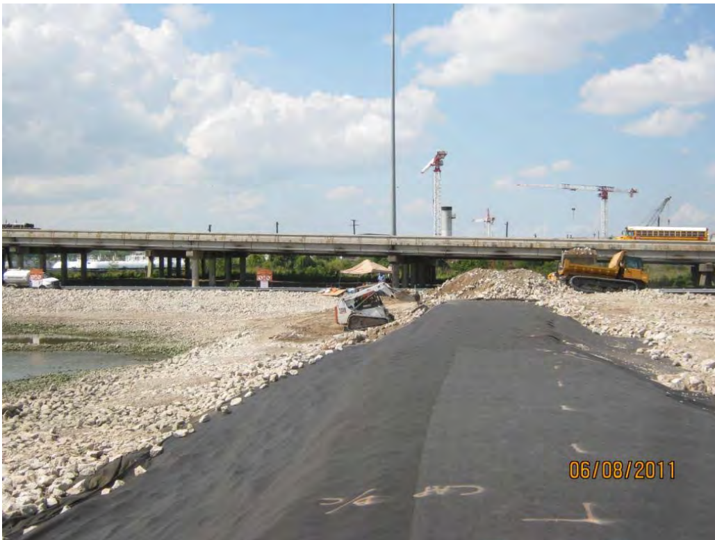
Photo 2 – Placing Armor Cap B/C rock adjacent to the central berm.
