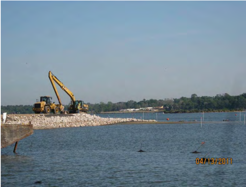
Photo 1 – Placing Armor Cap D rock to the east of the central berm.
