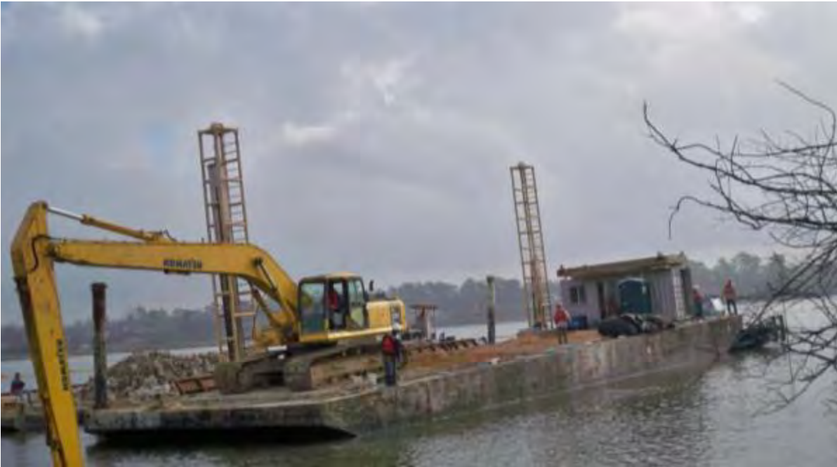
Photo 1 – Deploying geotextile and placing Armor Cap D rock in the east cell near the northern end of the central berm.
