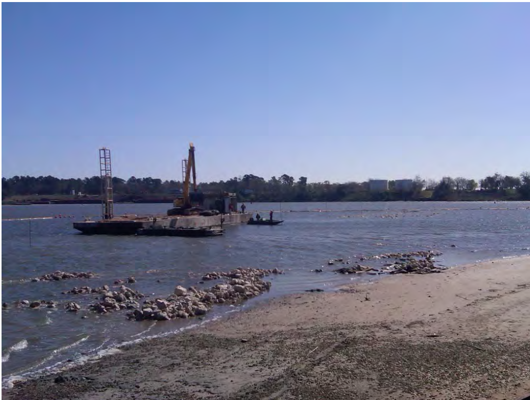
Photo 2 – Armor Cap D rock in the east cell during a low tide caused by north winds
