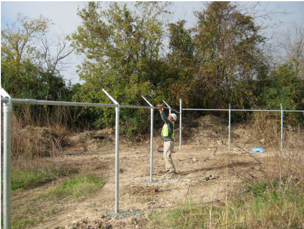
Photo 2 – Installing top post for 6-foot chain link fence at location along west edge of Big Star property.
