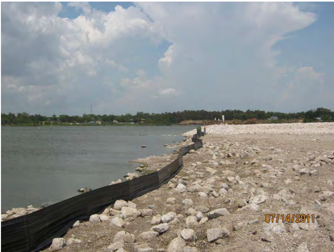
Photo 4 – Installing a silt fence at the north end of the Western Cell.
