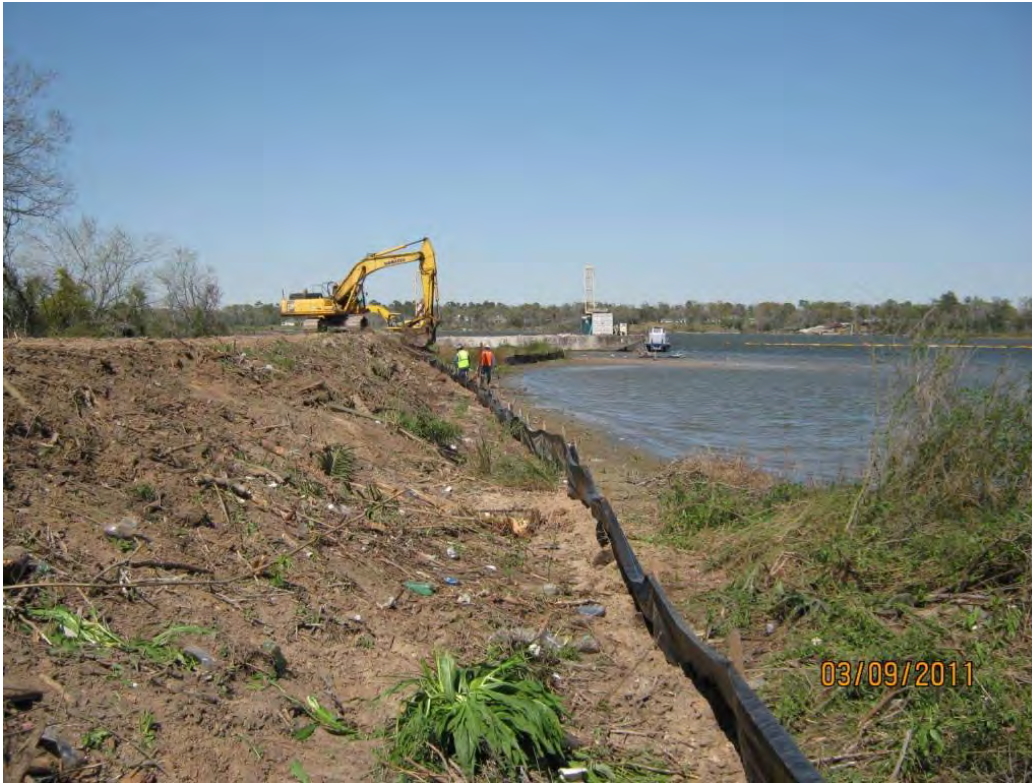
Photo 5 – Silt fence installed along the east side of the central berm
