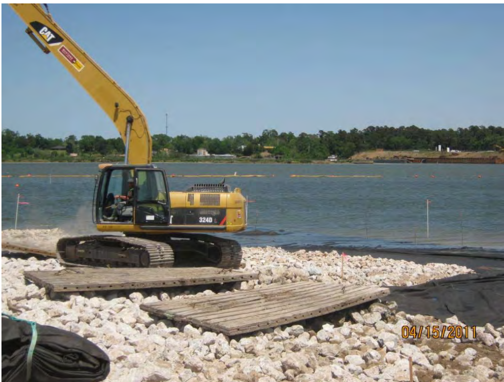
Photo 2 – Placing Armor Cap C rock in the east cell near the north end of the central berm.
