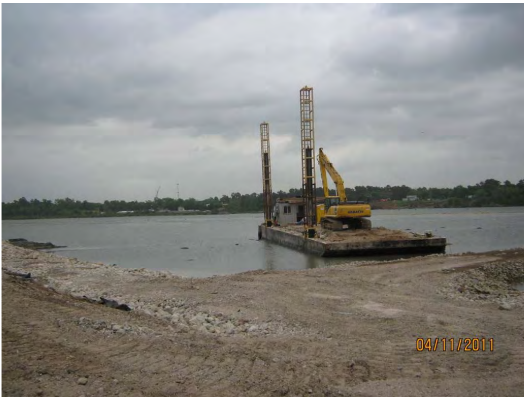
Photo 3 – Barge-mounted excavator idle in the east cell due to low tide conditions caused by a storm front and the resulting north winds, which prevented delivery of rock by the aggregate transport barge.
