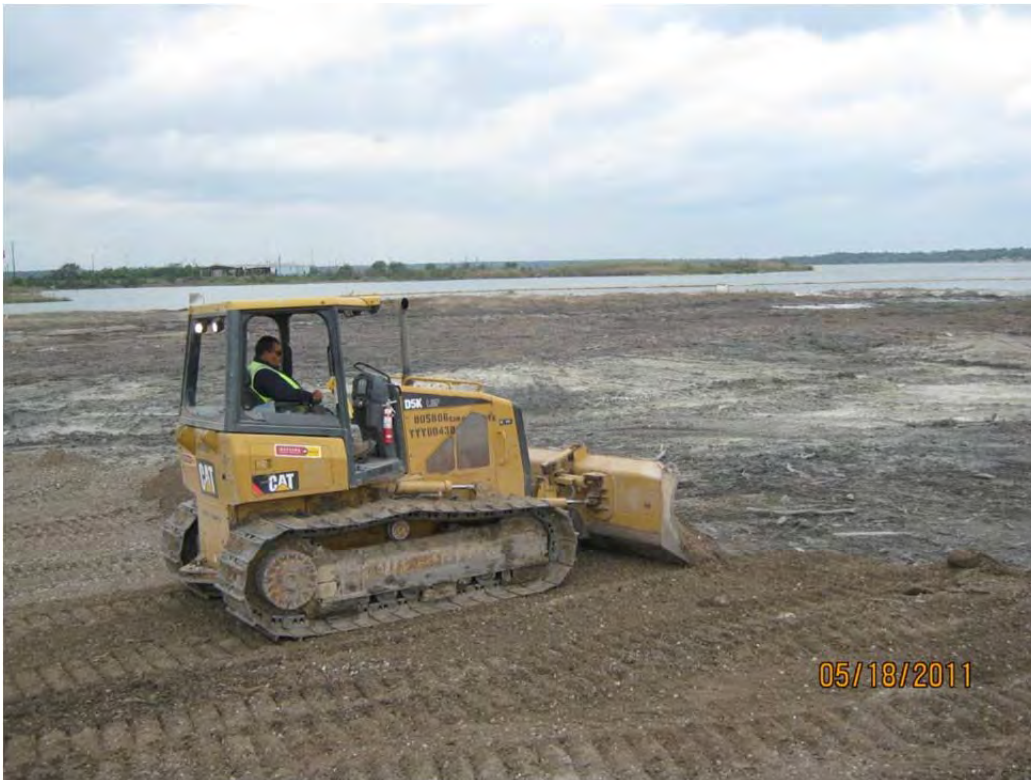
Photo 3 – Dozer spreading crushed concrete road base in the Western Cell to create a smoothly-graded surface.
