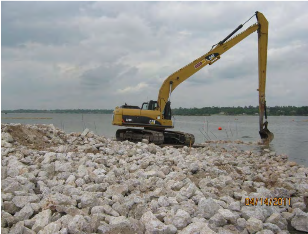
Photo 1 – Placing Armor Cap D rock at the north end of the central berm.
