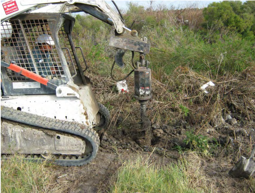
Photo 1 – Installing fence post hole to the southeast of the east gate of Big Star property using bobcat.
