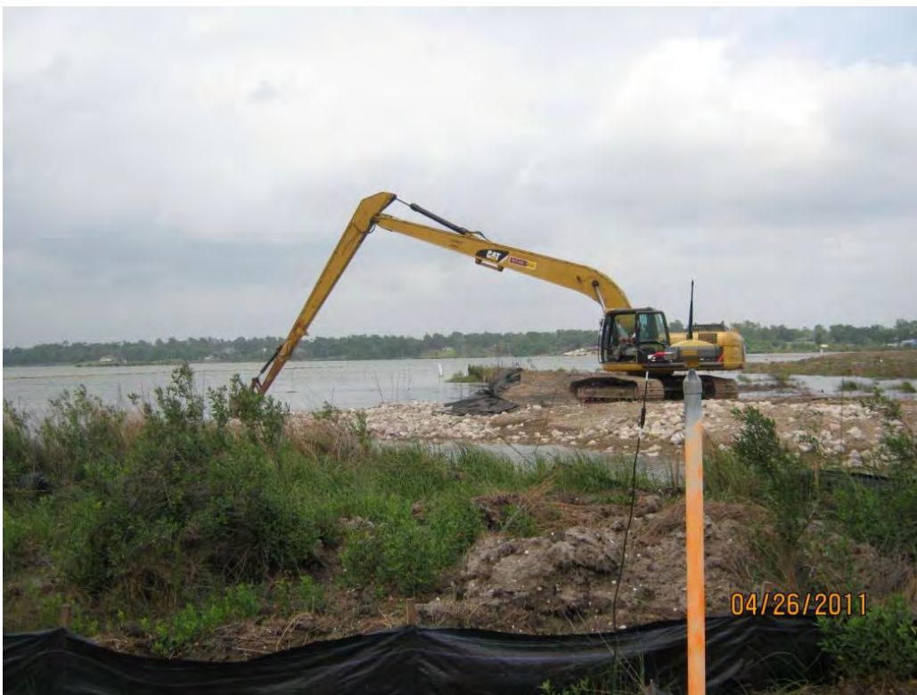
Photo 2 – Placing Armor Cap B/C rock outside the southwest corner of the west cell.
