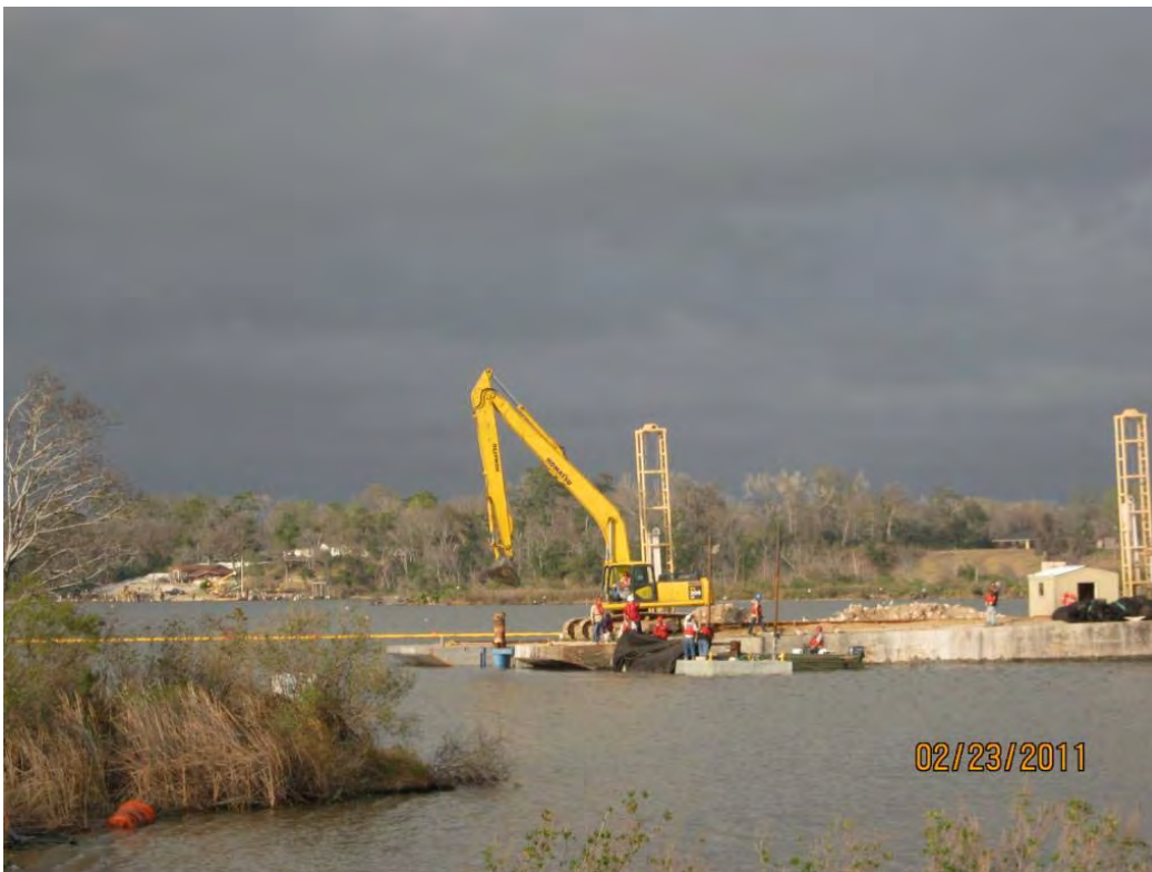
Photo 4 – Repositioning barge to deploy a new section of geotextile in the east cell
