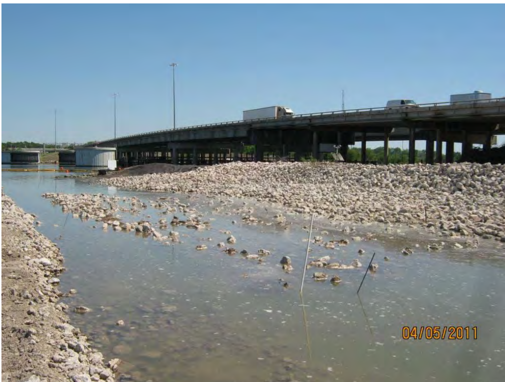
Photo 2 – Armor Cap B/C rock placed in the east cell near the south berm.
