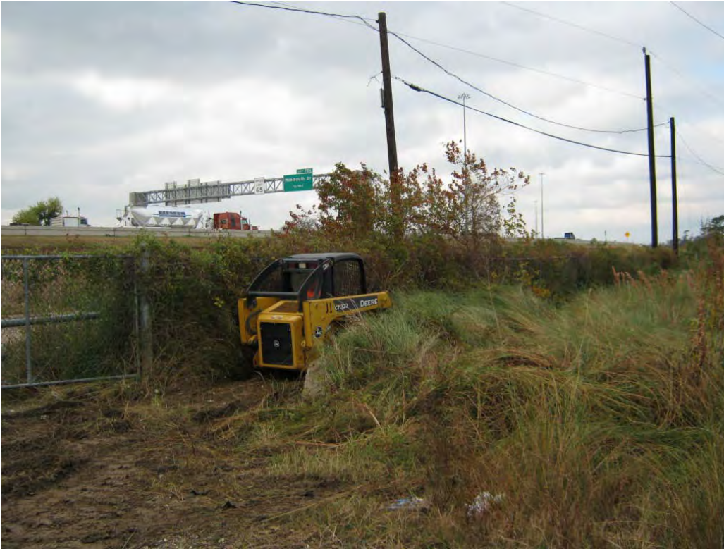
Photo 1 – Clearing vegetation from adjacent to existing fence using bobcat.
