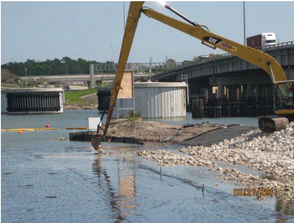
Photo 5 – Placing Armor Cap B/C rock in the east cell using land-based equipment.
