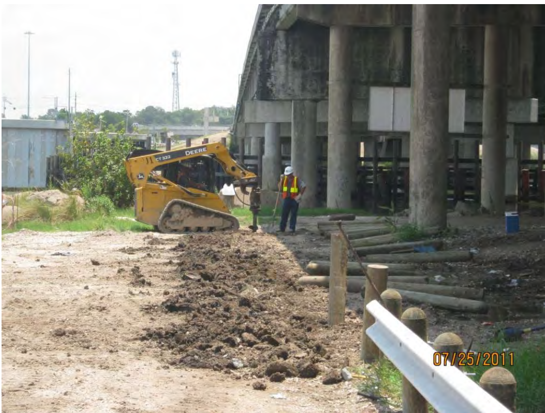
Photo 4 – Digging fence post holes for the remaining 100-foot long section of guardrail.
