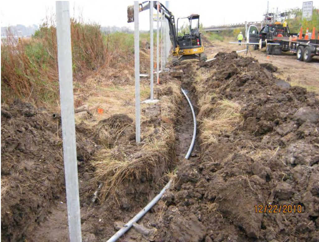
Photo 5 – Traf-Tex repairing power cable to TxDOT camera that overlooks I-10.
