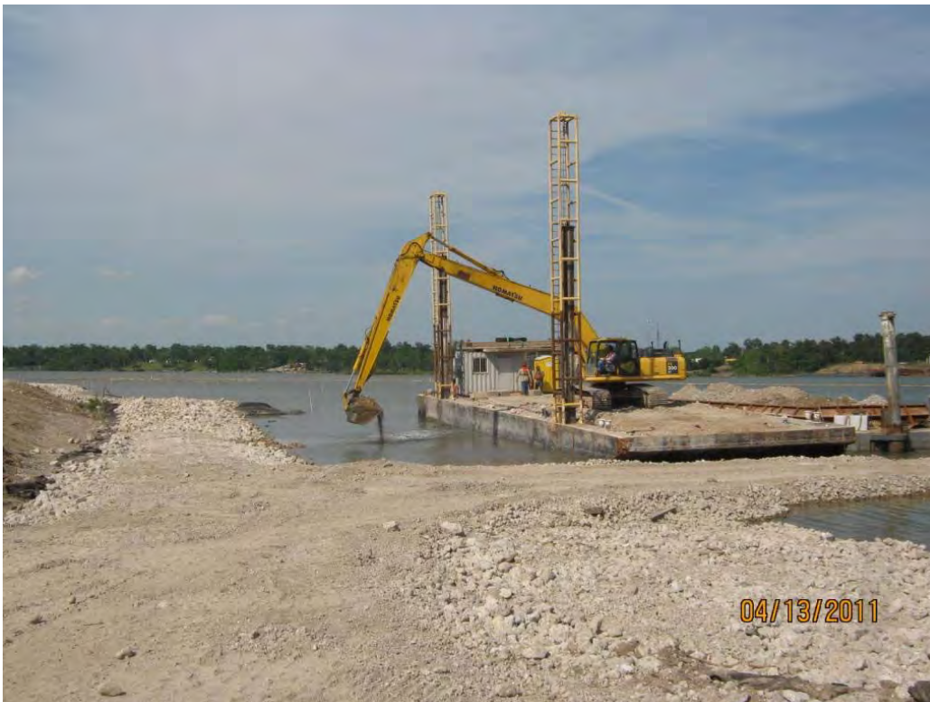
Photo 6 – Barge-mounted operations placing Armor Cap A in the east cell after the tide rose to a level sufficient to permit access by the aggregate transport barge; rock placement began at 16:20 on this date.
