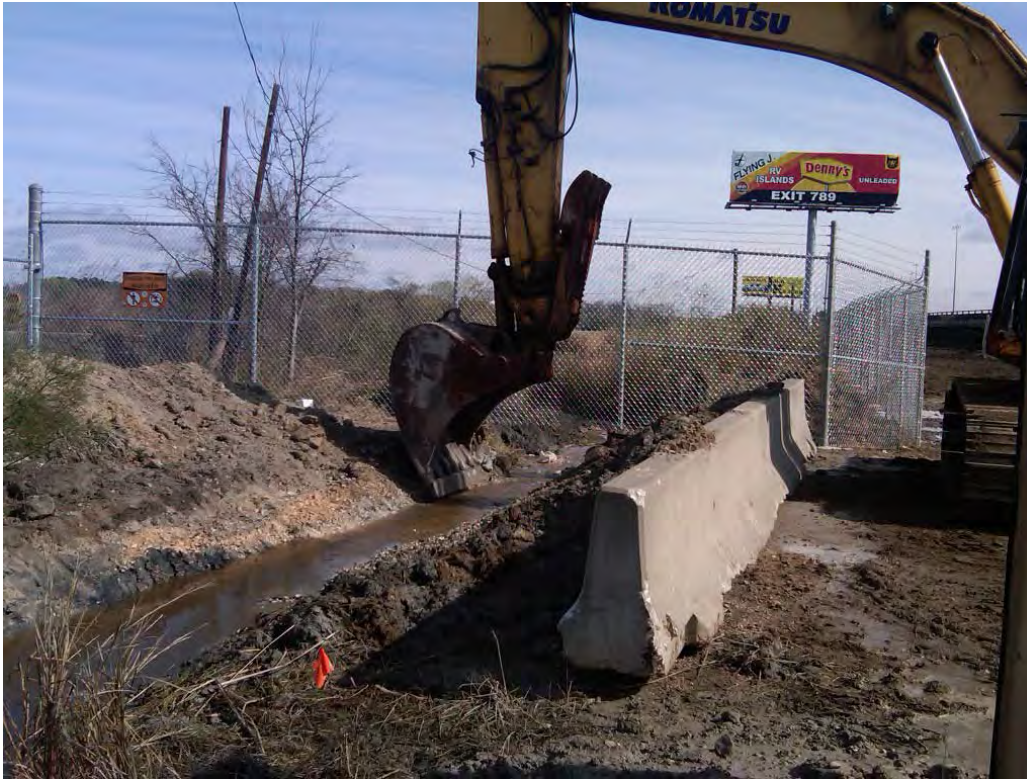
Photo 1 – Improving stormwater drainage along TxDOT ROW adjacent to Big Star property.
