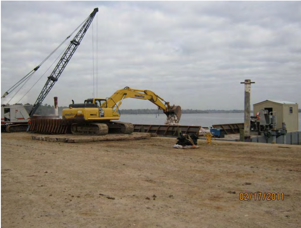
Photo 1 – Loading Armor Cap D rock onto aggregate transport barge at LaBarge Property
