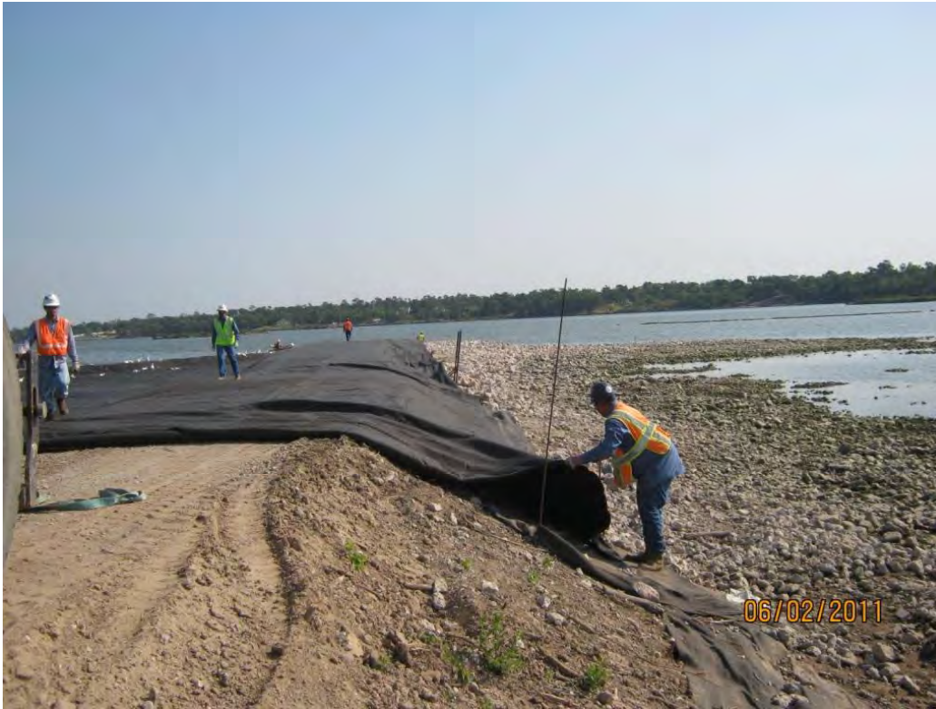
Photo 1 – Deploying geotextile over the top of the central berm and overlapping the adjacent geotextile.
