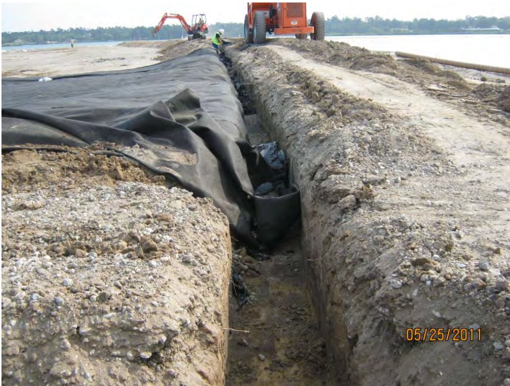
Photo 4 – Eastern edge of the geotextile panels placed in the anchor trench along the central berm.
