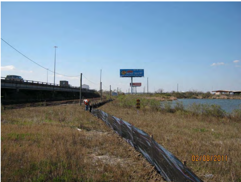
Photo 4 – Installing silt fence along north side of TxDOT ROW Property
