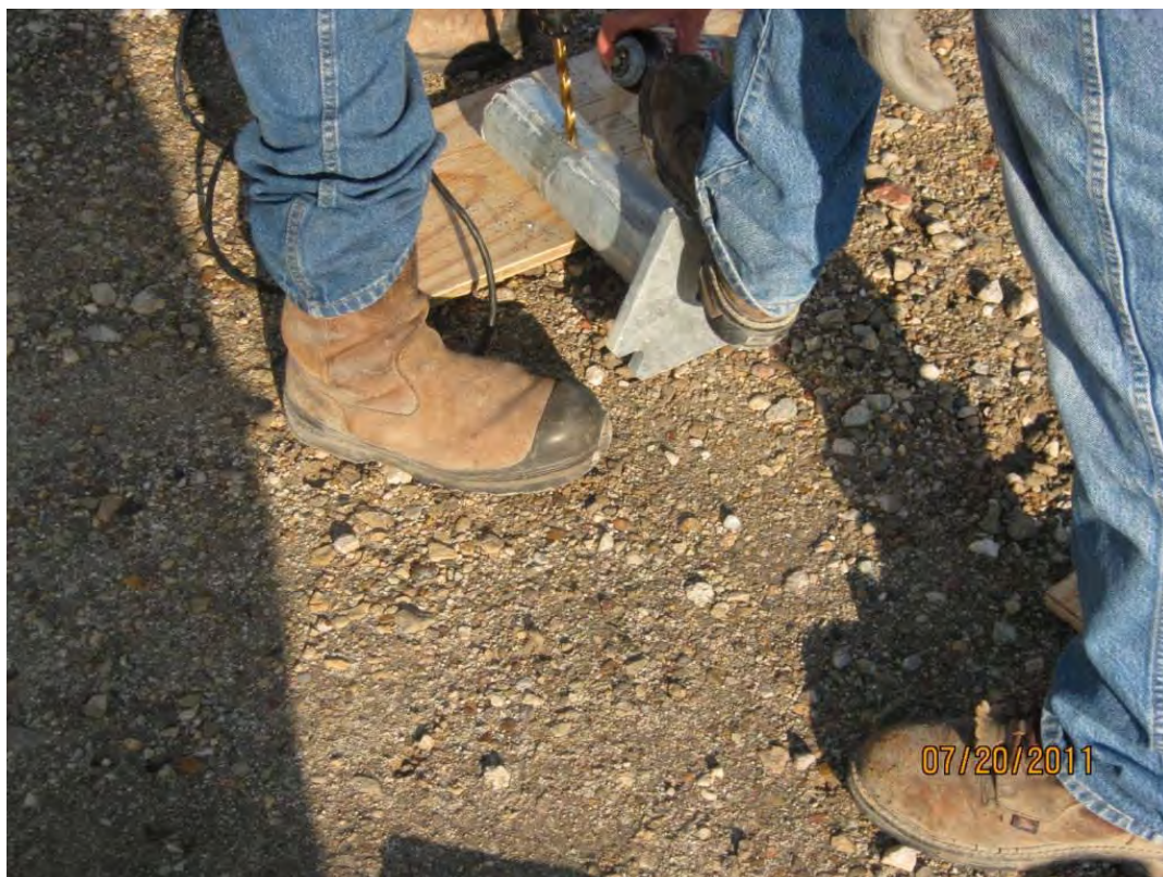
Photo 1 – Drilling a hole into the base of a guard rail post in preparation for construction of improved sign posts.
