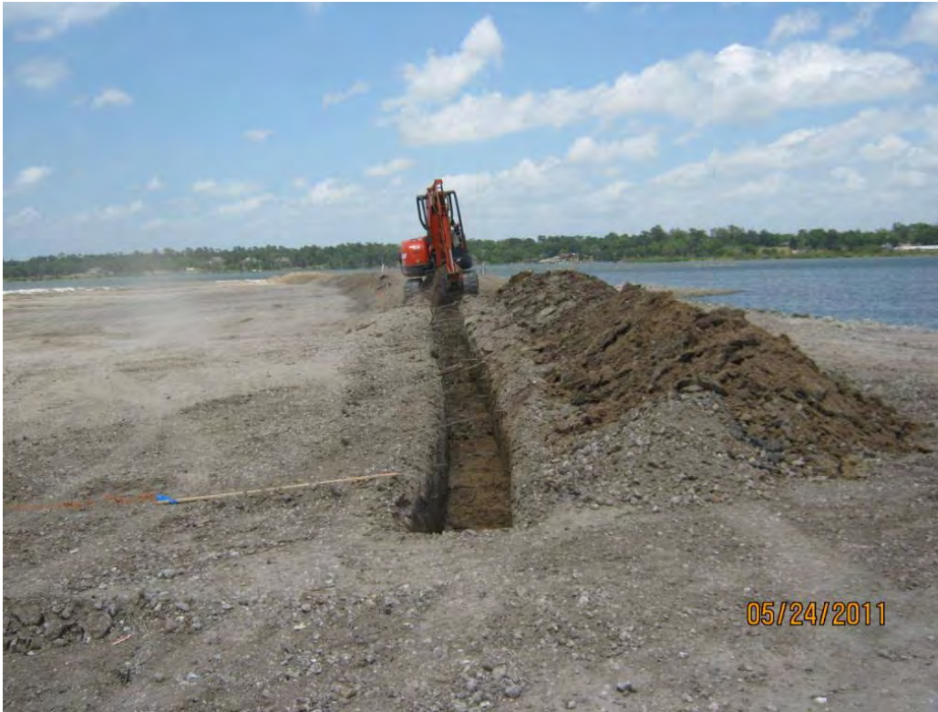
Photo 4 – Excavating a 2-foot deep anchor trench along the top of the central berm.
