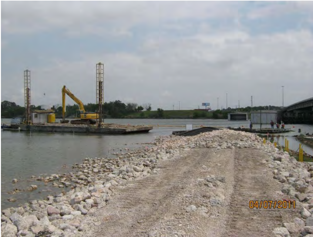
Photo 4 – Rock placement barge positioned in the south portion of the east cell to place Armor Cap D rock.
