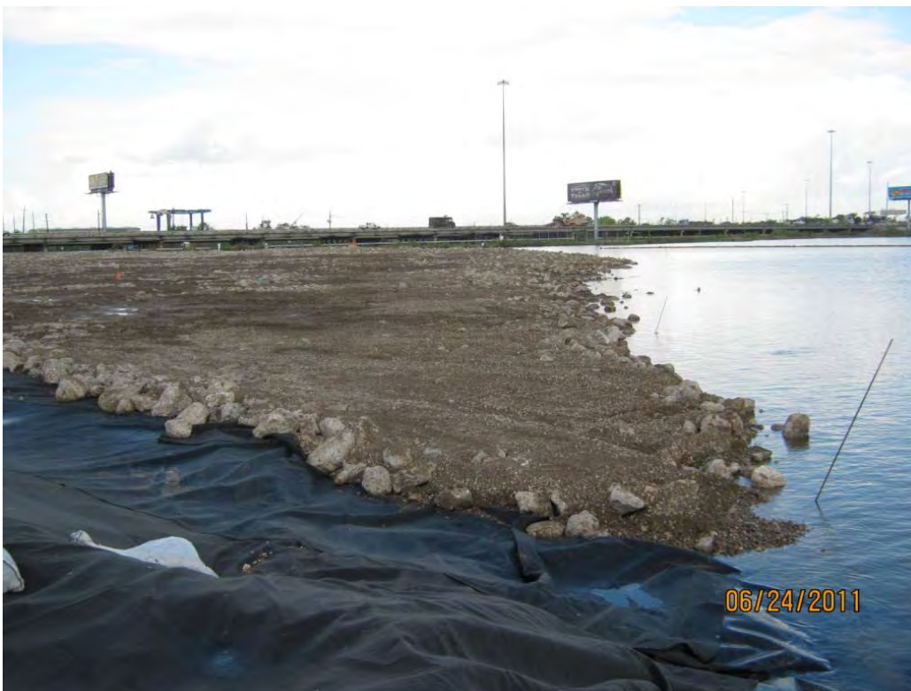
Photo 2 – Armor Cap B/C rock placed at the north end of the Western Cell (the uncovered geotextile at the foreground of the photo will receive Armor Cap D rock).
