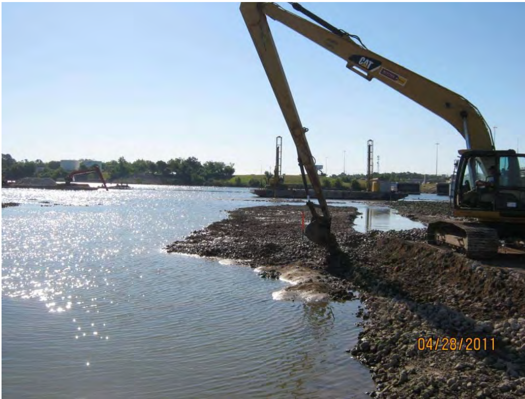
Photo 2 – Placing Armor Cap A rock in the east cell by removing rock finger roadway into the east cell.
