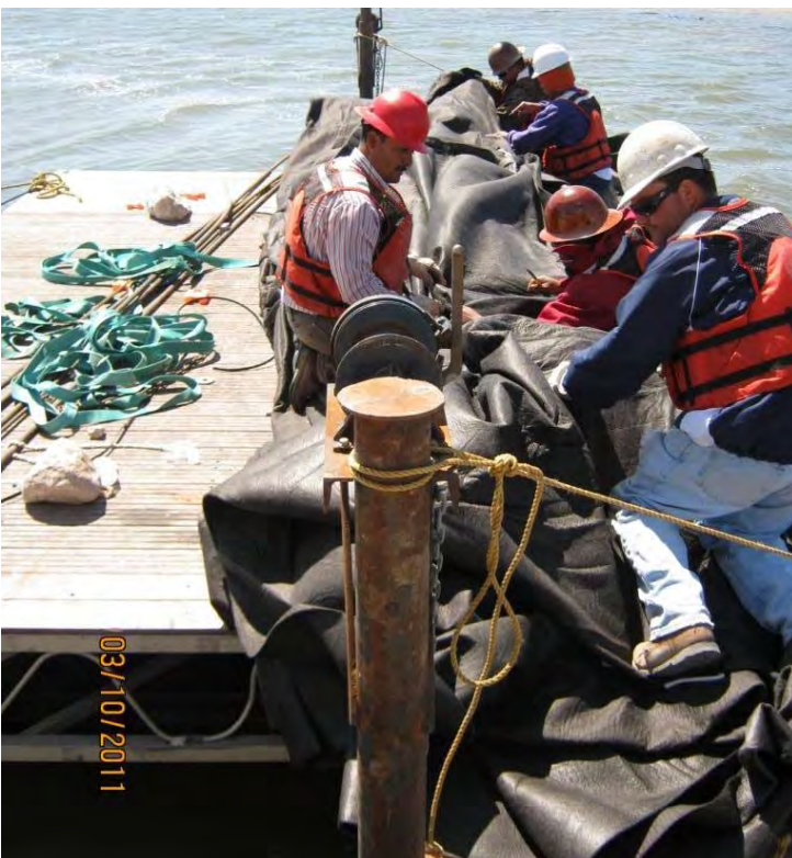
Photo 4 – Attaching new roll of geotextile to the end of the previous roll during Armor Cap D rock placement in the east cell
