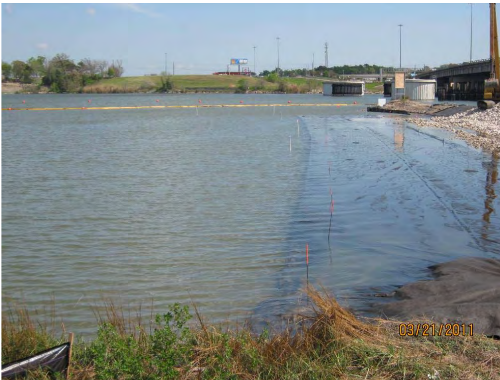
Photo 4 – Geotextile placed in the east cell; note orange-painted stakes 3 feet from edge of geotextile to provide the trackhoe operator a visual cue to leave 3 feet uncovered for overlap of the next panel.
