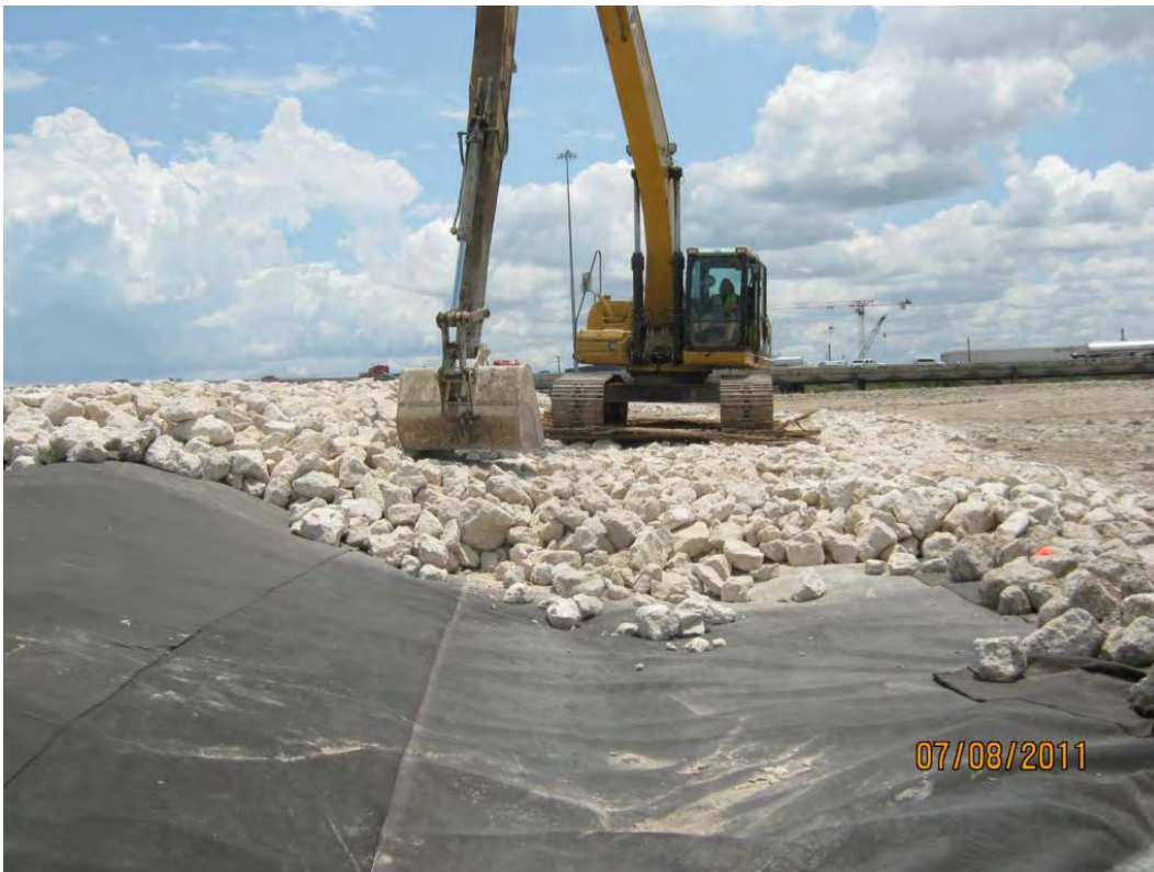
Photo 3 – Placing Armor Cap D rock along the central berm in the Western Cell.
