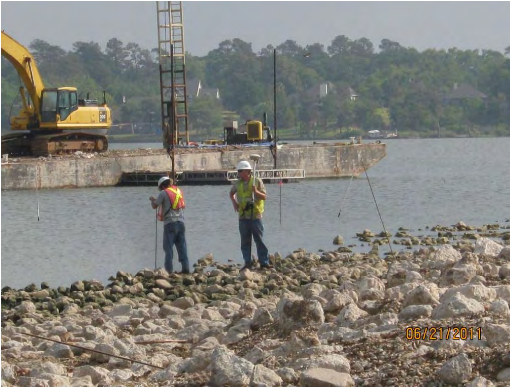
Photo 4 – Collecting Armor Cap B/C cap thickness data immediately west of the Western Cell.
