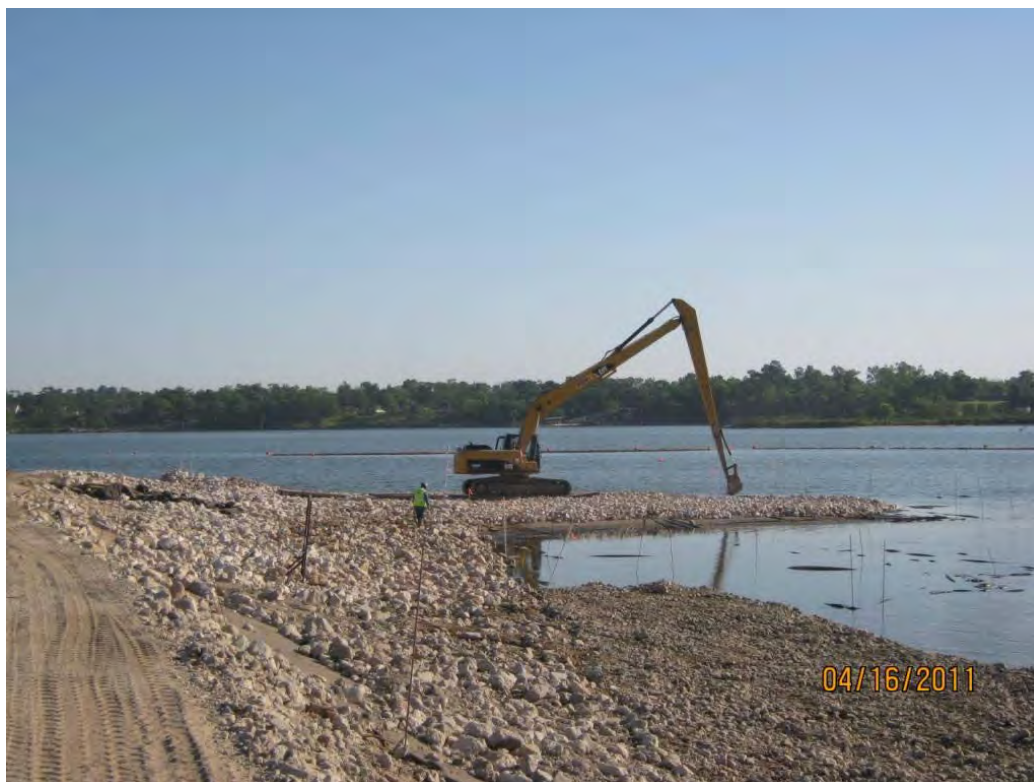
Photo 1 – Placing Armor Cap C rock in the east cell near the north end of the central berm.
