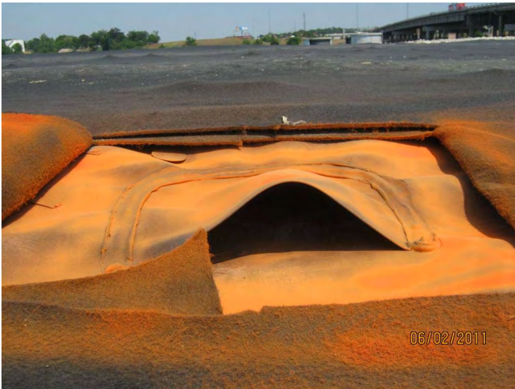
Photo 4 – Close-up of a vent installed on the inside slope of the central berm. A 2-inch diameter vent is beneath the flap; this flap was installed to divert water around the vent to prevent stormwater infiltration.
