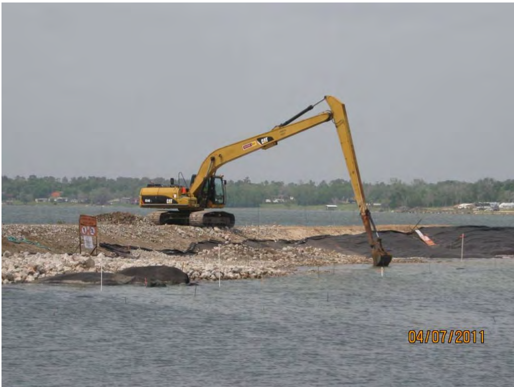
Photo 3 – Placing Armor Cap A rock to the east of the central berm.
