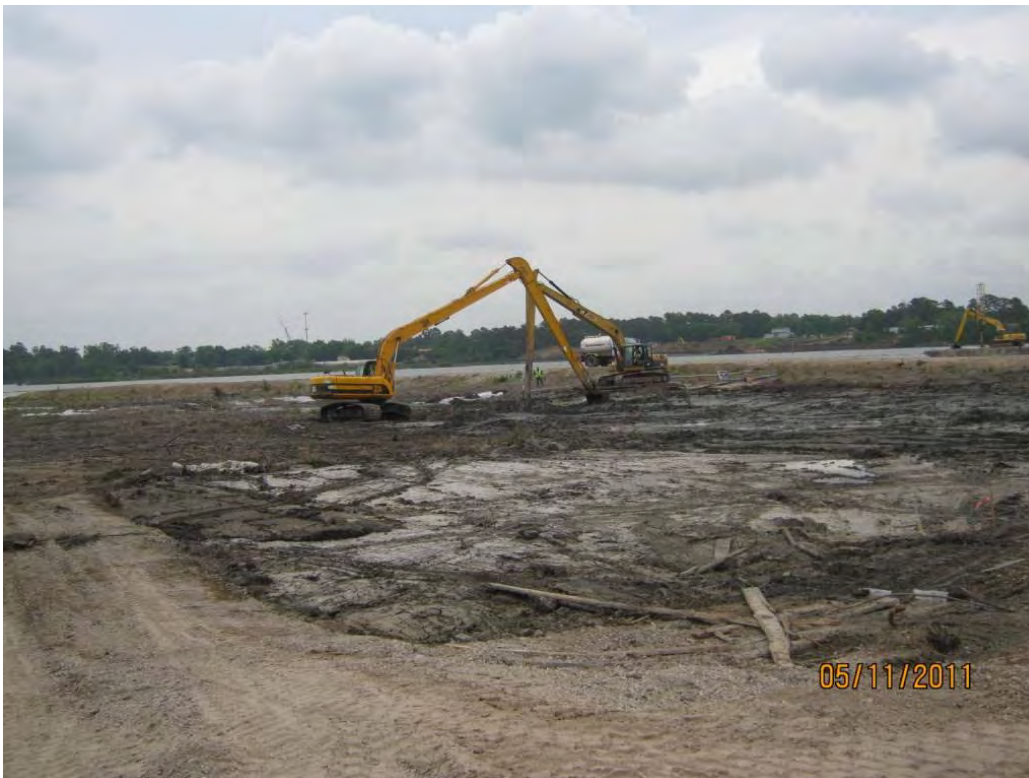
Photo 2 – Mixing Portland cement into the low-lying area in the east portion of the Western Cell.
