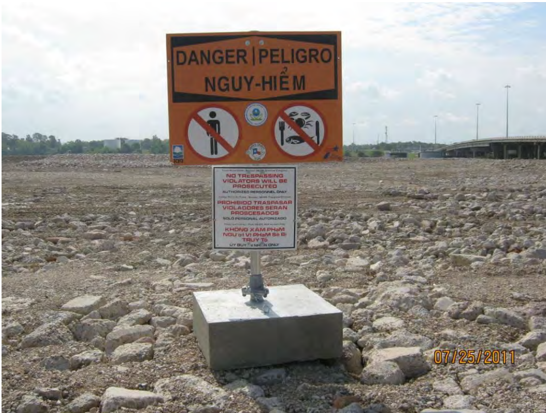
Photo 3 – Danger/No Trespassing signs mounted on a steel post attached to the base with a stainless steel cable.
