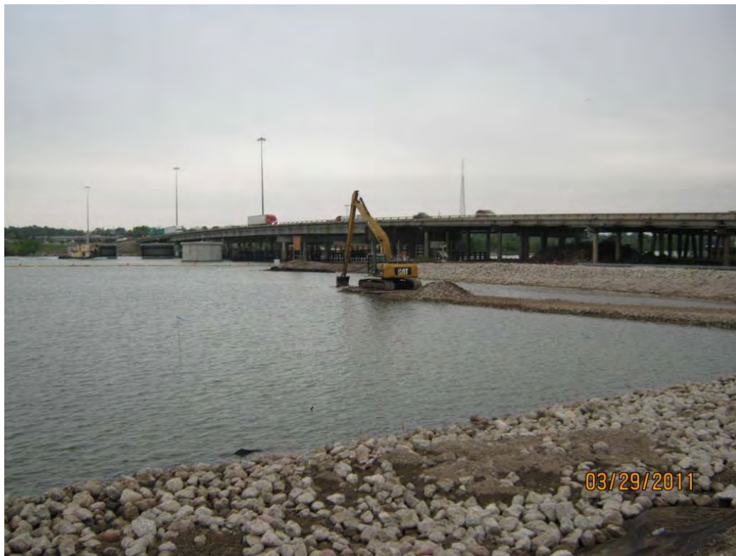
Photo 1 – Constructing a rock platform using Armor Cap A rock in the east cell.
