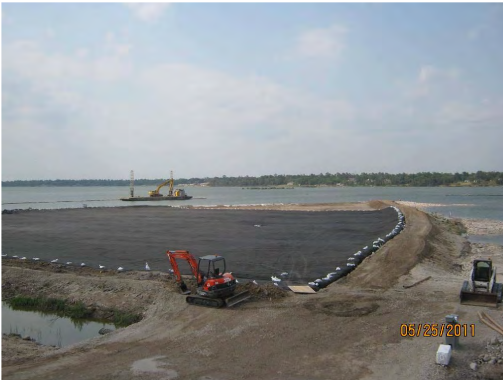
Photo 8 – Western Cell with geotextile installed over approximately 80 percent of its surface.
