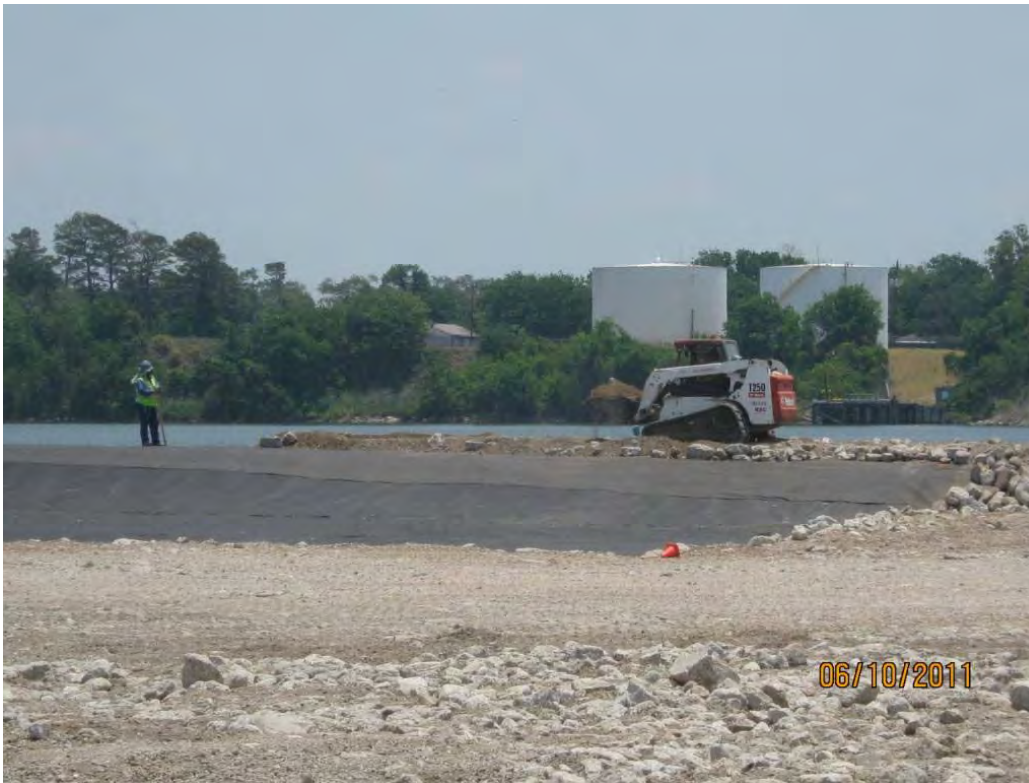
Photo 3 – Placing Armor Cap B/C rock along the top of the central berm.
