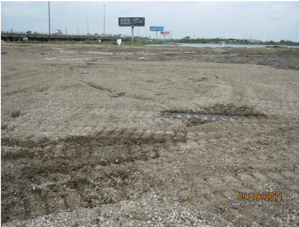
Photo 3 – Softer subgrade and water visible in the Western Cell; area will be marked and heavy equipment (e.g. dozer) will not track across this area during placement of the armored cap in the Western Cell.
