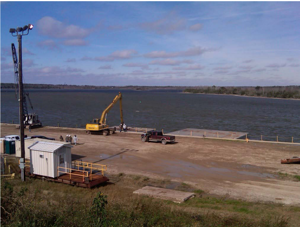
Photo 5 – Delivering sectional barges at LaBarge property and offloading to water using a crane.
