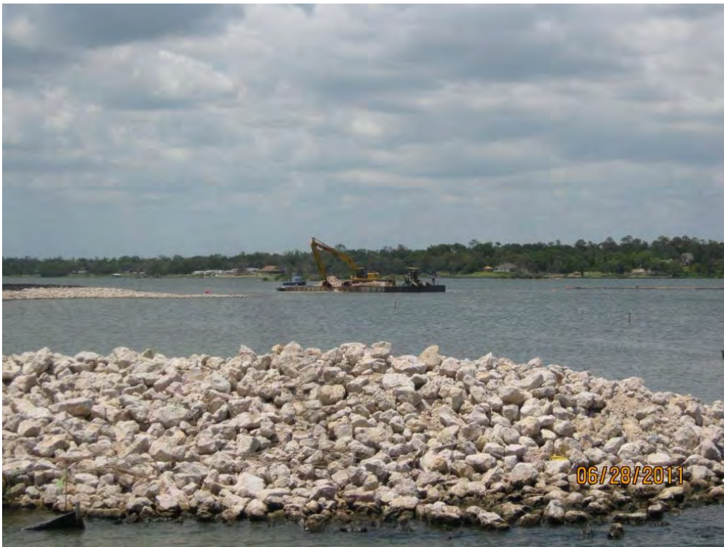
Photo 4 – Barge-mounted excavator placing Armor Cap D rock in the Eastern Cell.
