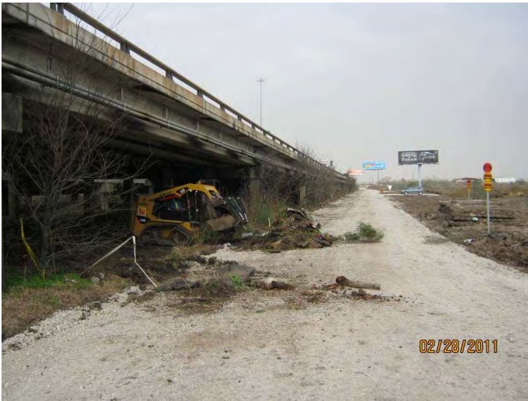
Photo 4 – Clearing debris from under I-10 Bridge onto haul road using a skidsteer
