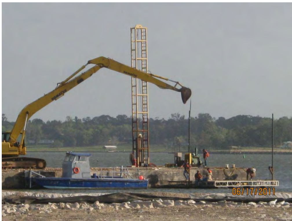
Photo 1 – Installing new, longer spuds onto the floating dock to improve access to deeper-water locations for probing armored cap thickness.
