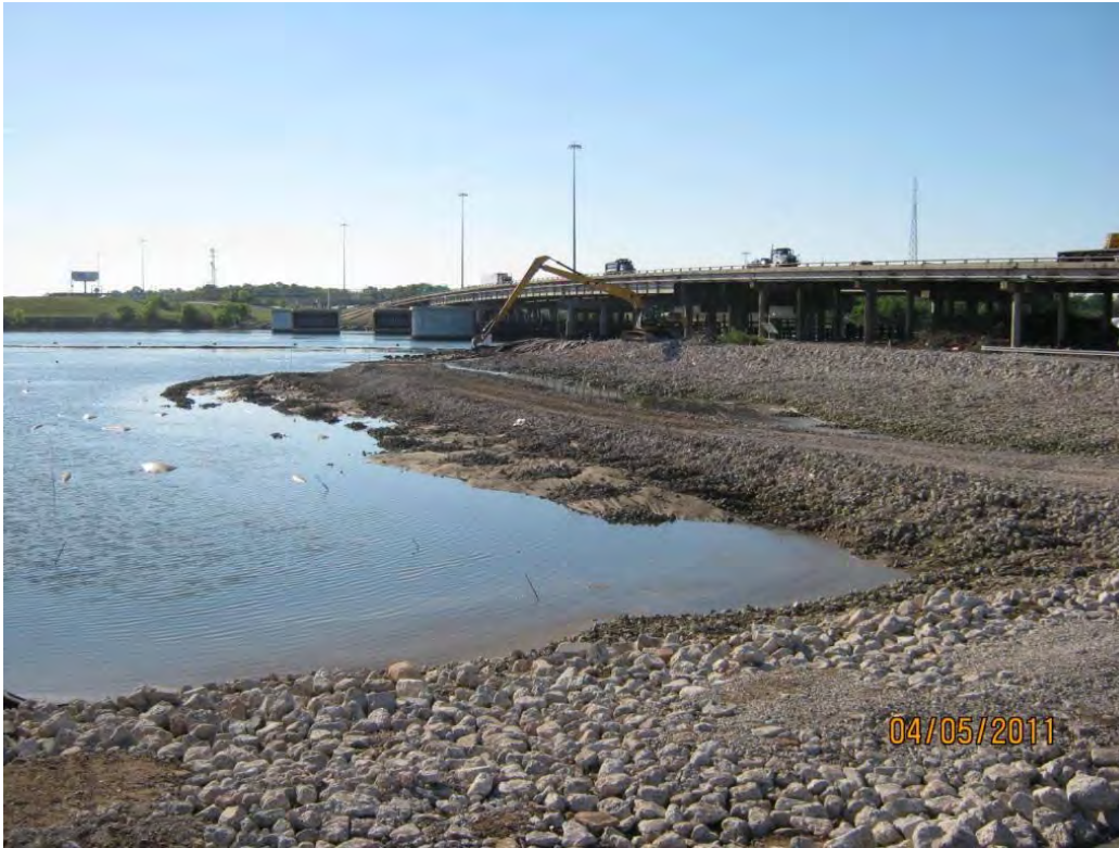
Photo 1 – Placing Armor Cap B/C rock in the east cell near the south berm.
