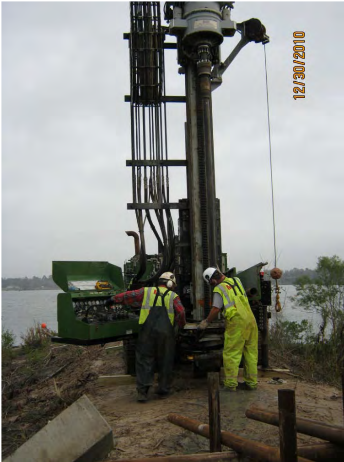
Photo 5: Sonic Drilling Rig and 2 crew on central berm
