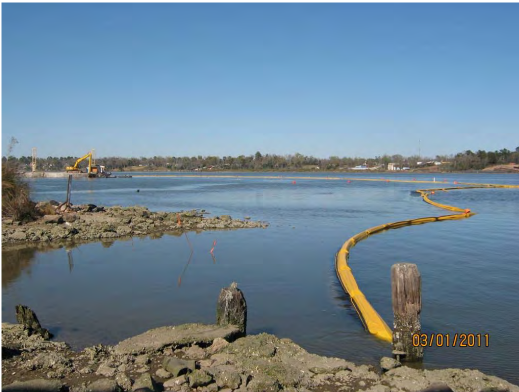
Photo 6 – Placing Armor Cap D rock in the east cell (at left) and the turbidity curtain during incoming tide (at right)
