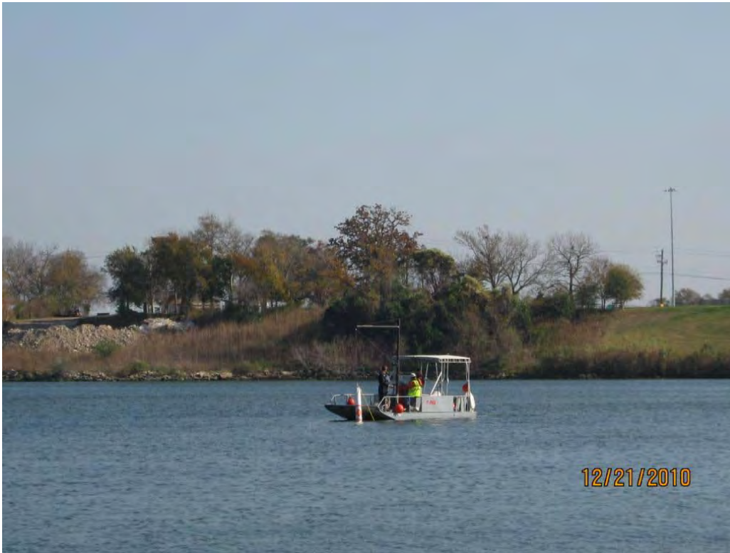
Photo 9 – Deploying concrete anchor and regulatory buoy using steel frame/winch.
