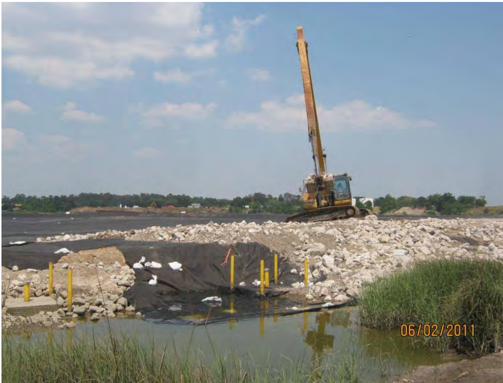
Photo 7 – Long-reach excavator placing Armor Cap B/C rock on the outside slope of the south berm.
