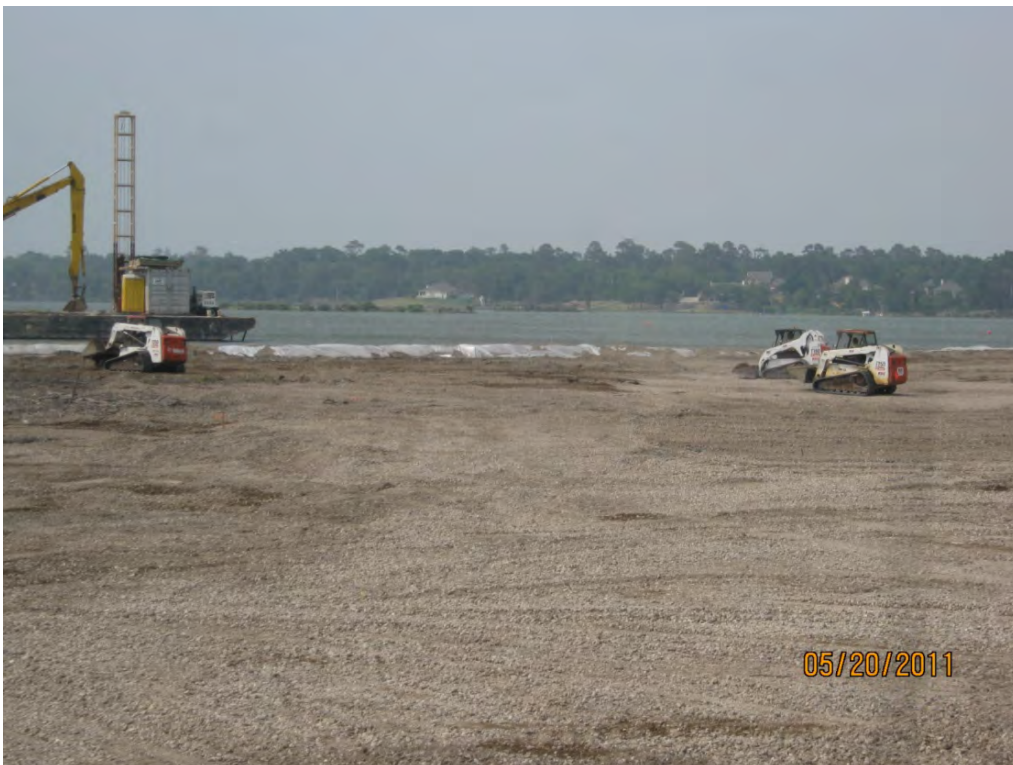
Photo 3 – Low-ground pressure skid-steers spreading CCRB in the Western Cell.
