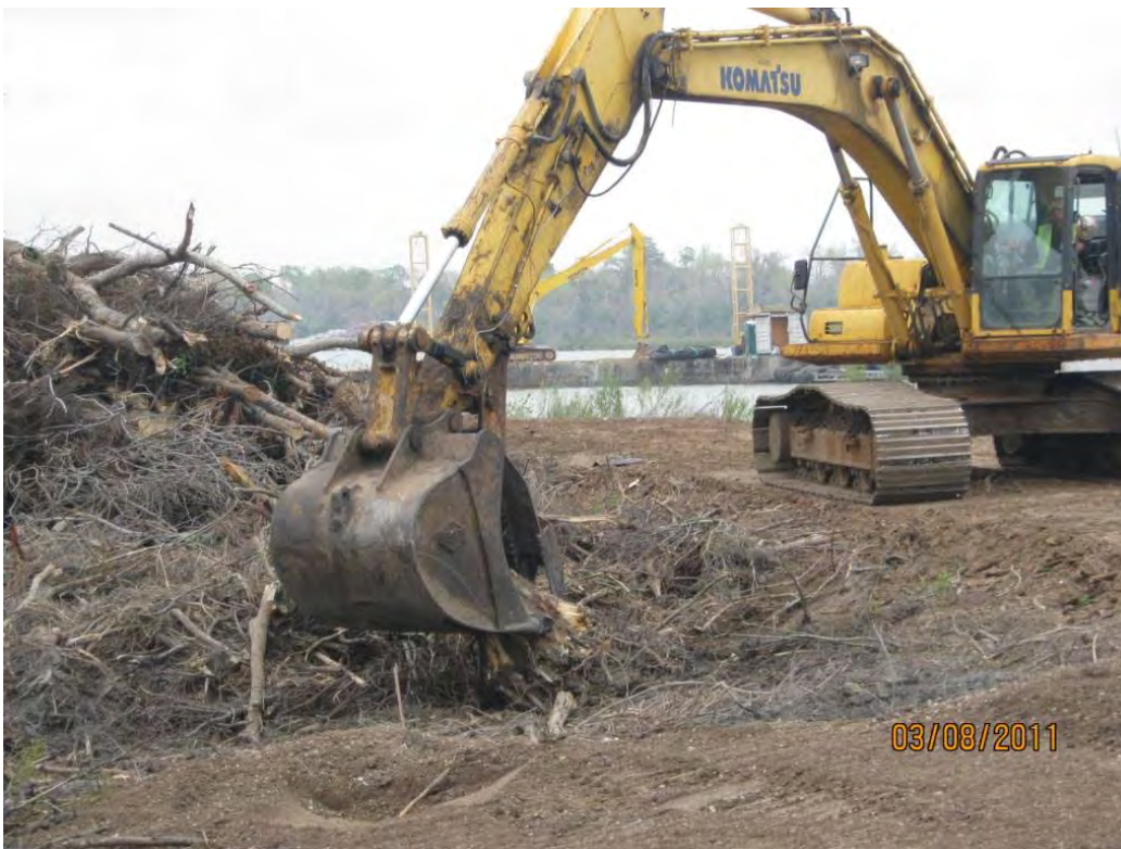
Photo 4 – Breaking root wad into smaller pieces using excavator bucket with thumb attachment
