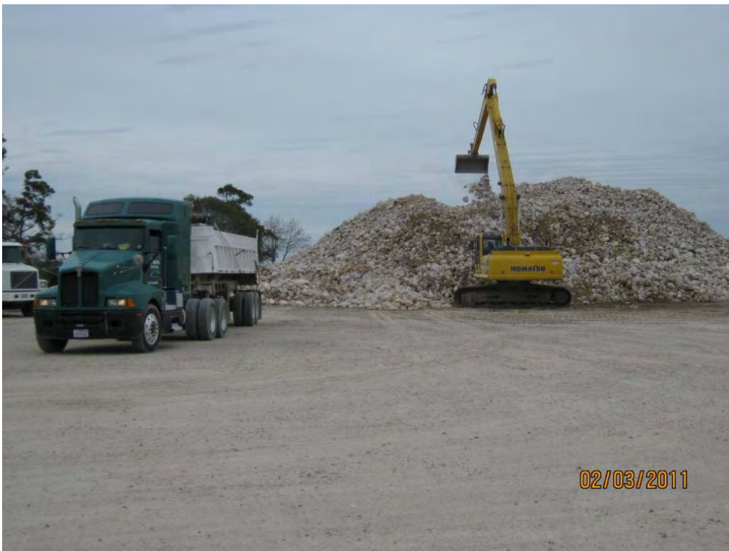
Photo 4 – Maintaining Armor Cap D stockpile at the LaBarge property using long-stick excavator
