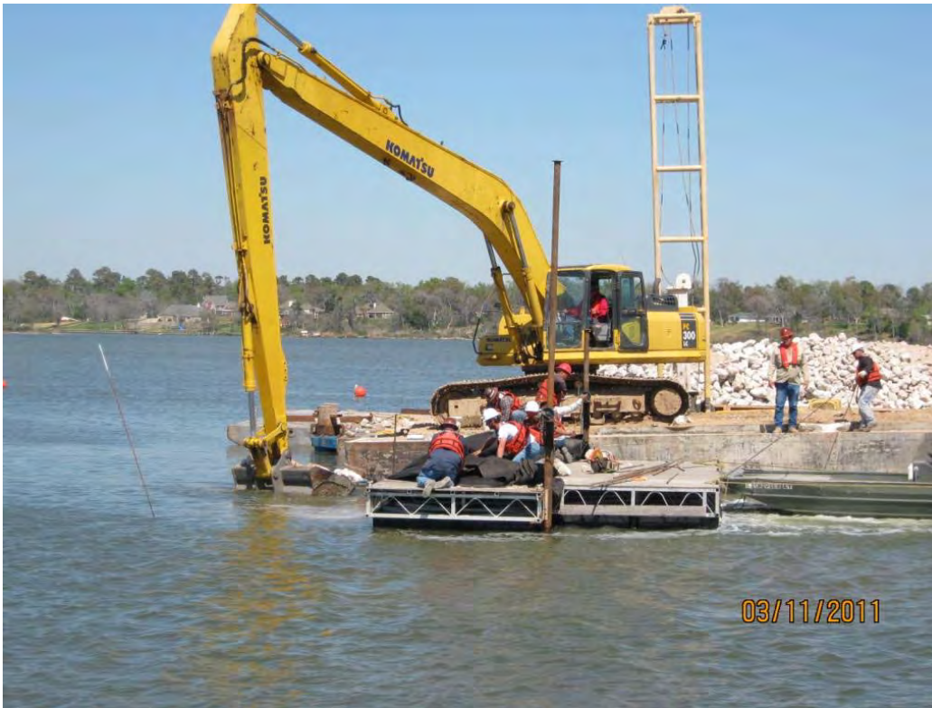
Photo 3 – Deploying geotextile and placing Armor Cap D rock in the east cell near the northern end of the central berm.
