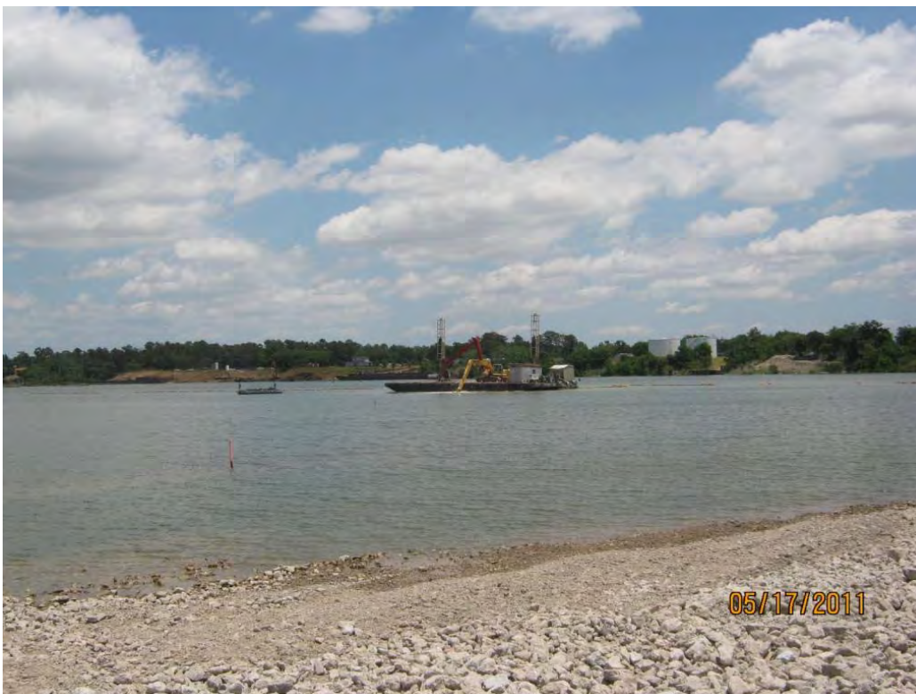
Photo 6 – Using excavator bucket to measure the thickness of Armor Cap D placement in the Eastern Cell.
