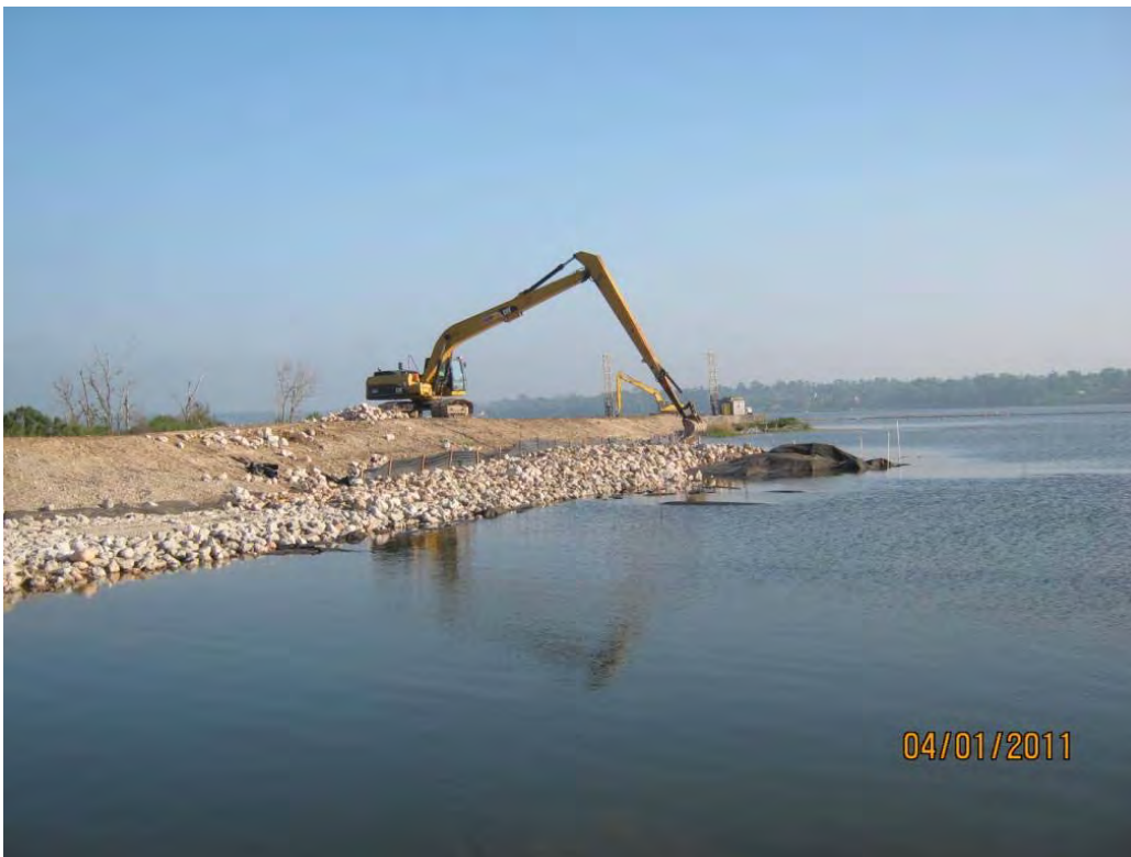
Photo 2 – Eastern Placing Armor Cap D rock near the central berm in the east cell.
