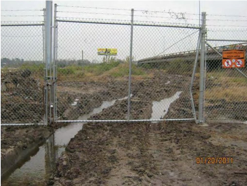
Photo 1. Main access gate north of I-10, with bent post and rutted entry way
