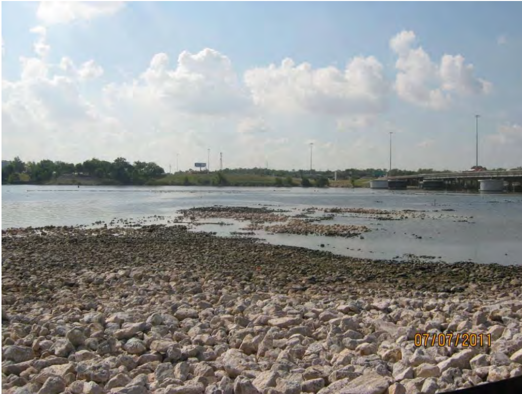
Photo 1 – Newly-placed (lighter-colored) rock placed in the Eastern Cell at the most distant areas of rock visible in this photo.
