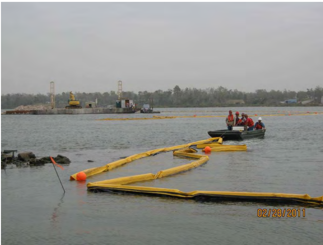
Photo 1 – Breach in turbidity curtain that occurred sometime between construction activities on Friday afternoon (2/25/11) and Monday morning (2/28/11)
