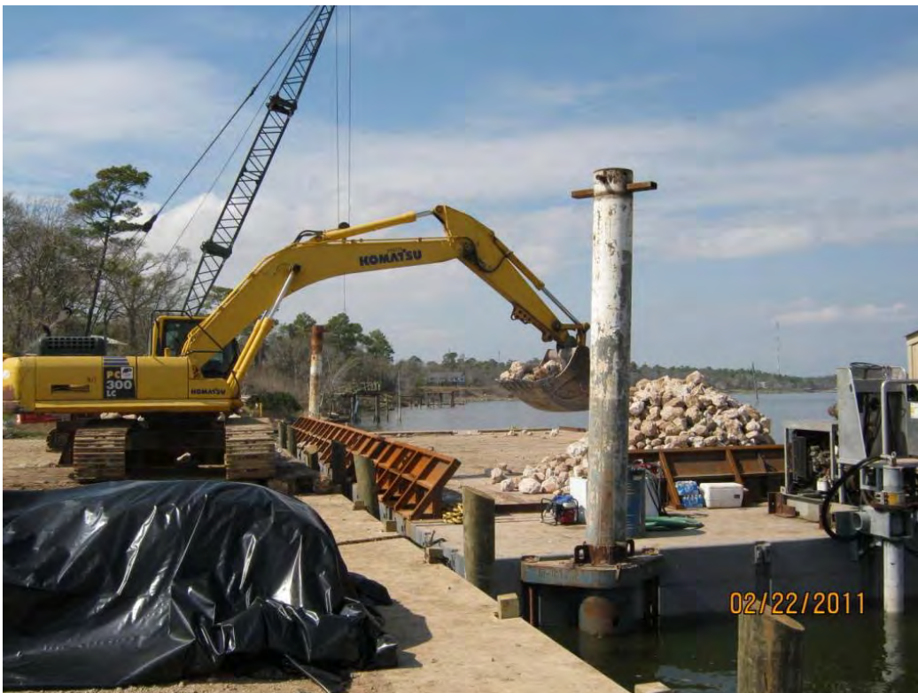
Photo 4 – Loading Armor Cap D rock onto aggregate transport barge at the LaBarge Property
