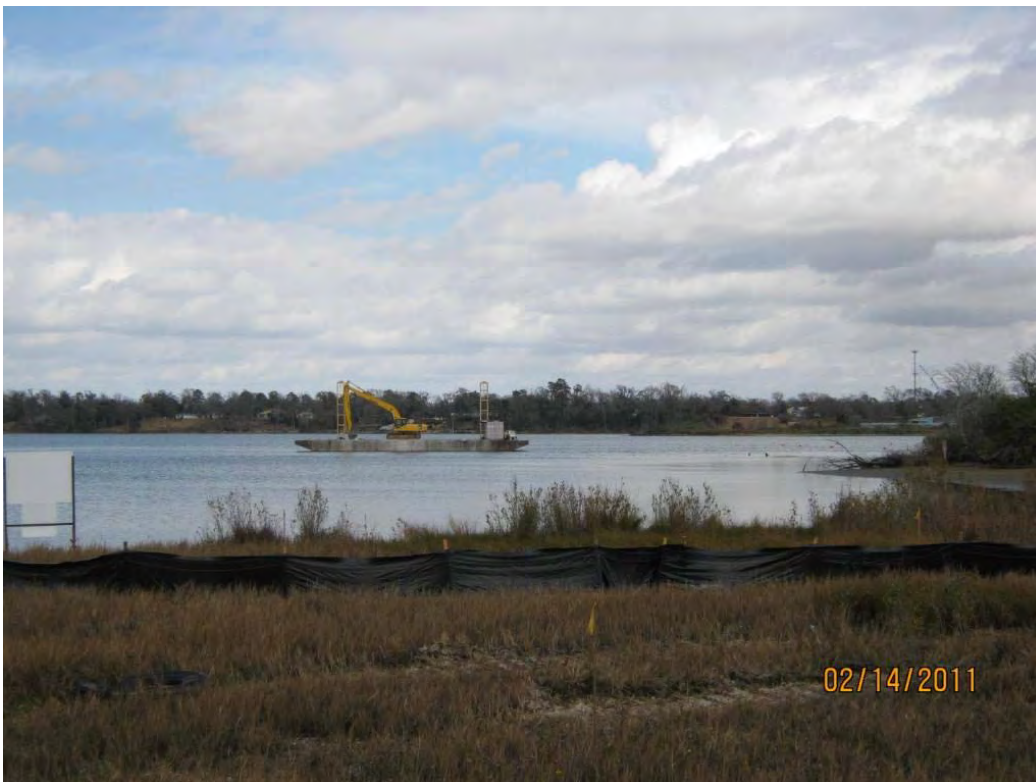
Photo 4 – Barge-mounted excavator for future water-based rock placement at SJRWP anchored to north of west cell
