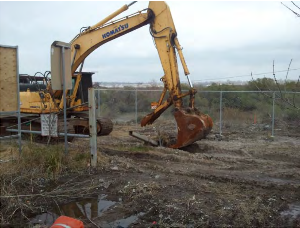
Photo 3. Komatsu PC300LC removing post in front of main access gate
