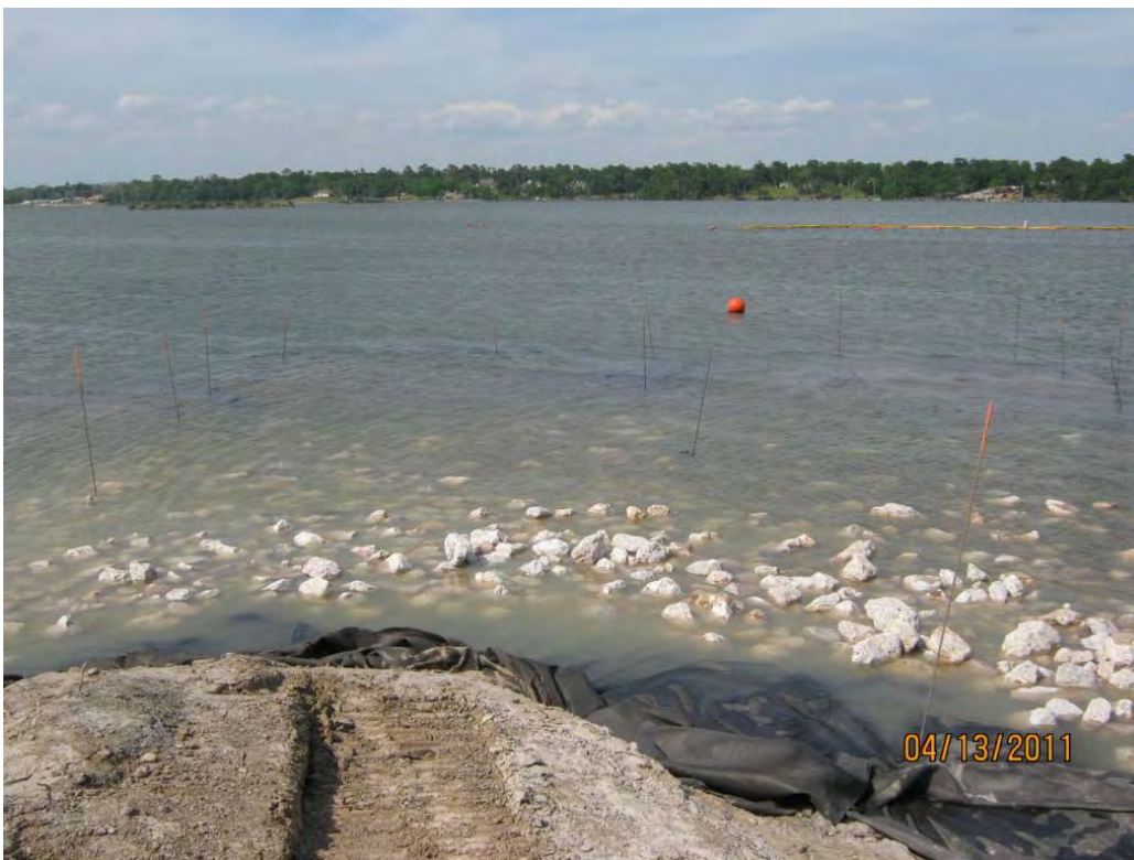
Photo 2 – Armor Cap D rock placed at the north end of the central berm.
