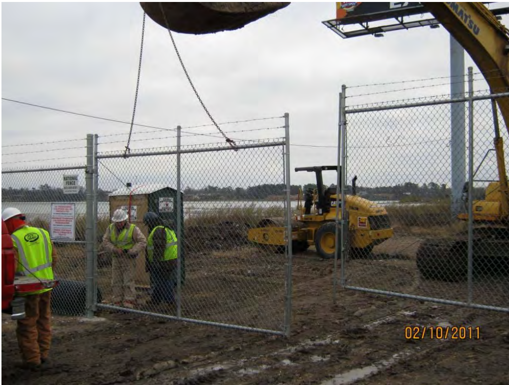
Photo 1 – Raising height of main access gate at TxDOT ROW to accommodate aggregate haul road scheduled for construction beginning tomorrow, 2/11
