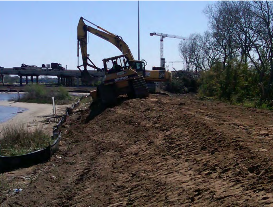
Photo 7 – Grading the east slope of the central berm to establish a stable slope for future rock placement
