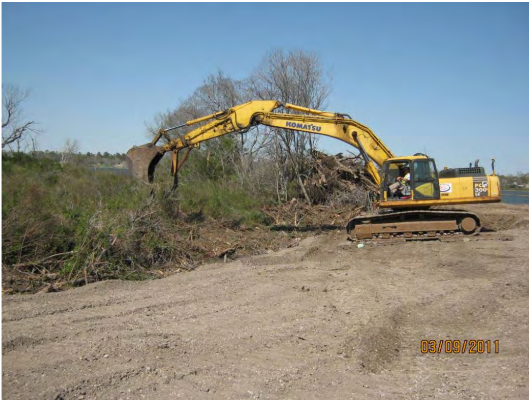
Photo 4 – Breaking root wads into smaller pieces and placing in the west cell
