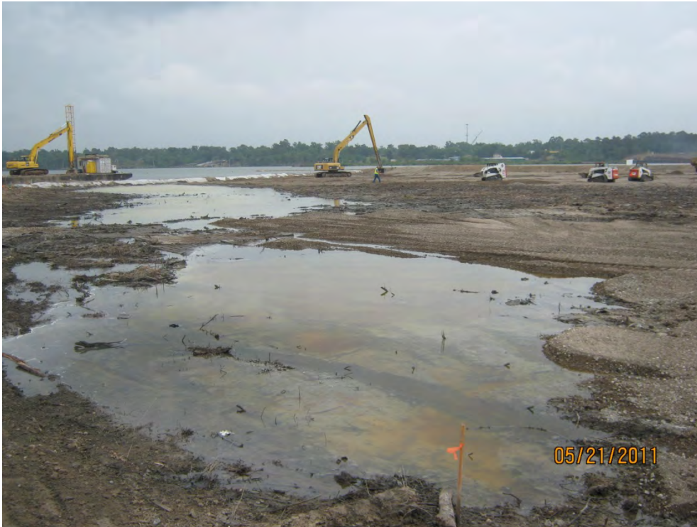
Photo 1 – Excavator and skid-steer application of CCRBin the Western Cell.
