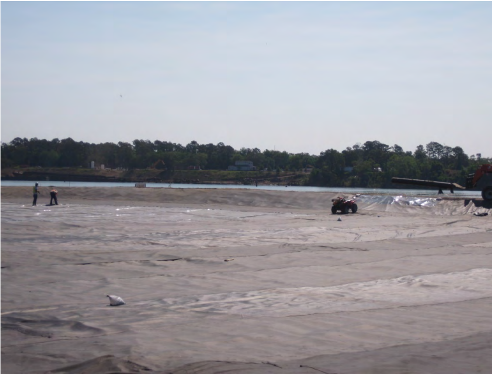
Photo 1 – Final detailing LLDPE liner to be overlaid by 16-oz geotextile in Western Cell.
