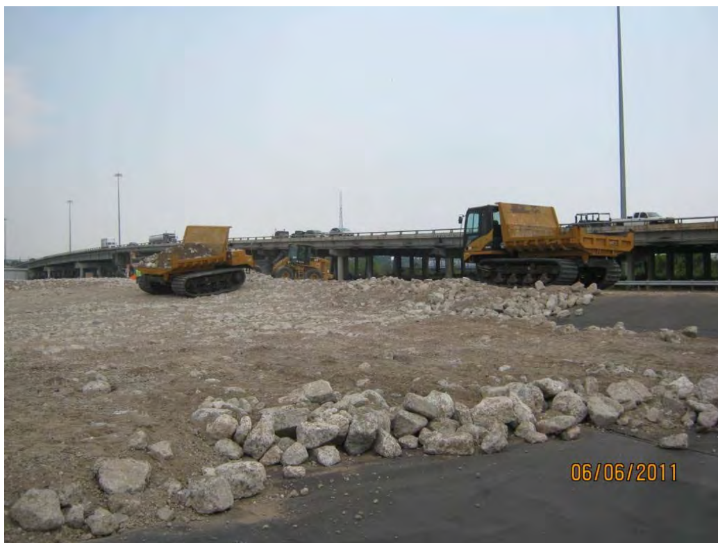
Photo 1 – Morooka trucks delivering Armor Cap B/C rock to the Western Cell for placement.
