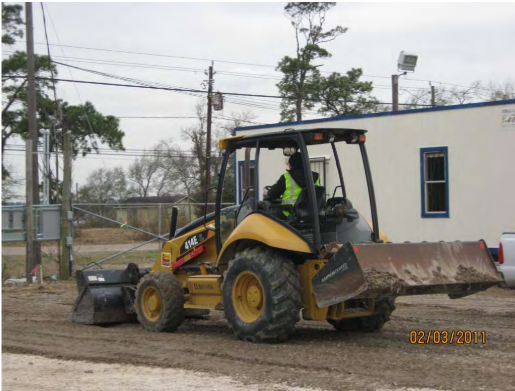
Photo 3 – Grading crushed concrete road base to improve parking lot at administrative area
