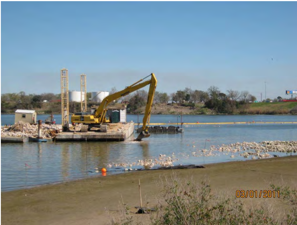
Photo 5 – Placing Armor Cap D rock in the east cell
