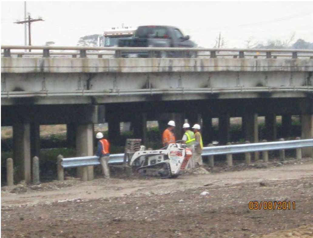
Photo 3 – Installing guard rail along haul road adjacent to I-10 Bridge
