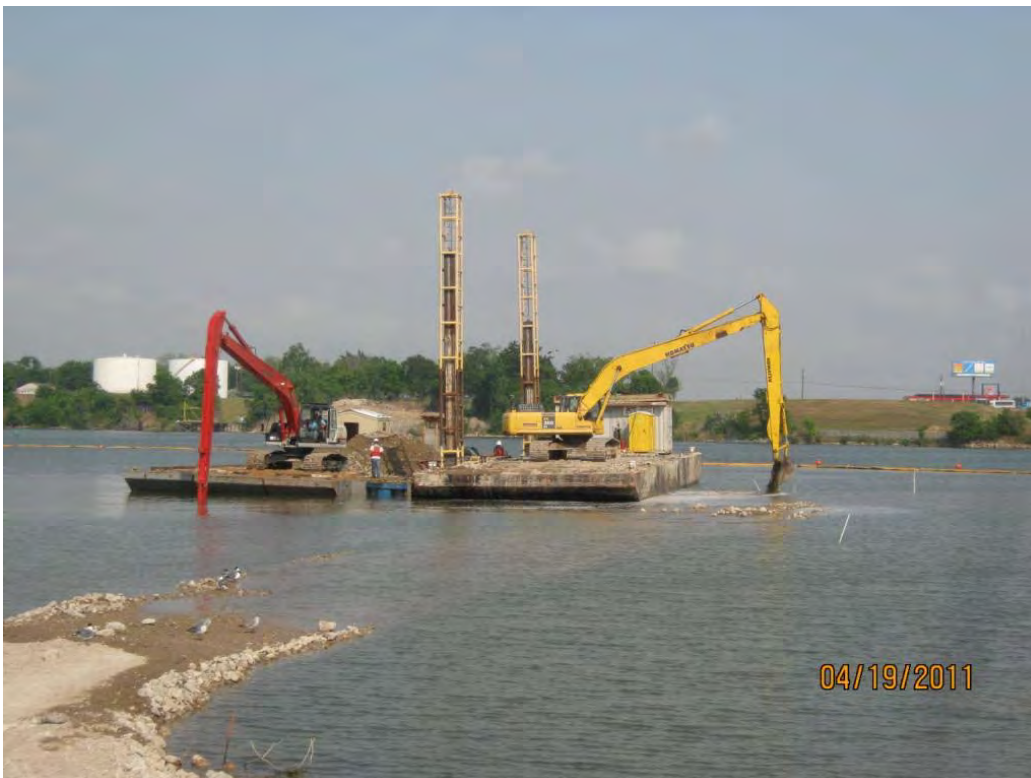
Photo 4 – Placing Armor Cap A rock in the east cell to the east of the rock access bridge.
