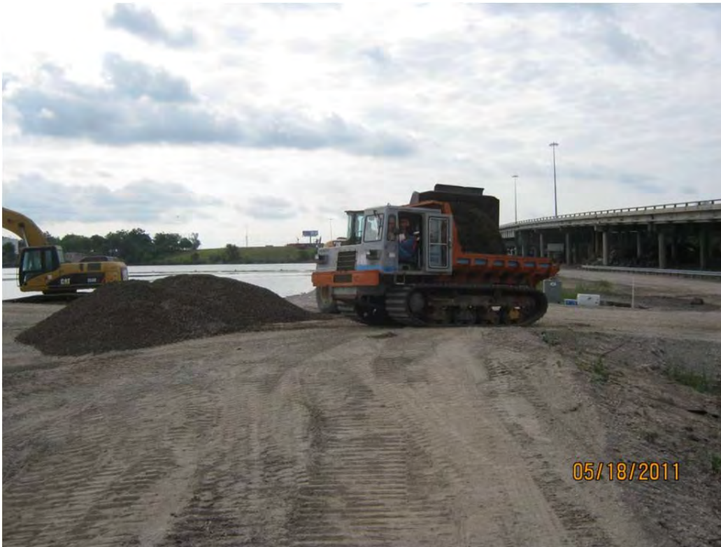
Photo 1 – Loading low-ground pressure Morooka truck with crushed concrete road base.
