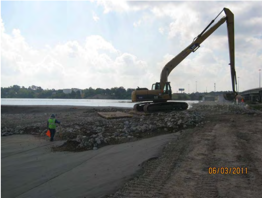
Photo 1 – Placing Armor Cap B/C rock near the southeast corner of the Western Cell.
