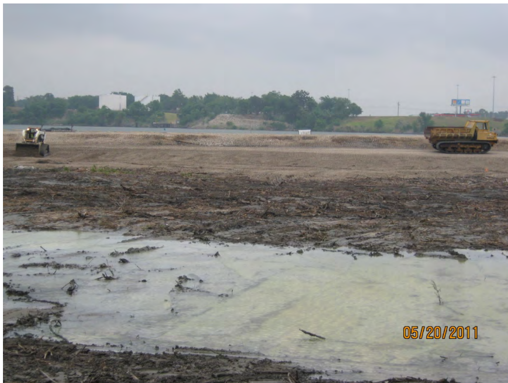
Photo 1 – Morooka truck unloading crushed concrete road base and spreading the CCRB using a skid-steer in the Western Cell.
