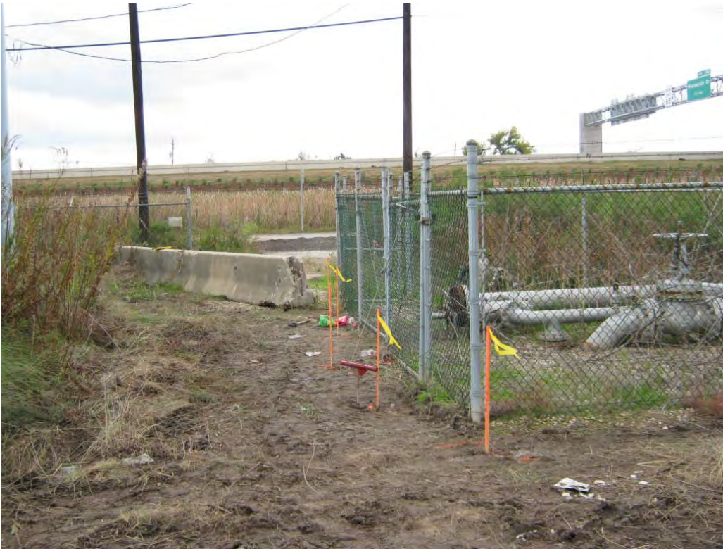
Photo 3 – Wood lathes installed by Exxon Mobil marking five pipe locations.
