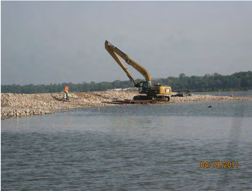
Photo 1 – Preparing to place Armor Cap A rock in the east cell via land-based operations.
