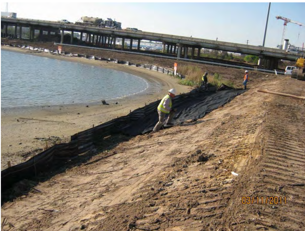
Photo 2 – Installation of geotextile prior to placement of CCRB on east face of central berm
