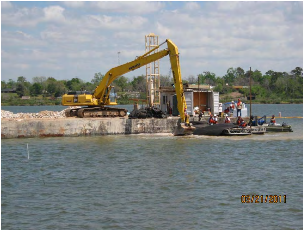
Photo 1 – Deploying geotextile and placing Armor Cap C rock in the east cell.
