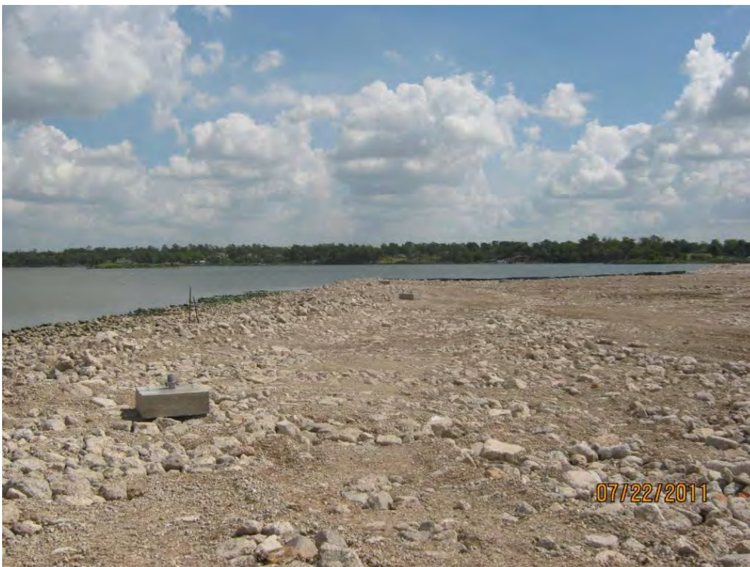
Photo 2 – Concrete pads for danger/no trespassing signs installed along the west end of the Western Cell.
