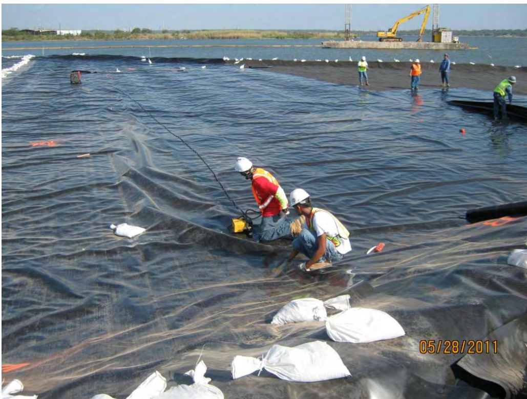
Photo 2 – Welding a seam into the LLDPE liner in the Western Cell.
