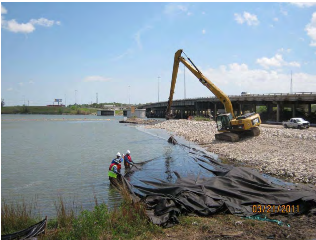
Photo 2 – Deploying geotextile using land-based equipment in the east cell.
