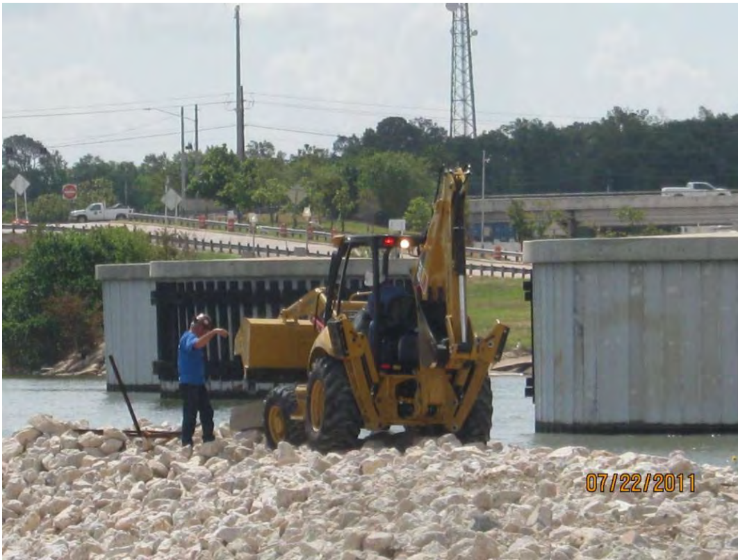
Photo 1 – Placing a 3'x3' concrete pad at the east end of the south berm at SJRWP.
