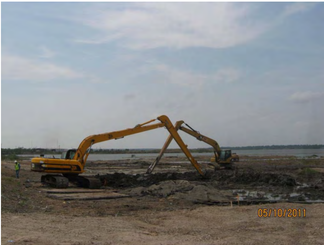
Photo 6 – Mixing cement into a low-lying area in the southeast portion of the Western Cell.
