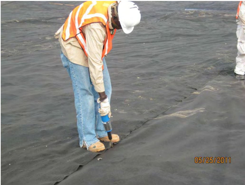
Photo 5 – Heating adjacent panels of geotextile to create a laster seam at the one-foot overlap between panels.
