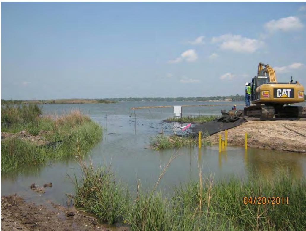
Photo 4 – Geotextile deployed in the southwest corner of the armored cap area outside the west cell.
