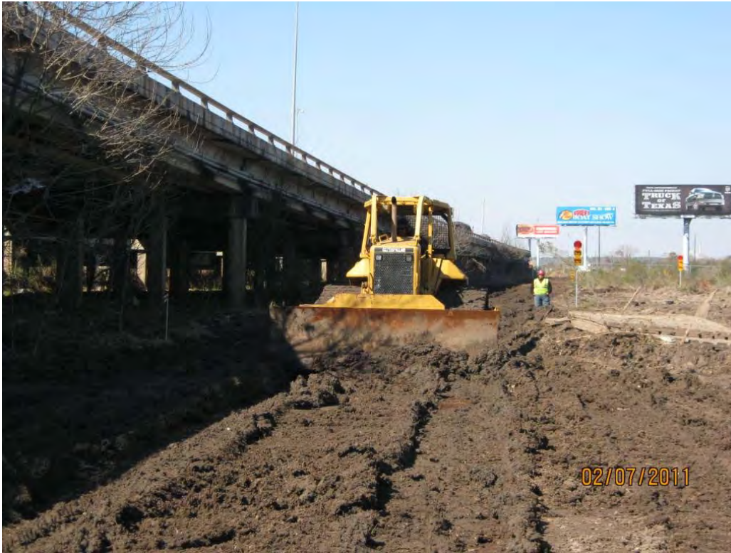
Photo 1 – Grading soil on TxDOT ROW to expose wet soil to the sun for drying
