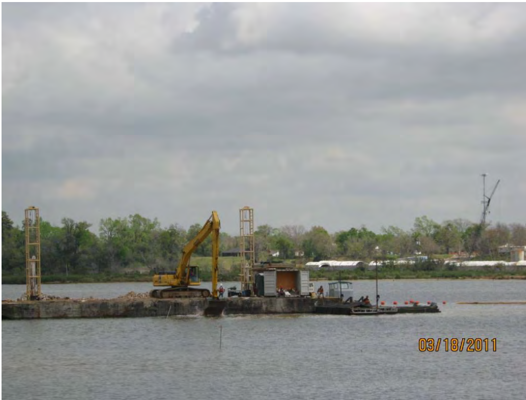
Photo 3 – Deploying geotextile and placing Armor Cap D rock in the east cell.
