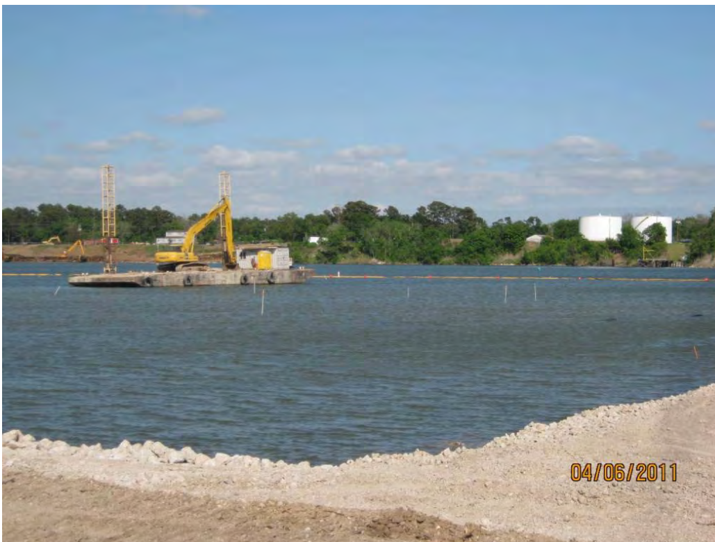
Photo 4 – Rock placement barge repositioned in the east cell to continue in this area.
