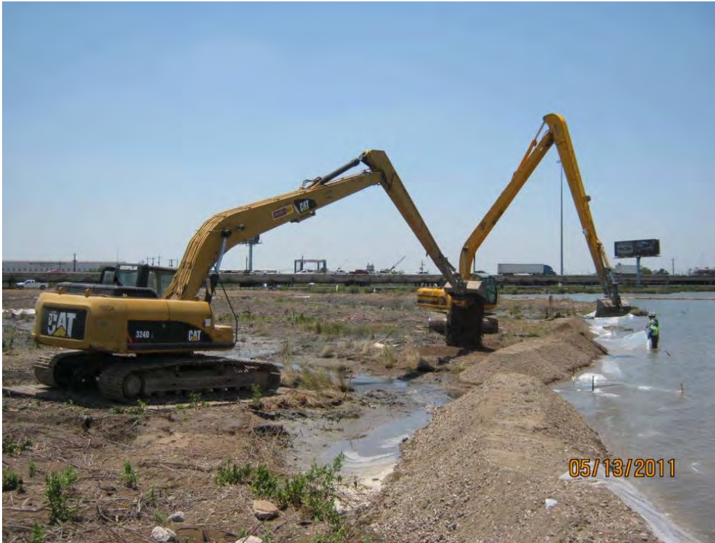
Photo 3 – Construction of the northern berm in the Western Cell.
