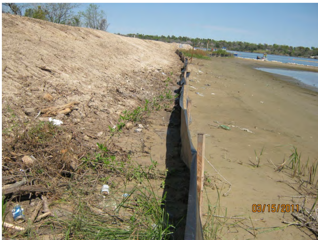
Photo 1 – Silt fence effectively retained soil washed from east face of central berm by rain on March 14.
