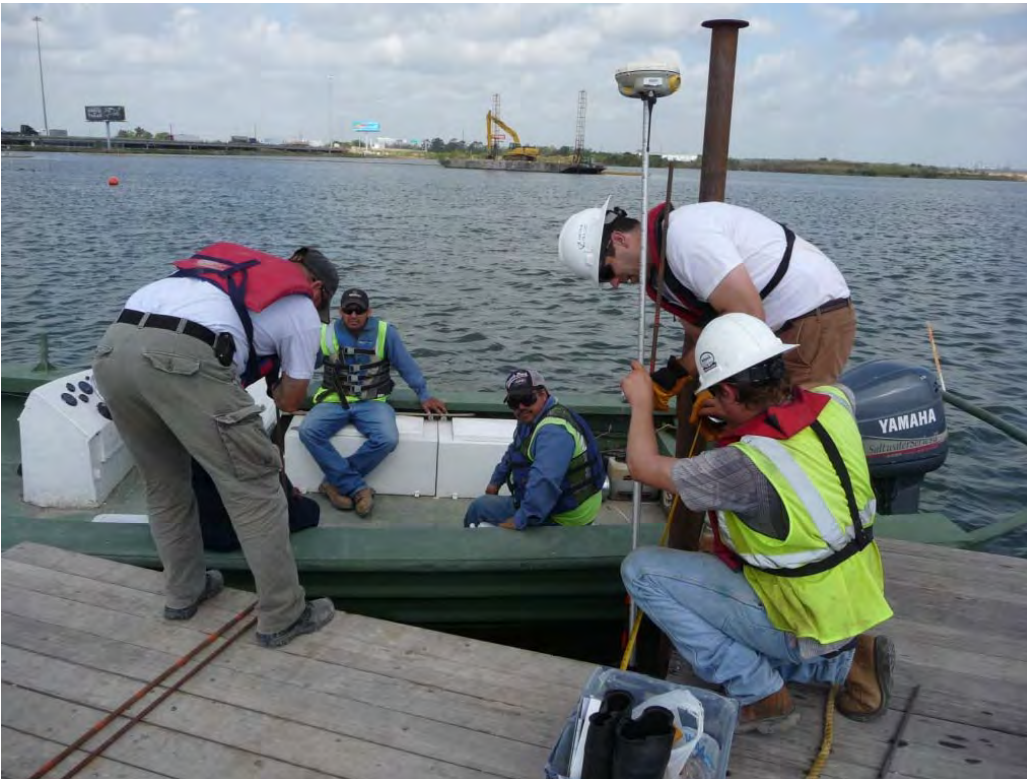
Photo 3 – Probing armored cap thickness at a grid point and using GPS equipment to record the collected data.
