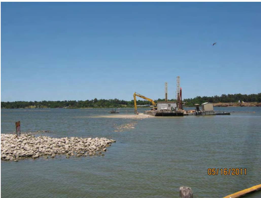
Photo 6 – Placing Armor Cap D rock in the Eastern Cell; note turbidity localized in the area to the left of the barge.
