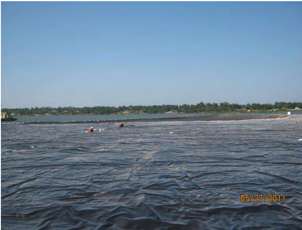
Photo 2 – LLDPE liner and geotextile to the north of the LLDPE liner in the Western Cell.
