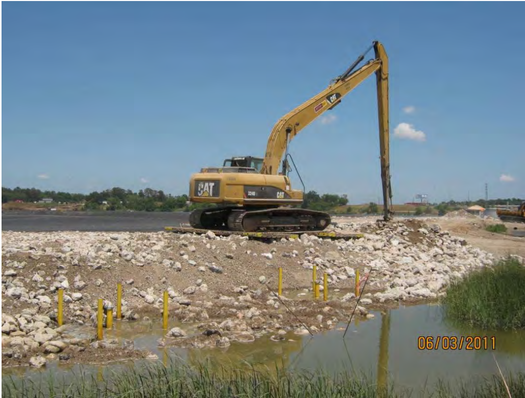
Photo 5 – Placing Armor Cap B/C rock outside the southwest corner of the Western Cell.
