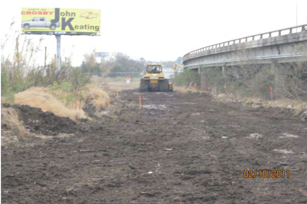
Photo 2 – Grading TxDOT ROW in advance of aggregate haul road construction
