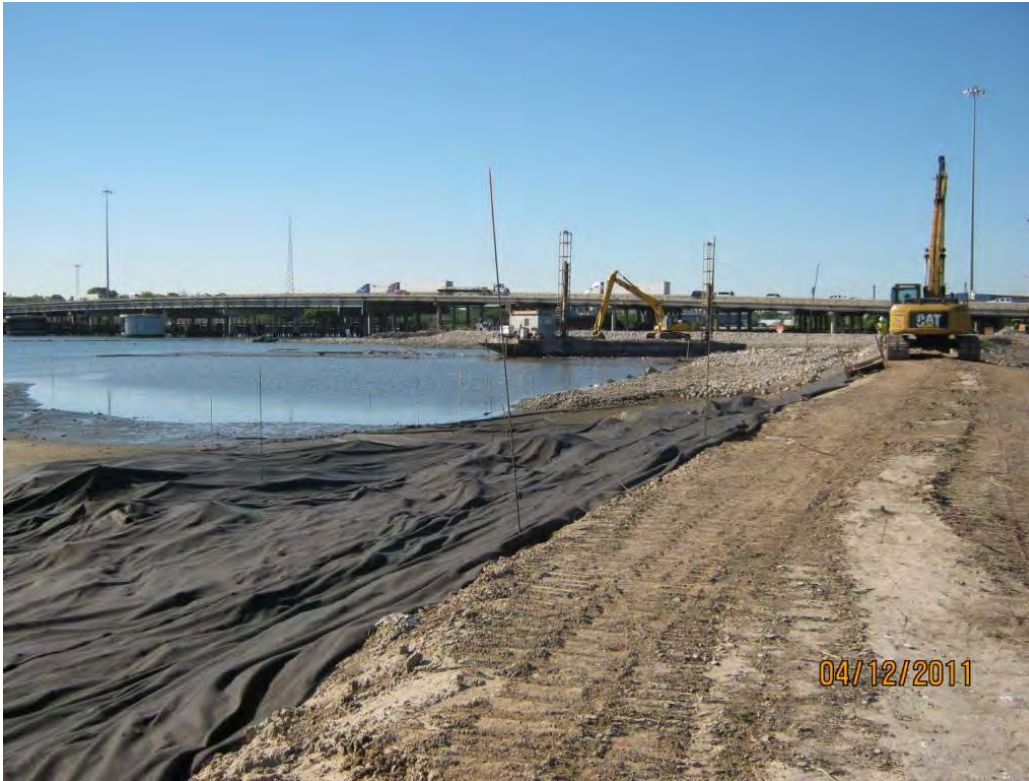
Photo 1 – Geotextile deployed to the east of the central berm (foreground), and the rock placement barge idle in the east cell due to low tide conditions caused by north winds (background).
