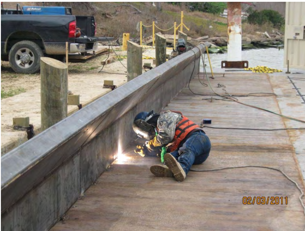
Photo 6 – Welding 2-foot steel rail to side of aggregate transport barge
