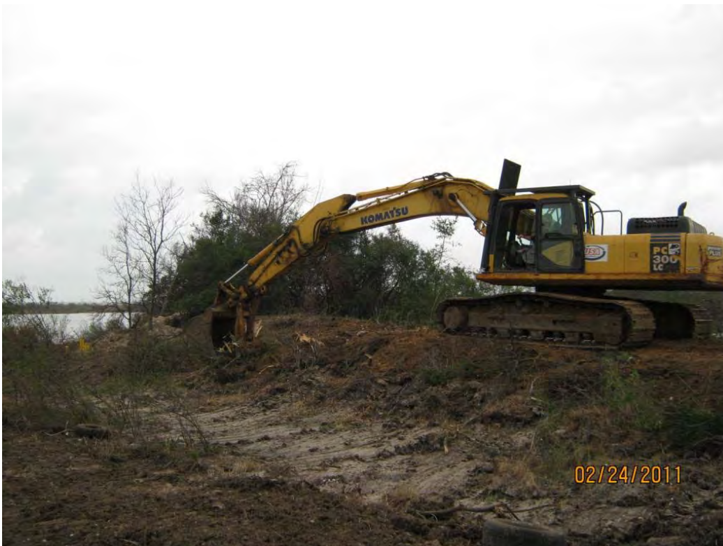
Photo 4 – Removing stump from the outer side of the south berm of the west cell
