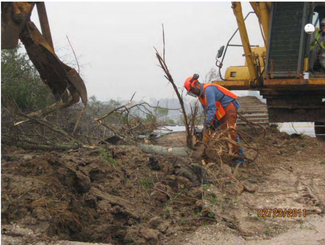
Photo 2 – Cutting root mass from tree with chainsaw
