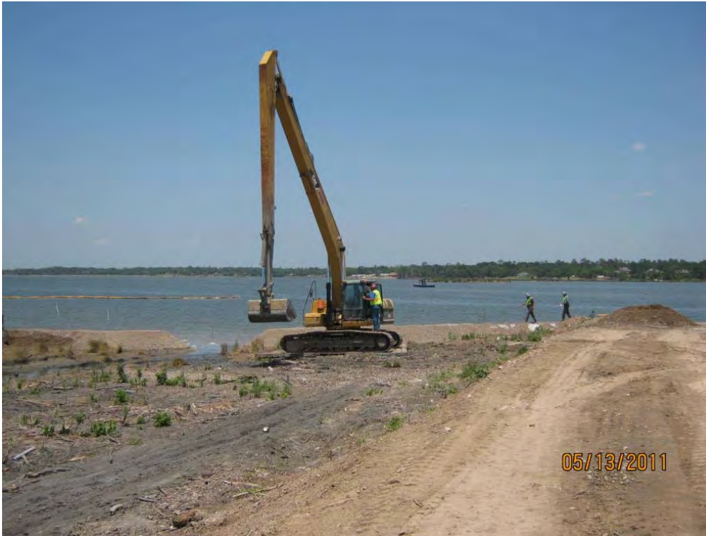
Photo 1 – Construction of the northern berm in the Western Cell.
