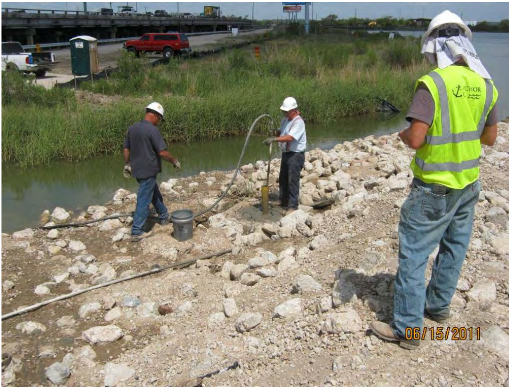
Photo 1 – Pumping grout into a monitoring well with a tremie pipe.
