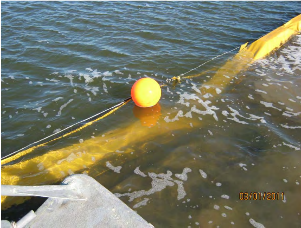
Photo 1 – Damaged 10-foot section of the floating boom; turbidity curtain underlying the boom was observed to be intact
