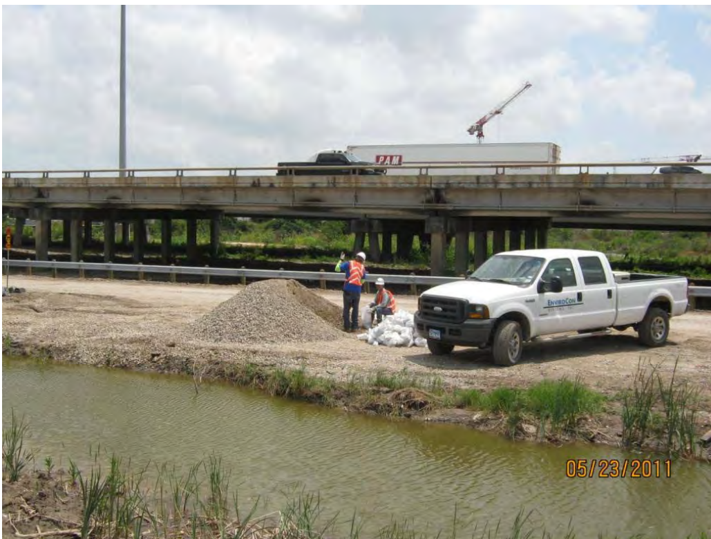
Photo 6 – Filling sand bags with crushed concrete road base for future use in the Western Cell.
