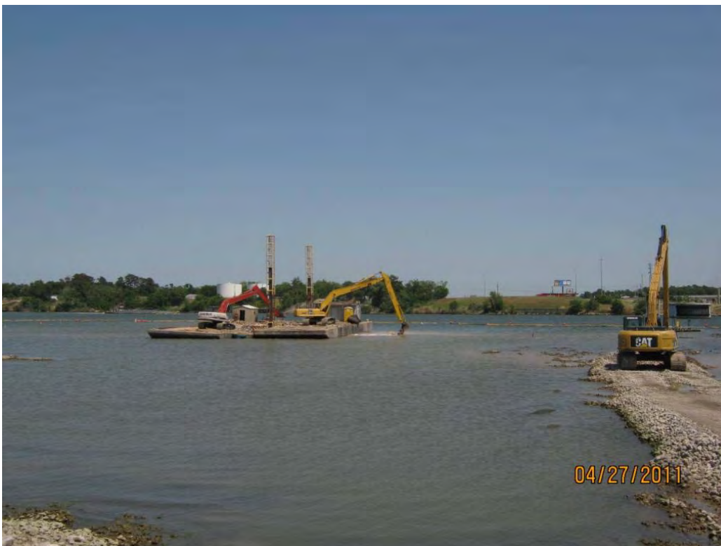
Photo 4 – Placing rock in the east cell via water-based operations (at left) and land-based operations (at right).
