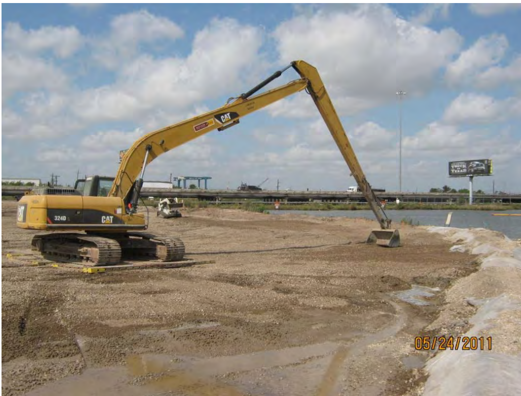
Photo 1 – Grading the surface of the Western Cell using long-reach excavator to spread crushed concrete road base.
