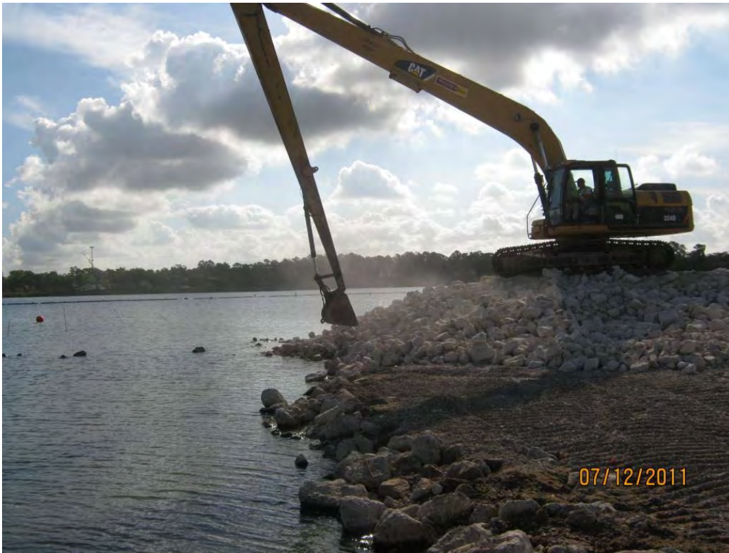
Photo 1 – Placing Armor Cap D rock at the north end of the central berm in the Western Cell.
