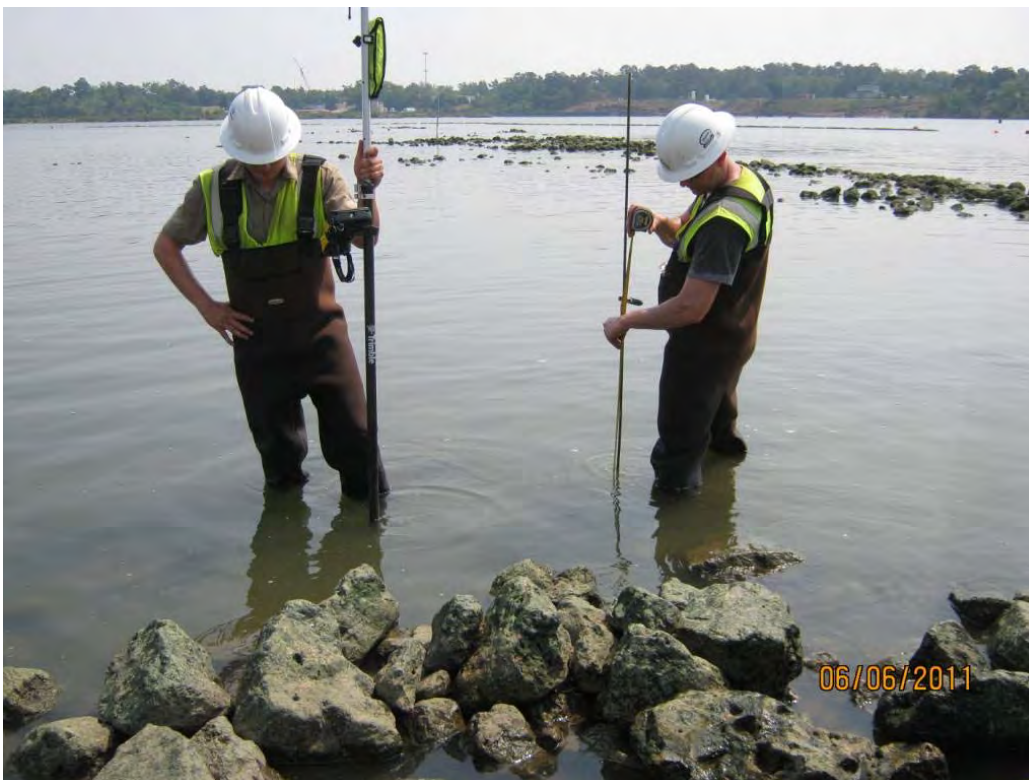
Photo 5 – Measuring the thickness of rock placed at a select location in the Eastern Cell.
