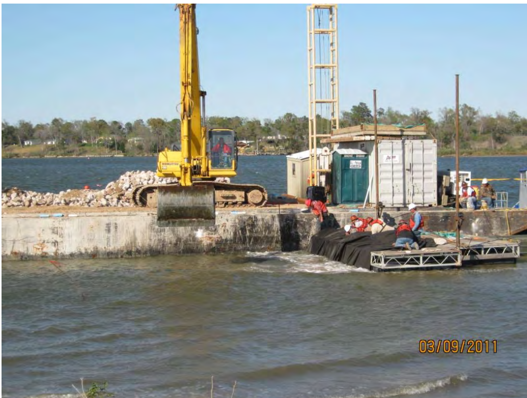
Photo 6 – Deploying geotextile and placing the Armor Cap D rock in the east cell
