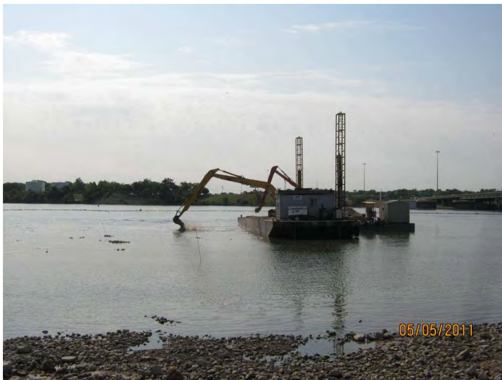
Photo 1 – Placing Armor Cap C rock in the Eastern Cell.
