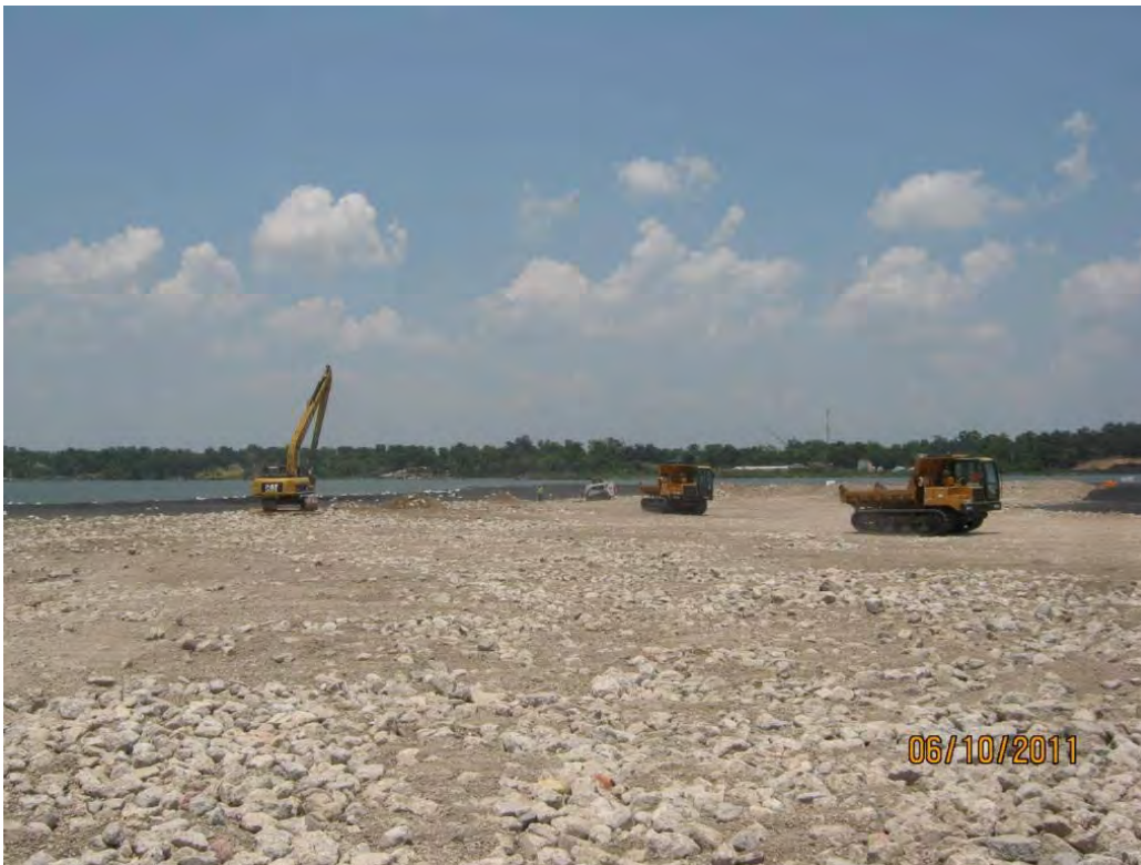
Photo 4 – Delivering and placing Armor Cap B/C rock in the Western Cell.
