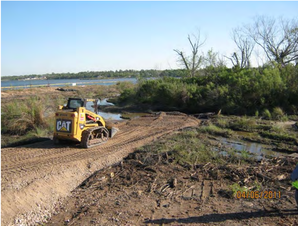
Photo 1 – Constructing access road into the center portion of the west cell.
