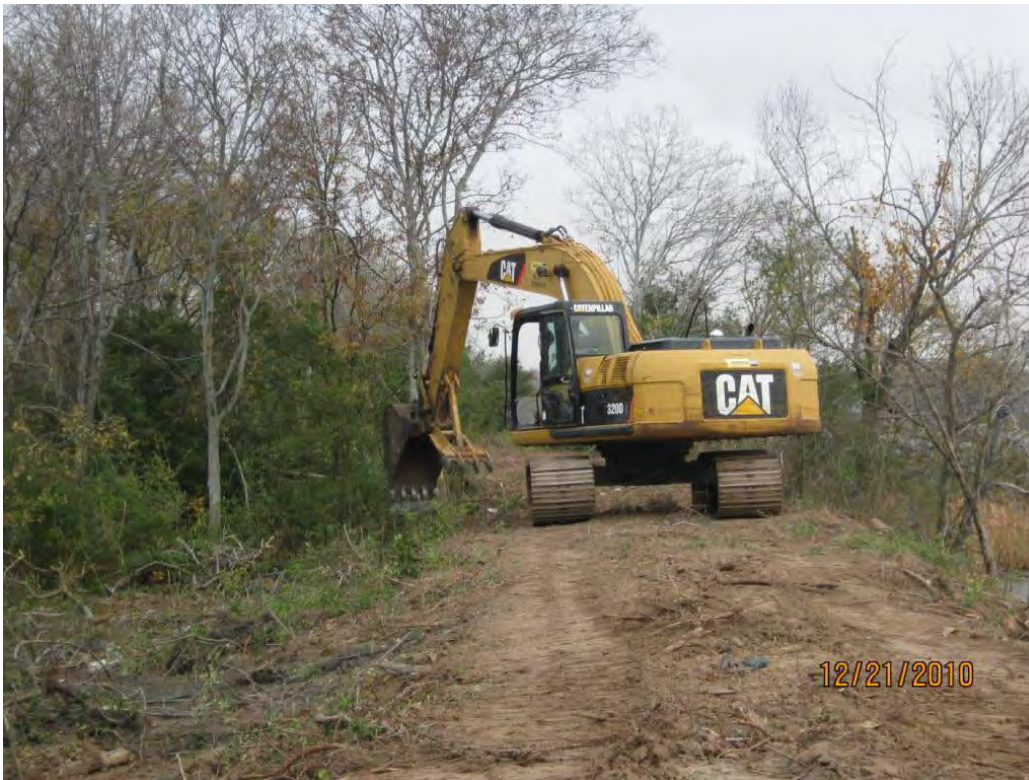
Photo 2 – Clearing vegetation from atop central berm, approximately 100 feet north of southern berm.
