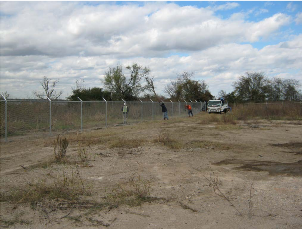
Photo 3 – Installing chain link for 6-foot fence along west edge of Big Star property.
