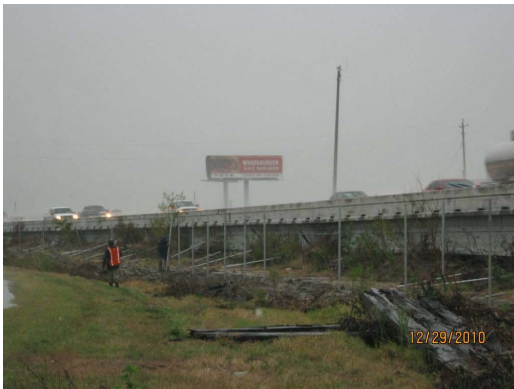
Photo 1 – Installing fence posts to south of I-10.
