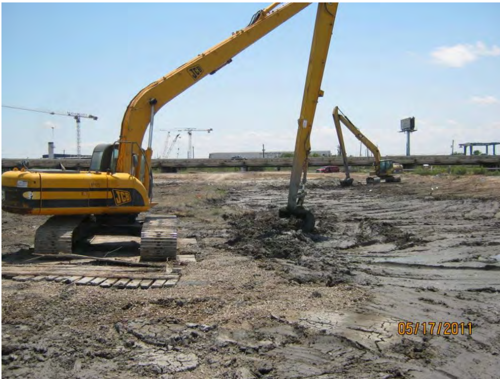
Photo 4 – Mixing Portland cement into a low-lying area in the northwest portion of the Western Cell.
