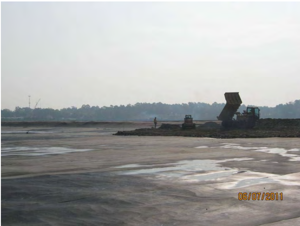
Photo 2 – Placing Armor Cap B/C rock near the central berm in the Western Cell.
