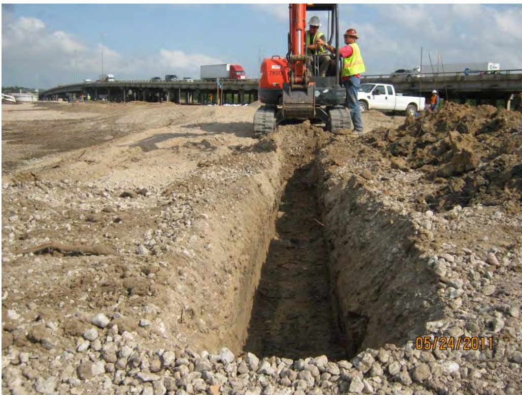
Photo 5 – Excavating a 2-foot deep anchor trench atop the berm near the southwest corner of the Western Cell.
