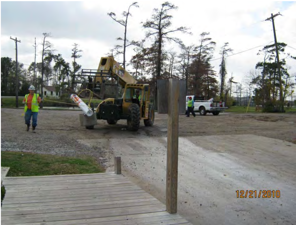
Photo 7 – Loading concrete anchor and regulatory buoy onto work boat using rubber-tired hydraulic forklift.
