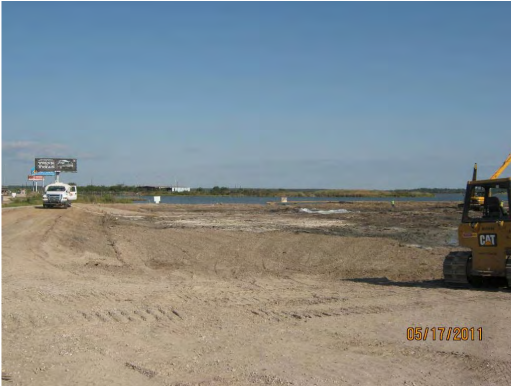
Photo 1 – Crushed concrete road base used to grade the surface of the Western Cell near the south berm.
