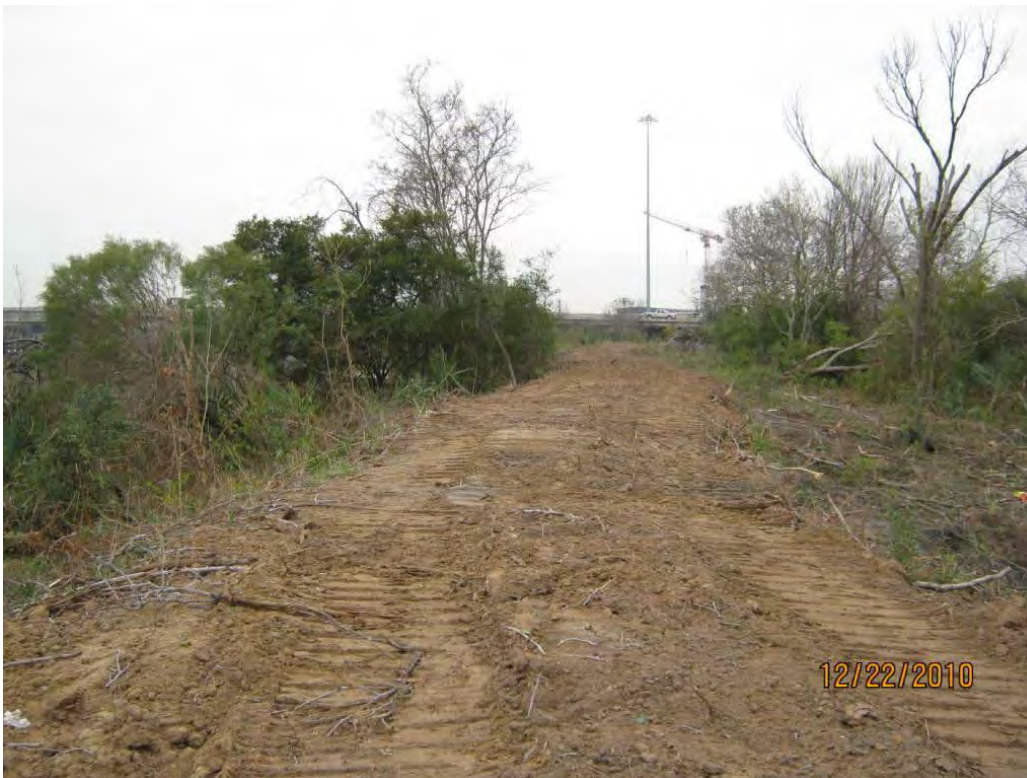
Photo 2 – Vegetation cleared from atop central berm, standing near north end of berm and looking south.
