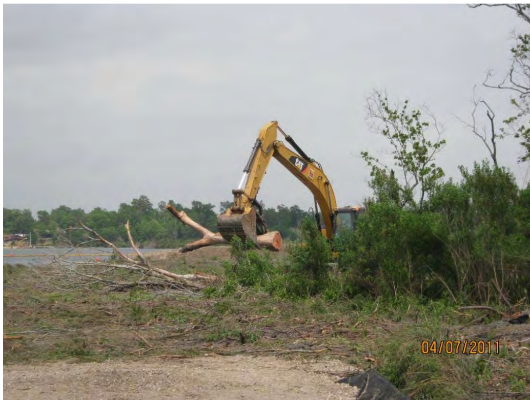
Photo 1 – Clearing vegetation in the central portion of the west cell; note the stump was removed from the tree.
