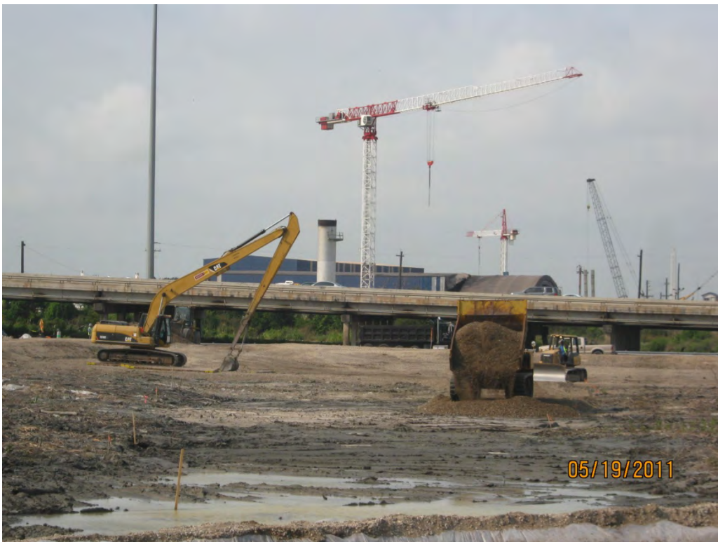
Photo 2 – Morooka truck unloading crushed concrete road base in the Western Cell.
