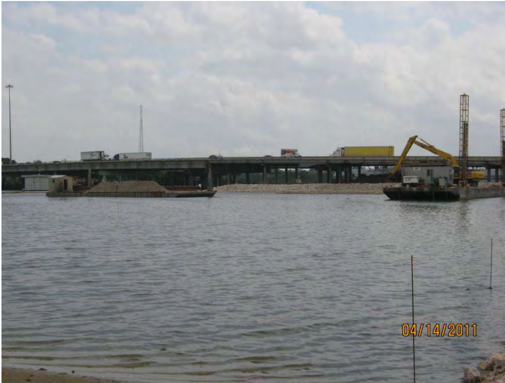
Photo 3 – Maneuvering aggregate transport barge to the west portion of the east cell, using a combination of a tug boat and a tow rope attached between the aggregate transport barge and the excavator.
