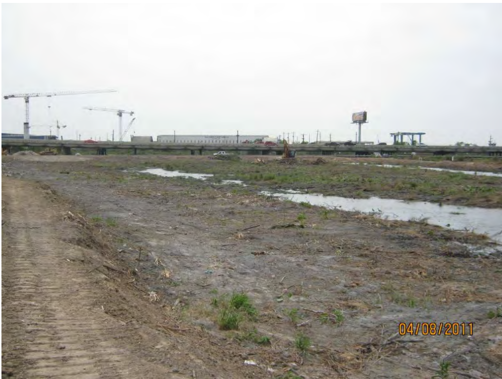
Photo 3 – West cell following the completion of clearing and grubbing, as viewed from the central berm.
