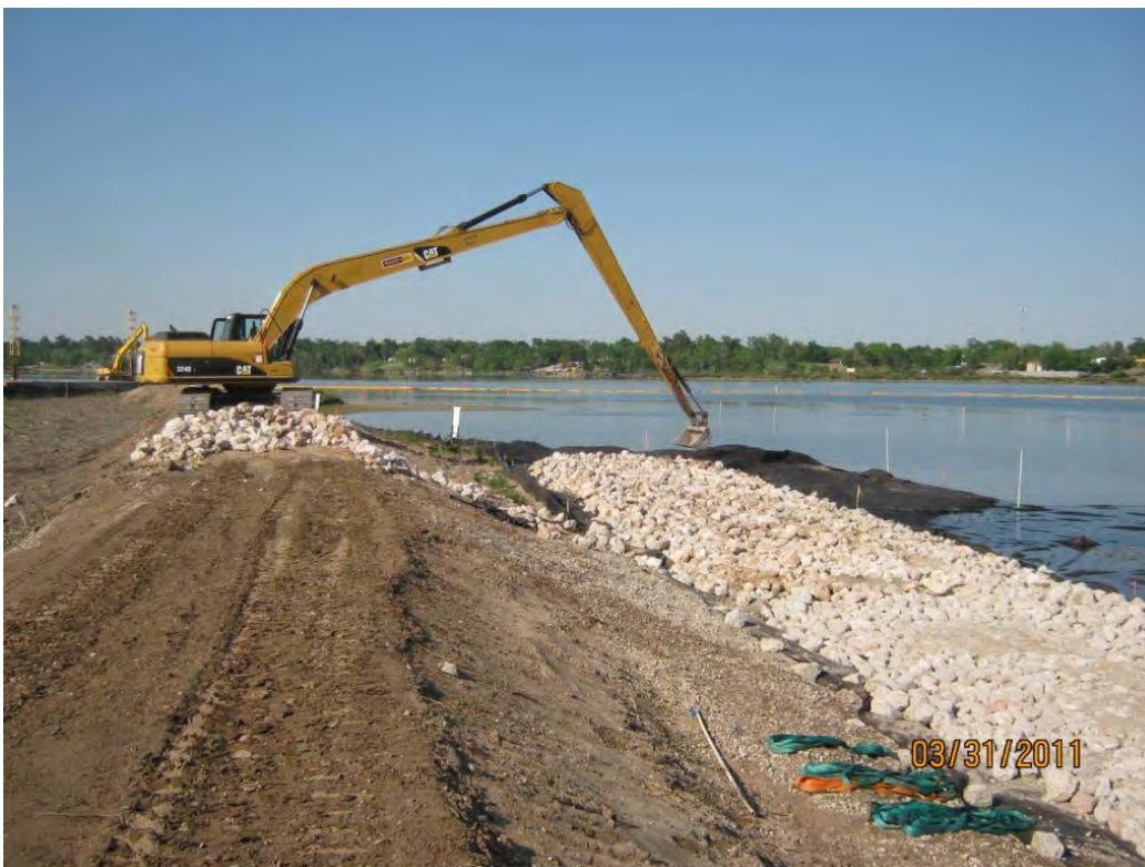
Photo 6 – Placing Armor Cap D rock on the east side of the central berm.
