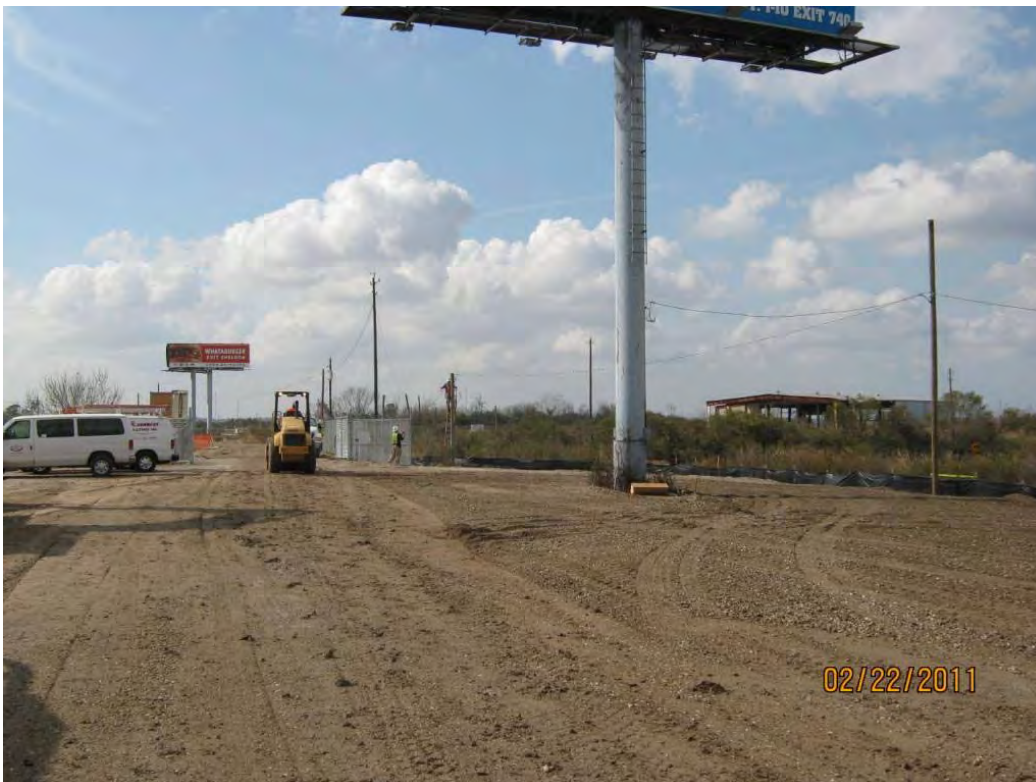
Photo 6 – Compacting CCRB at equipment laydown area and relocating power poles for billboards at the TxDOT ROW
