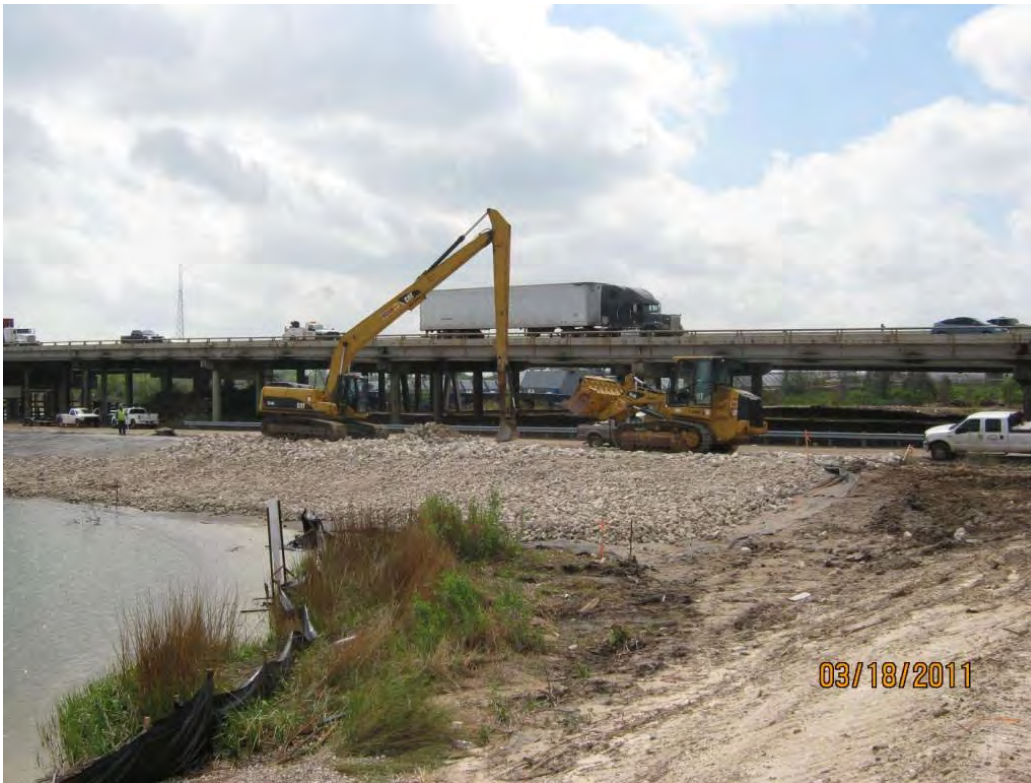
Photo 5 – Transporting Armor Cap B/C rock to the long-reach excavator for placement of rock on the south berm.
