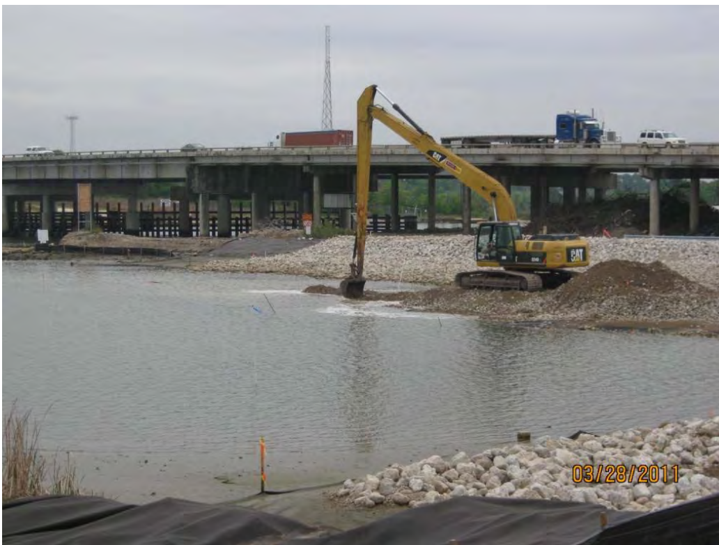
Photo 4 – Constructing a rock platform using Armor Cap A rock in the east cell.
