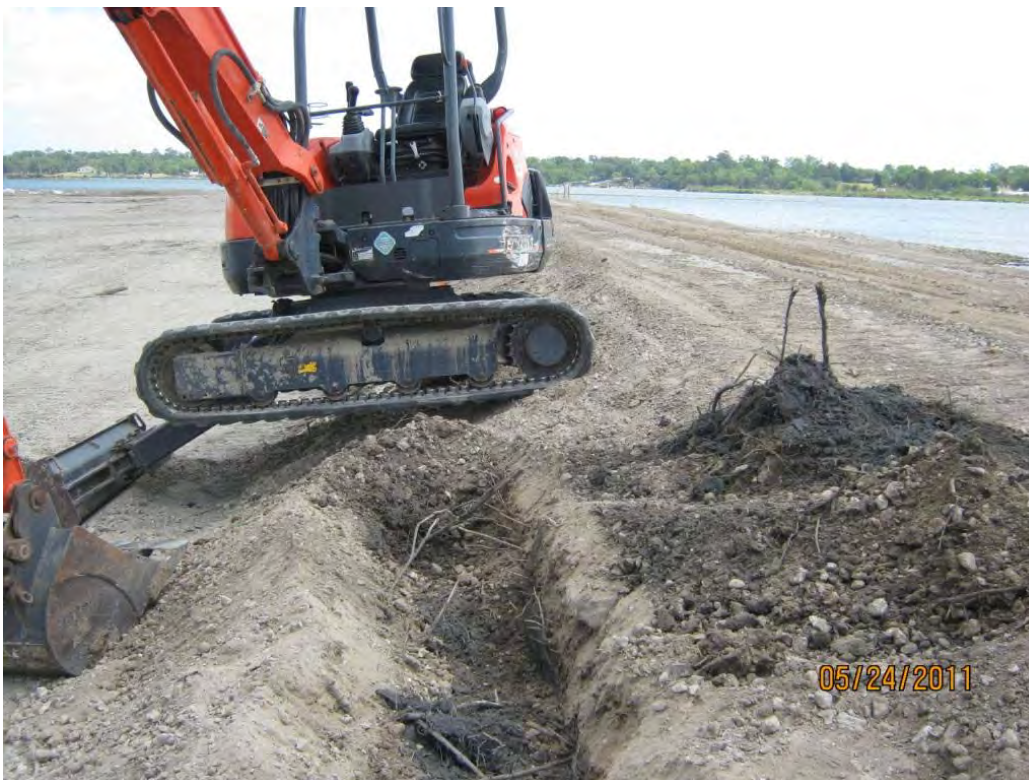
Photo 3 – Anchor trench for future geomembrane deployment on the inner slope of the central berm; due to encountering suspected paper mill sludge, the trench was filled in and relocated to the top of the central berm.
