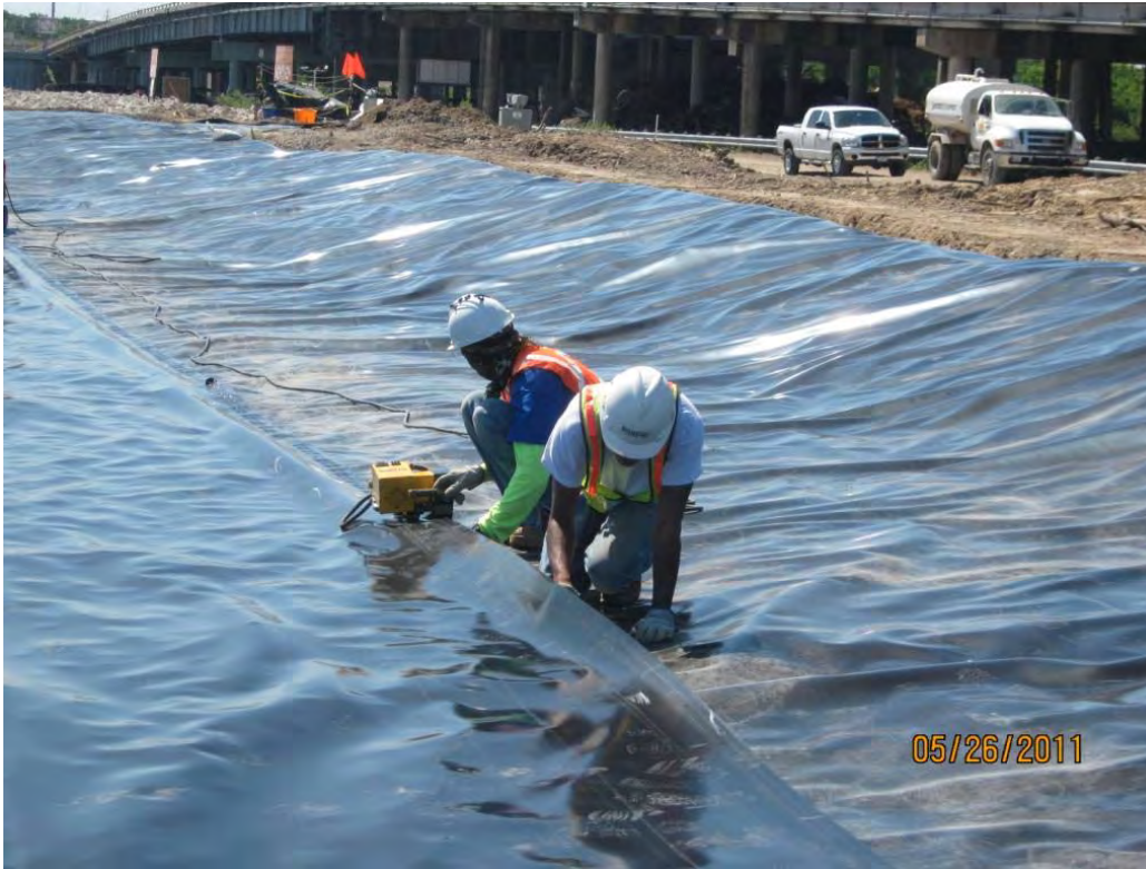
Photo 3 – Welding a double seam into two overlapping panels of LLDPE.
