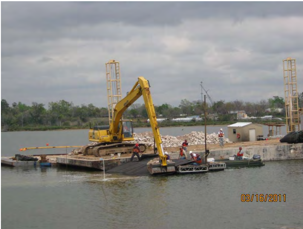
Photo 2 – Deploying geotextile and placing Armor Cap D rock in the east cell.
