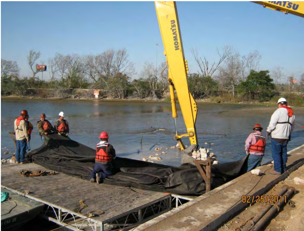
Photo 3 – Barge-mounted excavator placing Armor Cap D rock atop geotextile in east cell
