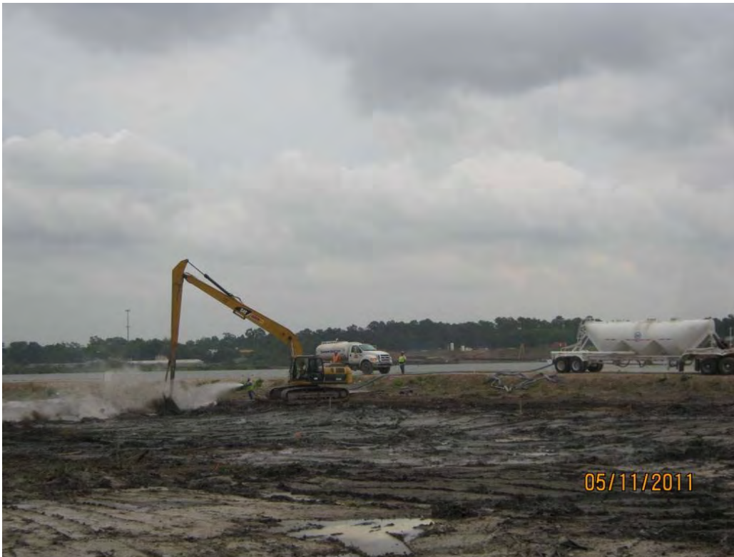
Photo 1 – Delivering Portland cement to the Western Cell and spraying with water hose to mitigate dust generation.
