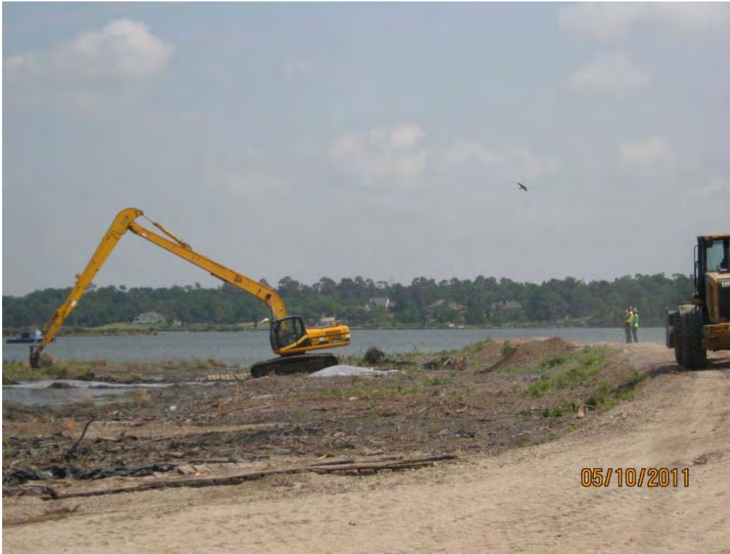
Photo 3 – Constructing an interim berm in the eastern portion of the Western Cell.
