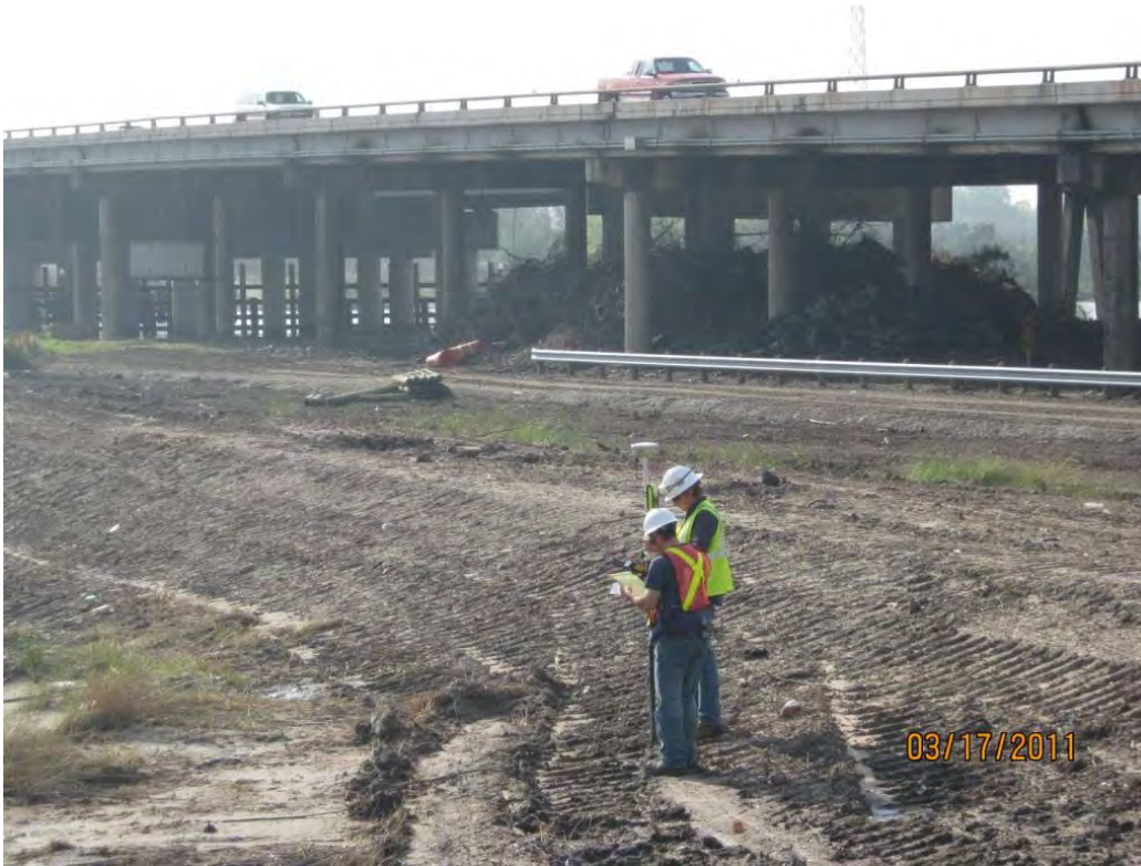
Photo 1 – Surveying the south berm of the east cell prior to placement of Armor Cap A material.
