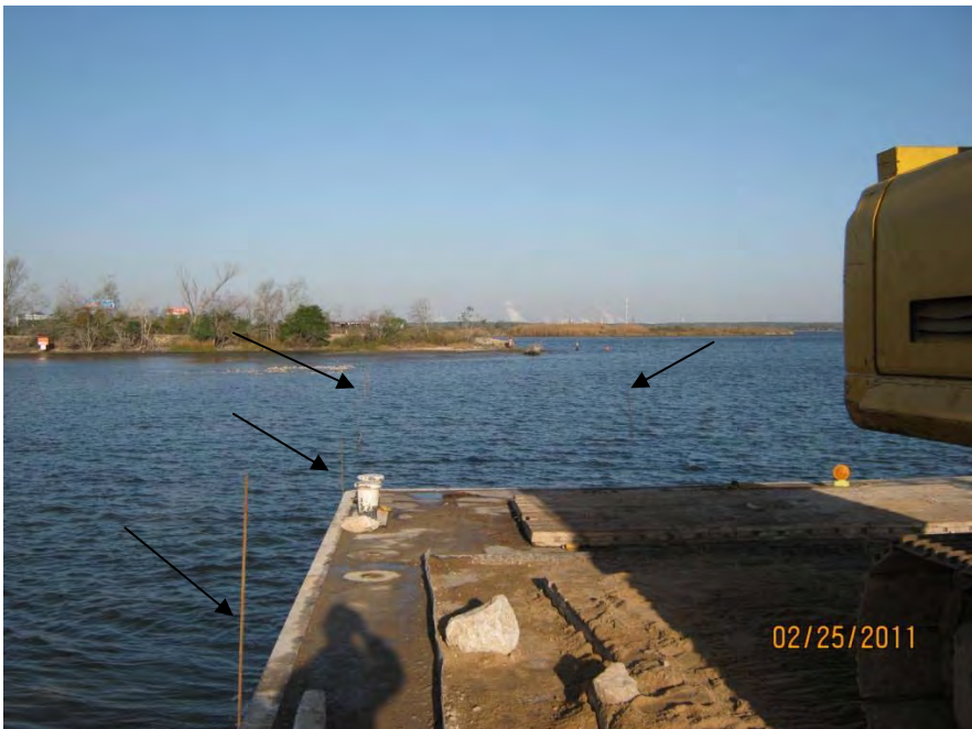
Photo 2 – Rebar placed at surveyed locations to guide barge-mounted excavator into proper position for rock placement
