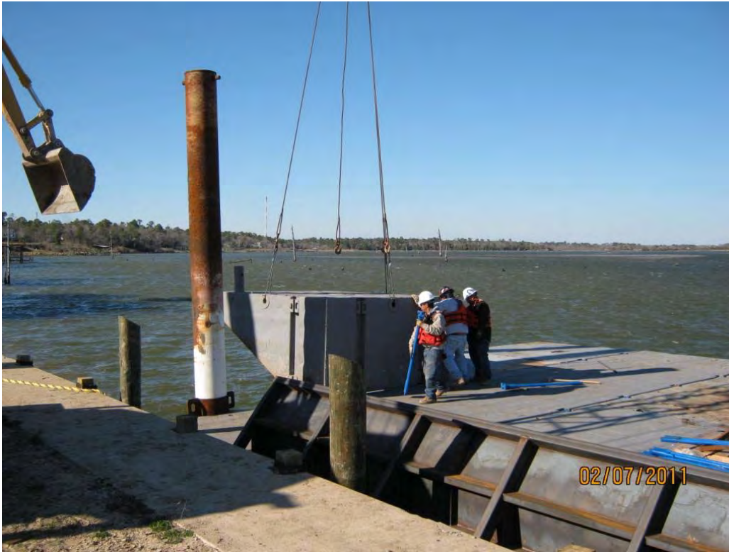
Photo 5 – Placing bow portion of sectional barge using crane and crew with barge pins (painted blue steel)
