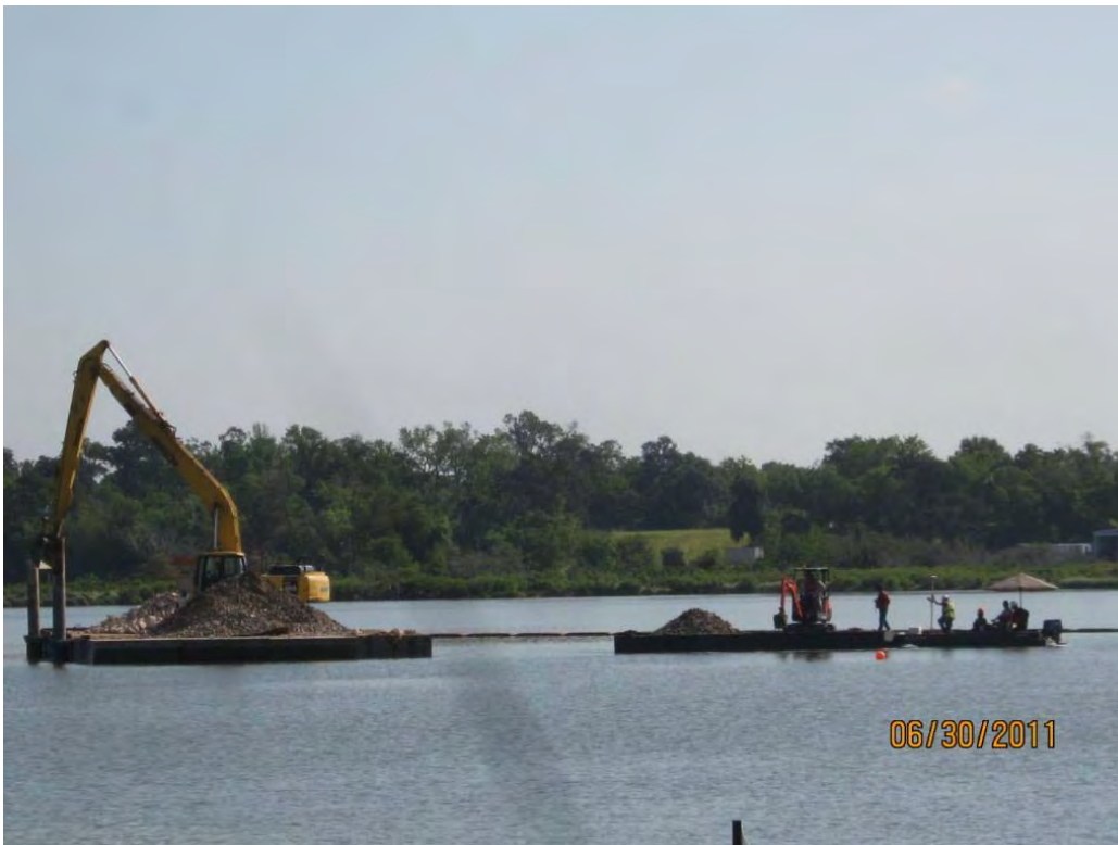
Photo 2 – Mini-barge loaded with Armor Cap A rock for placement in the Eastern Cell.
