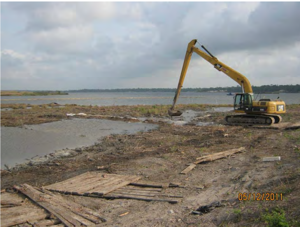
Photo 2 – Breaking an opening into the interim berm to allow the tide to recede in the Western Cell.
