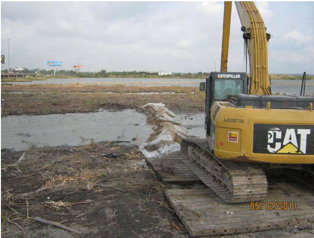
Photo 3 – Breaking an opening into the interim berm to allow the tide to recede in the Western Cell.
