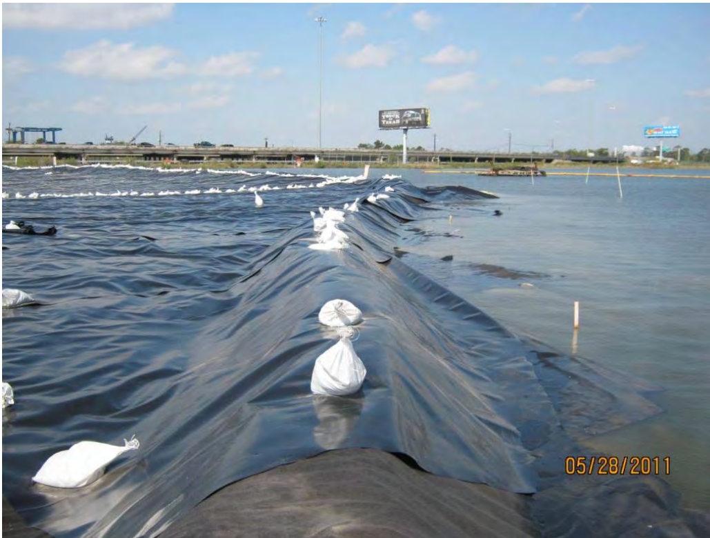
Photo 3 – LLDPE liner extended over the northern berm in the Western Cell and held in place by sand bags.
