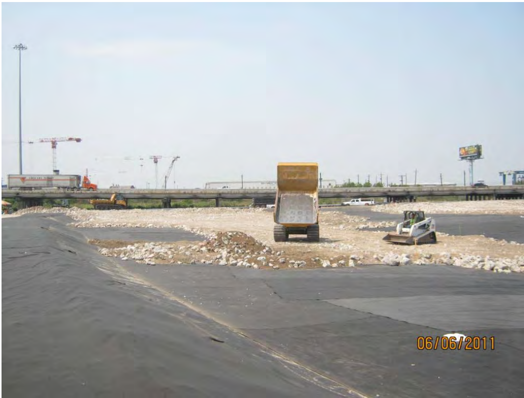
Photo 2 – Placing Armor Cap B/C rock near the central berm in the Western Cell.
