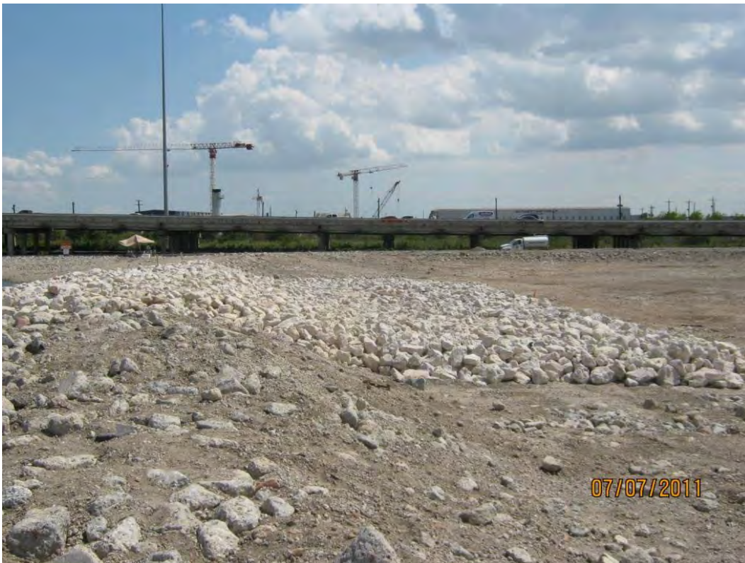
Photo 4 – 24-inch thick layer of Armor Cap D rock placed in the Western Cell; Armor Cap B/C in foreground of photo.
