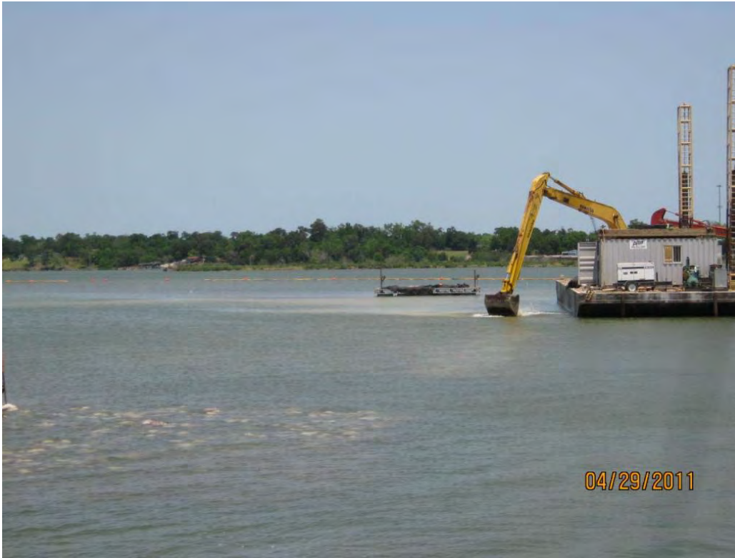
Photo 3 – Placing Armor Cap D rock placed in the east cell; note previously placed Armor Cap D rock visible just under the water surface in the foreground of the photo.
