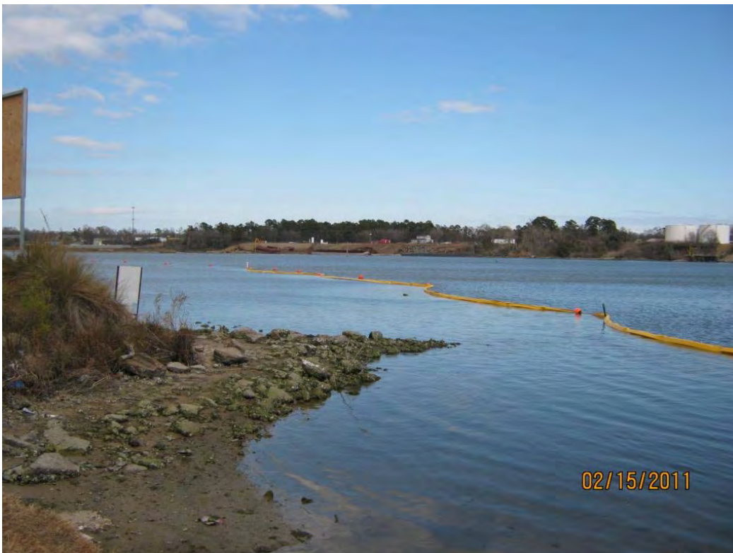
Photo 4 – Approximately 400 feet of turbidity curtain deployed at south portion of east cell; deployment is ongoing
