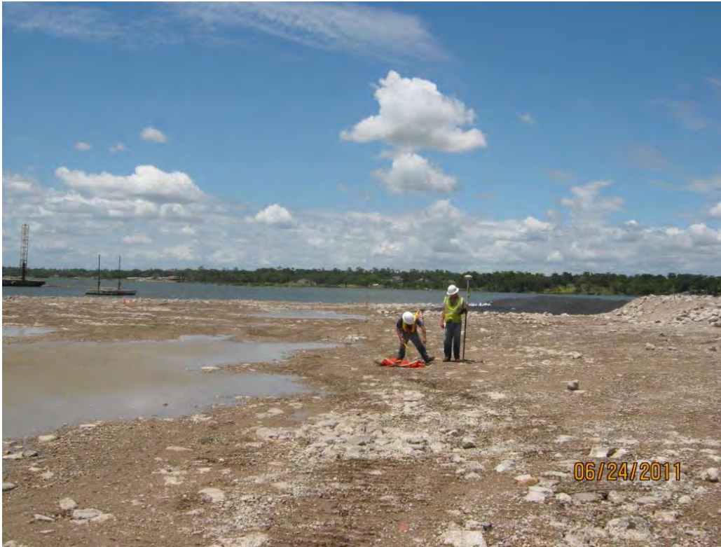
Photo 3 – Surveyors probing the thickness of Armor Cap B/C rock in the Western Cell.
