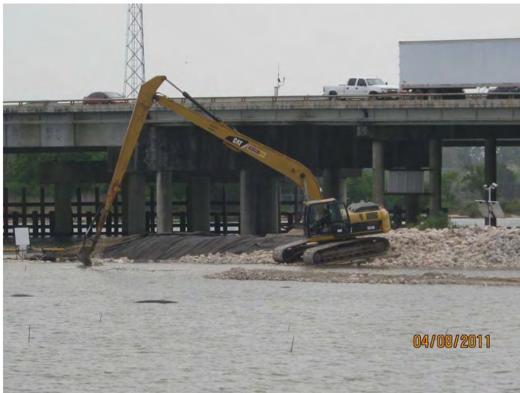
Photo 1 – Placing Armor Cap B/C rock in the east cell.
