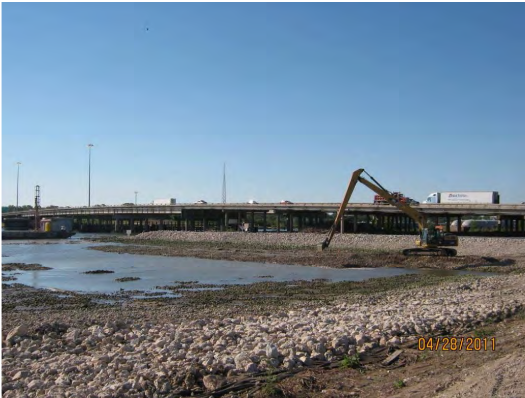
Photo 1 – Placing Armor Cap A rock in the east cell by removing rock finger roadway into the east cell.
