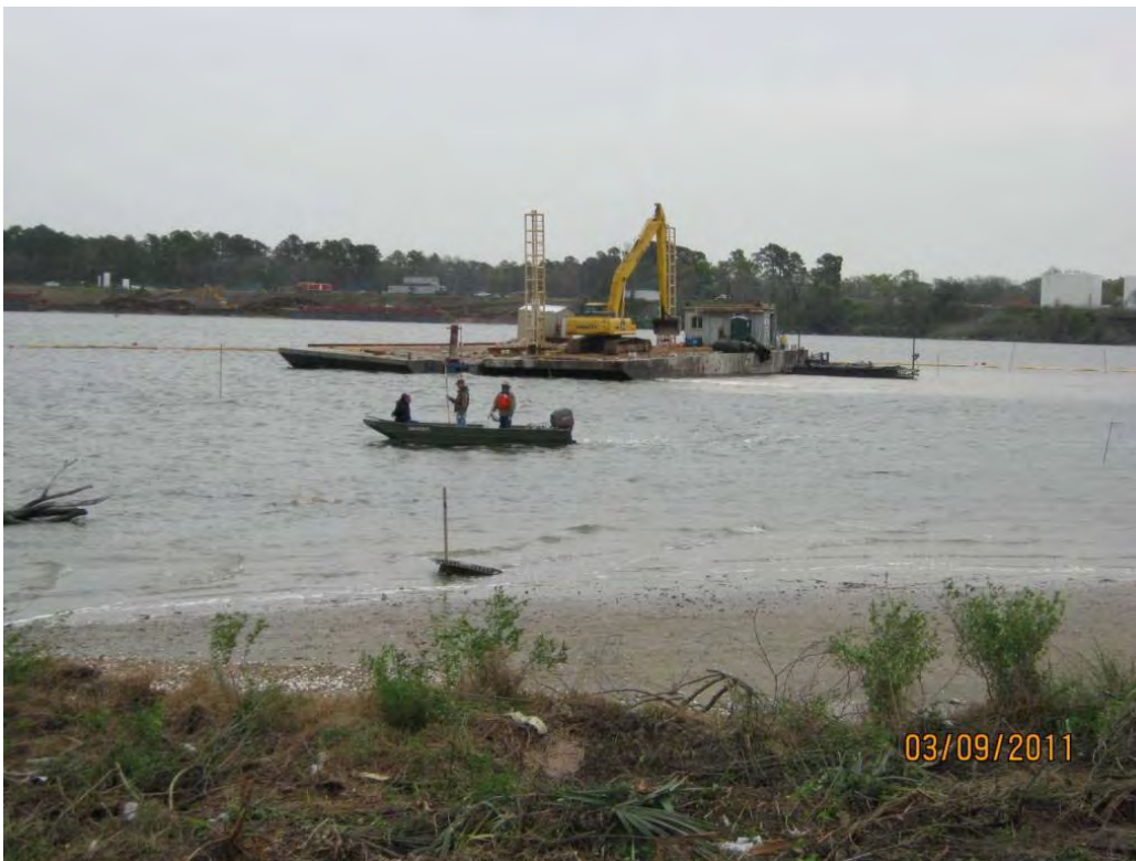
Photo 2 – Progress surveying (foreground) and placing Armor Cap D rock (background) in the east cell
