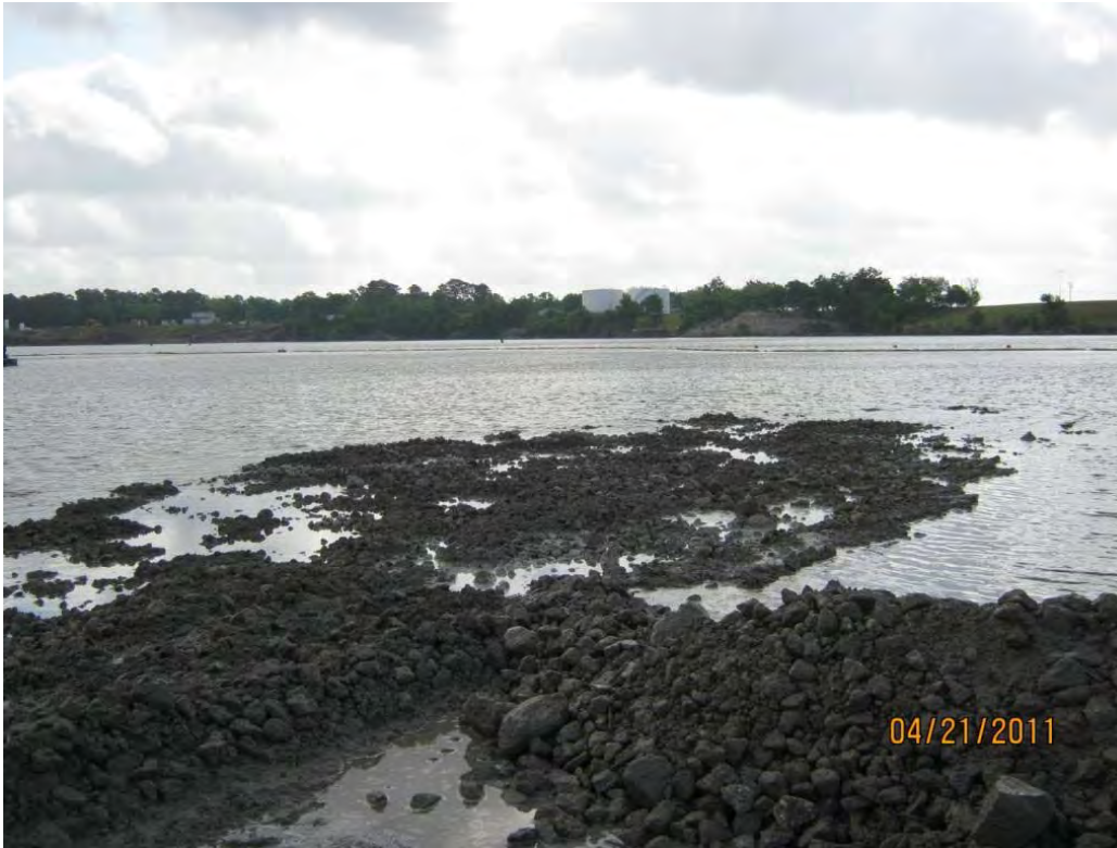
Photo 1 – Armor Cap A rock placed in the east cell by casting material from the rock access bridge from side to side.
