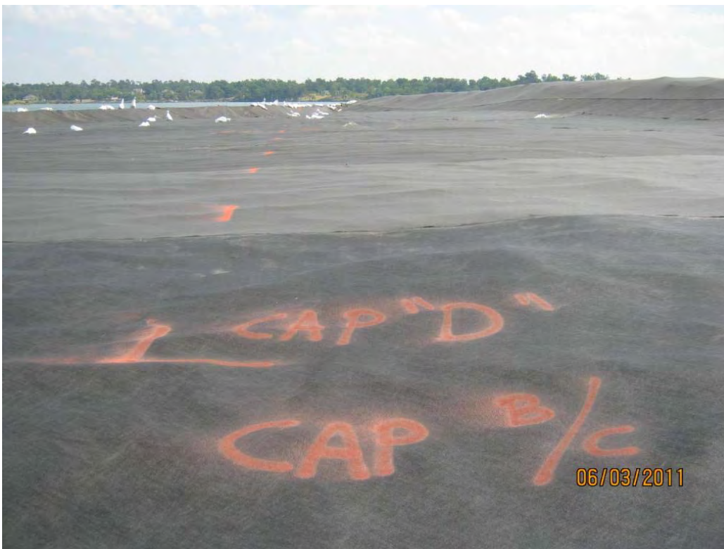
Photo 4 – Transition area between Armor Cap B/C and D rock marked by surveyors in the Western Cell.
