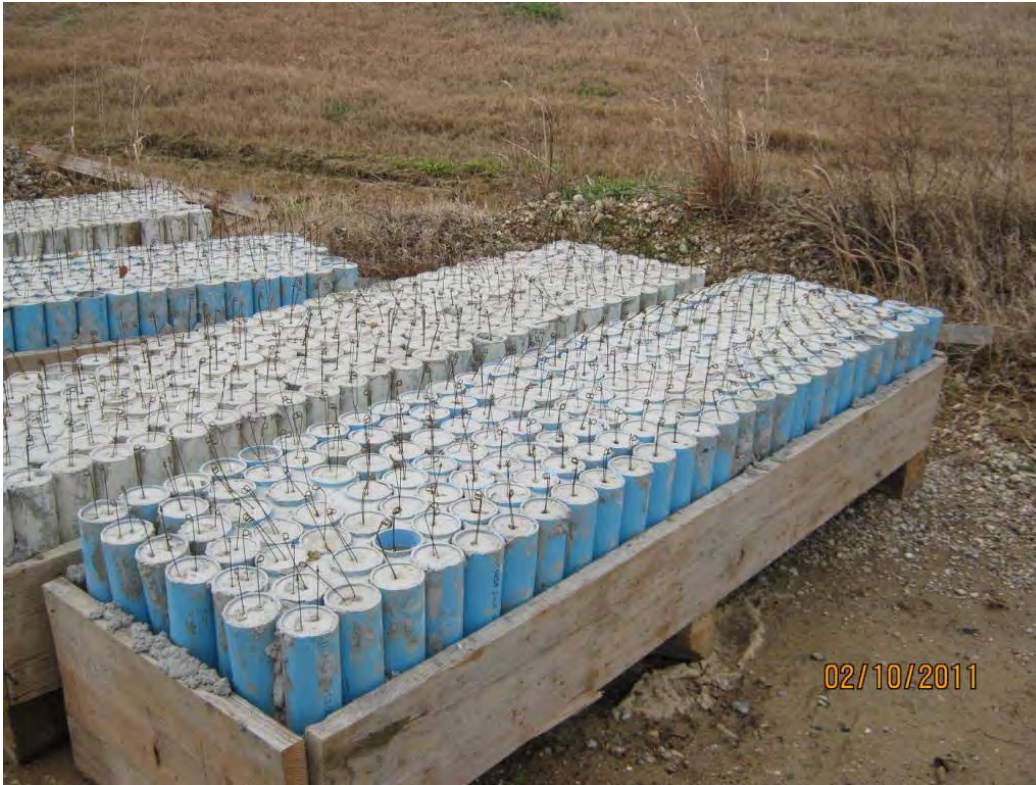
Photo 3 – Concrete weights for future use in placing geotextile under water in eastern cell
