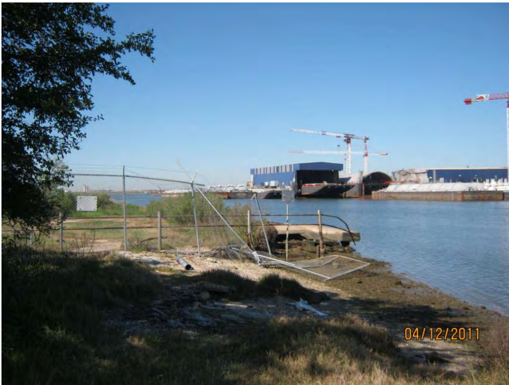
Photo 4 – Damage to the fence caused by a barge at the TxDOT property on the east side of the San Jacinto River.
