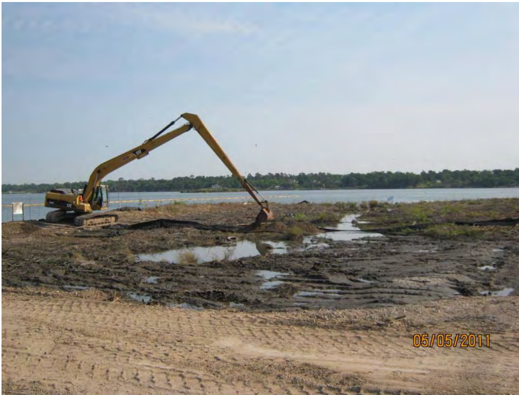
Photo 2 – Installing an interim berm in the Western Cell using crushed concrete road base and geotextile.
