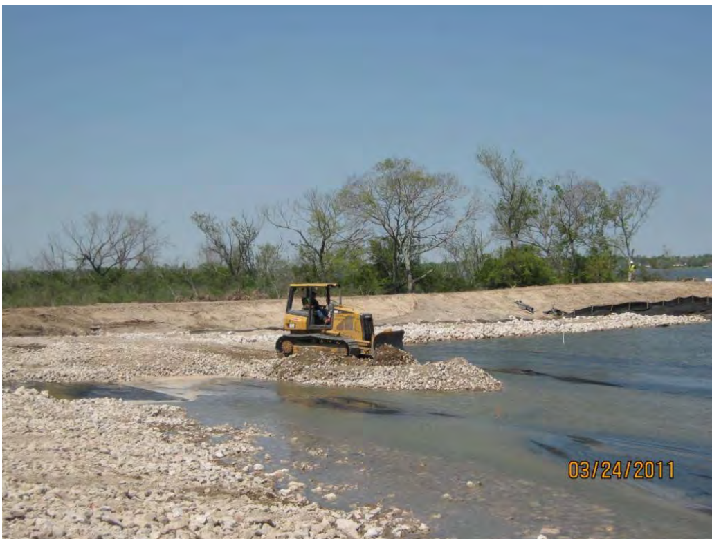
Photo 2 – Constructing a rock platform in the east cell to be used for armored cap placement.
