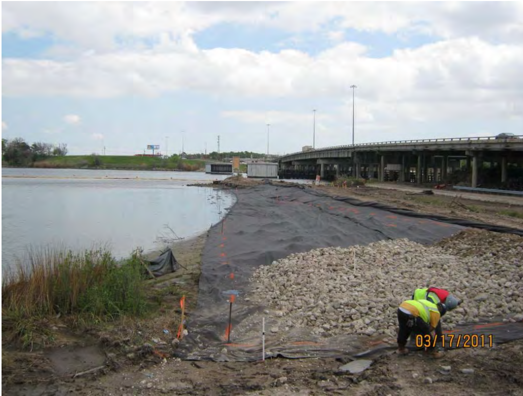
Photo 7 – Placing Armor Cap A on the south berm of the east cell.
