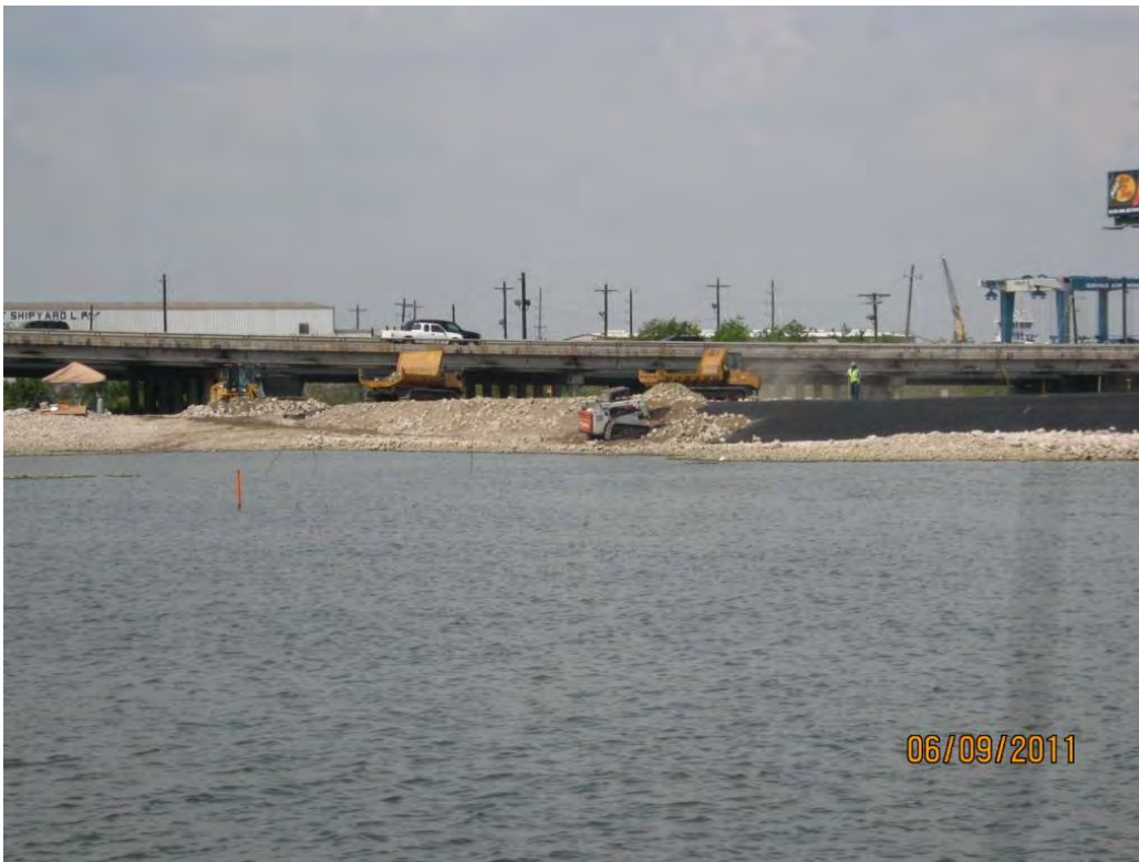
Photo 2 – Placing Armor Cap B/C rock on the eastern slope of the central berm using a skidsteer.
