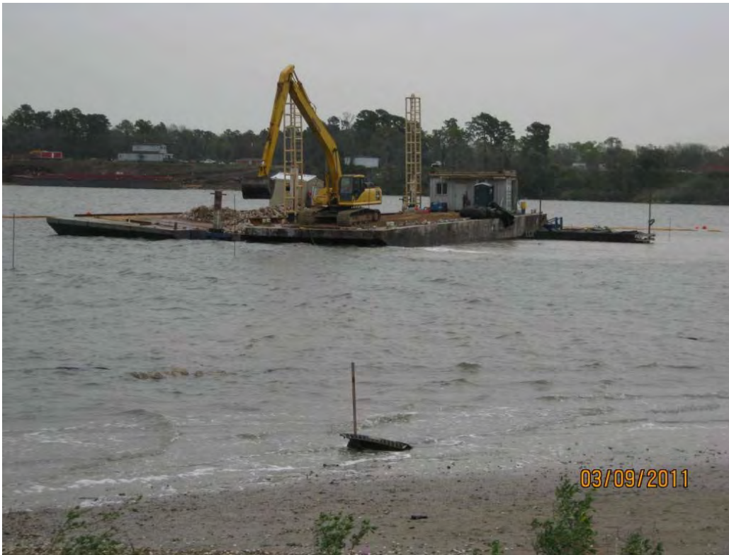
Photo 1 – Placing Armor Cap D rock in the east cell; survey poles marking the rock placement area at left of photo
