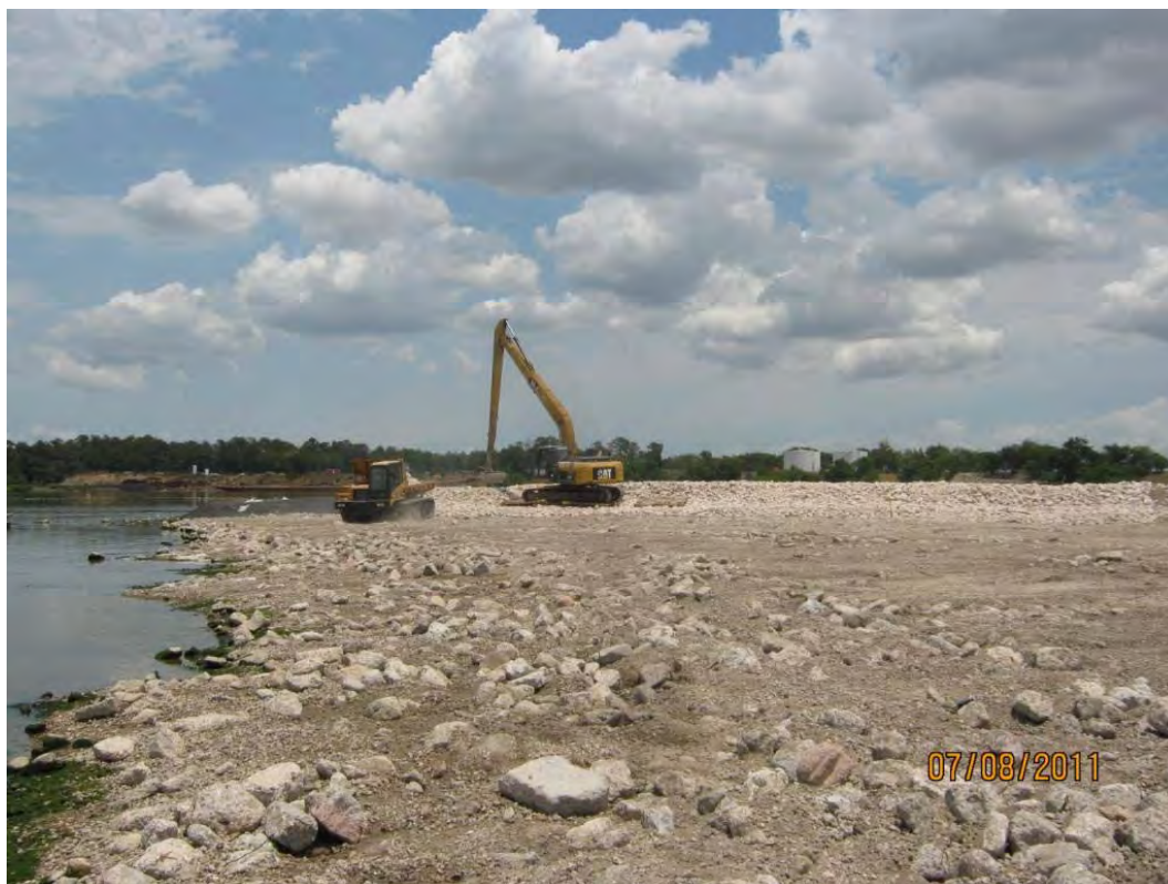
Photo 1 – Delivering Armor Cap D rock to the long-reach excavator for placement in the Western Cell.
