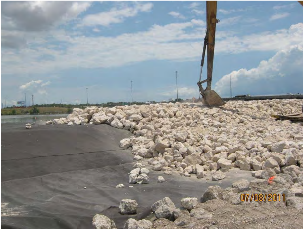
Photo 2 – Placing Armor Cap D rock along the central berm in the Western Cell.
