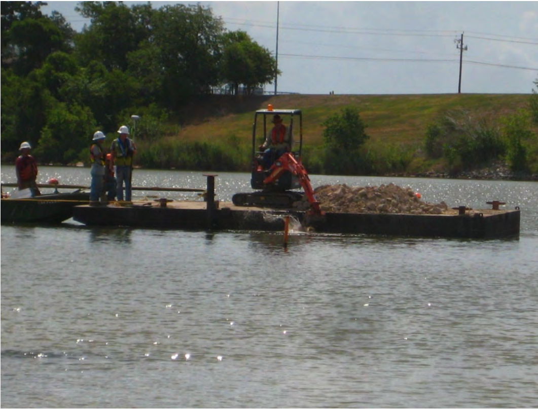
Photo 1 – Mini-excavator placing Armor Cap A rock in a shallow water area in the Eastern Cell.
