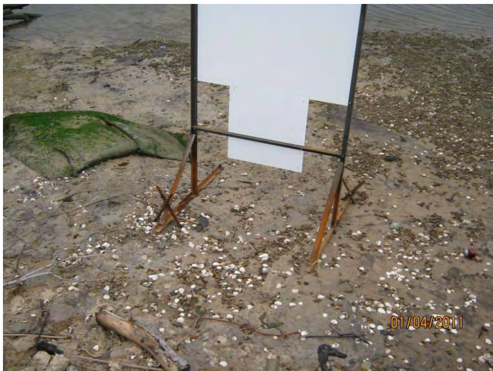
Photo 2: Stakes installed on signs to securely anchor the sign posts to the ground
