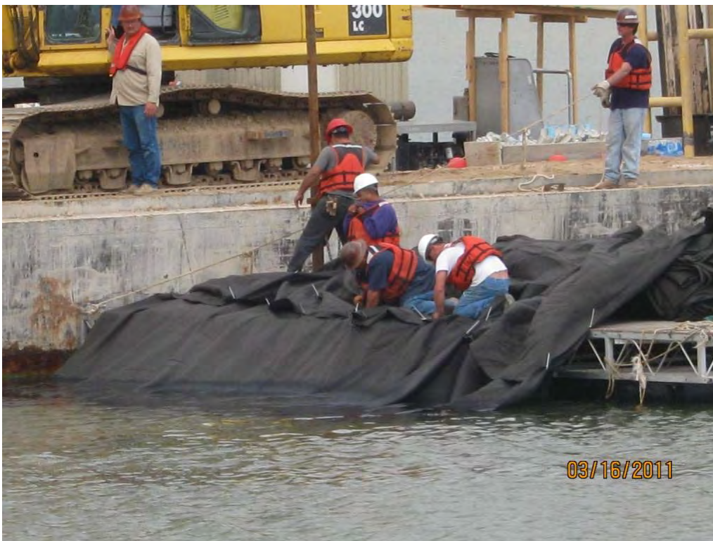
Photo 3 – Consecutive panels of geotextile tied together.
