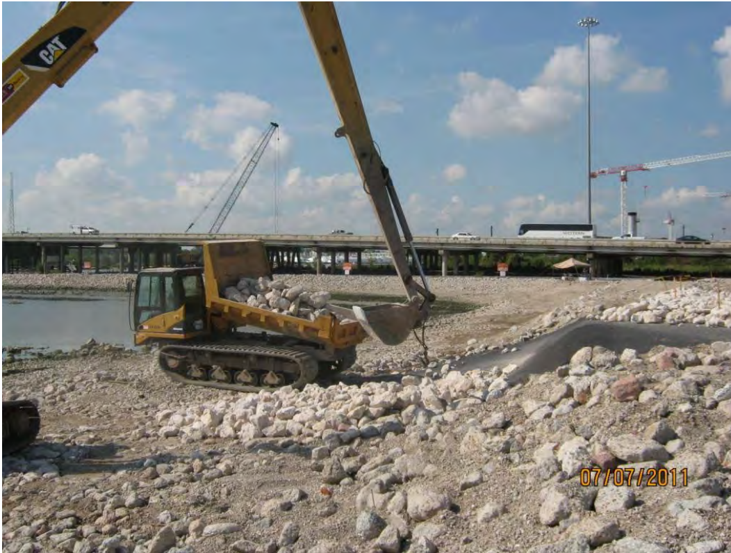
Photo 3 – Delivering and placing Armor Cap D rock on the eastern slope of the central berm.
