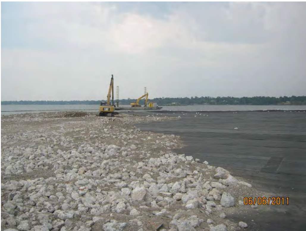
Photo 3 – Placing Armor Cap B/C rock near the west berm in the Western Cell.
