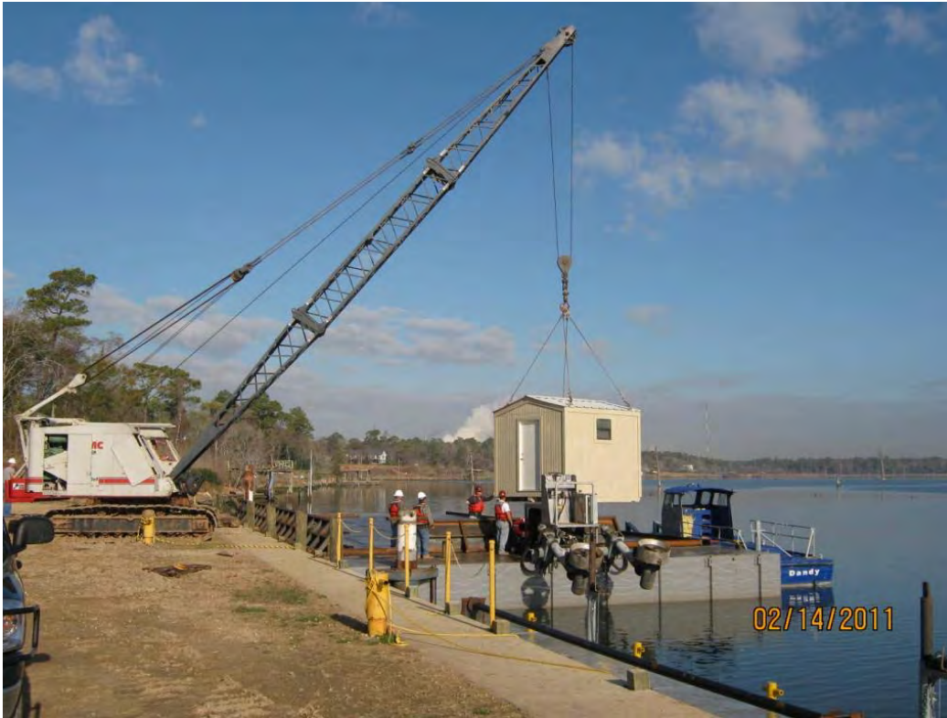
Photo 1 – Placing 10' x 10' weather shed on aggregate transport barge
