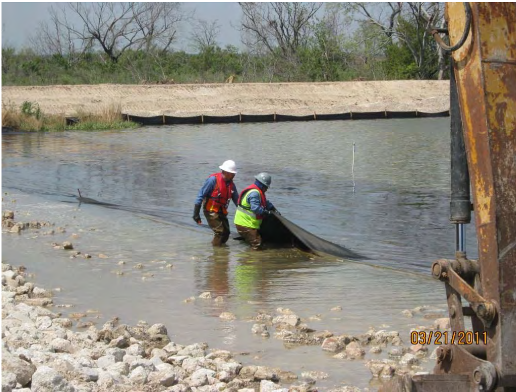
Photo 3 – Deploying geotextile to have a 3-foot overlap with the adjoining panel of geotextile.
