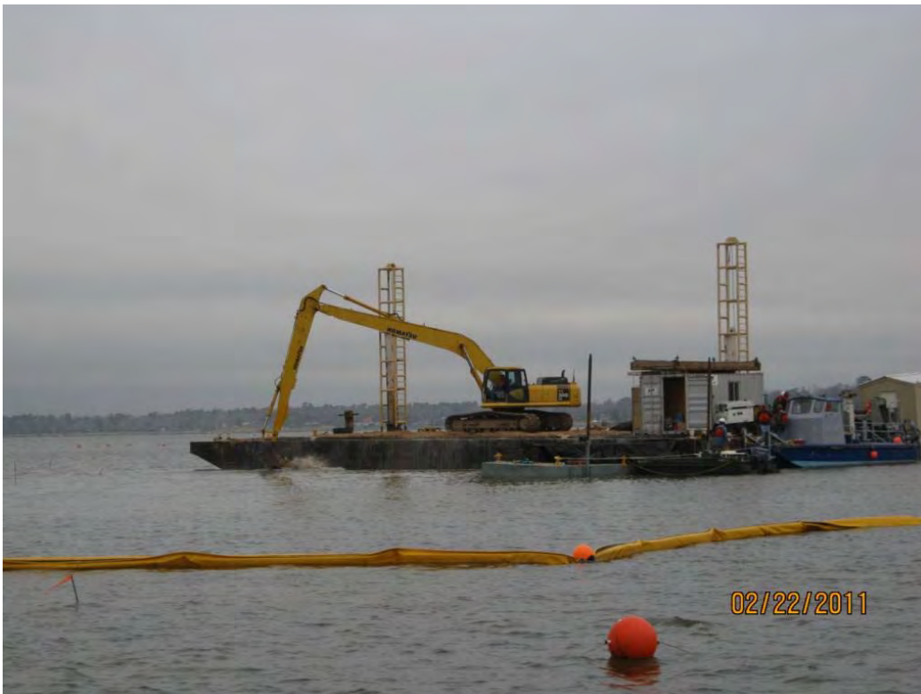
Photo 2 – Placing Armor Cap D rock in the east cell, as viewed from work boat outside the turbidity curtain
