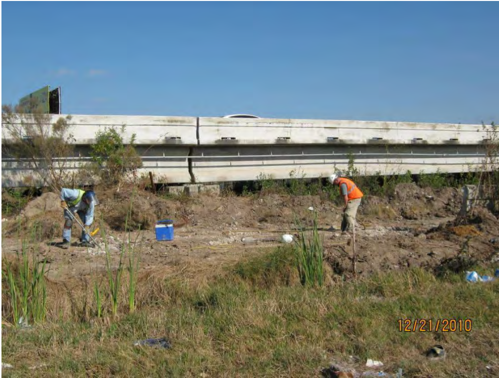
Photo 5 – Clearing concrete from future fence post holes for Phase II fence line south of I-10.
