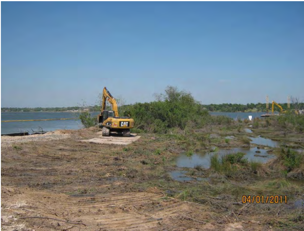
Photo 1 – Smoothing the ground surface in the west cell in preparation for geotextile deployment.
