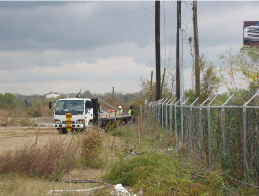
Photo 3 – Installing brackets along top of existing fence for installation of razor wire strands.
