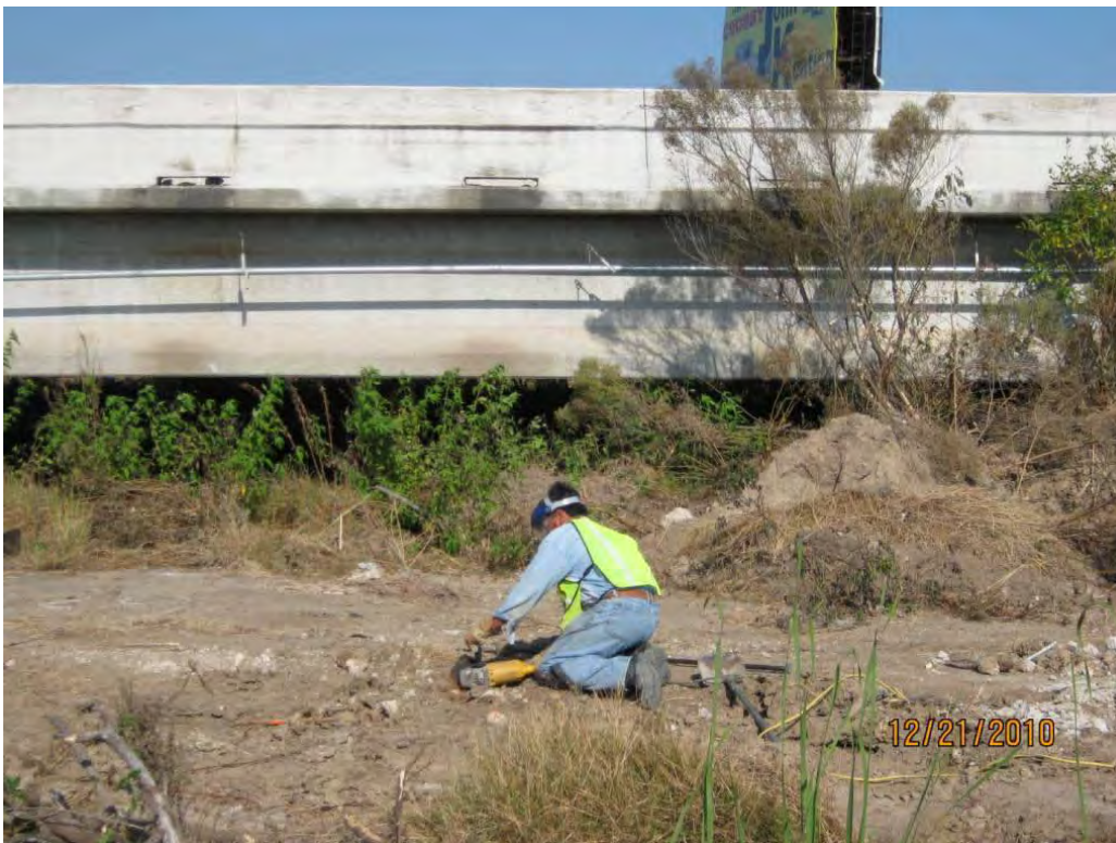
Photo 6 – Cutting rebar from future fence post hole for Phase II fence line south of I-10.
