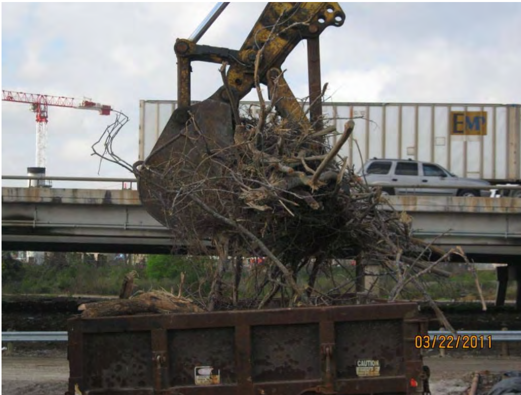
Photo 5 – Loading the vegetative debris originating from the above-ground vegetation in the west cell into a roll-off box for eventual disposal at the Atascocita Landfill in Humble, TX.
