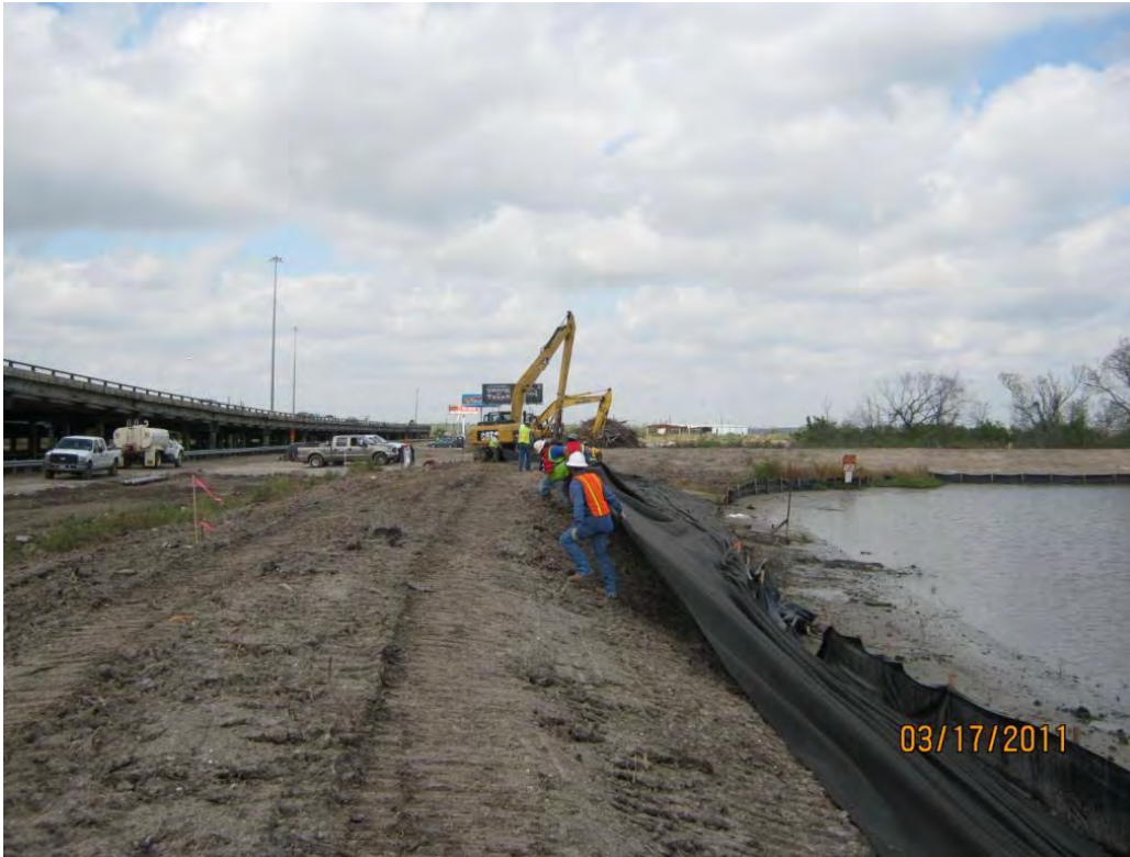
Photo 5 – Deploying geotextile on the south berm of the east cell for land-based placement of Armor Cap A.
