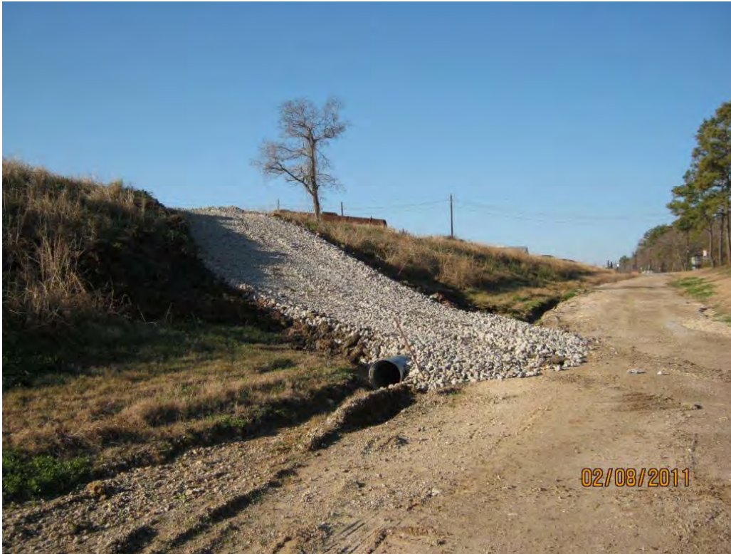
Photo 1 – Approximately 150-foot long access road installed at LaBarge Property from rock stockpile to dock area
