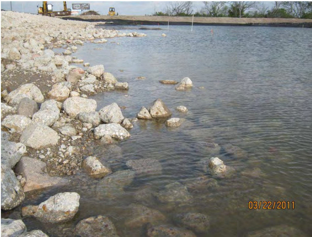
Photo 3 – Armor Cap B/C rock placed adjacent to south berm in east cell; minor additional work may be necessary to establish a uniform thickness (12-inch minimum).
