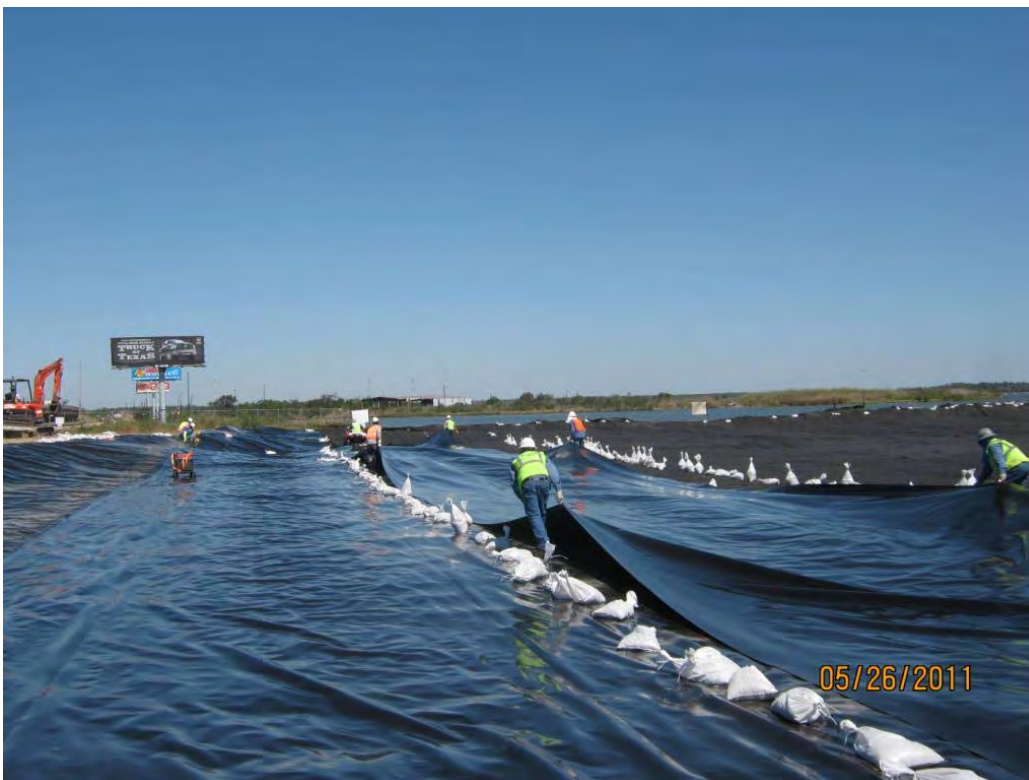
Photo 2 – Deploying LLDPE liner in the Western Cell.
