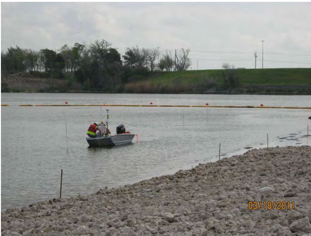
Photo 2 – Surveyors staking locations for future rock placement areas.
