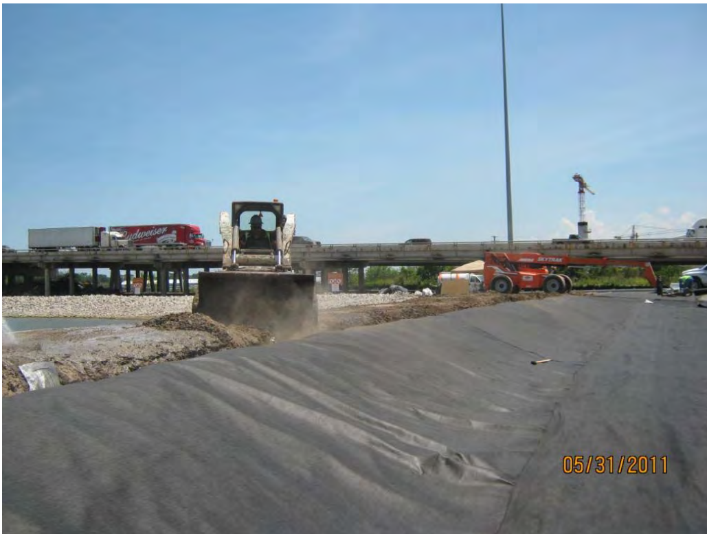
Photo 3 –Filling in the anchor trench atop the central berm following deployment of the 16-oz geotextile in the anchor trench.
