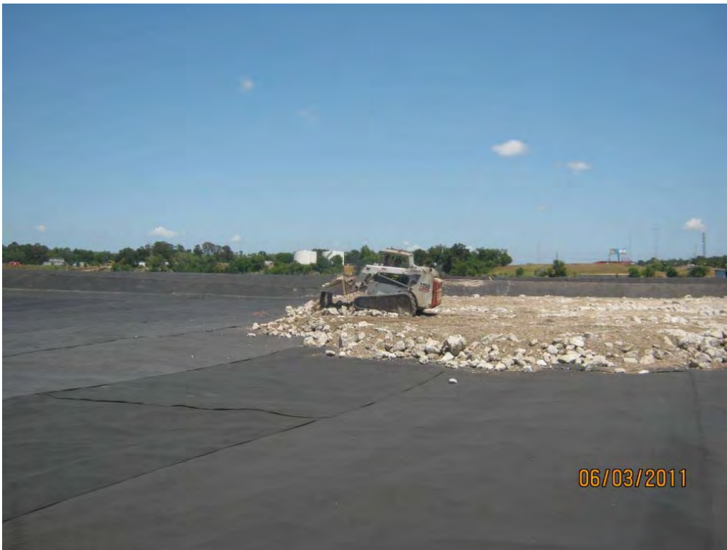
Photo 6 – Skidsteer placing Armor Cap B/C rock in east portion of the Western Cell.
