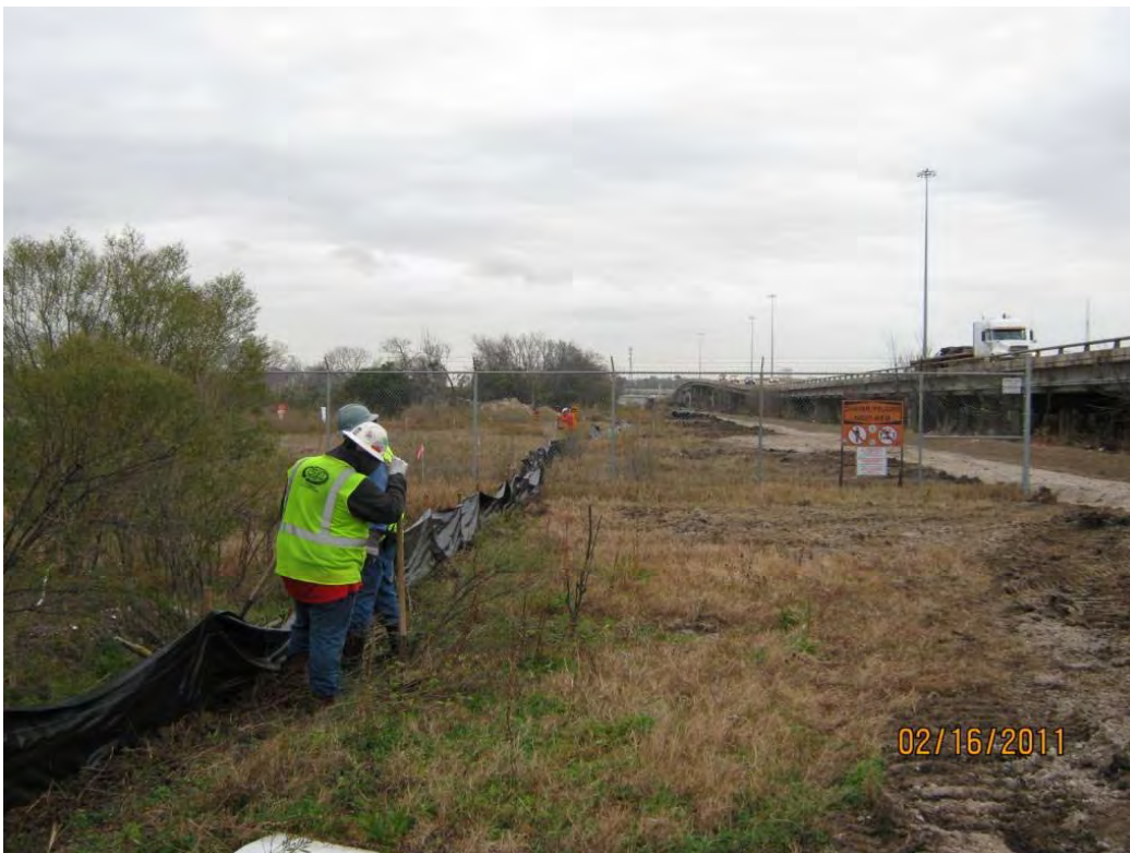
Photo 2 – Relocating a portion of the silt fence along the north border of TxDOT ROW
