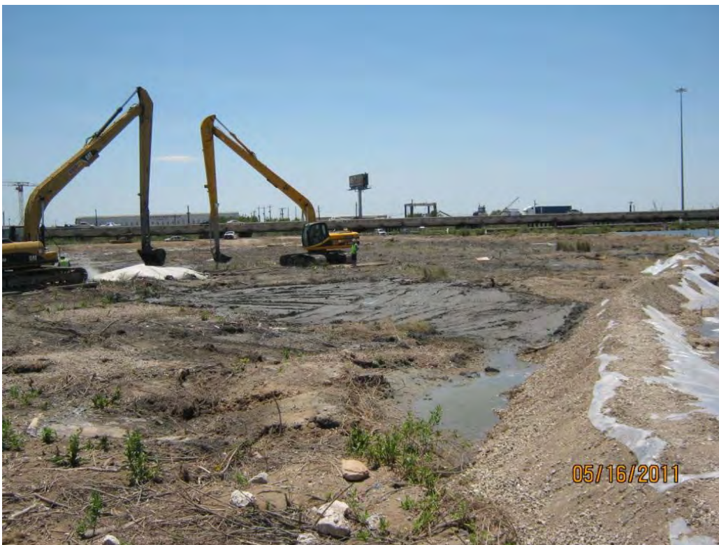
Photo 4 – Low-lying area of the Western Cell shortly after mixing with Portland cement (center of photo) and receiving Portland cement in the Western Cell (under plastic sheeting at left of photo).
