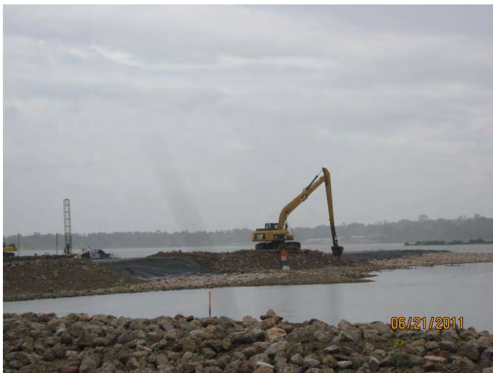
Photo 1 – Placing Armor Cap B/C rock along the central berm; uncovered area to left of excavator will receive Armor Cap D.
