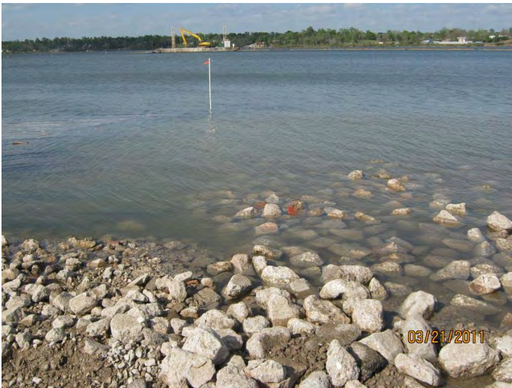
Photo 6 – Armor Cap B/C rock placed atop geotextile in the east cell.
