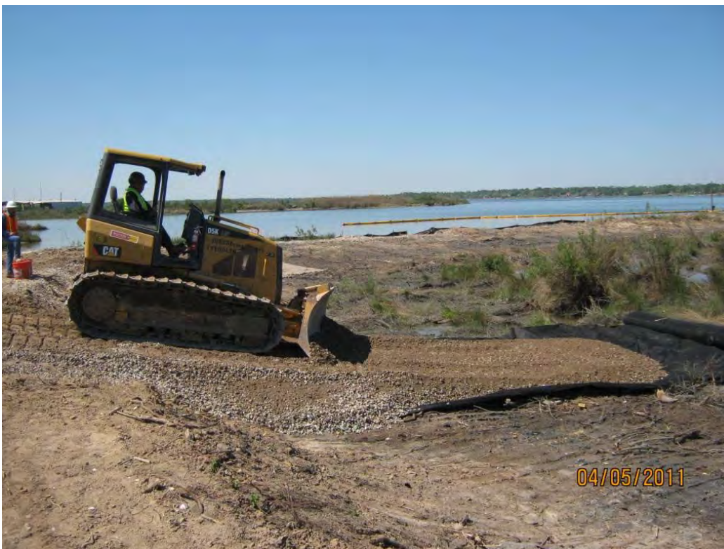
Photo 4 – Constructing an access road to the center of the west cell using geogrid and CCRB.
