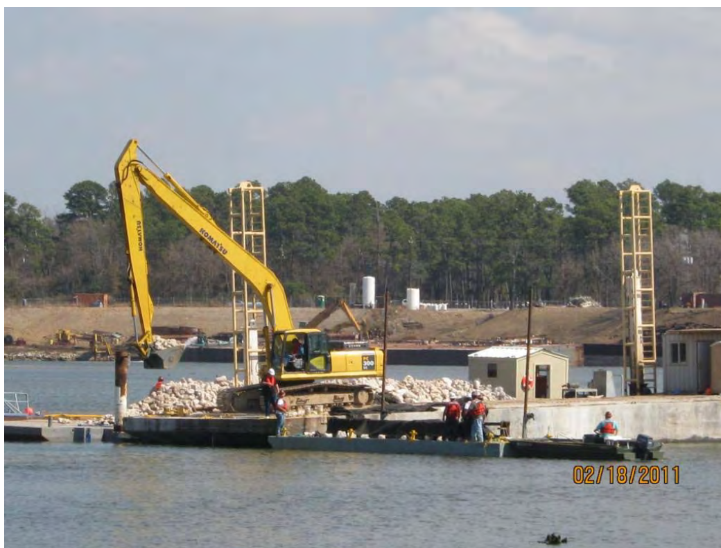
Photo 1 – Preparing to deploy geotextile using rock as weights, and place Armor Cap D rock atop geotextile
