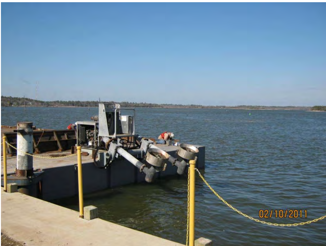
Photo 6 – Welding rope cleat onto starboard side of aggregate transport barge
