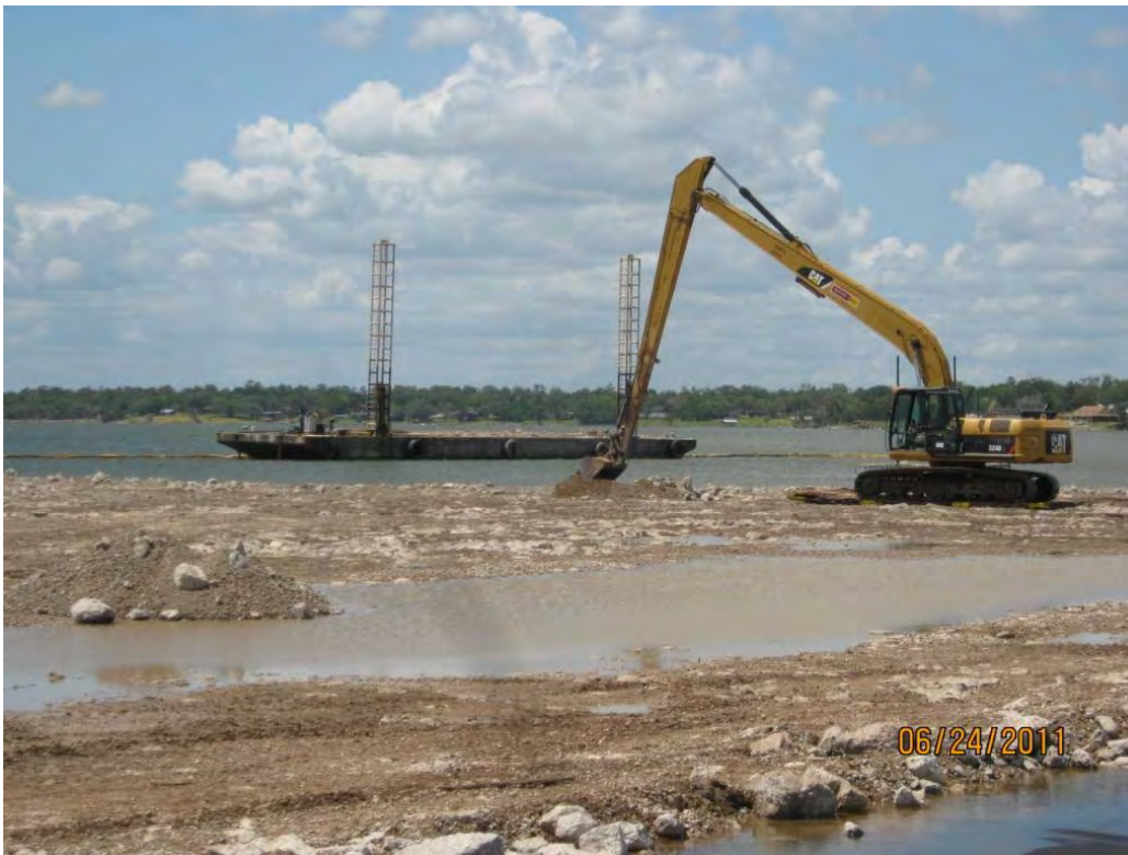
Photo 4 – Long-reach excavator placing Armor Cap B/C in an area identified as less than 1.0 feet by the surveyors.
