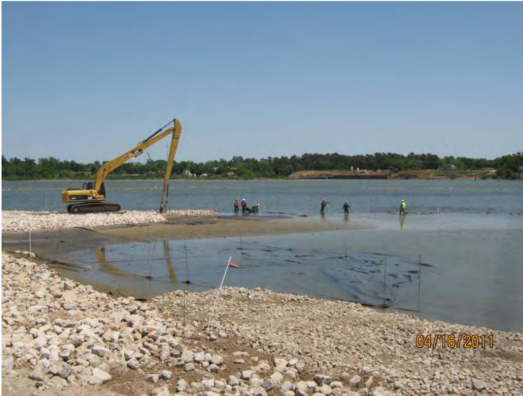
Photo 2 – Deploying a panel of geotextile in the east cell near the north end of the central berm.
