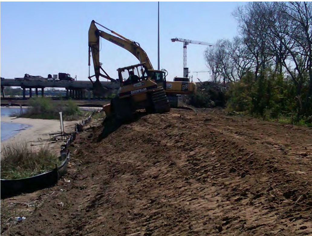
Photo 8 – Grading the east slope of the central berm to establish a stable slope for future rock placement
