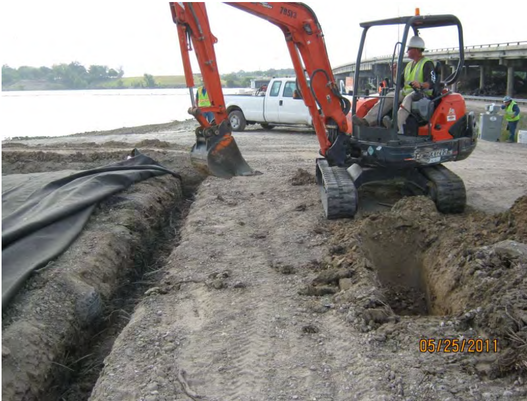
Photo 3 – Relocating a 40-foot section of anchor trench on the south berm due to suspected paper mill sludge observed in a 40-foot section of the original trench.
