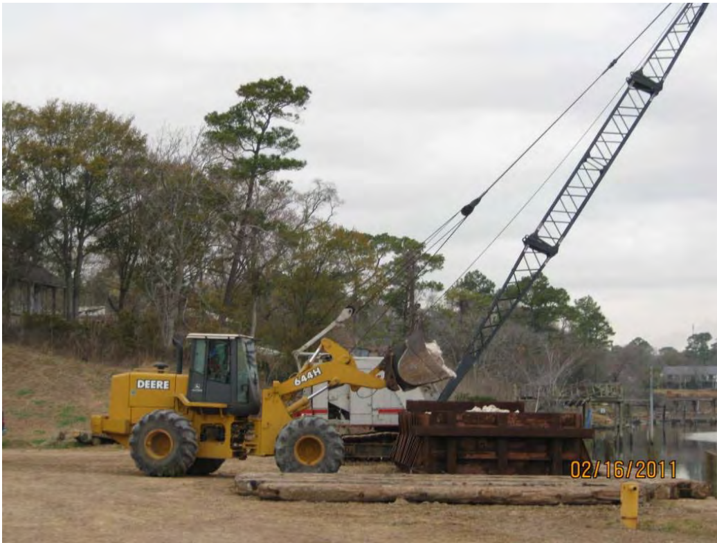
Photo 1 – Loading Armor Cap D rock into steel box at LaBarge dock area for future loading onto transport barge
