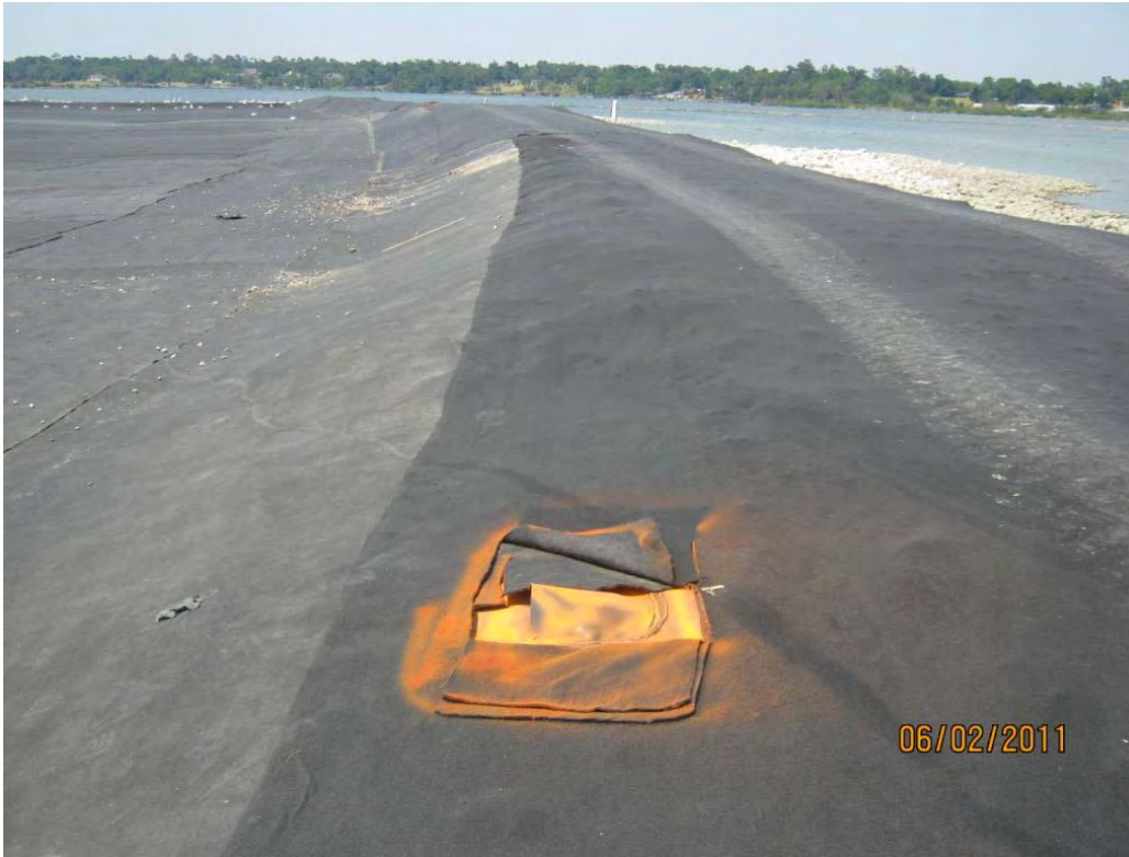
Photo 3 – One of two vents installed on the inside slope of the central berm.
