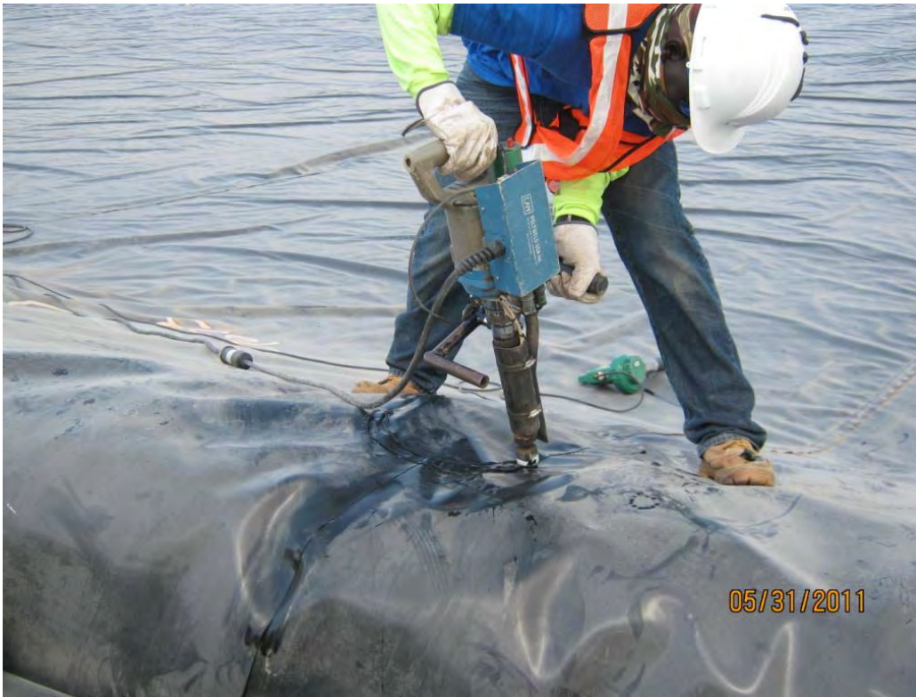
Photo 4 – Patching a location where a double-seam pressure test had been performed on the LLDPE liner.
