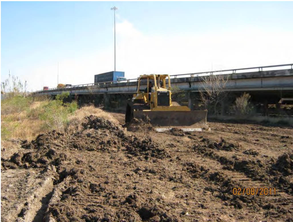
Photo 5 – Grading TxDOT ROW along future haul road
