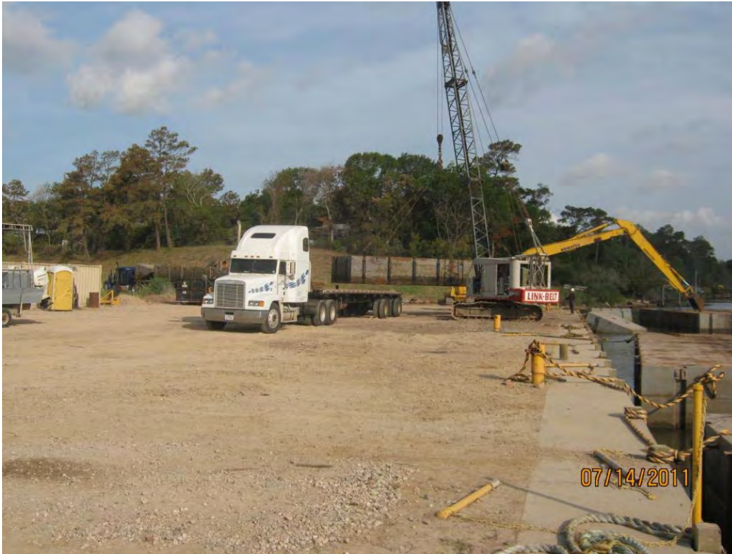
Photo 3 – Loading a section of the aggregate transport barge onto a flatbed truck for removal from the project.
