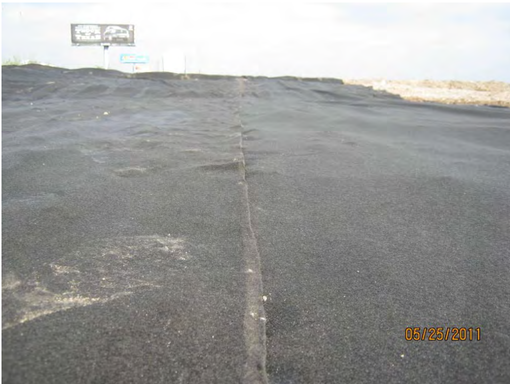
Photo 6 – Laster seam connecting adjacent panels of geotextile.
