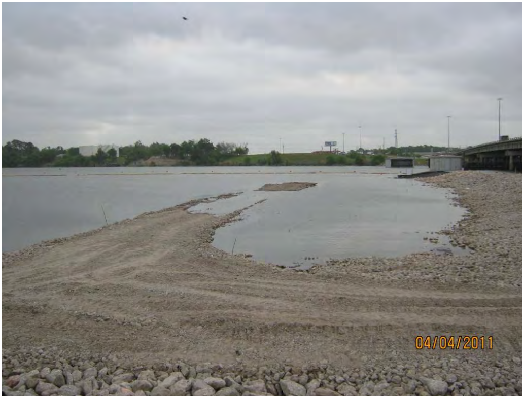
Photo 1 – Rock platform in the east cell partially submerged during a high tide resulting from south winds.
