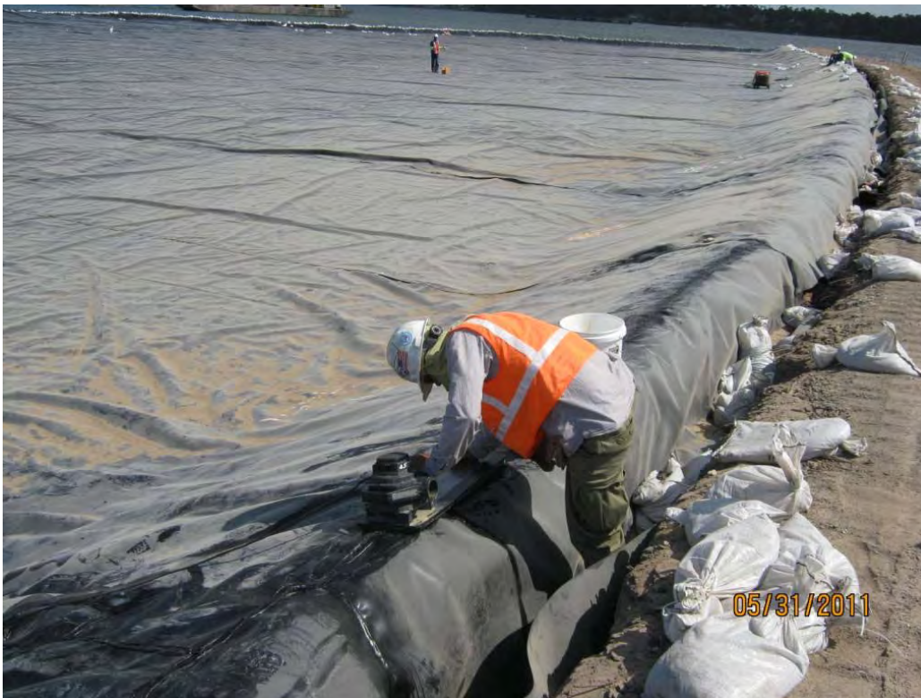
Photo 5 – Vacuum testing a patch on the LLDPE liner.
