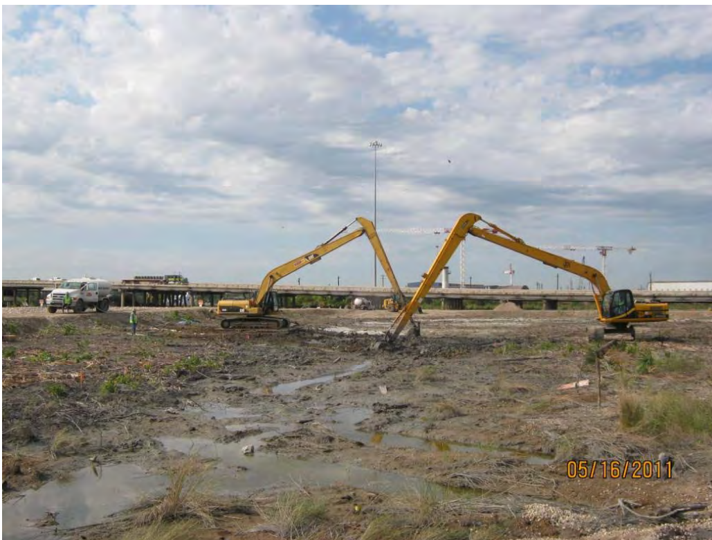
Photo 2 – Mixing Portland cement into a low-lying area in the east portion of the Western Cell.
