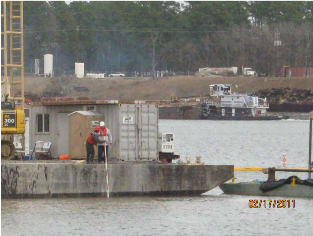
Photo 5 – Probing thickness of Armor Cap D placement in east cell at SJRWP
