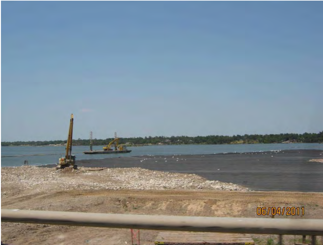
Photo 3 – Overview of Armor Cap B/C rock placement in the Western Cell.
