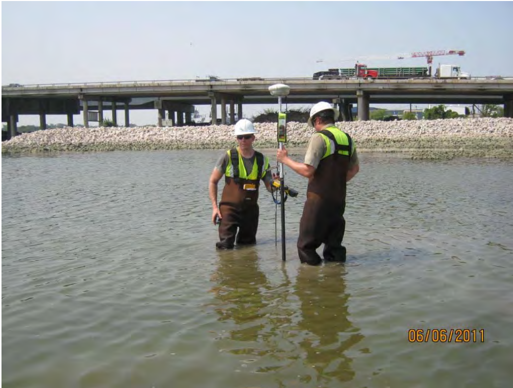
Photo 4 – Probing the thickness of rock placed at a select location in the Eastern Cell.
