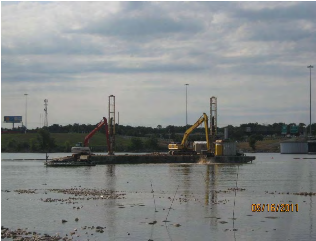
Photo 5 – Placing Armor Cap D rock in the Eastern Cell.
