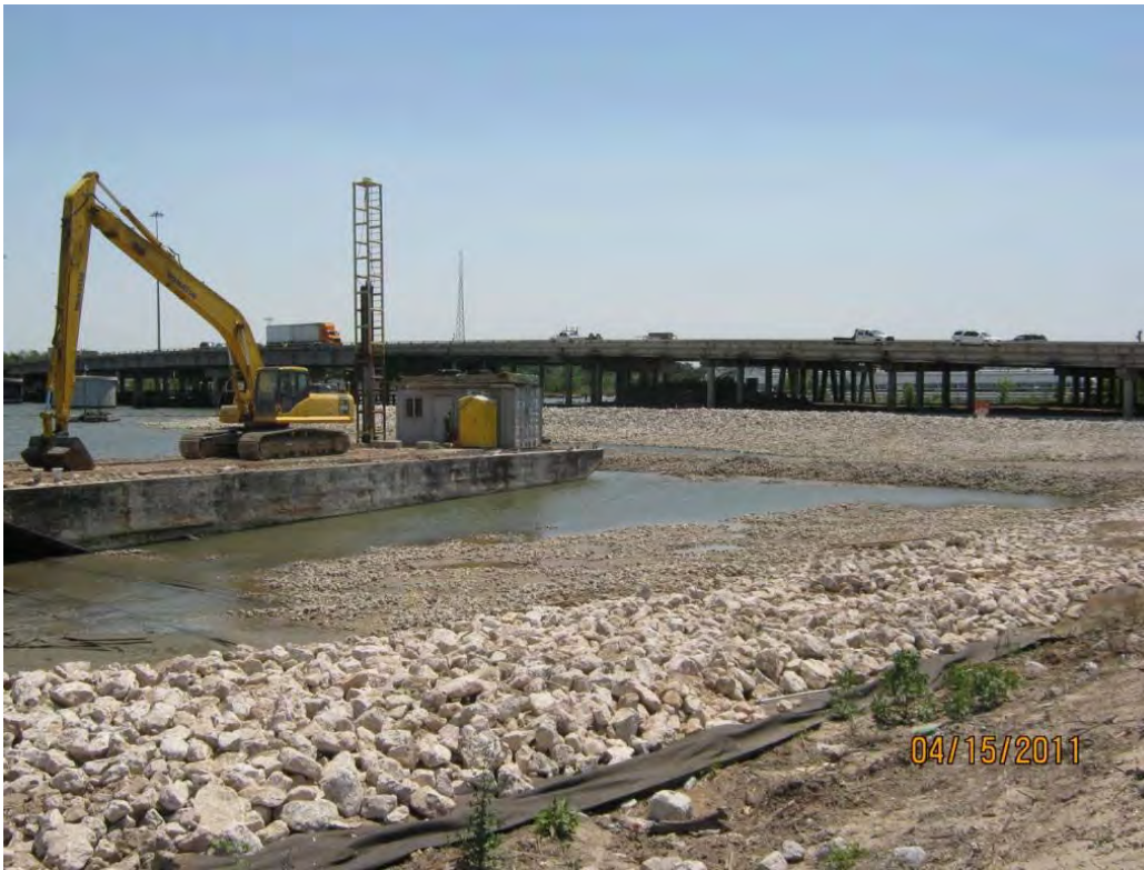
Photo 1 – Armor Cap A rock placed on April 13 and 14, 2011, visible in the east cell at low tide.
