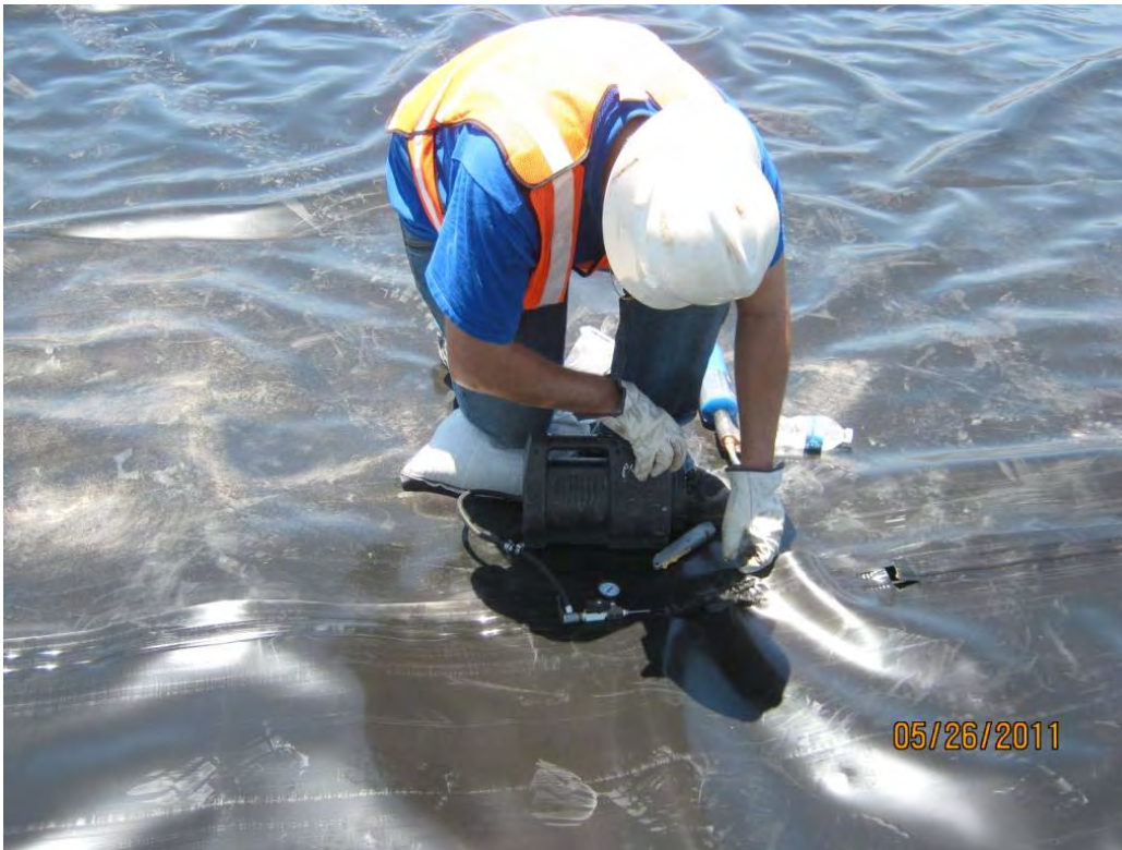
Photo 5 – Pressure-testing a double seam to verify the integrity of the seam.
