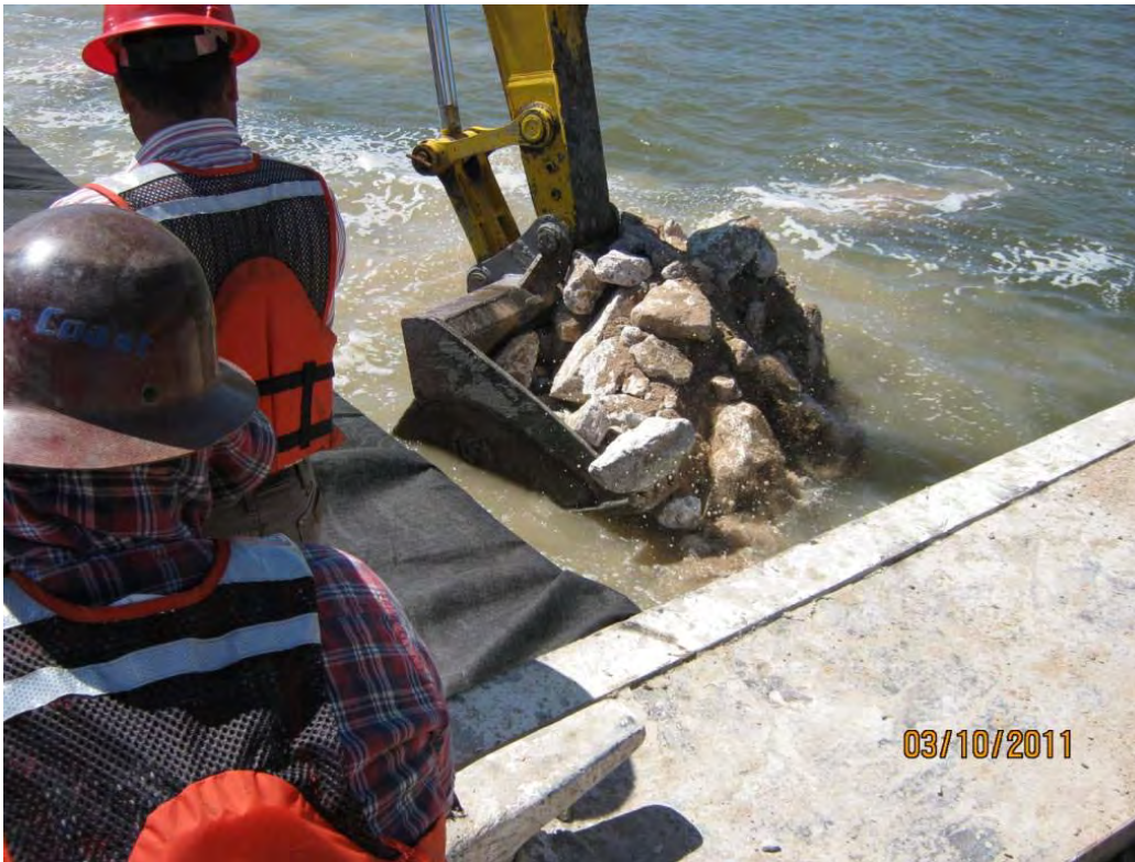
Photo 5 – Deploying geotextile and placing Armor Cap D rock in the east cell
