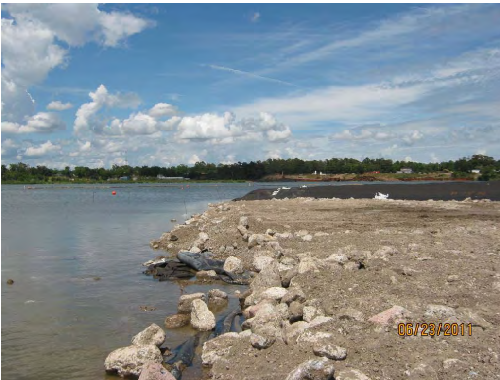
Photo 5 – Armor Cap B/C rock placed at the north end of the Western Cell (not 100% complete at time of photo).
