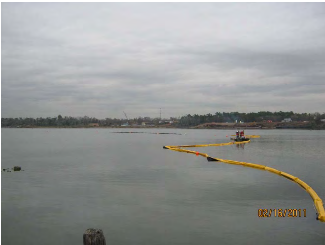
Photo 4 – Shirley & Sons deploying turbidity curtain around perimeter of east cell at SJRWP
