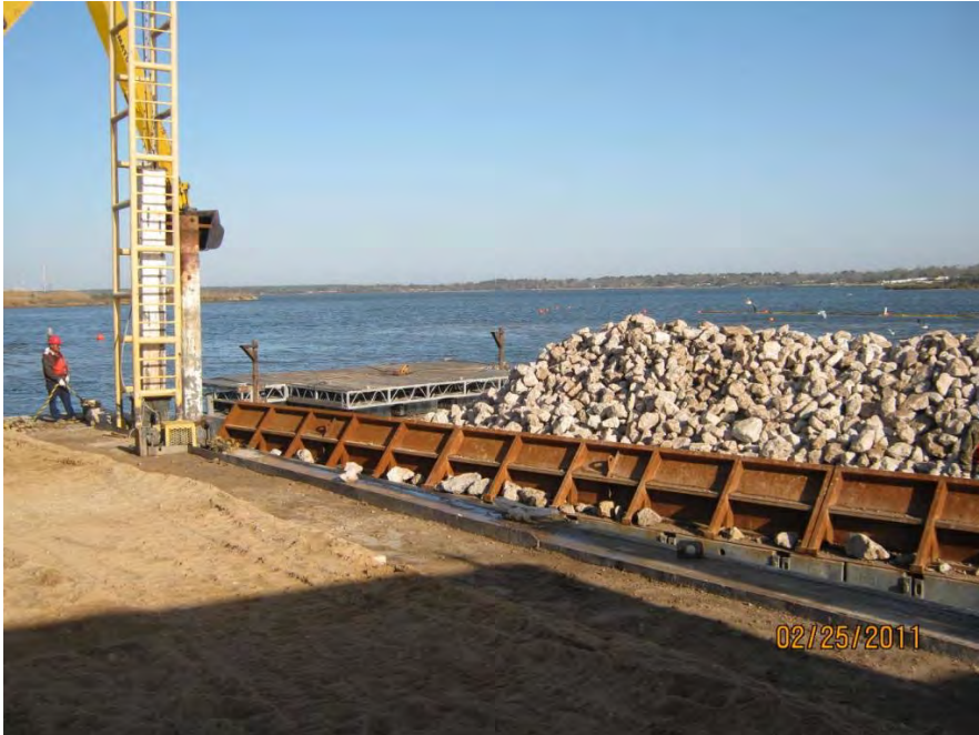
Photo 1 – Aggregate transport barge maneuvered into position adjacent to barge-mounted excavator
