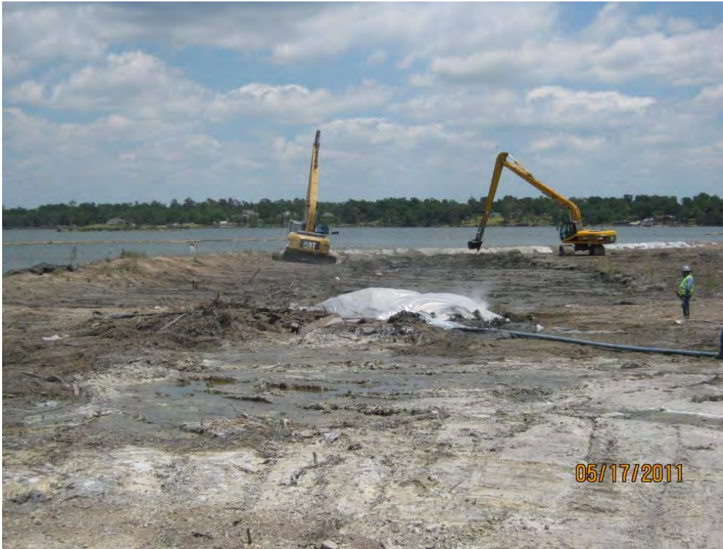
Photo 3 – Receiving Portland cement in the Western Cell (foreground) and mixing Portland cement into a low-lying area in the Western Cell (background).
