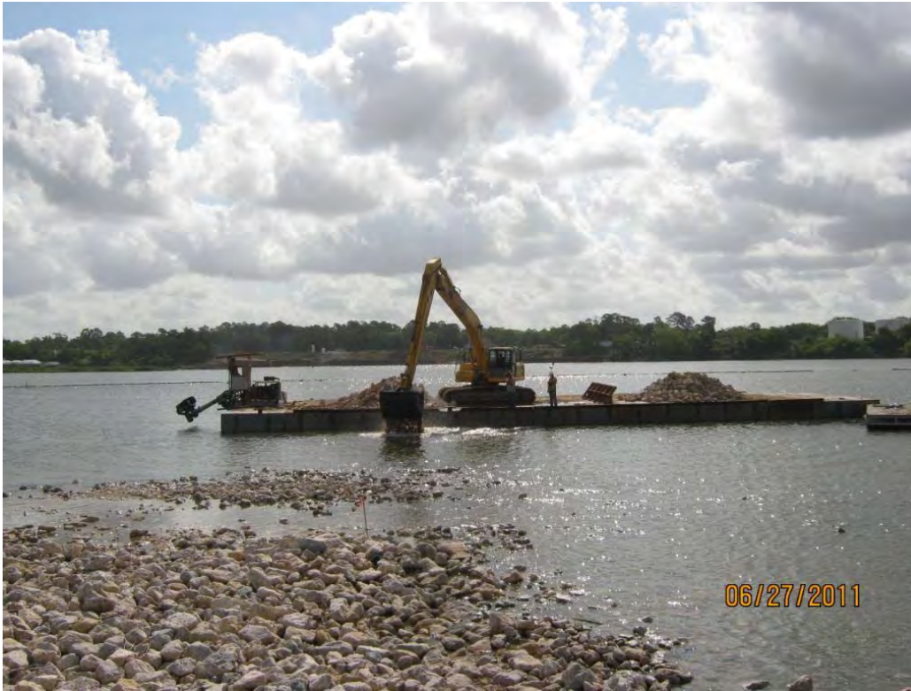
Photo 3 – Barge-mounted excavator placing Armor Cap D rock in the Eastern Cell at a location identified by the surveyor.
