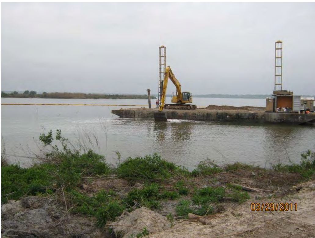
Photo 3 – Water-based operations placing Armor Cap A rock in the northwestern area.
