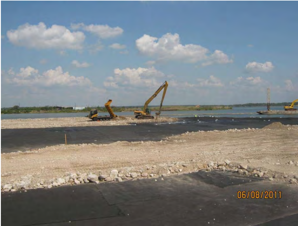
Photo 1 – Placing Armor Cap B/C rock near the west berm in the Western Cell; the uncovered geotextile in the foreground of the photo is an area scheduled to receive Armor Cap D rock.
