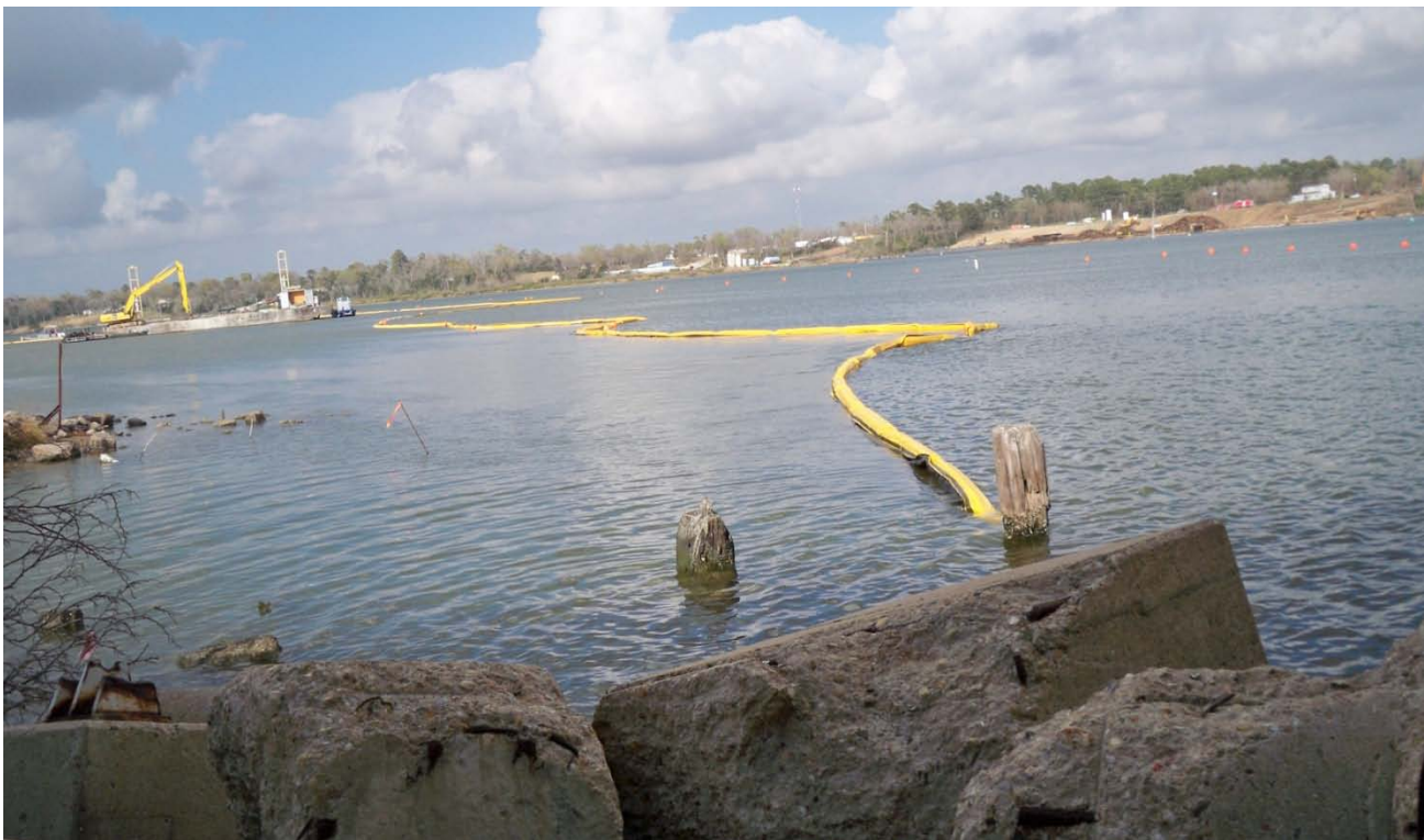
Photo 2 – Repositioning boom; increasing tidal velocity and winds from the south
