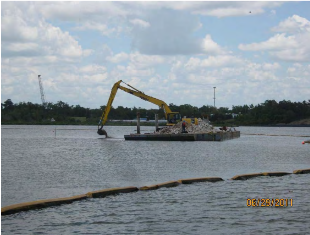
Photo 1 – Barge-mounted excavator placing Armor Cap D rock in the Eastern Cell.
