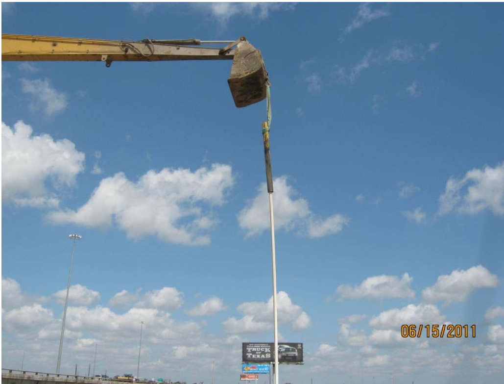
Photo 3 – Removing the stick-up pipe and monitoring well from the subsurface after grout addition.
