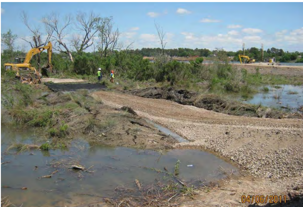
Photo 2 – Access road constructed into the center portion of the west cell for clearing of vegetation.
