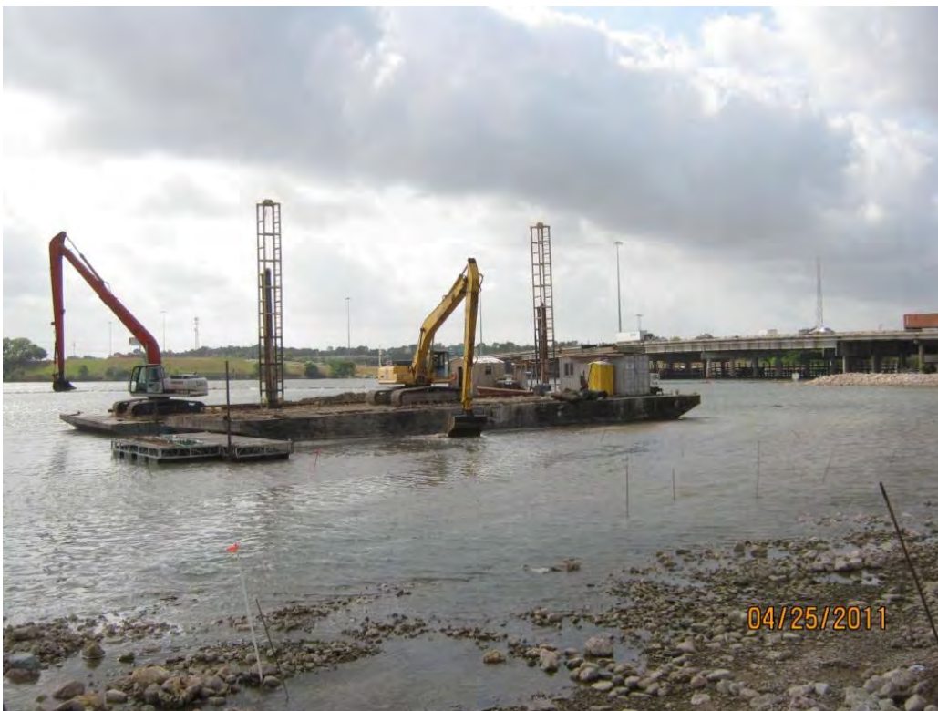
Photo 4 – Placing Armor Cap A rock in the cell.
