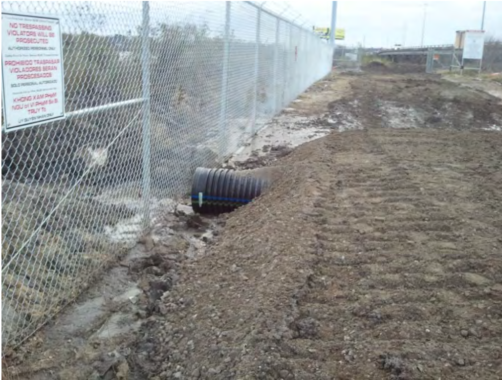
Photo 1 – Culvert installation in the TxDOT ROW to improve drainage west of main access gate
