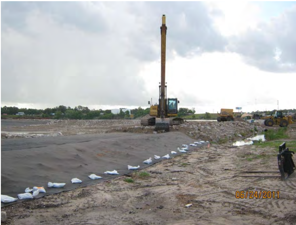
Photo 1 – Long-reach excavator placing Armor Cap B/C rock atop the south berm of the Western Cell.
