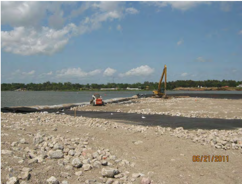
Photo 2 – Skidsteer and long-reach excavator placing Armor Cap B/C rock near the north end of the Western Cell.
