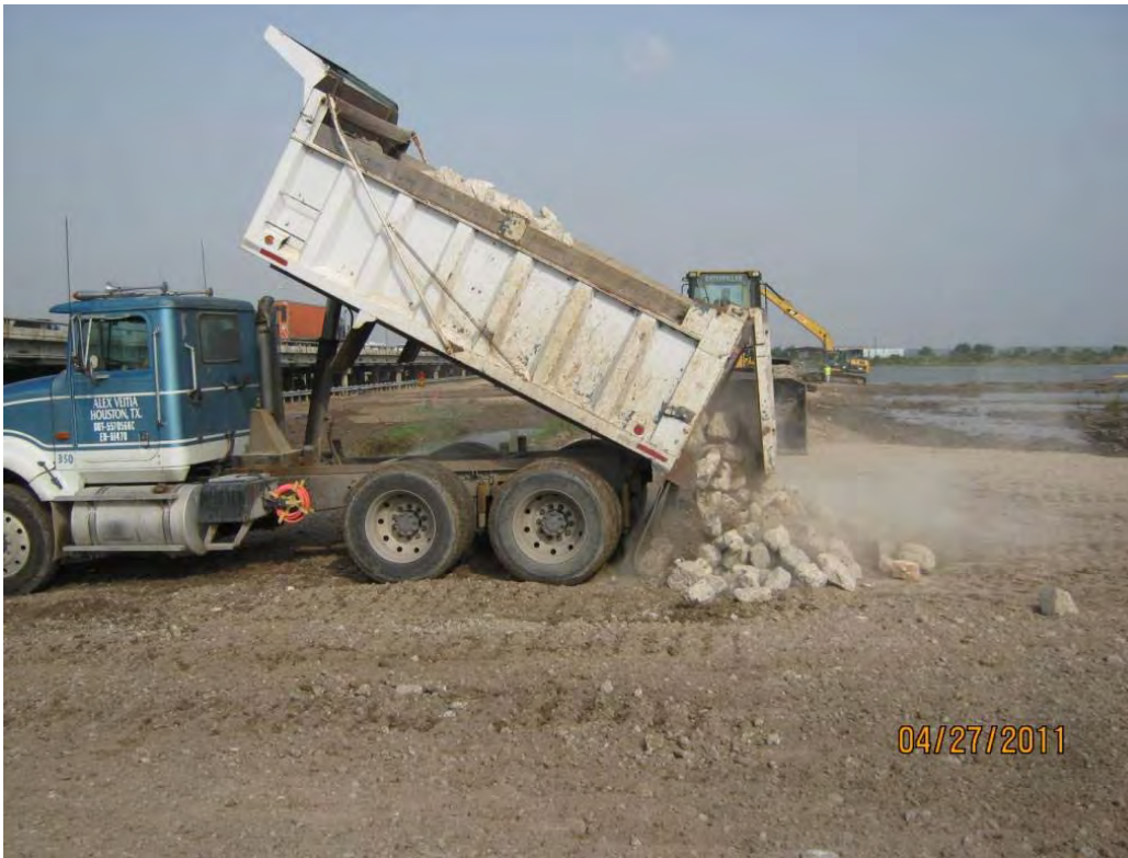
Photo 1 – Receiving Armor Cap B/C rock for placing outside the southwest corner of the west cell.
