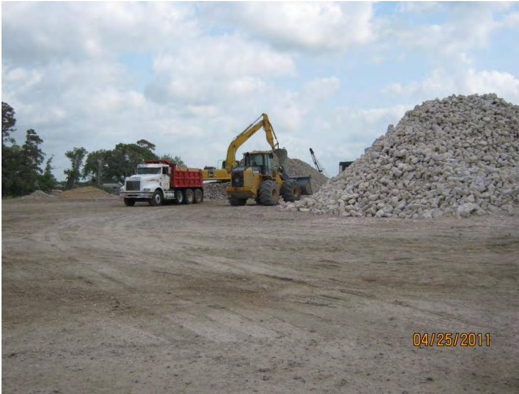
Photo 3 – Receiving and stockpiling Armor Cap A rock at the La Barge Property; Armor Cap D stockpile at right.
