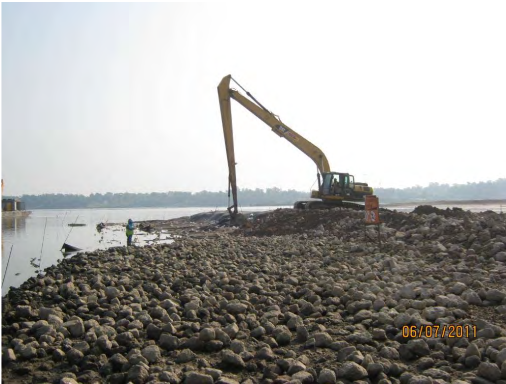
Photo 1 – Placing Armor Cap B/C rock across the western berm in the Western Cell.
