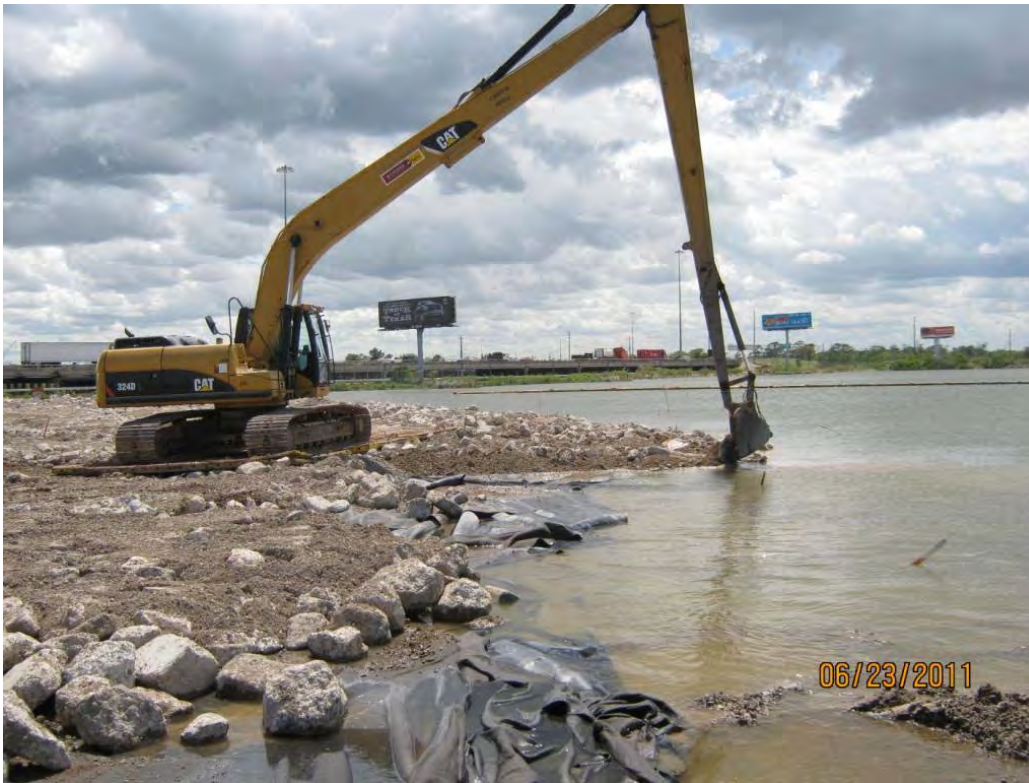
Photo 4 – Long-reach excavator placing Armor Cap B/C at the north end of the Western Cell.
