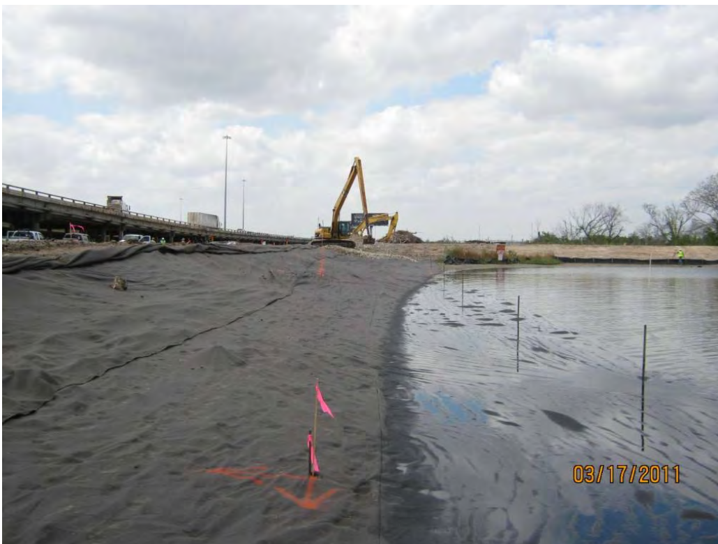
Photo 6 – Geotextile placed on the south berm with stakes marking future overlap area and areas with differing cap types.
