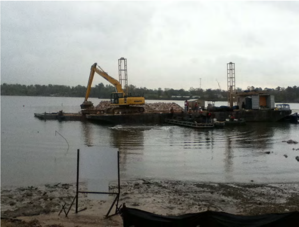
Photo 1 – Beginning to place first barge load of Armor Cap D rock for the day.
