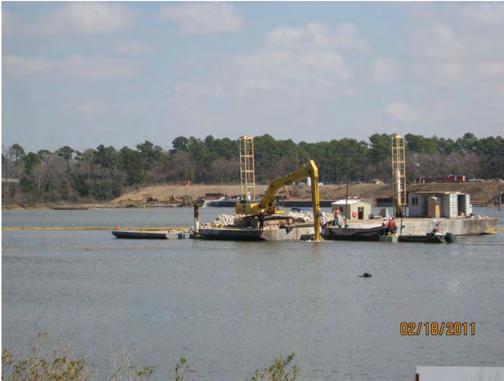
Photo 2 – Placing Armor Cap D rock in east cell and deploying geotextile ahead of the rock placement
