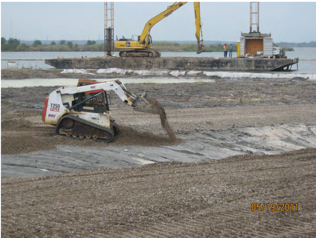
Photo 4 – Spreading crushed concrete road base in the Western Cell using a low-ground pressure skid-steer.
