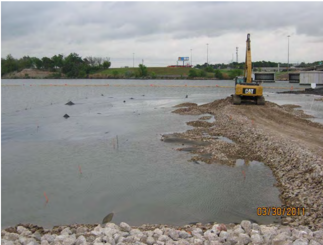
Photo 5 – Rock platform in the east cell and displaced sediment to the north of the rock platform.
