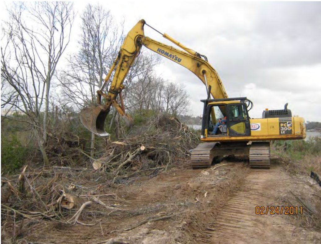
Photo 1 – Staging vegetation cleared from the central berm onto plastic sheeting within west cell
