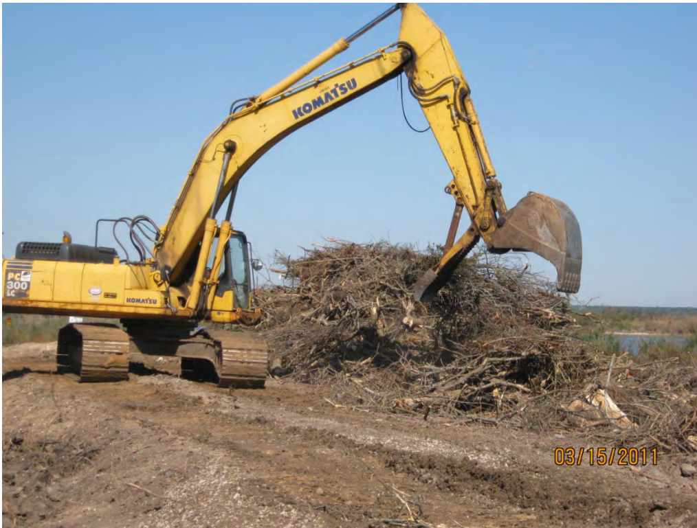
Photo 2 – Processing large, clean woody debris for off-site transportation and disposal.
