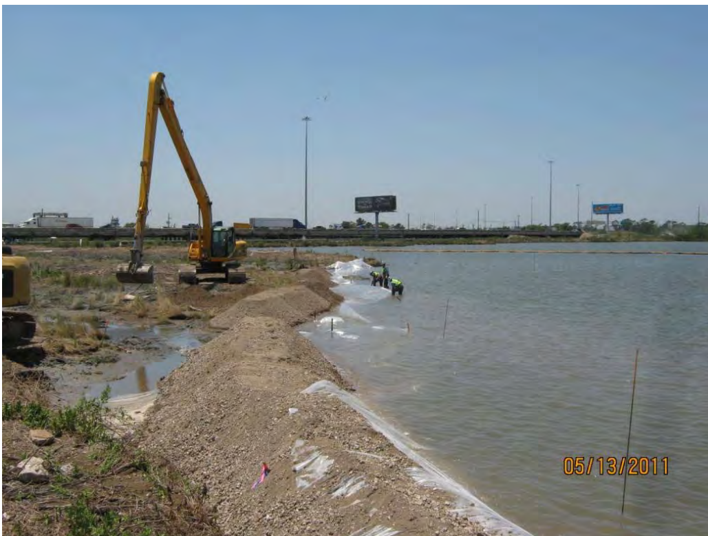
Photo 4 – Construction of the northern berm in the Western Cell.
