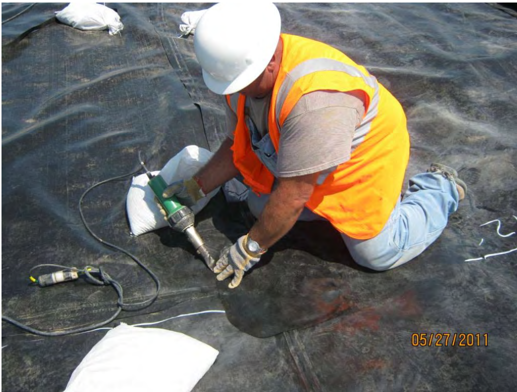
Photo 3 – Welding a patch over a location on the LLDPE liner where a seam test had been performed.
