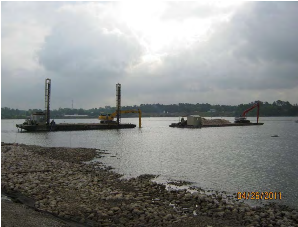
Photo 1 – Repositioning barges to continue placement of Armor Cap C rock in the east cell.
