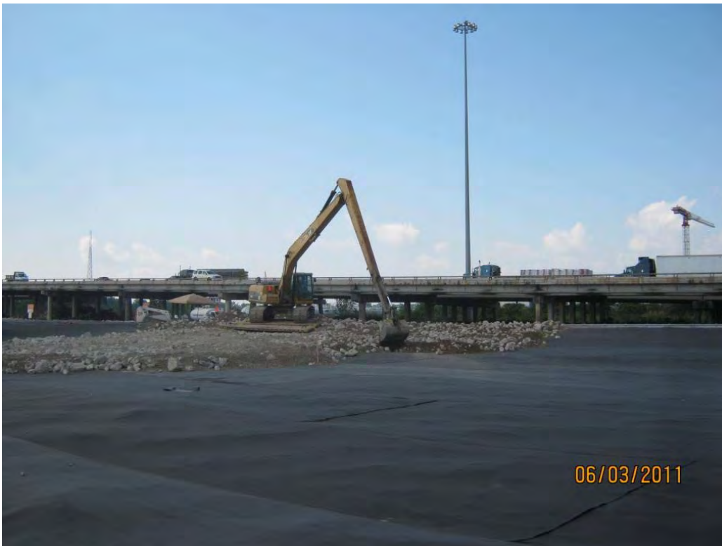
Photo 2 – Placing Armor Cap B/C rock near the southeast corner of the Western Cell.
