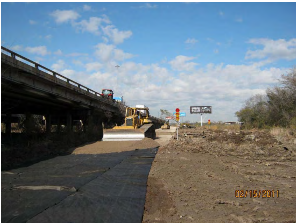
Photo 2 – Receiving and compacting CCRB atop geotextile south of SJRWP along TxDOT ROW
