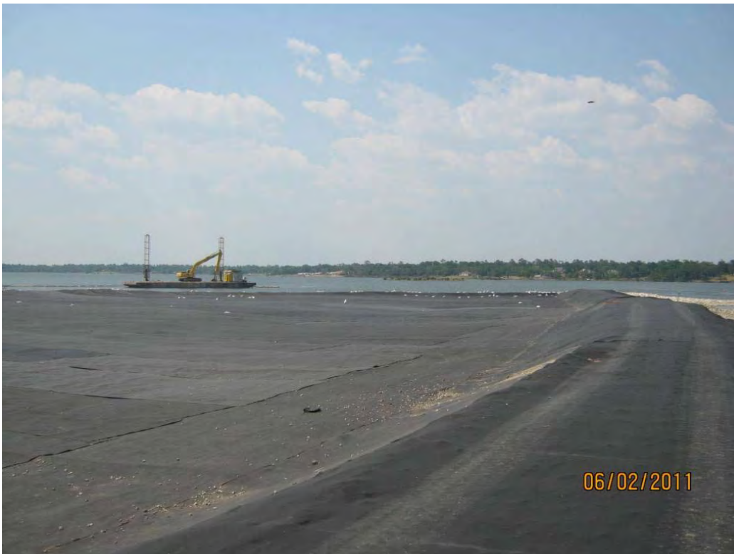
Photo 2 – Western Cell following the installation of all geotextile and geomembrane (LLDPE) materials.
