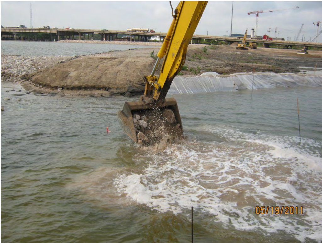
Photo 1 – Water-based spreading of Armor Cap D rock (24 inch thick area) to the north of the central berm.
