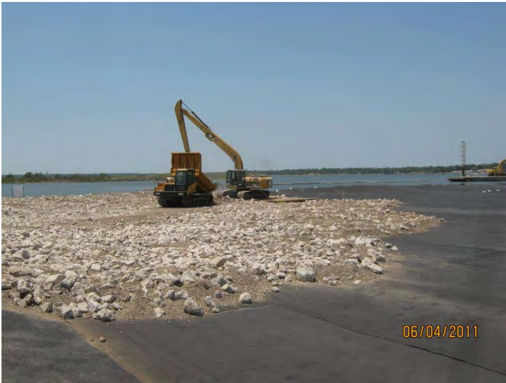
Photo 1 – Morooka truck delivering Armor Cap B/C rock to the Western Cell for placement.
