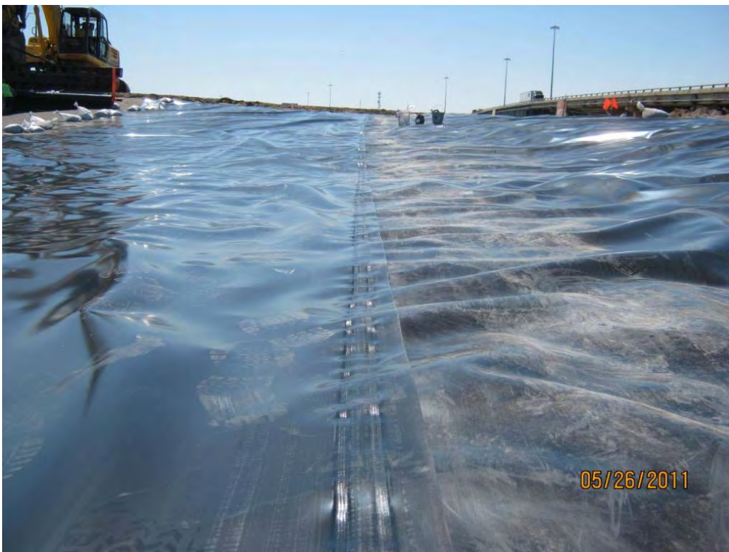
Photo 4 – Double seam used to weld together two overlapping panels of LLDPE.
