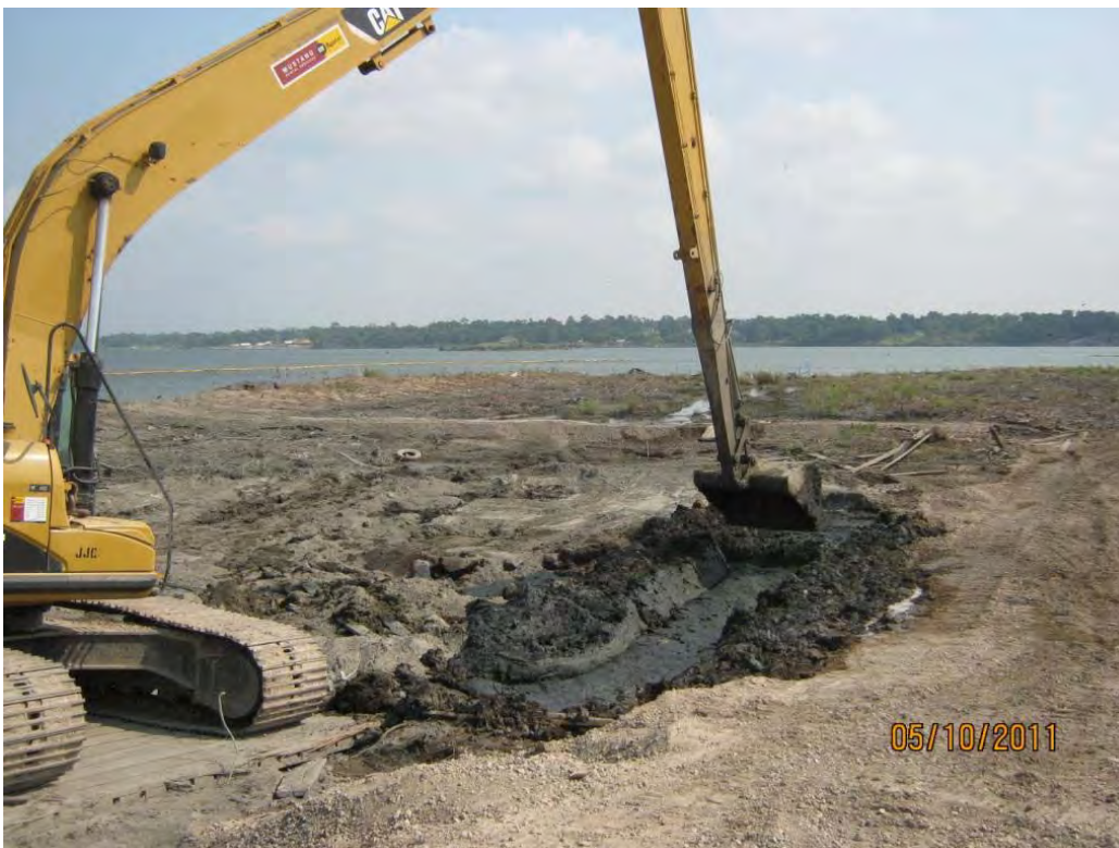
Photo 2 – Mixing Portland cement into the Western Cell to the left of the rock access point.
