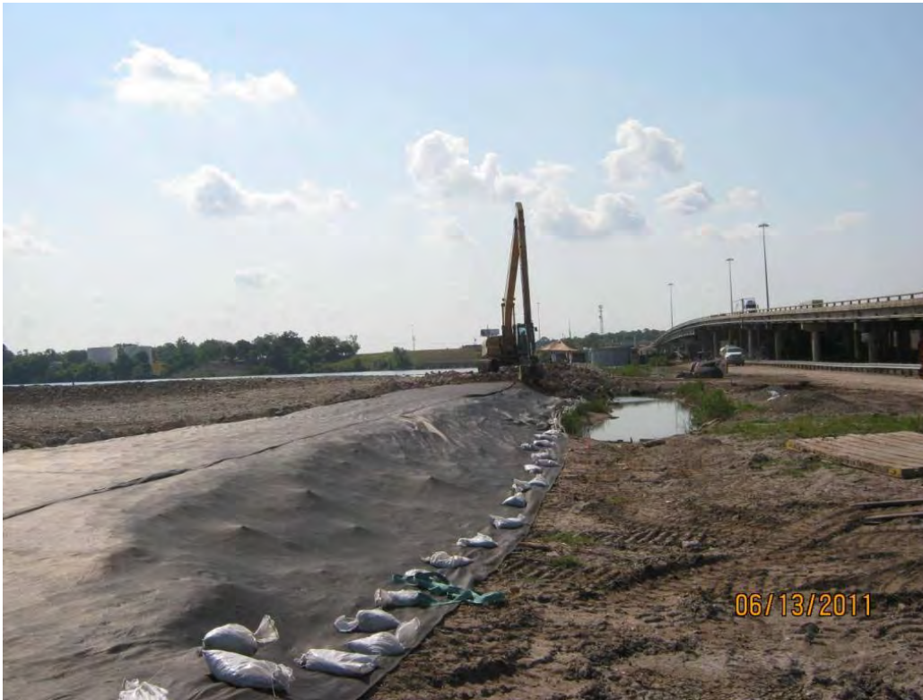
Photo 1 – Placing Armor Cap B/C rock atop the south berm of the Western Cell.
