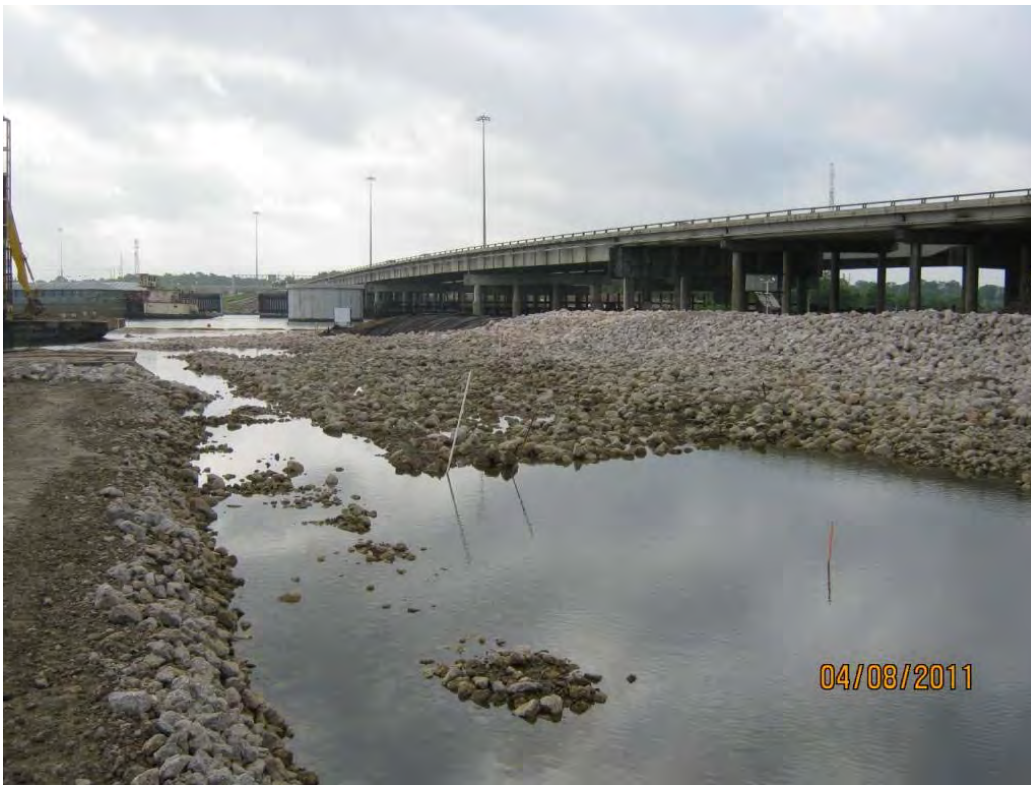
Photo 2 – Armor Cap B/C rock placed in the east cell.
