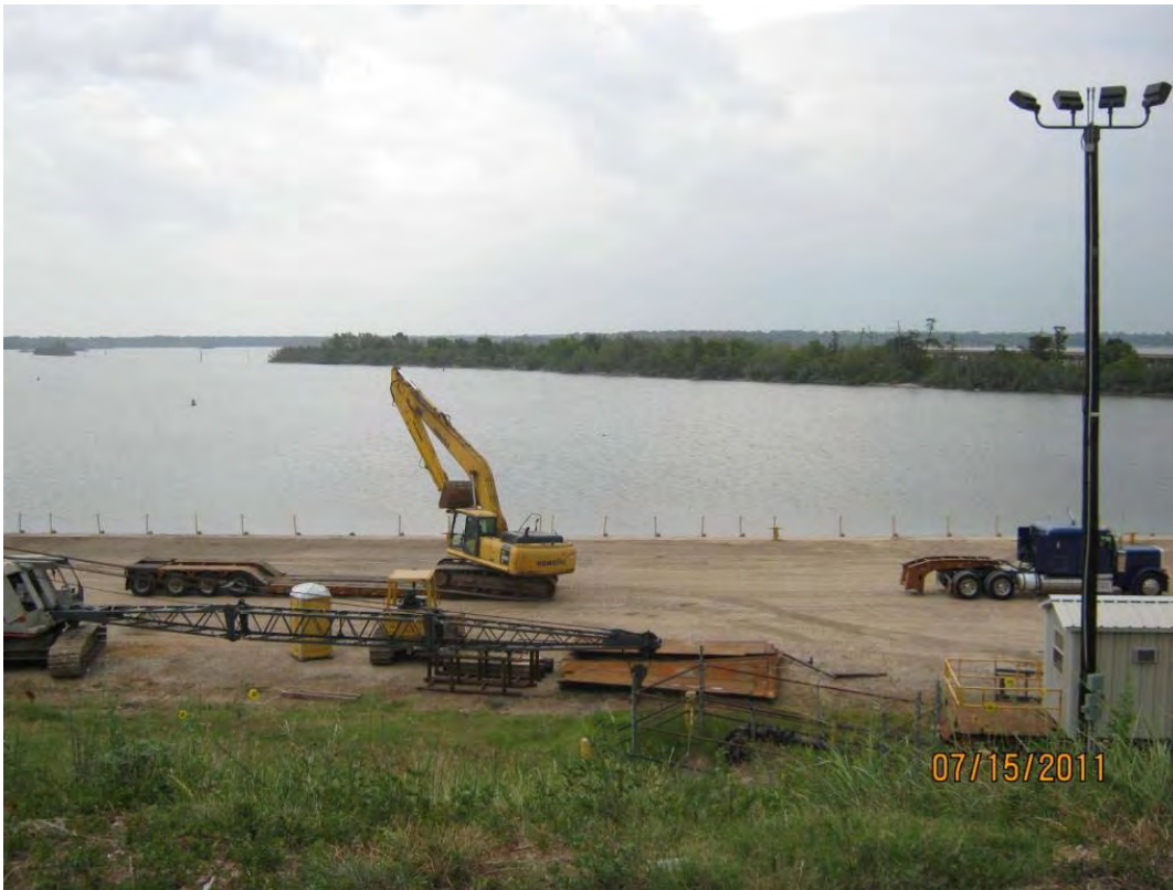
Photo 3 – Loading an excavator onto a lo-boy truck at the LaBarge Property for demobilization.
