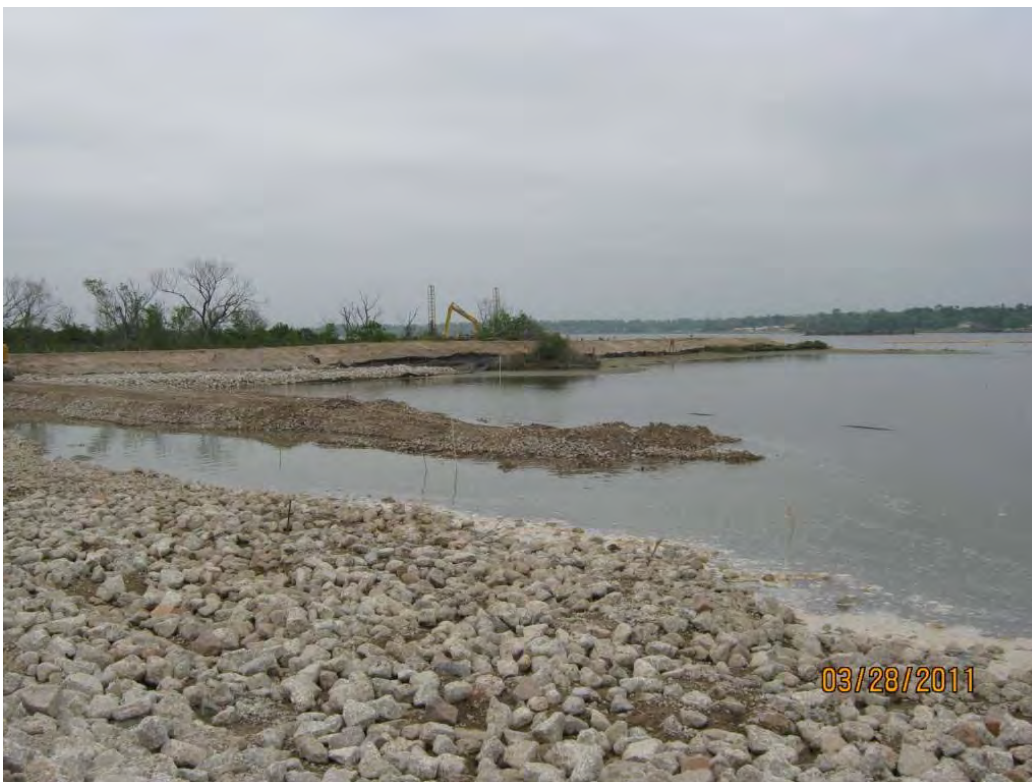
Photo 6 – Leading edge of the rock platform in the east cell following a bearing capacity failure (long-stick excavator is located near the central berm to the left of this photo).
