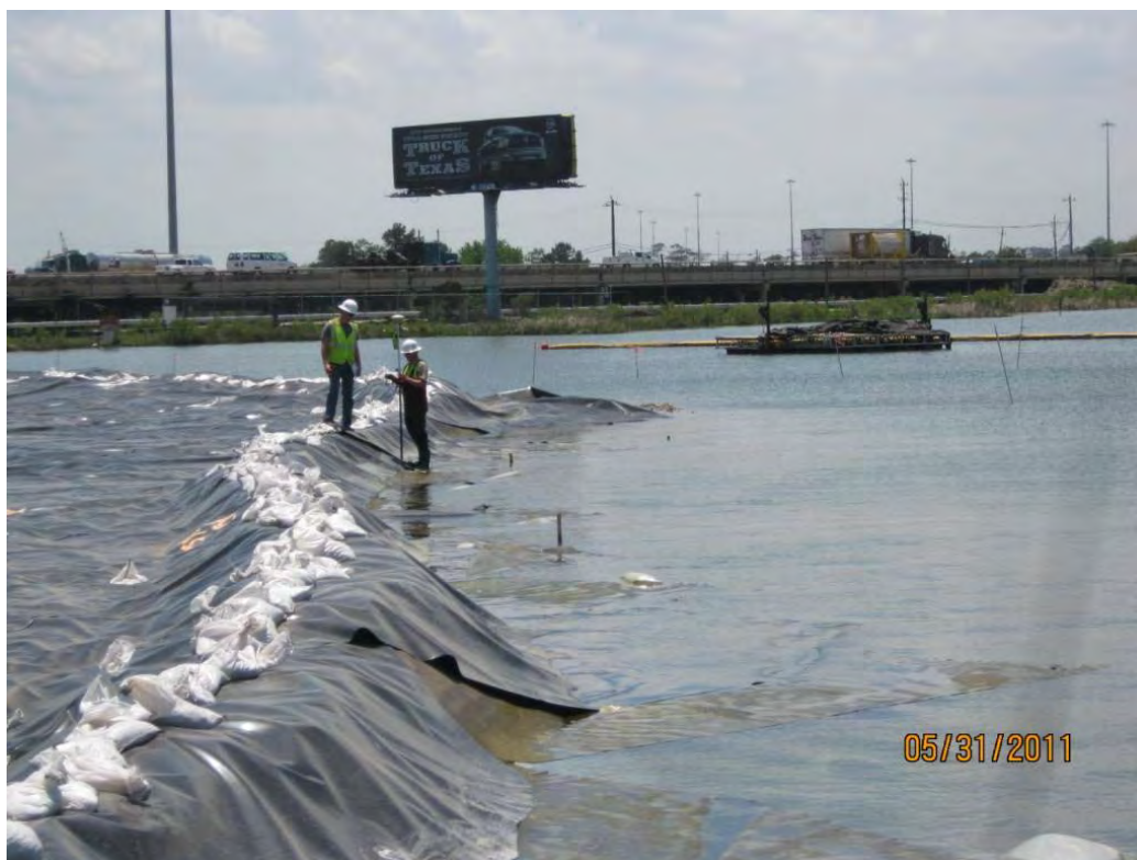
Photo 1 – Collecting as-built survey data for the LLDPE liner installed in the Western Cell.
