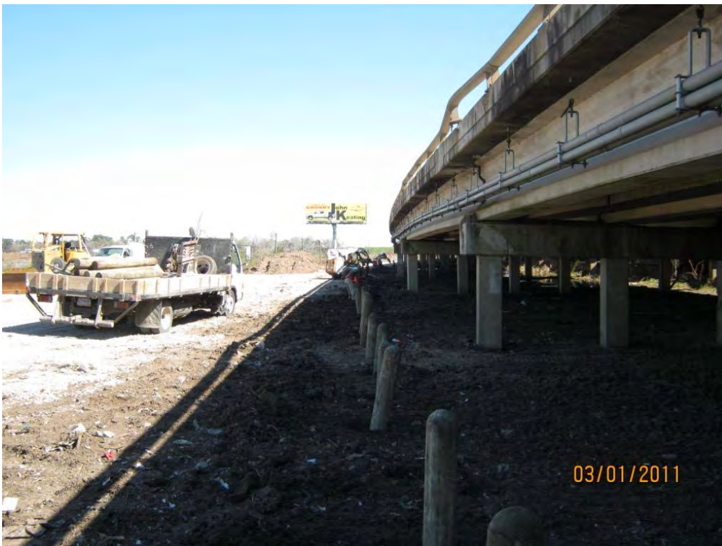
Photo 4 – Excavating post holes for the guard rail posts adjacent to the I-10 Bridge
