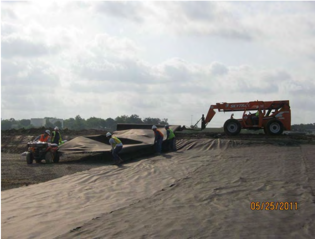
Photo 1 – Deploying geotextile in the Western Cell.
