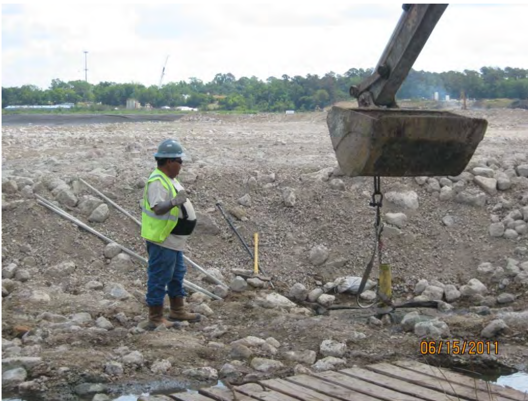
Photo 2 – Preparing to remove the stick-up pipe around a monitoring well.
