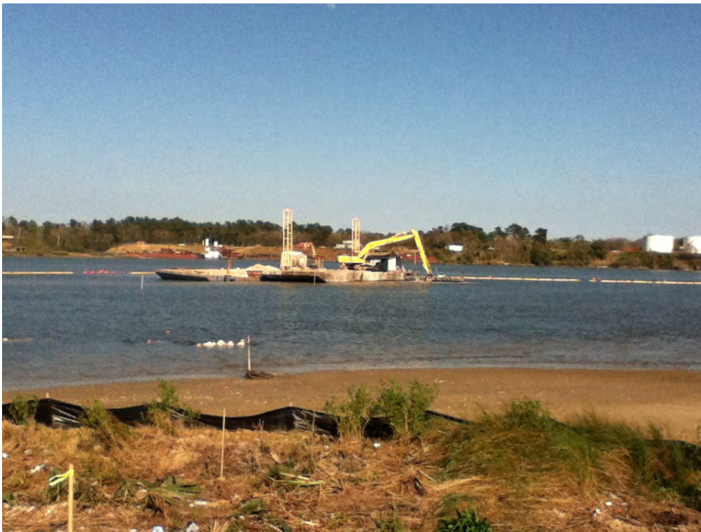
Photo 3 – Placing second barge load of the day of Armor Cap D rock in the east cell.
