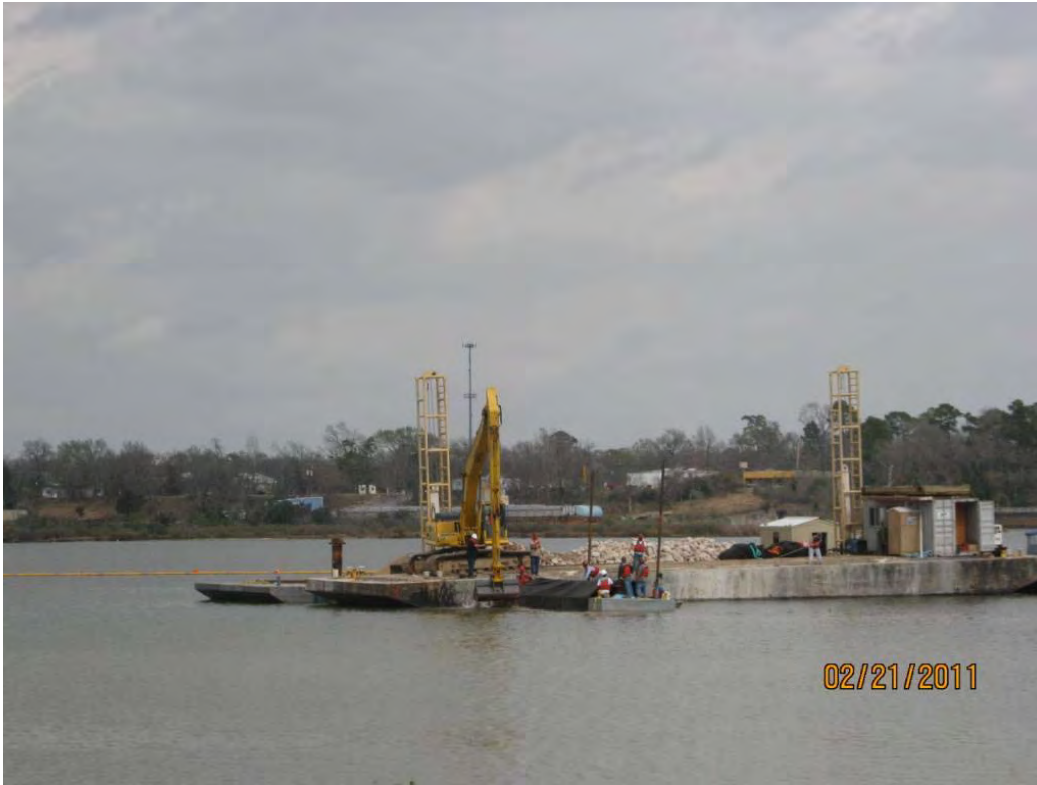
Photo 1 – Placing Armor Cap D rock in east cell and deploying geotextile ahead of the rock placement
