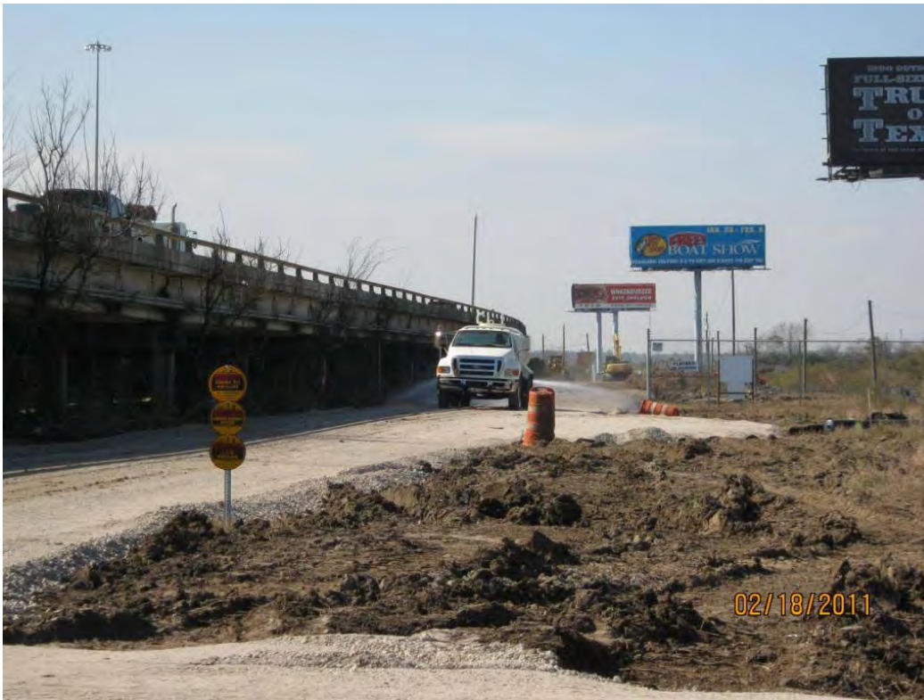
Photo 4 – Spraying water on TxDOT ROW haul road for dust control
