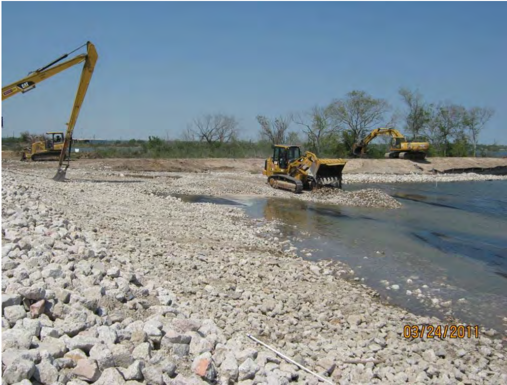
Photo 1 – Constructing a rock platform in the east cell to be used for armored cap placement.
