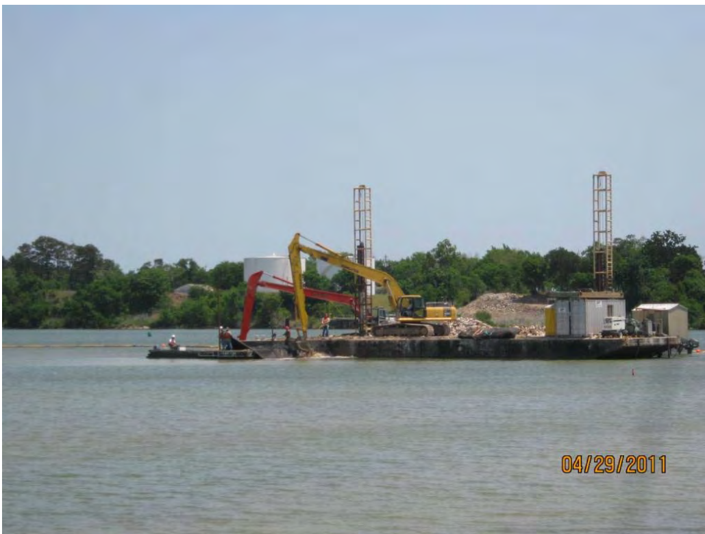
Photo 2 – Placing geotextile and Armor Cap D rock in the east cell.
