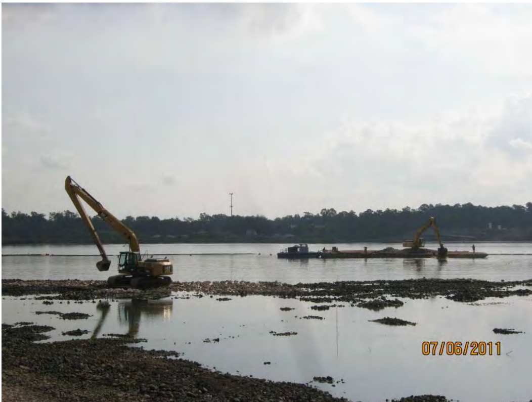
Photo 2 – Placing Armor Cap D rock in the Eastern Cell via barge-based and land-based equipment.
