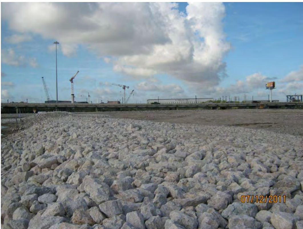
Photo 2 –Armor Cap D rock atop the central berm in the Western Cell following the completion of rock placement.
