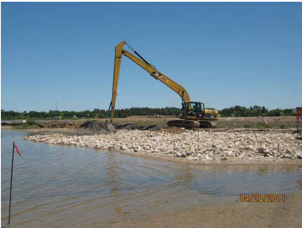
Photo 7 – Placing Armor Cap B/C rock to the west of the west cell.
