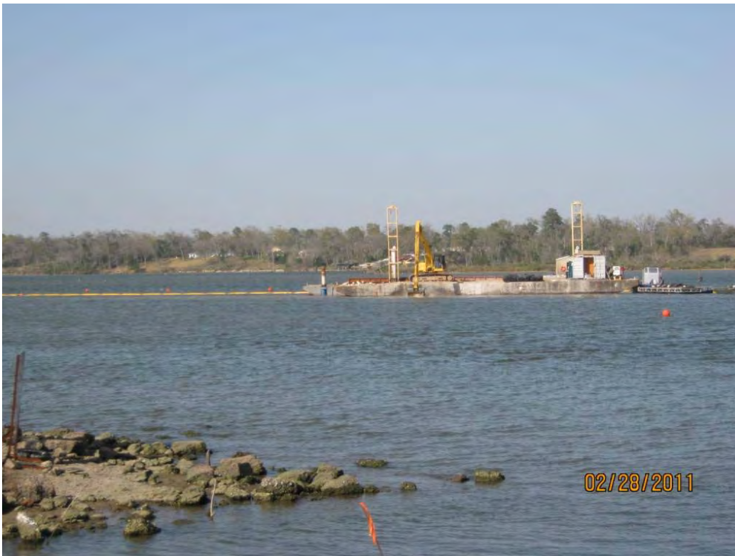
Photo 5 – Placing Armor Cap D rock in east cell after the breach in turbidity curtain was closed
