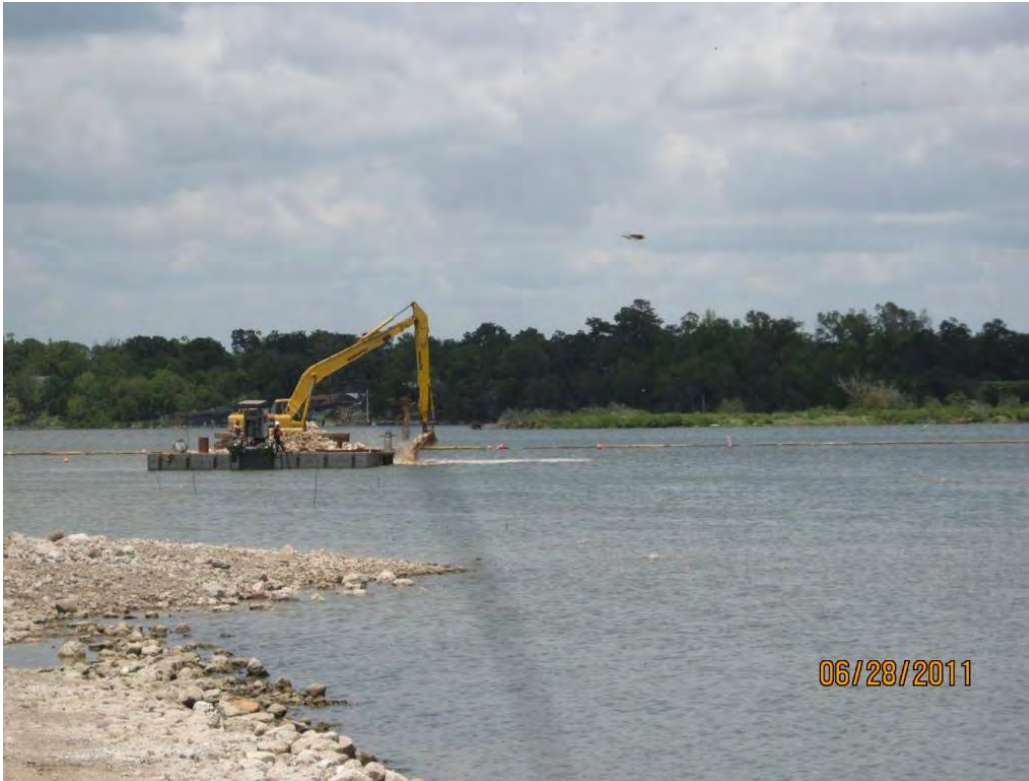
Photo 3 – Barge-mounted excavator placing Armor Cap D rock in the Eastern Cell.
