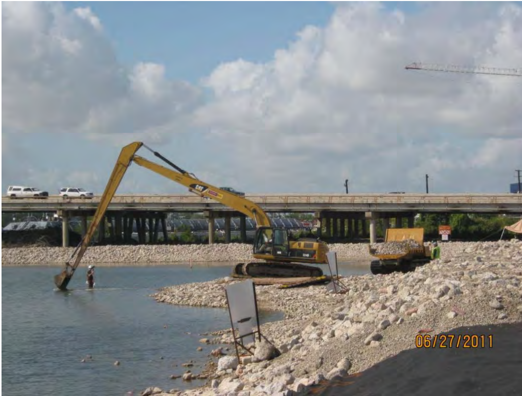
Photo 1 – Long-reach excavator placing Armor Cap A rock in the Eastern Cell at a location identified by the surveyor.
