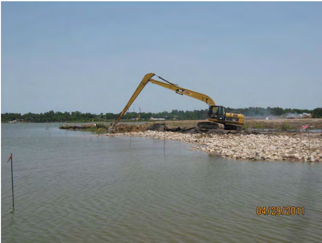
Photo 4 – Placing Armor Cap B/C rock outside the west end of the west cell.
