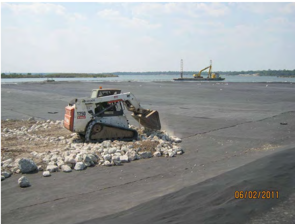
Photo 8 – Skidsteer placing Armor Cap B/C rock in the southeast portion of the Western Cell.
