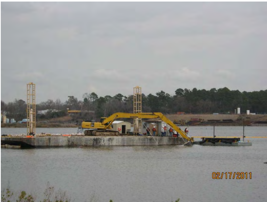
Photo 4 – Placing Armor Cap D rock in east cell at SJRWP
