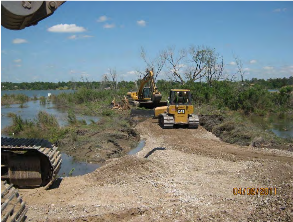
Photo 3 – Access road constructed into center portion of the west cell for clearing of vegetation.
