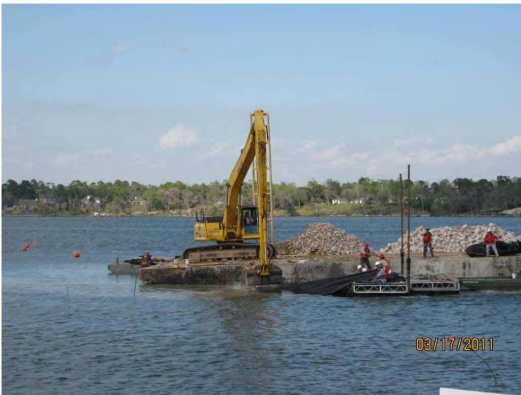
Photo 4 – Deploying geotextile and placing Armor Cap C rock in the east cell.
