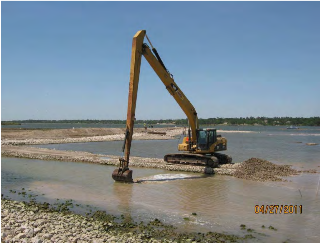
Photo 3 – Placing Armor Cap A rock for in the east cell by removing the rock finger access road.
