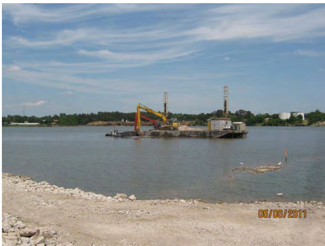
Photo 1 – Placing geotextile and Armor Cap C rock in the Eastern Cell.
