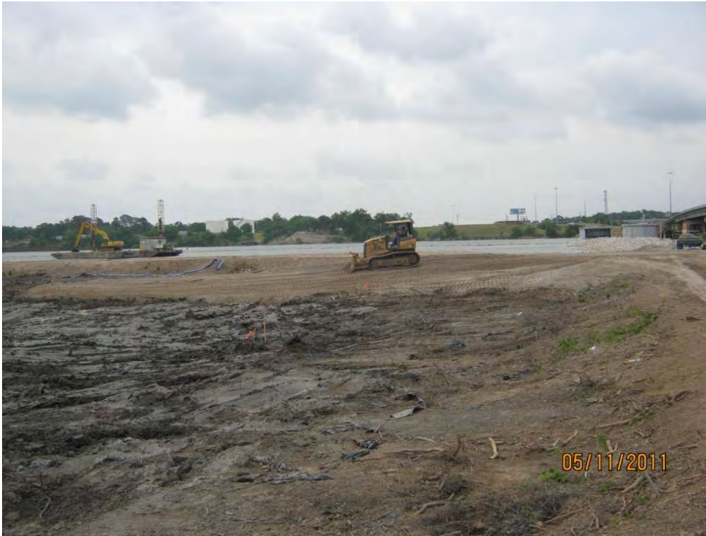
Photo 3 – Using CCRB to create a smoothly-graded surface in the southeast portion of the Western Cell.
