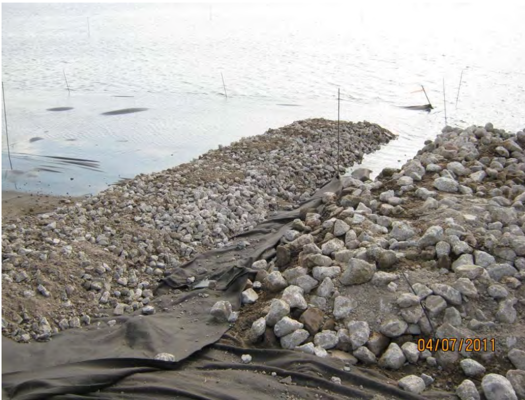
Photo 2 – Armor Cap A rock (at left) and Armor Cap B/C rock (at right) placed to the east of the central berm.
