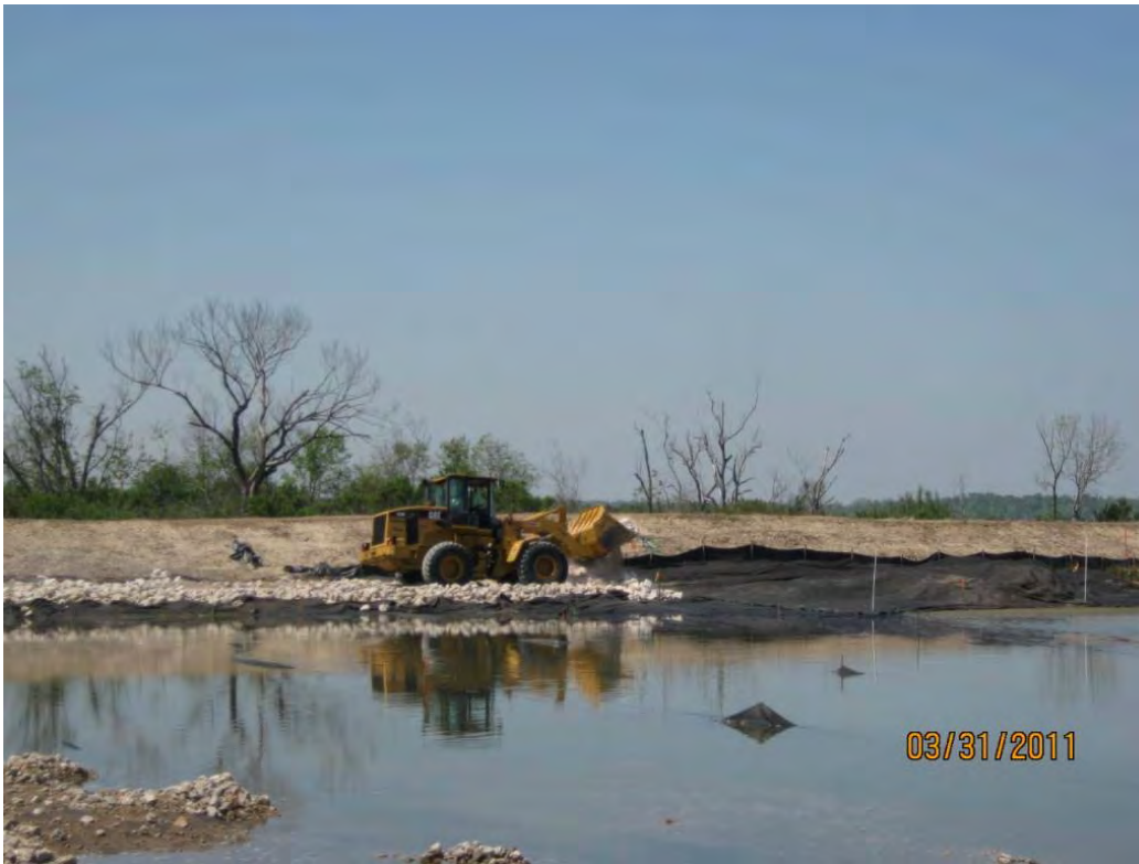
Photo 5 – Placing Armor Cap D rock on the east side of the central berm.
