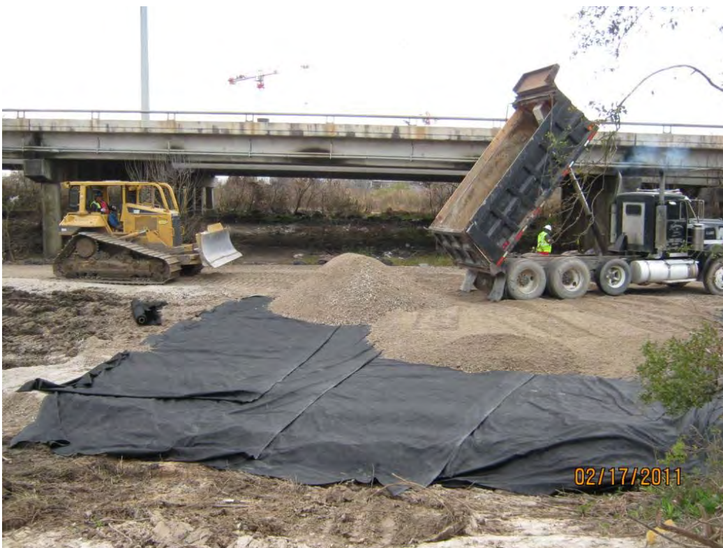
Photo 8 – Haul road construction at TxDOT ROW from main haul road to the central berm at SJRWP
