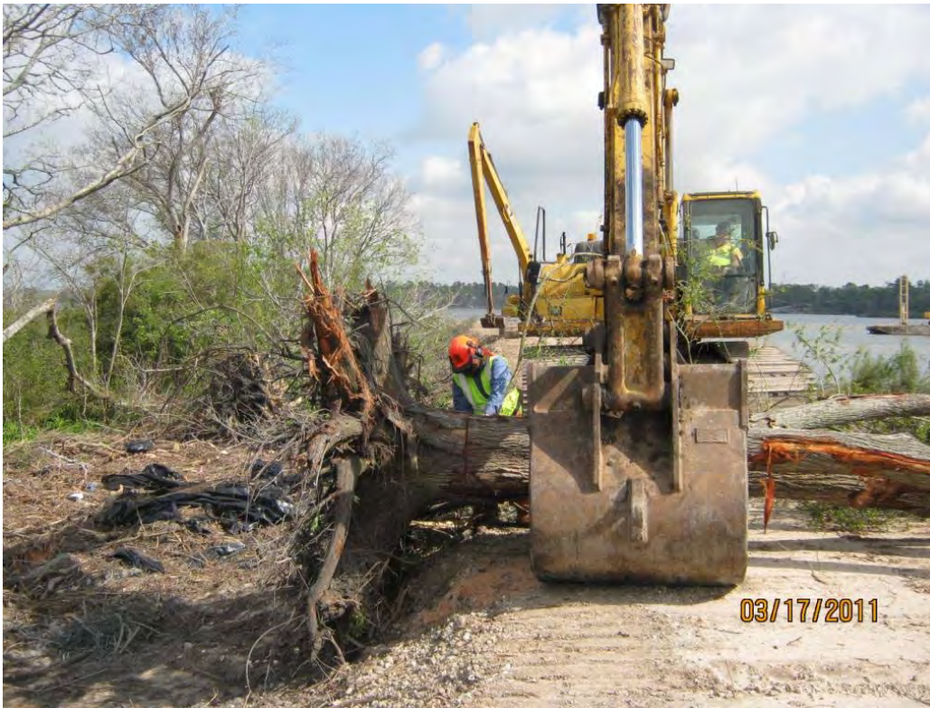
Photo 3 – Using a chainsaw to remove the root mass from a tree cleared from the west cell.
