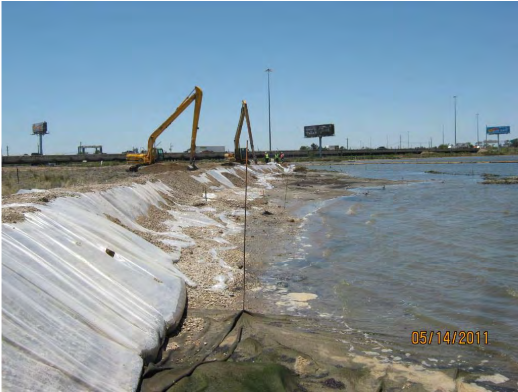
Photo 2 – Construction of the northern berm of the Western Cell.
