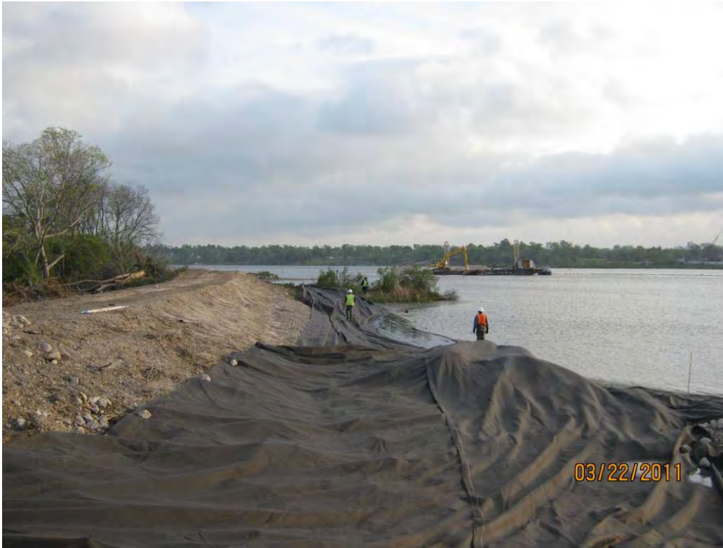
Photo 1 – Deploying geotextile along the east side of the central berm in the east cell.
