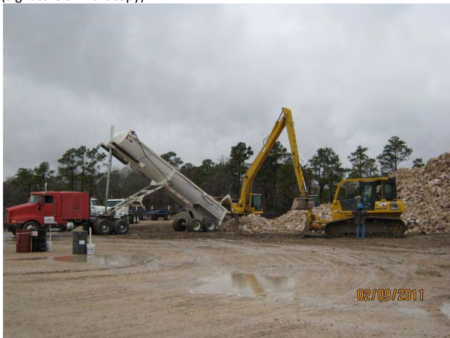
Photo 1 – Receiving Armor Cap D at LaBarge Property and maintaining stockpile with long-stick excavator
