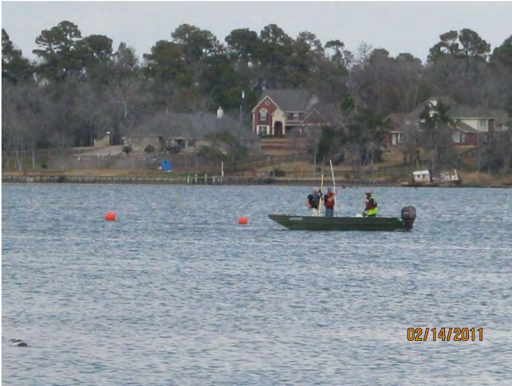
Photo 3 – Land Surveying, Inc. marking rock placement areas around the perimeter of the east cell of SJRWP
