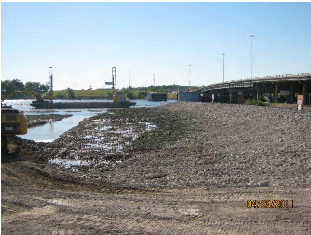
Photo 3 – Armor Cap A rock placed in the east cell to the south of the rock finger access road.
