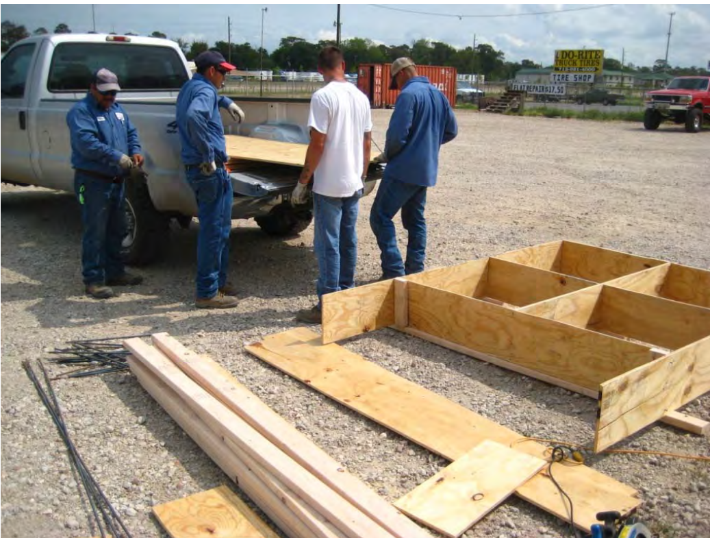
Photo 2 – Construction of concrete molds at the Admin area for pop-up signs to be placed at the SJRWP.
