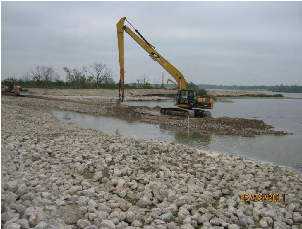
Photo 5 – Leading edge of the rock platform in the east cell prior to a bearing capacity failure.
