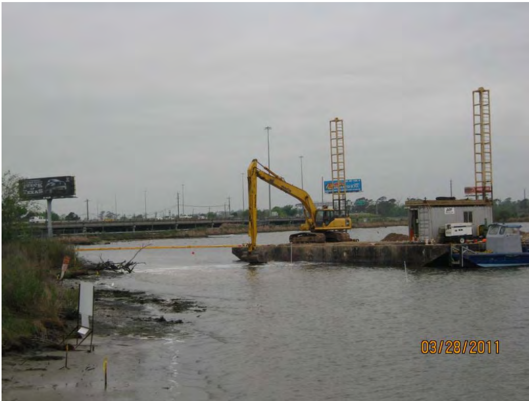
Photo 1 – Water-based operations placing Armor Cap A rock in the northwestern area.
