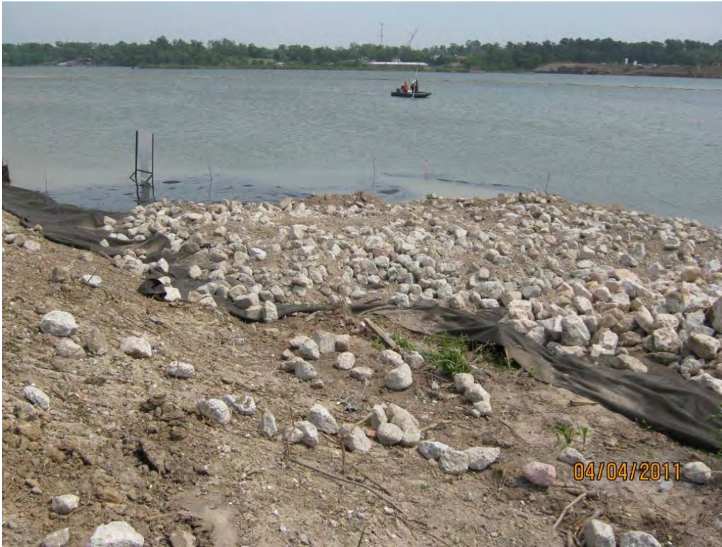
Photo 3 – Armor Cap B/C rock placed near the central berm in the east cell.
