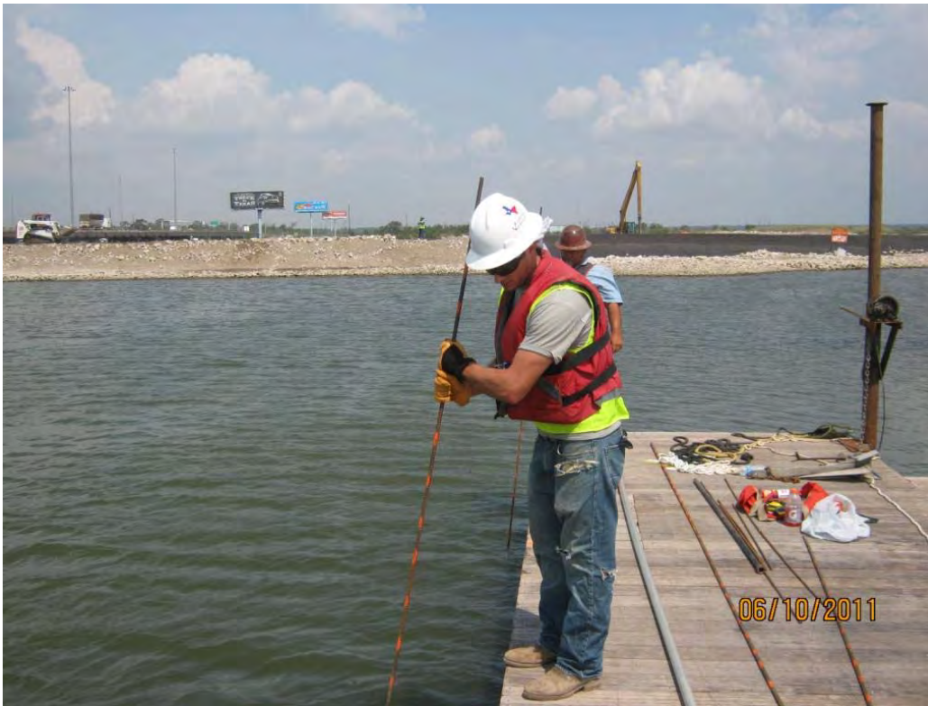
Photo 1 – Using a section of rebar to probe cap thickness in the Eastern Cell.
