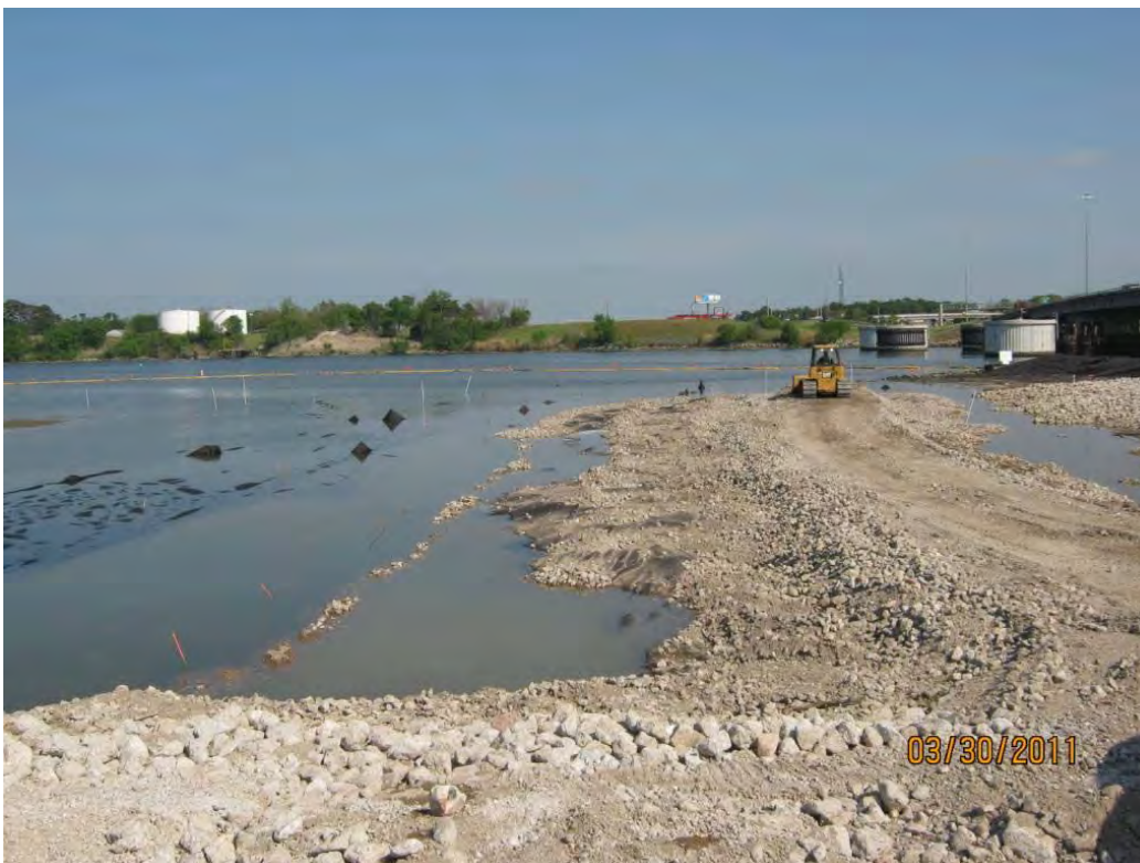
Photo 6 – New geotextile panel placed in the east cell north of the rock platform with rock placed along the north seam of the geotextile panel.
