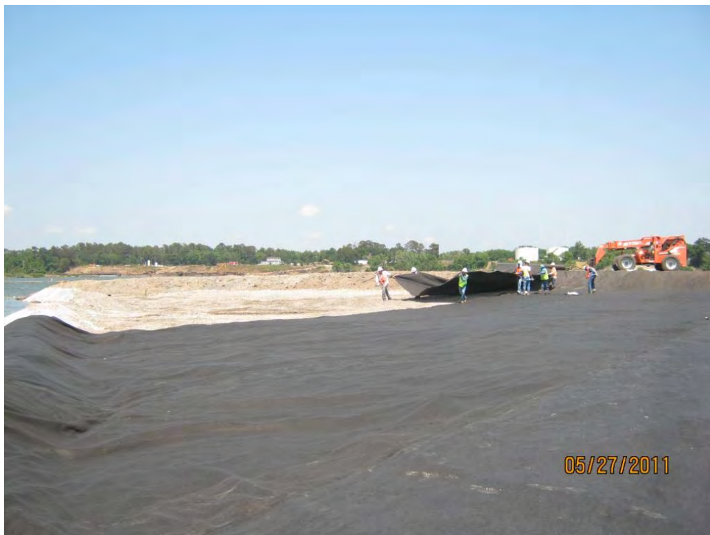
Photo 1 – Deploying 12-oz geotextile in the Western Cell.
