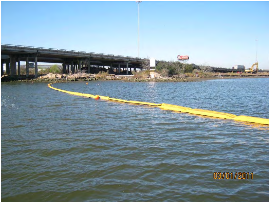
Photo 2 – Section of the turbidity curtain in the south half of the east cell that was repaired the morning of 2/28/11
