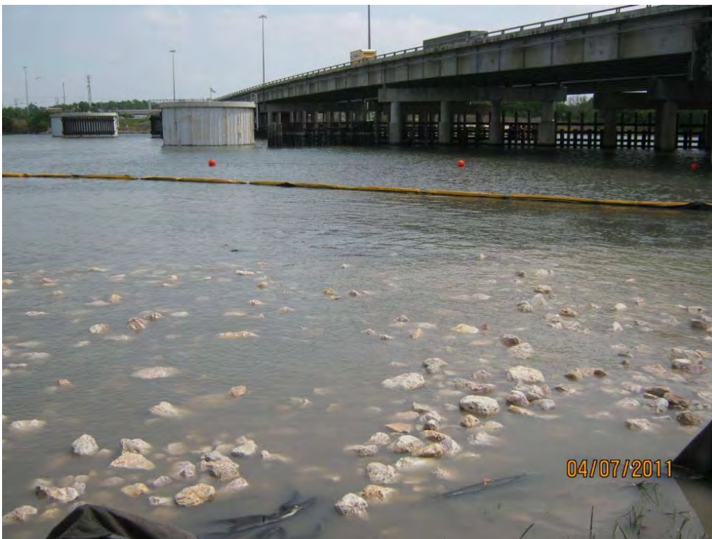
Photo 5 – Armor Cap D rock placed off the east end of the south berm.
