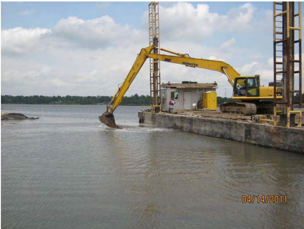
Photo 4 – Placing Armor Cap A rock in the east cell.
