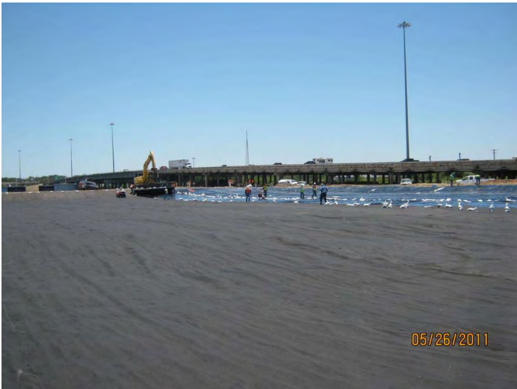
Photo 6 – Deploying LLDPE liner in the Western Cell.
