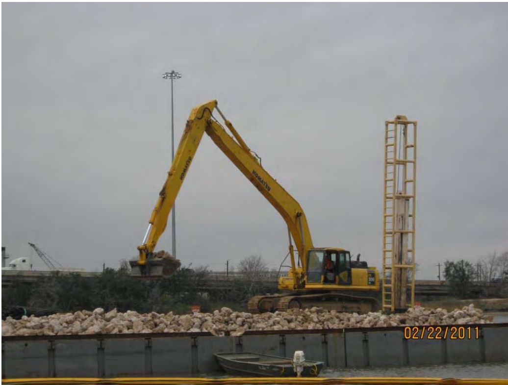
Photo 3 – Barge-mounted excavator loading rock from transport barge, viewed from work boat north of east cell
