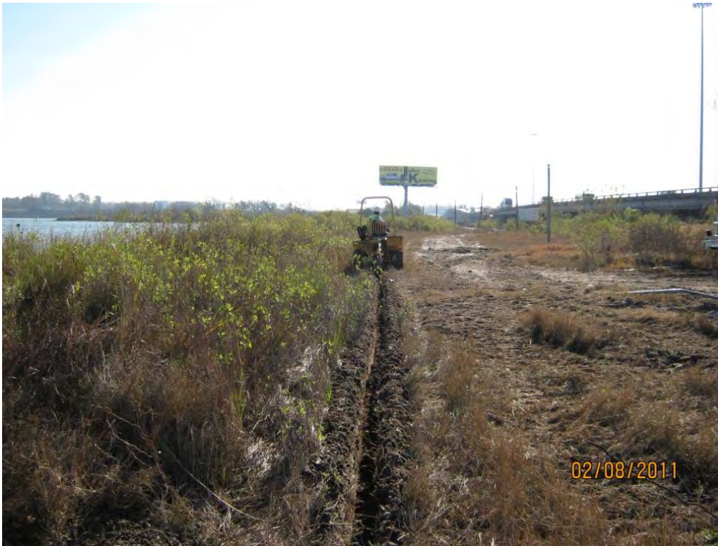
Photo 3 – Trenching machine for installation of silt fence along north side of TxDOT ROW property
