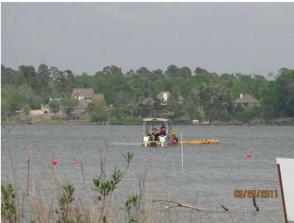
Photo 3 – USA crew deploying a turbidity curtain around the northwestern area.
