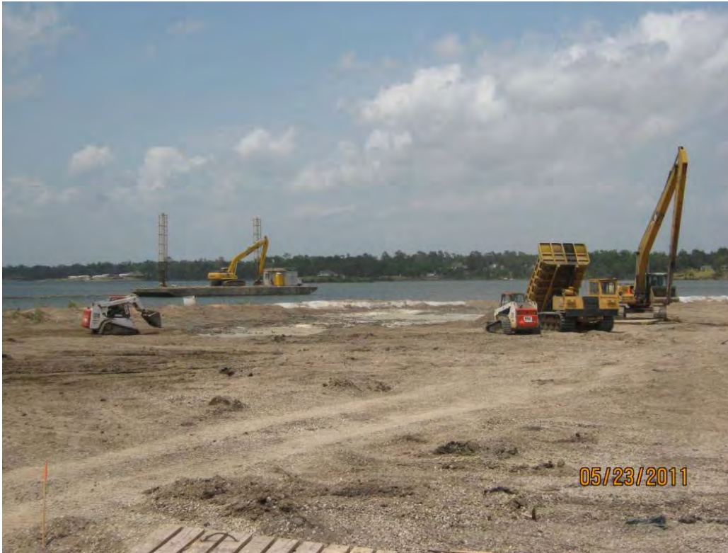
Photo 1 – Grading the surface of the Western Cell using long-reach excavator, Morooka truck, and skid-steers.
