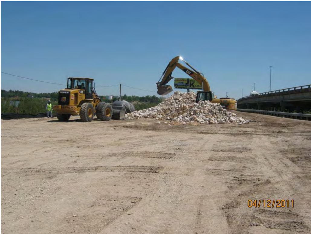
Photo 2 – Stockpiling Armor Cap D rock at the laydown area near the main access gate.
