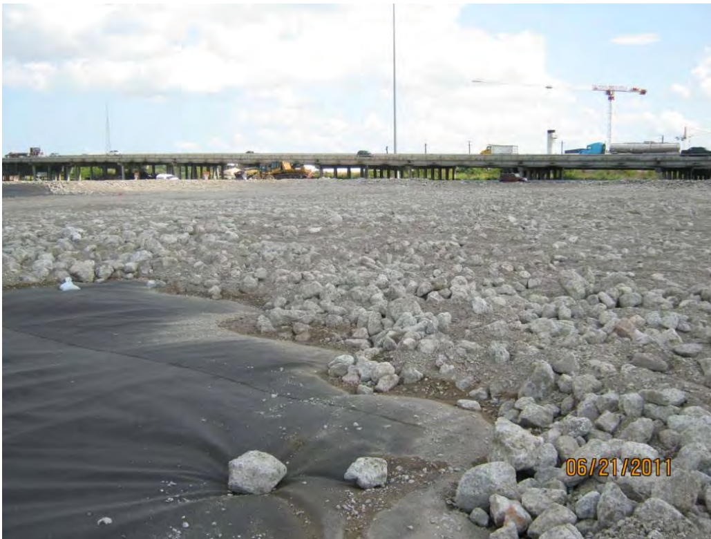
Photo 3 – Armor Cap B/C rock placed near the north end of the Western Cell.
