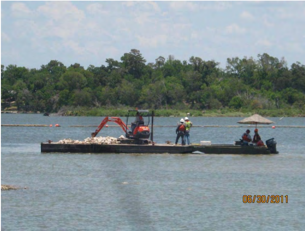
Photo 3 – Mini-excavator placing Armor Cap D rock in a shallow water area in the Eastern Cell.
