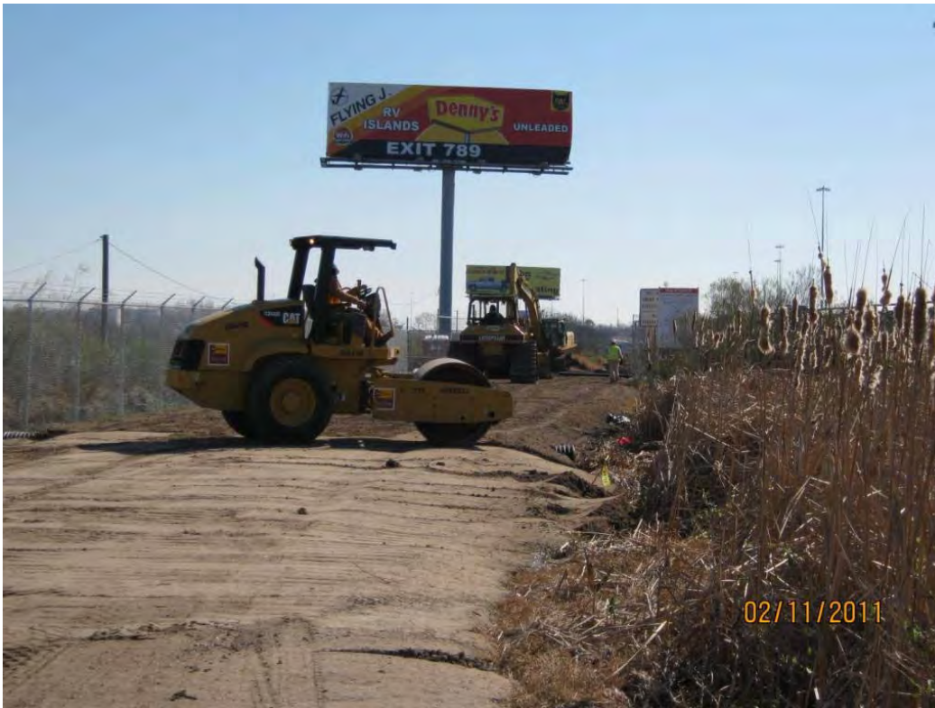
Photo 3 – Grading crushed concrete road base (background of photo) and compacting (foreground) at TxDOT ROW
