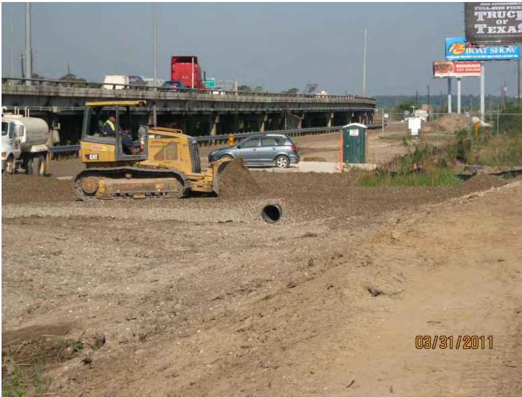
Photo 3 – Constructing a new access ramp to the south berm of the west cell.
