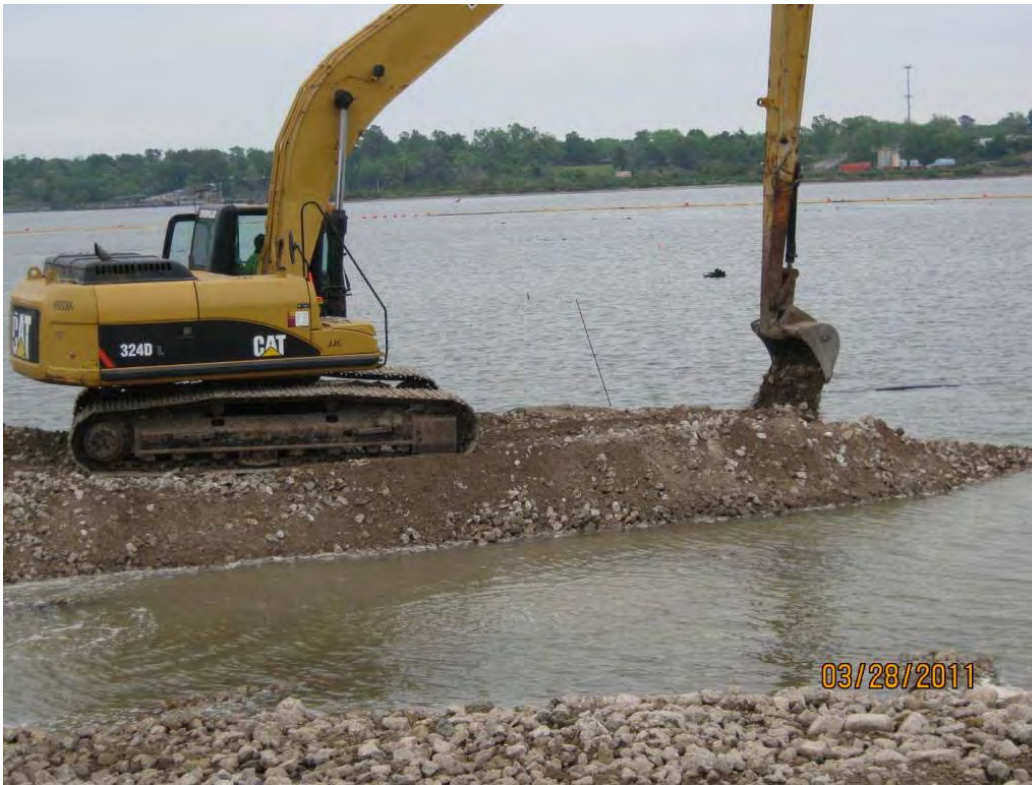
Photo 3 – Constructing a rock platform using Armor Cap A rock in the east cell.
