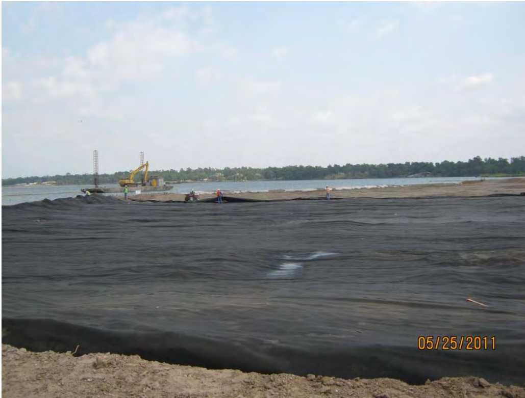
Photo 7 – Deploying geotextile in the Western Cell.
