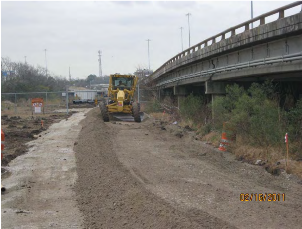
Photo 3 – Road grader shaping TxDOT ROW haul road to improve compaction of CCRB
