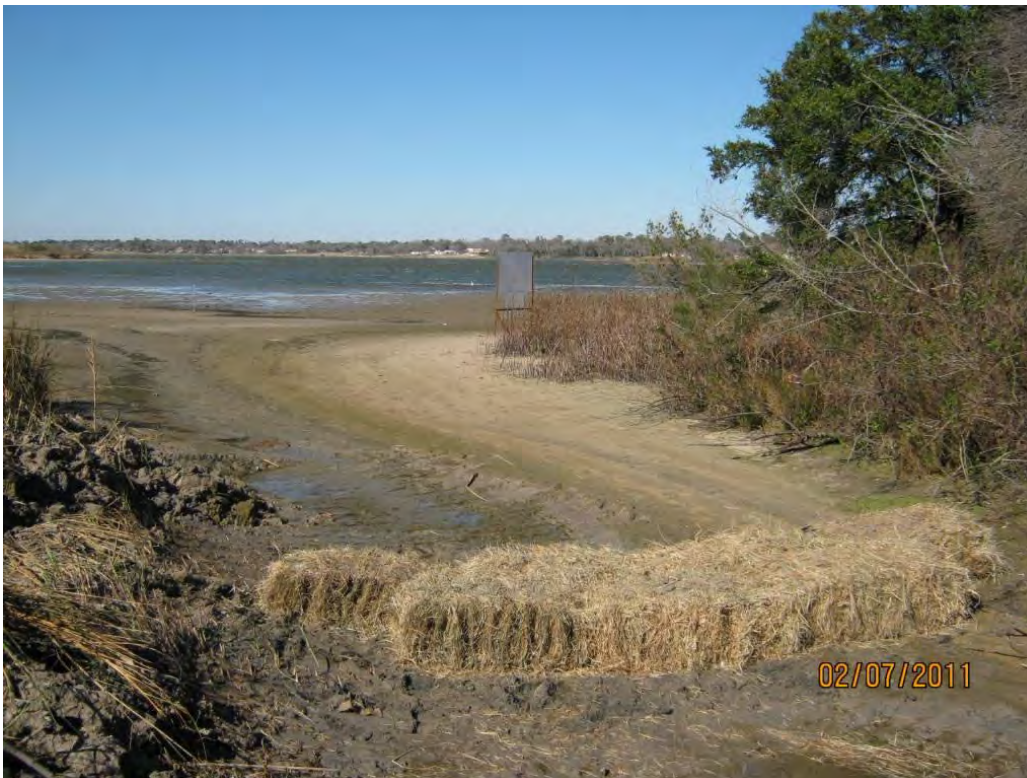
Photo 2 – Straw bales placed in surface water inlet and secured with stakes near southwest corner of western cell
