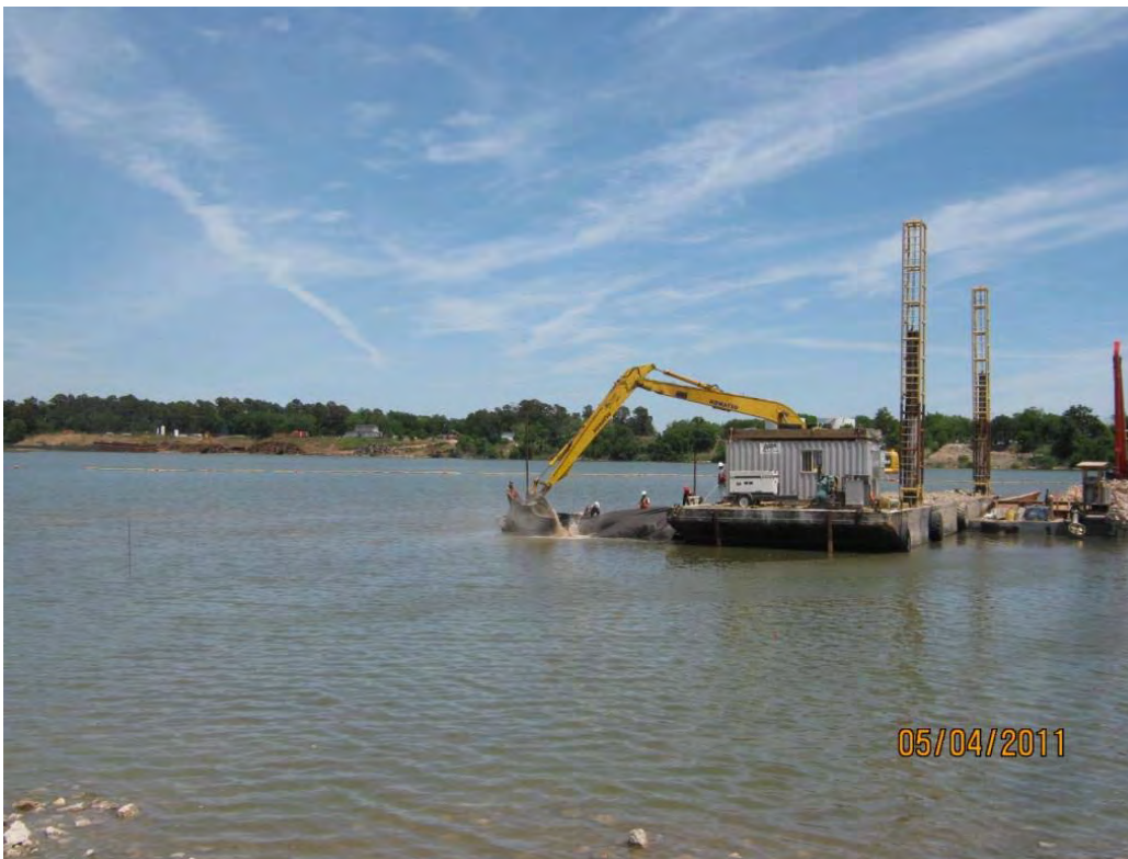
Photo 1 – Placing Armor Cap C rock in the Eastern Cell.
