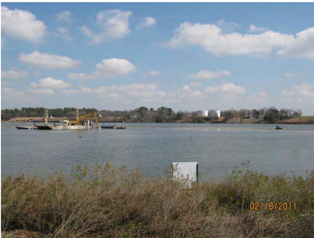
Photo 3 – Placing Armor Cap D rock in east cell (at left of photo) and monitoring turbidity (at right of photo)
