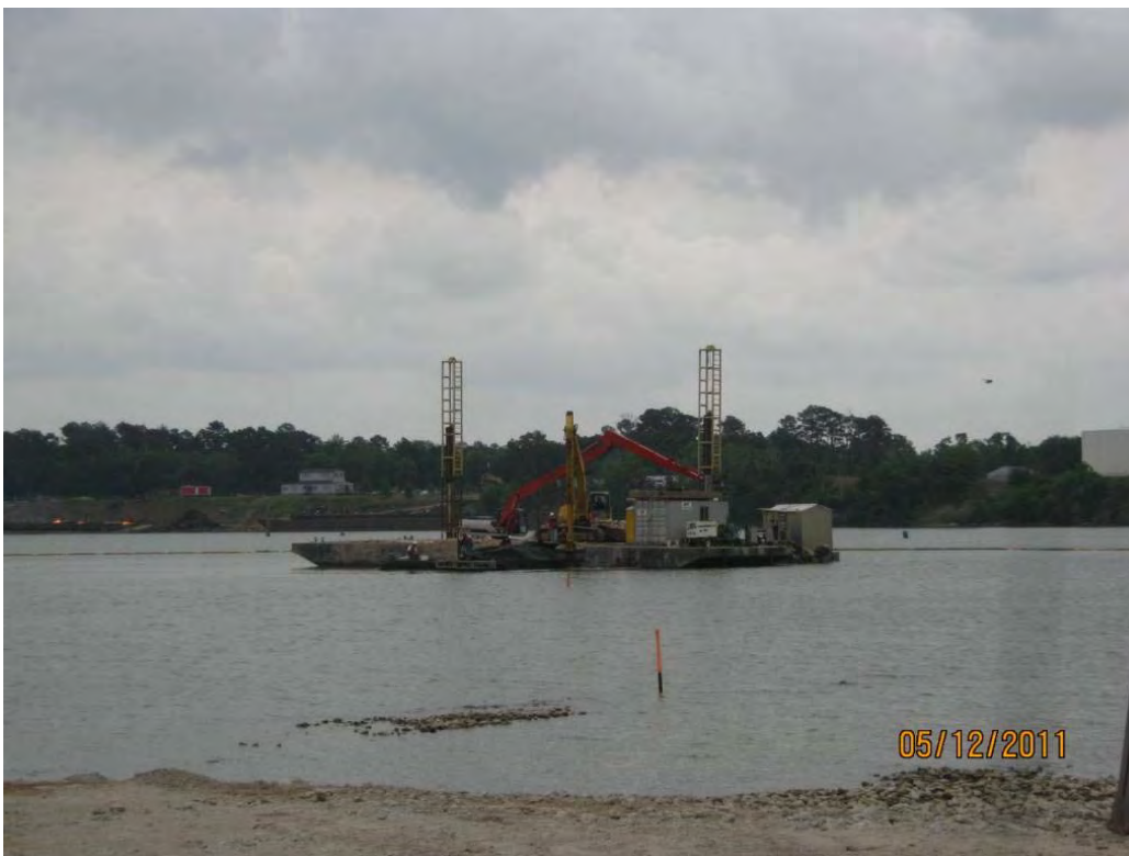
Photo 4 – Placing geotextile and Armor Cap C rock in the Eastern Cell.
