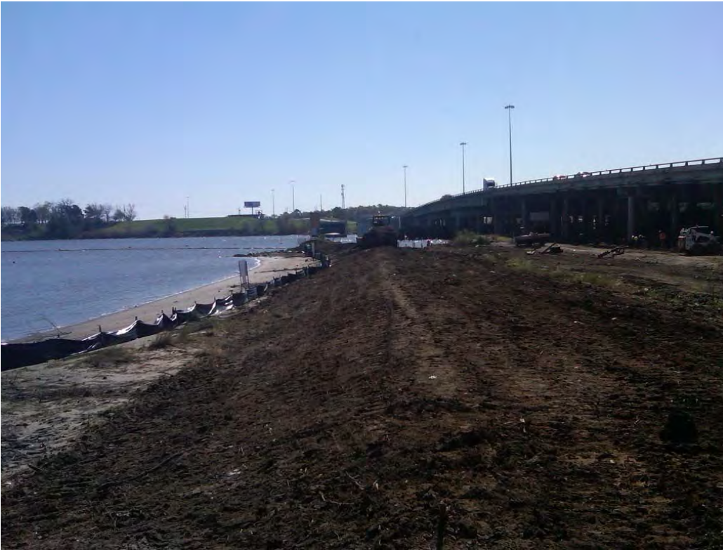
Photo 3 – Grading the north slope of the east cell to establish a stable slope for future rock placement
