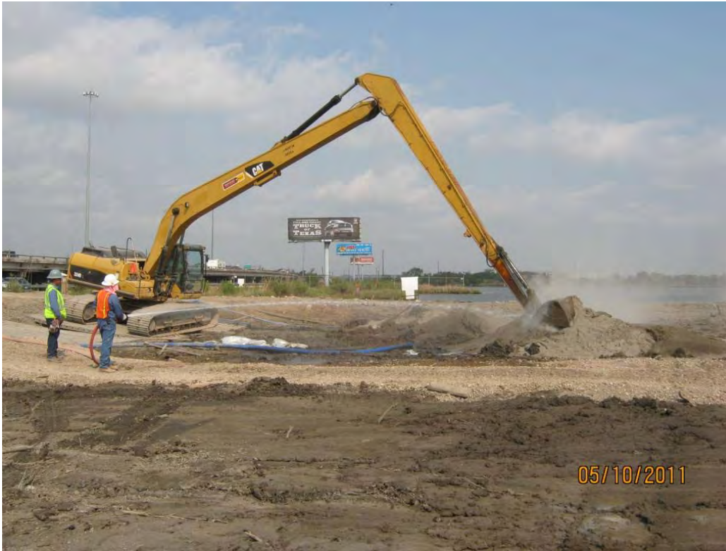
Photo 1 – Delivering Portland cement to the Western Cell; crew with water hose at left of photo to mitigate dust.
