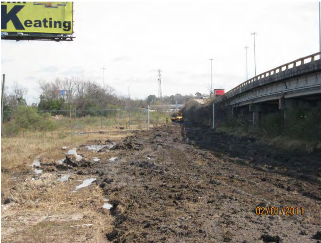
Photo 2 – Dozer performing grading and drainage improvements on TxDOT ROW.
