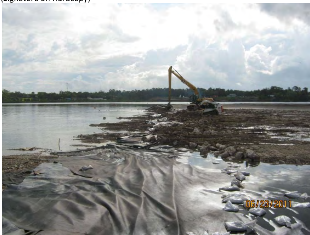
Photo 1 – Long-reach excavator removing the temporary northern berm and skidsteer placing Armor Cap B/C rock.
