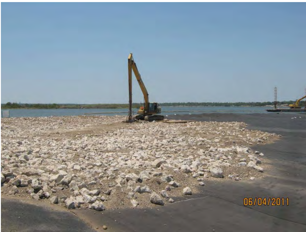
Photo 2 – Placing Armor Cap B/C rock in the west portion of the Western Cell.
