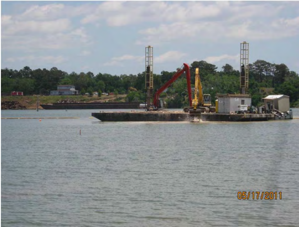
Photo 5 – Placing Armor Cap D rock in the Eastern Cell.
