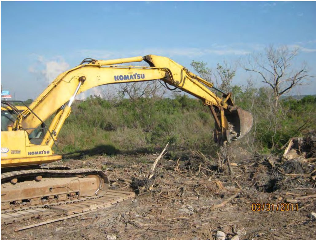
Photo 1 – Mashing stumps in the west cell and placing in low-lying areas in the west cell.
