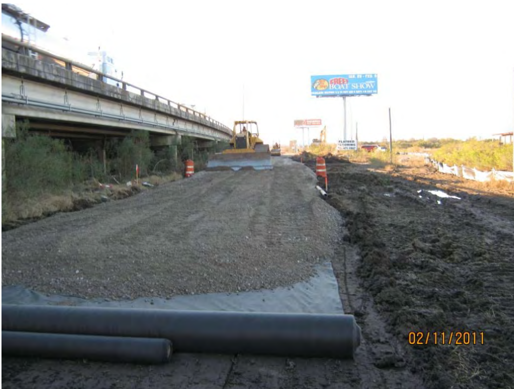
Photo 4 – Grading crushed concrete road base atop geotextile (foreground) and compacting (background) at TxDOT ROW
