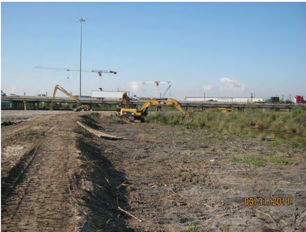
Photo 2 – Eastern portion of the west cell after smoothing the ground surface in preparation for geotextile deployment.
