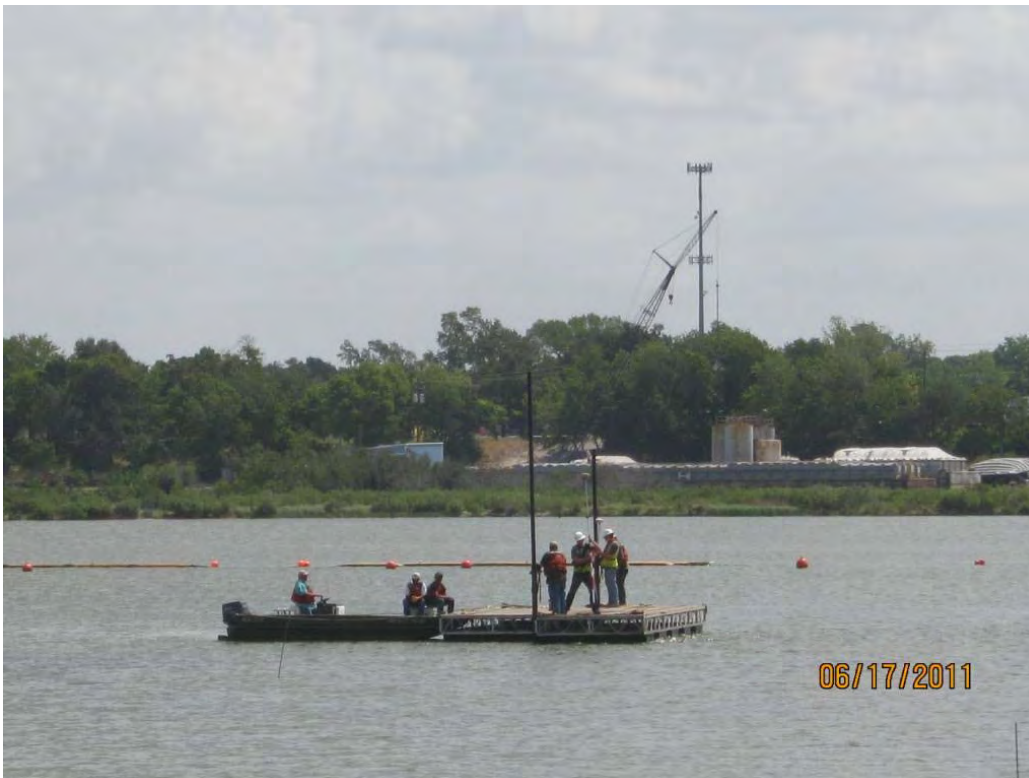
Photo 3 – Work and survey crews positioning the floating dock for probing armored cap thickness.
