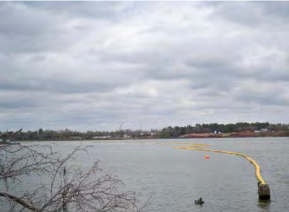
Photo 3 – Minor curtain displacement onto the site.
