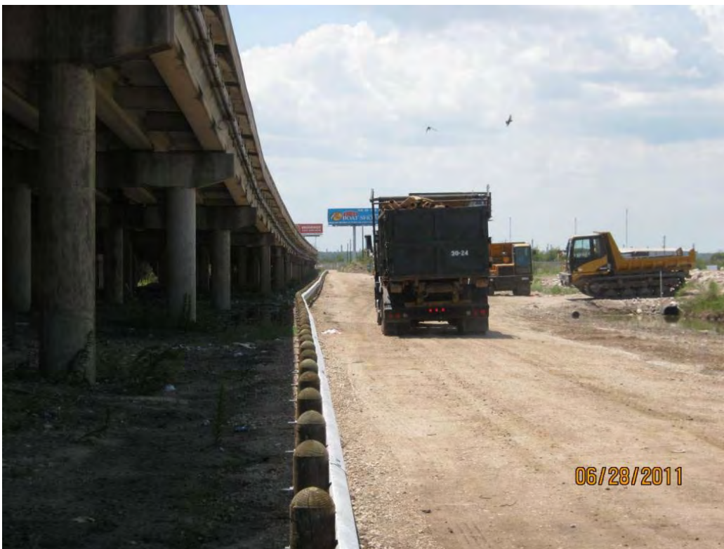
Photo 2 – Loaded roll-off box departing the TxDOT ROW to transport debris to Coastal Plains RDF.
