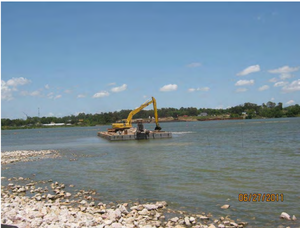
Photo 4 – Barge-mounted excavator placing Armor Cap D rock in the Eastern Cell at a location identified by the surveyor.
