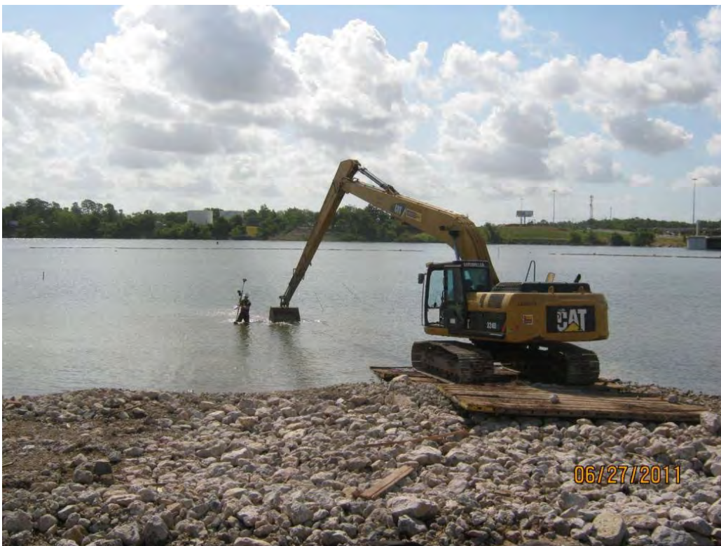
Photo 2 – Long-reach excavator placing Armor Cap A rock in the Eastern Cell at a location identified by the surveyor.
