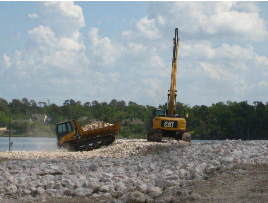
Photo 2 – Delivering and placing Armor Cap D rock at the north end of the central berm in the Western Cell.
