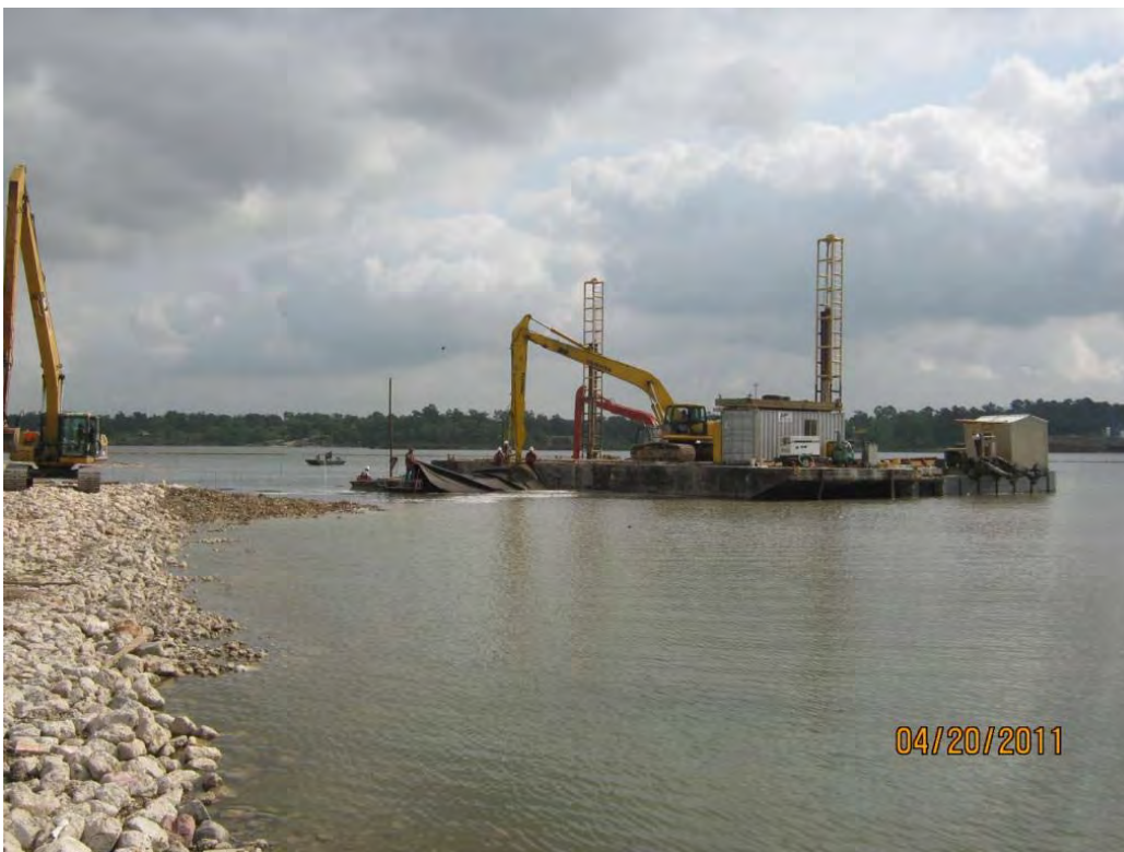
Photo 2 – Placing Armor Cap A rock via land-based operations (at left) and water-based operations (at right).
