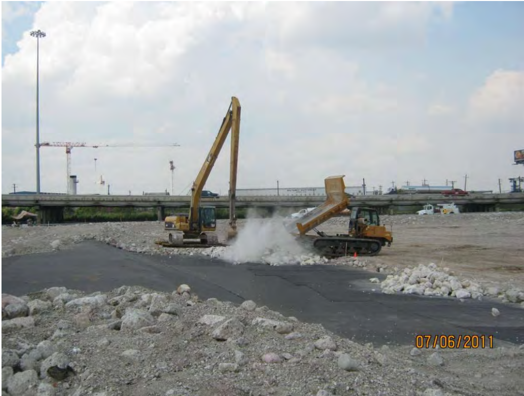
Photo 3 – Delivering and placing Armor Cap D rock in the Western Cell.
