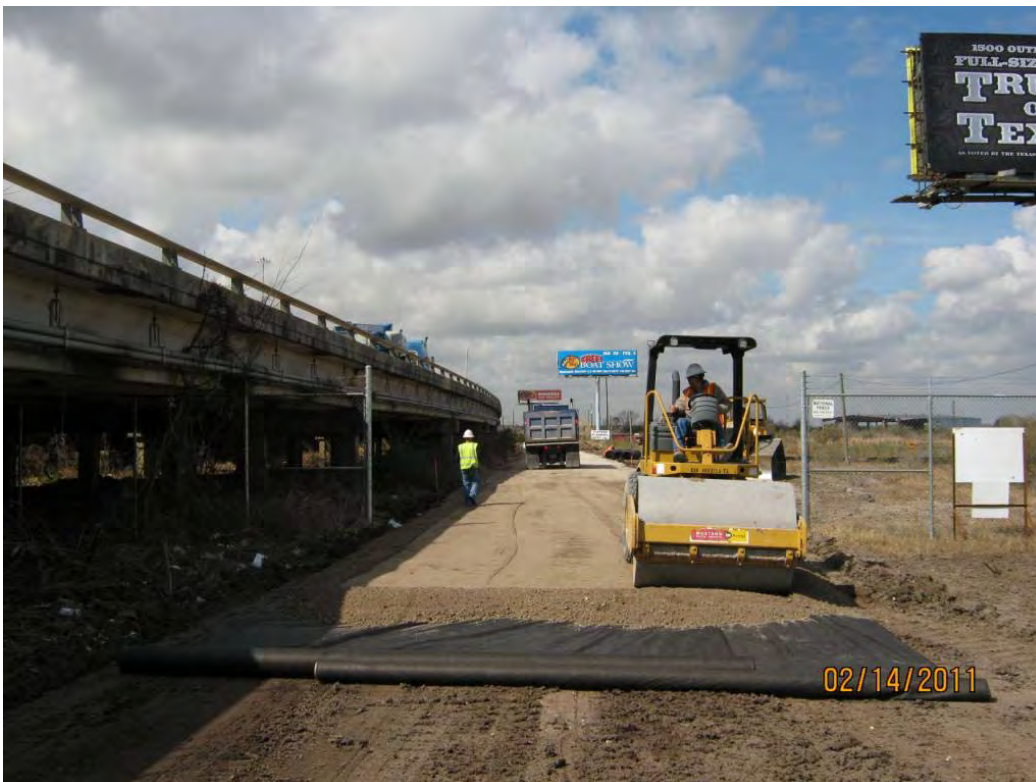
Photo 2 – Receiving and compacting CCRB atop geotextile near the Phase I fence line along TxDOT ROW
