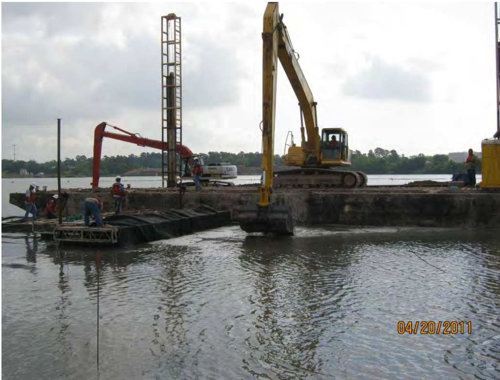
Photo 3 – Deploying geotextile and placing Armor Cap A rock in the east cell.
