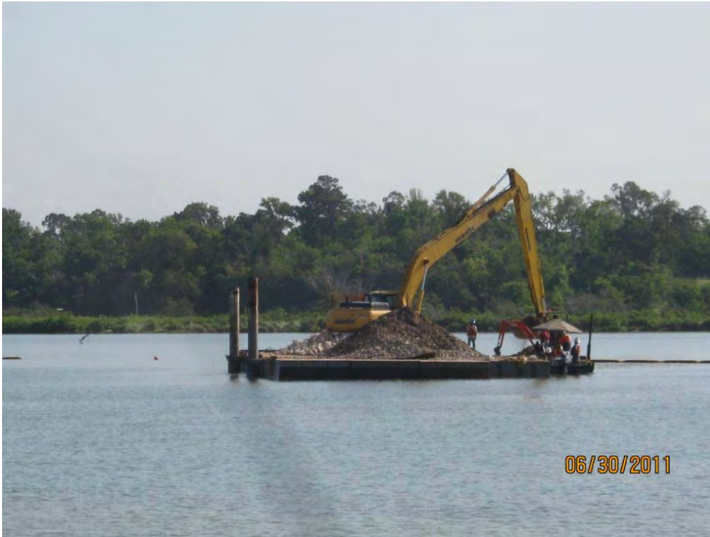
Photo 1 – Barge-mounted excavator placing Armor Cap A rock onto mini-barge to access shallow-water areas.
