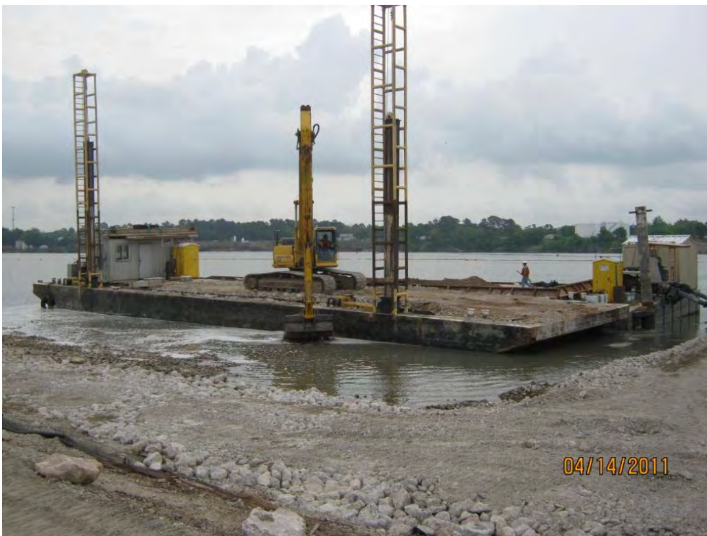
Photo 2 – Placing Armor Cap A rock in the east cell.
