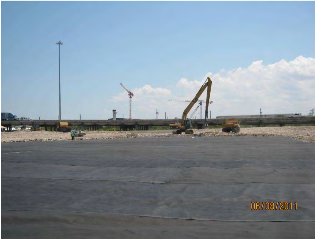
Photo 3 – Placing Armor Cap B/C rock in the south portion of the Western Cell.
