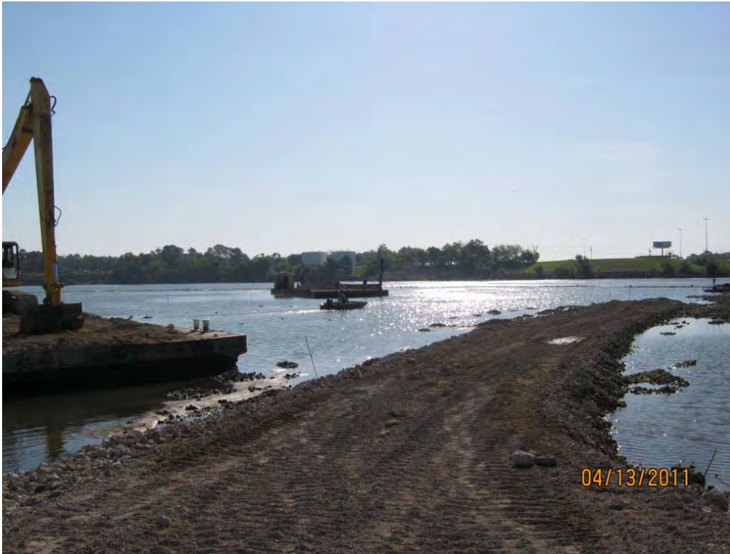
Photo 5 – Aggregate transport barge unable to reach the barge-mounted excavator in the morning due to low tide elevation, despite the barge being loaded to only one-half of its capacity.
