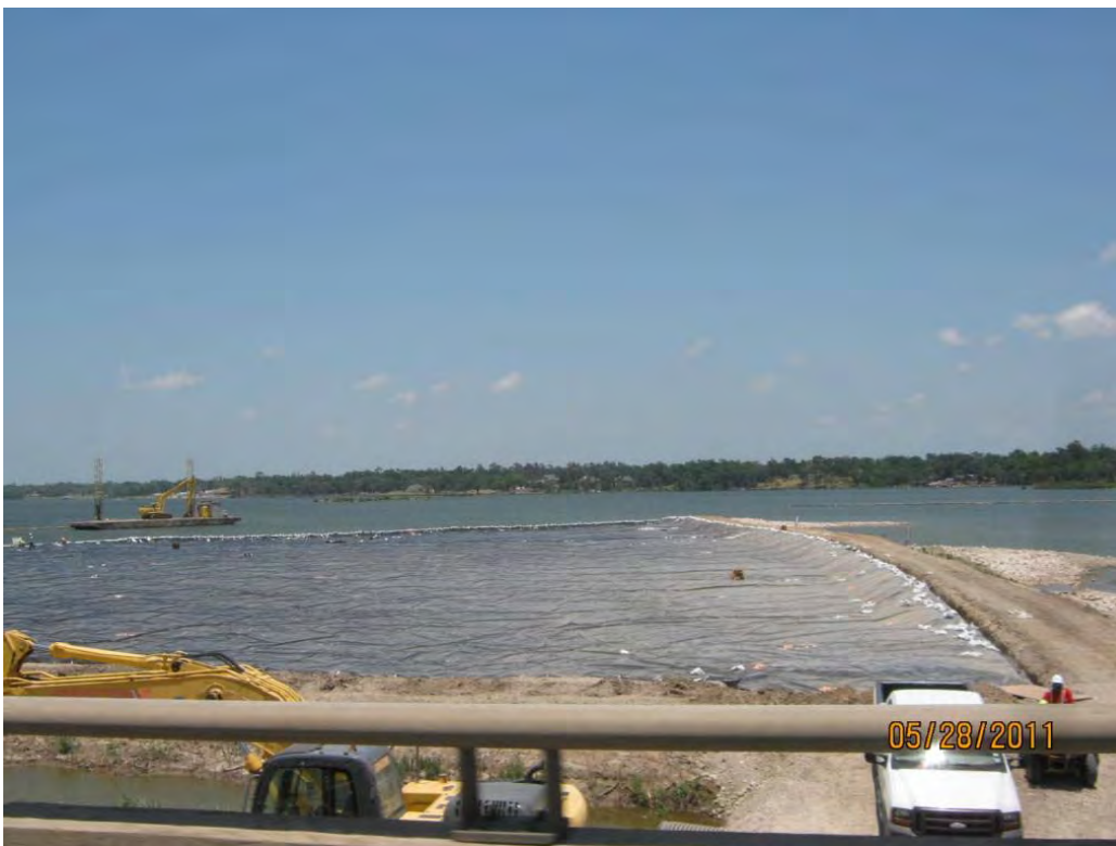
Photo 4 – Overview of the Western Cell after the LLDPE liner has been fully deployed.
