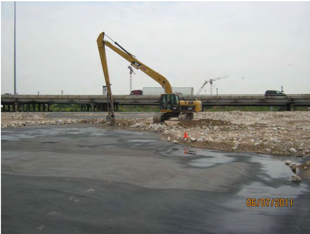
Photo 3 – Placing Armor Cap B/C rock near the south berm in the Western Cell.
