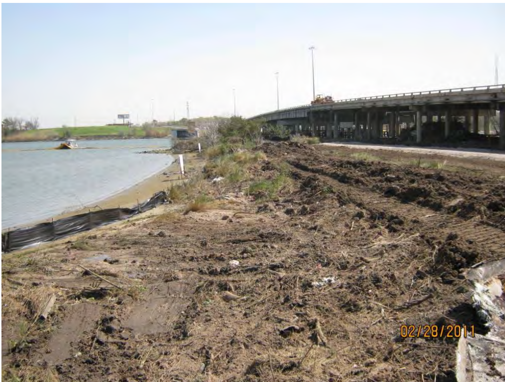
Photo 3 – Repairing breach in turbidity curtain (to left of photo) and south berm of east cell (to right of photo)
