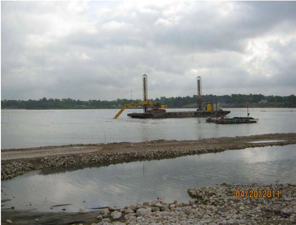
Photo 1 – Repositioning the barge-mounted excavator in the east cell to a position closer to the central berm.
