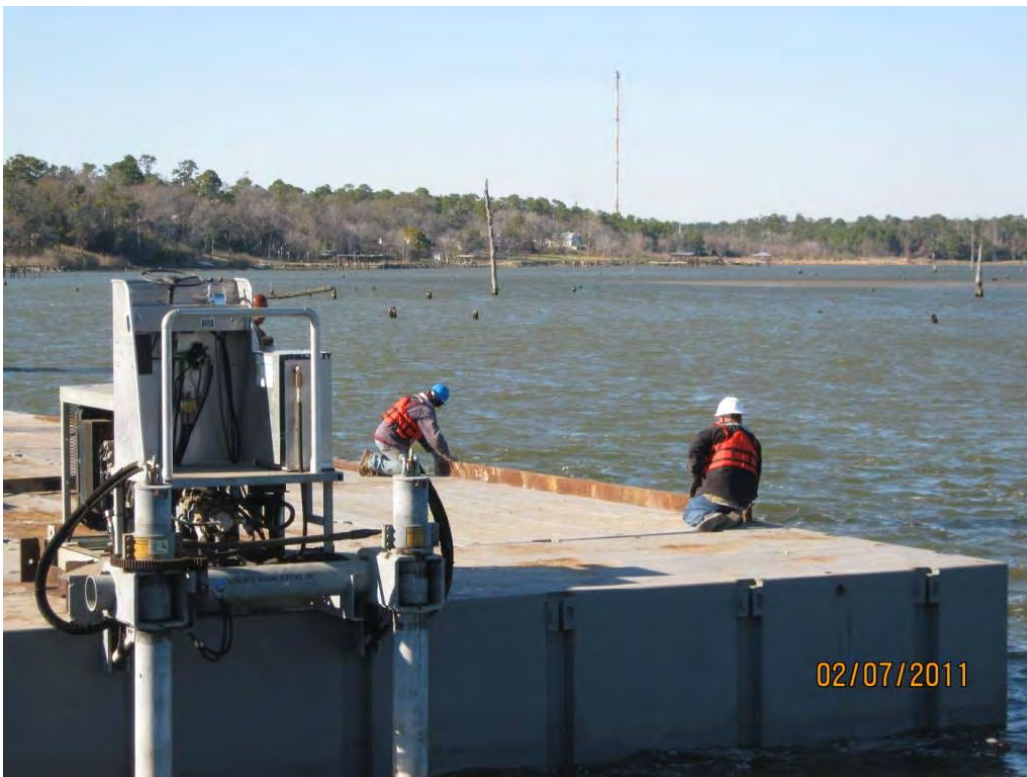
Photo 6 – Affixing 6-inch steel rail to starboard side of aggregate transport barge
