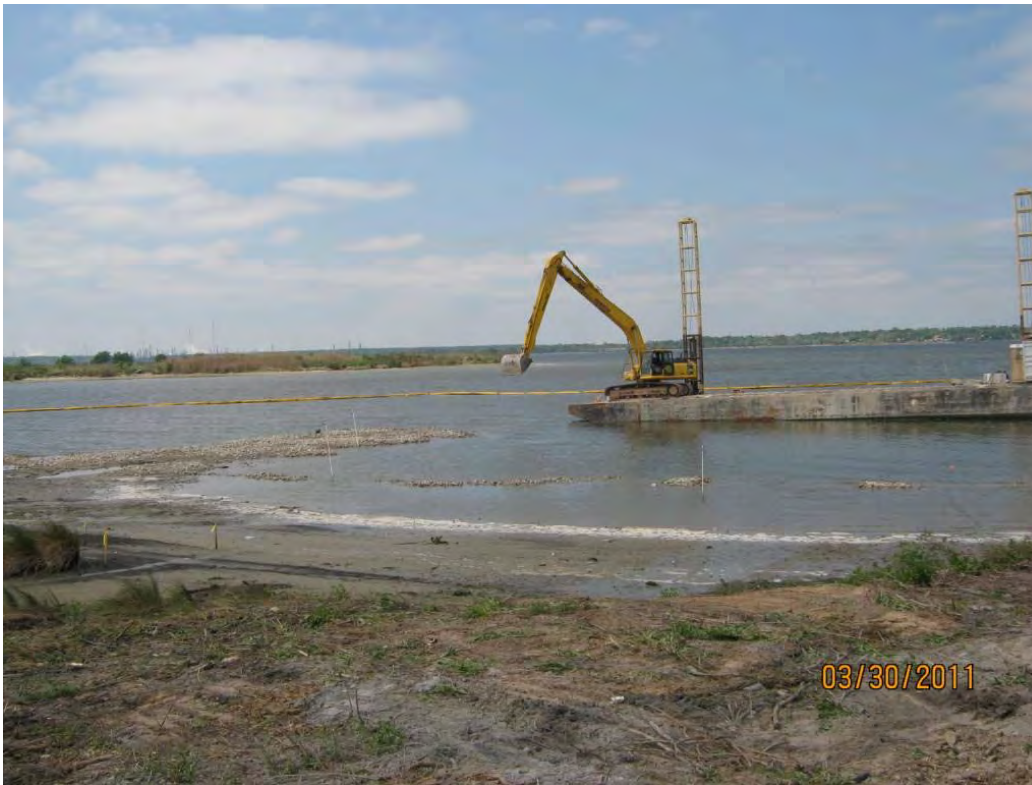
Photo 3 – Water-based operations placing Armor Cap A rock in the northwestern area.
