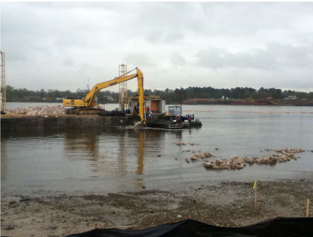
Photo 2 – Placing Armor Cap D rock in east cell.
