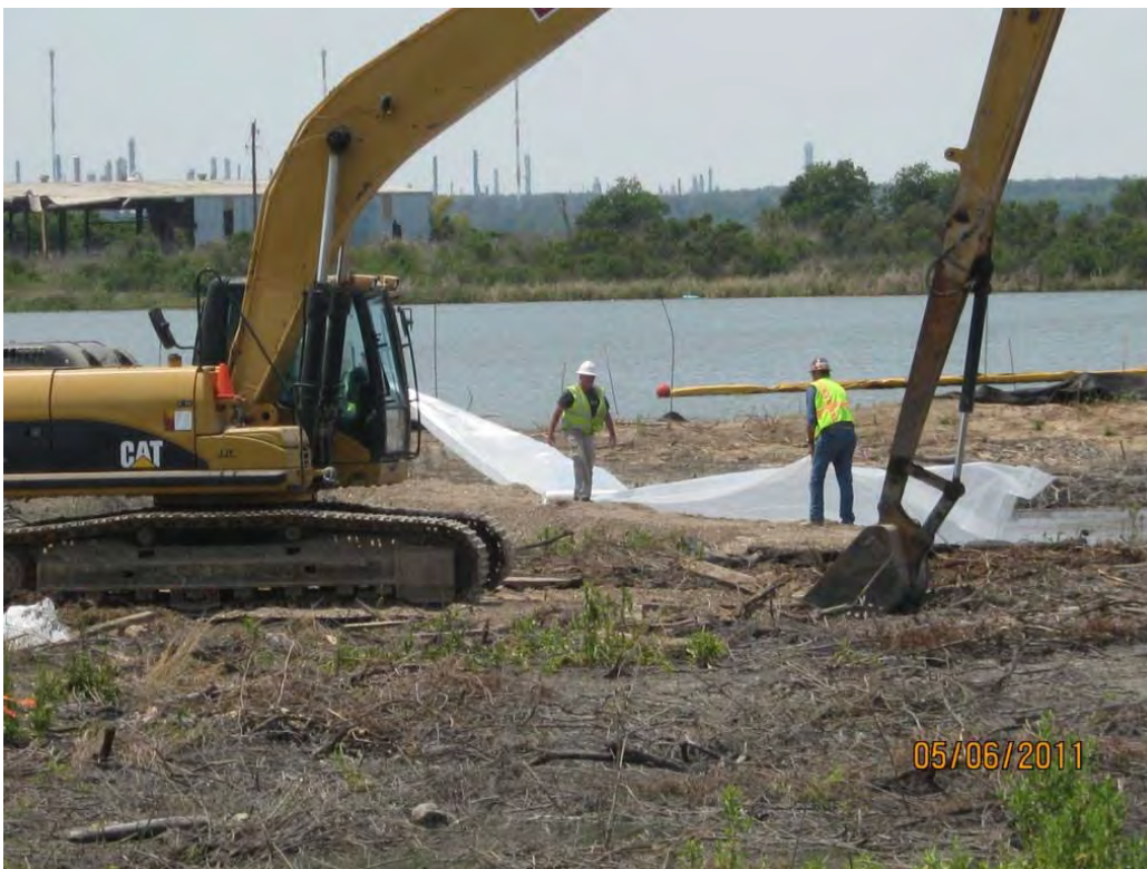
Photo 3 – Installing visqueen plastic along the interim berm in the west low-lying area in the Western Cell.
