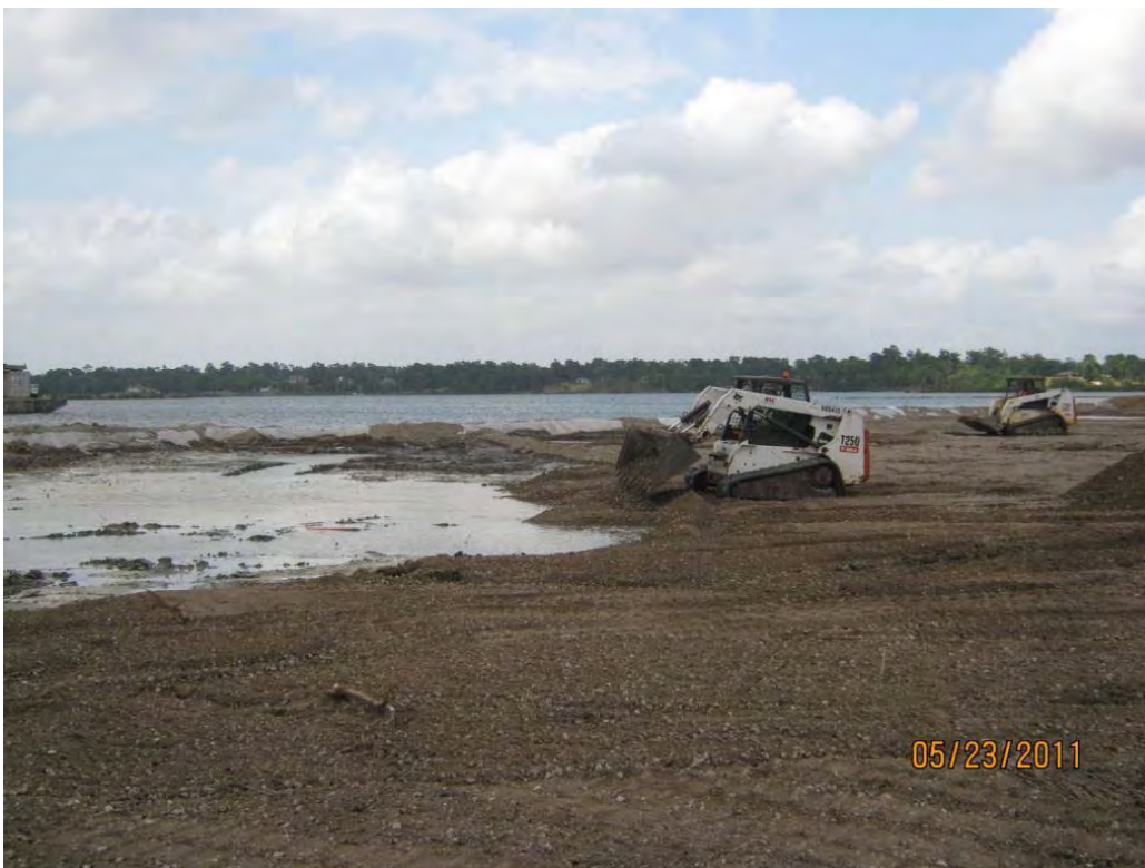
Photo 2 – Skid-steer using crushed concrete road base to grade the surface of the Western Cell.
