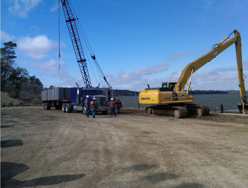
Photo 5 – Delivering sectional barges at LaBarge property and offloading to water using a crane.
