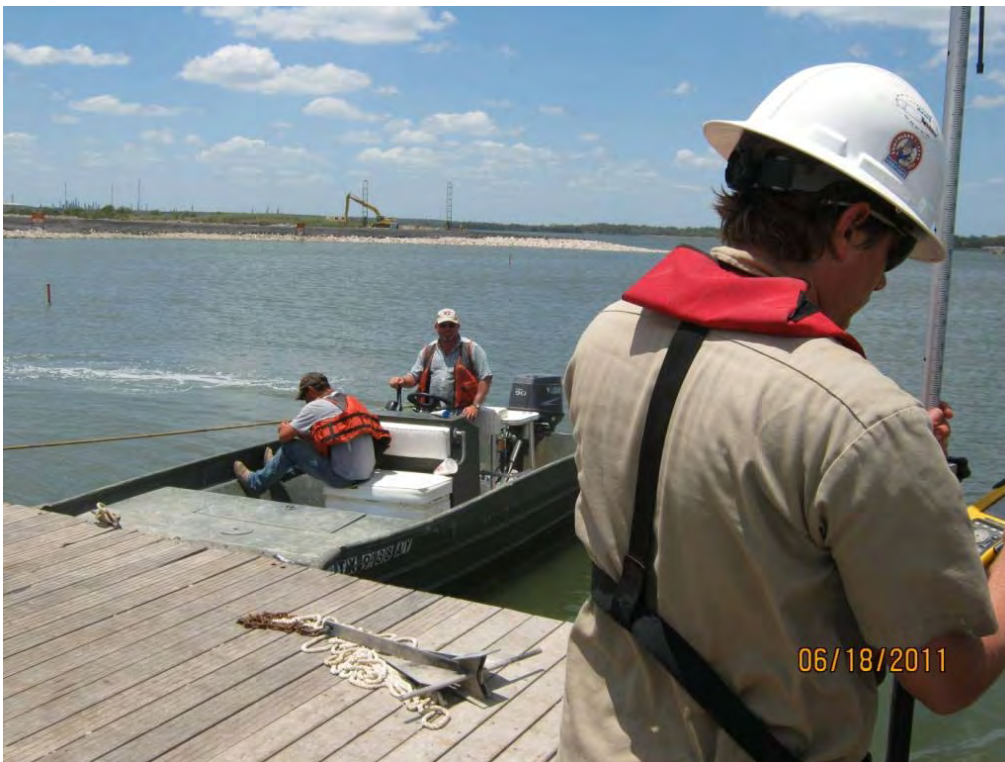
Photo 1 – Surveyor guiding the boat operator to an armored cap thickness probe location.
