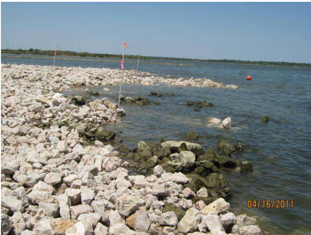
Photo 3 –Armor Cap C rock placed via land-based operations adjacent to Armor Cap D rock placed via water-based operations.
