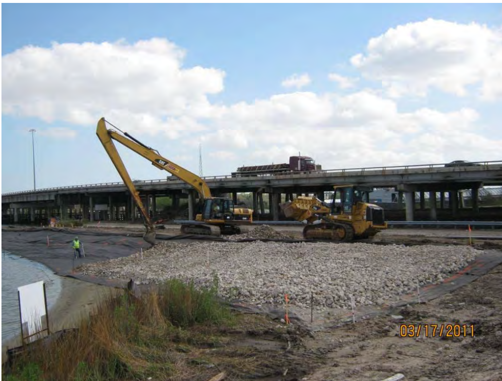
Photo 8 – Placing Armor Cap A on the south berm of the east cell.
