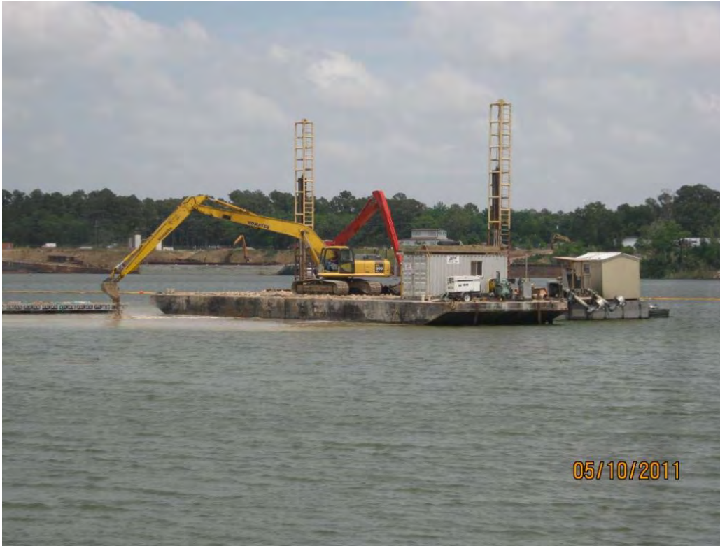
Photo 5 – Placing Armor Cap C rock in the Eastern Cell.
