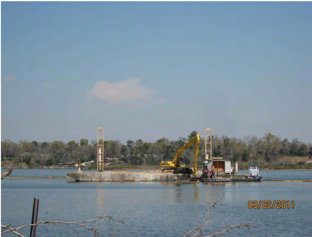
Photo 1 – Deploying geotextile and placing Armor Cap D rock in the east cell
