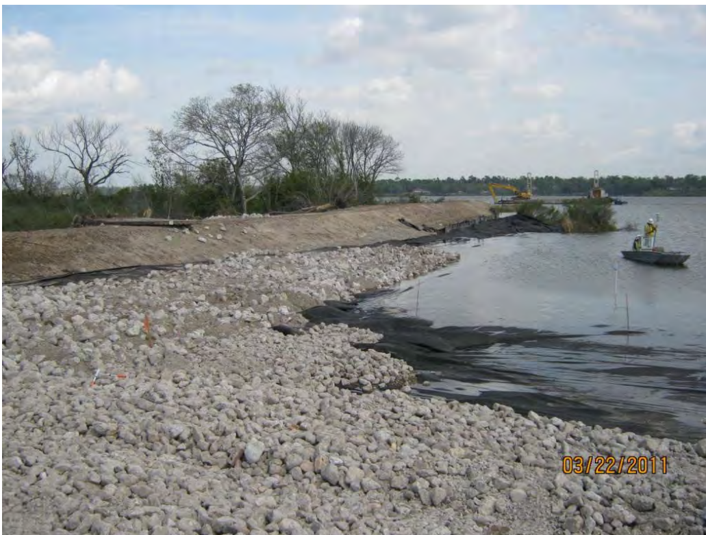
Photo 2 – Armor Cap B/C placed parallel to the central berm in the east cell.
