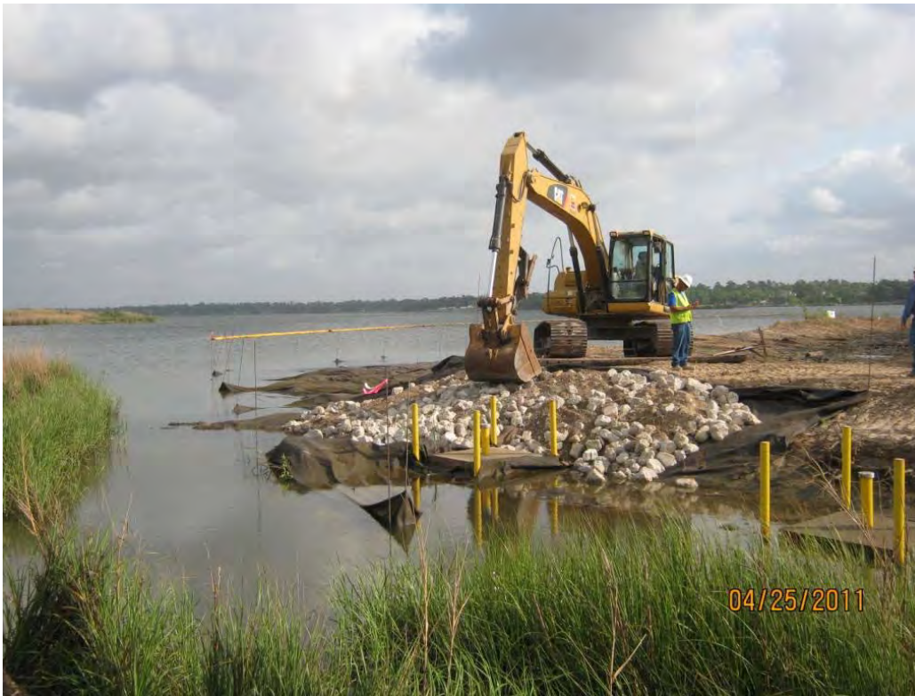
Photo 1 – Armor Cap B/C rock placed outside the southwest corner of the west cell.
