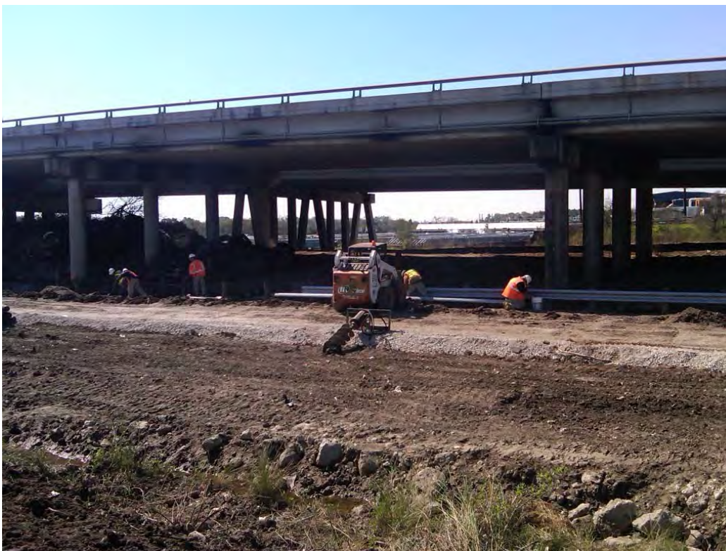
Photo 6 – Installing the guard rail adjacent to the I-10 Bridge to the south of the east cell
