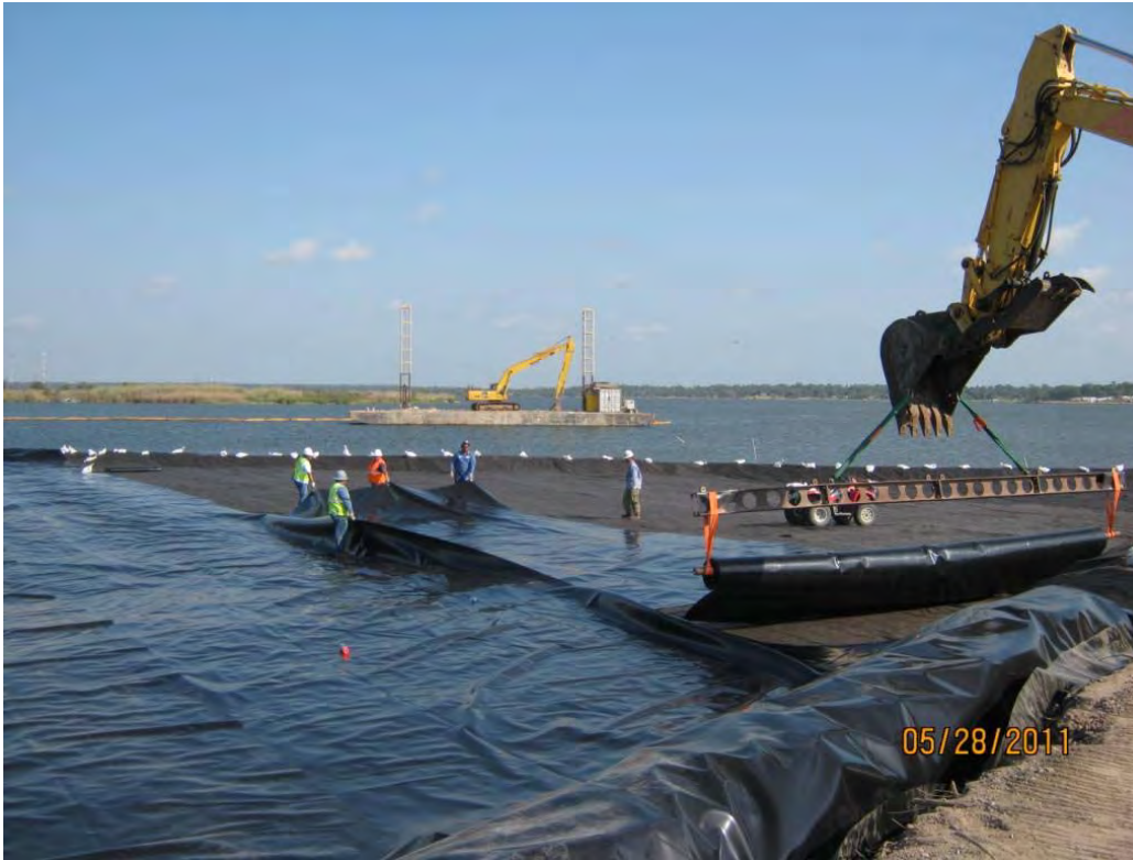
Photo 1 – Deploying LLDPE liner in the Western Cell.
