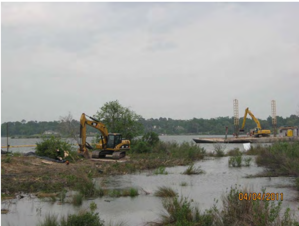
Photo 2 – Clearing vegetation along the west berm of the west cell in preparation for geotextile deployment.
