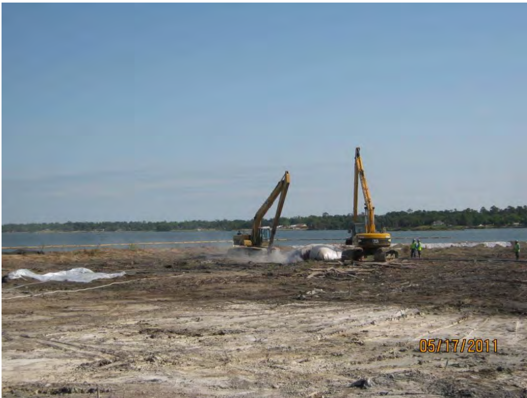
Photo 2 – Receiving Portland cement for mixing into a low-lying area in the northwest portion of the Western Cell.
