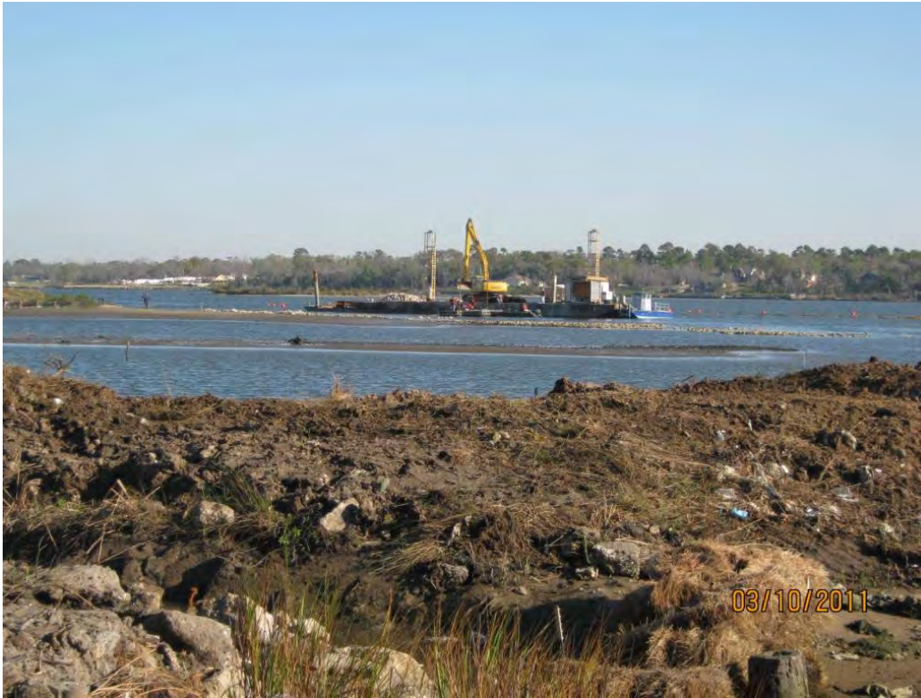
Photo 1 – Placing Armor Cap D rock in the east cell during low tide caused by north wind; the south berm of the east cell is in the foreground of the photo
