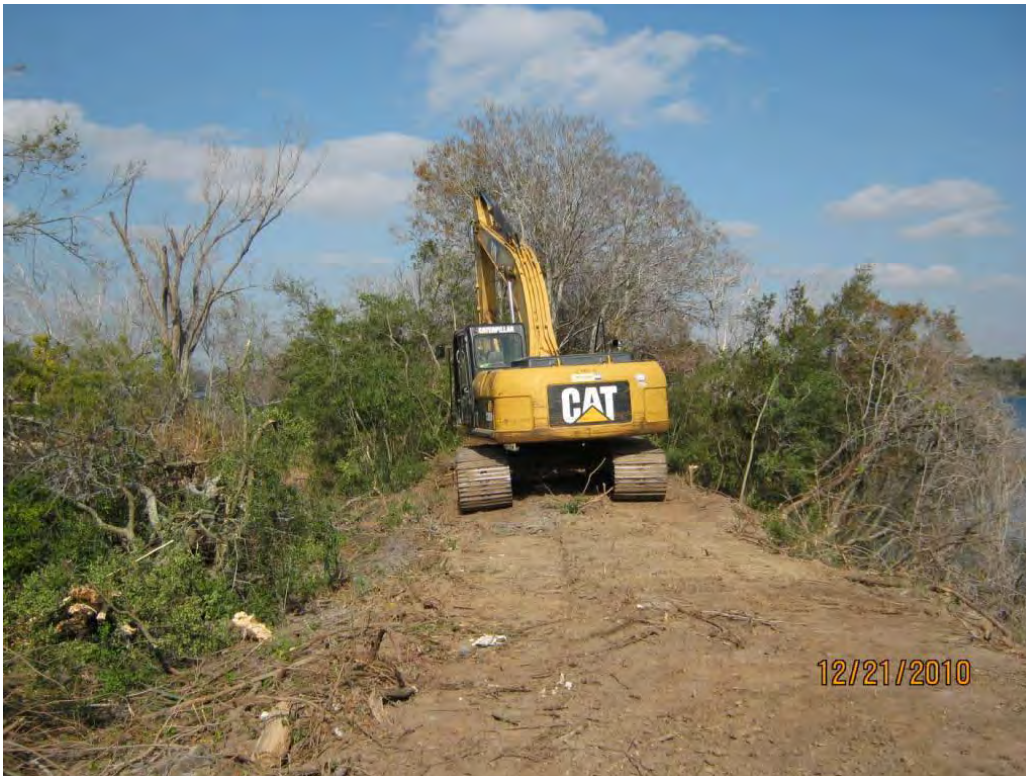
Photo 2 – Clearing vegetation from atop central berm, approximately 100 feet north of southern berm.
