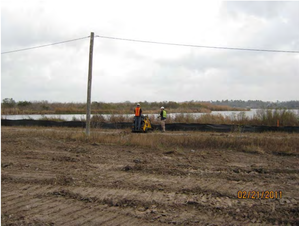
Photo 3 – Digging post hole for relocation of overhead electric line to billboards at TxDOT ROW
