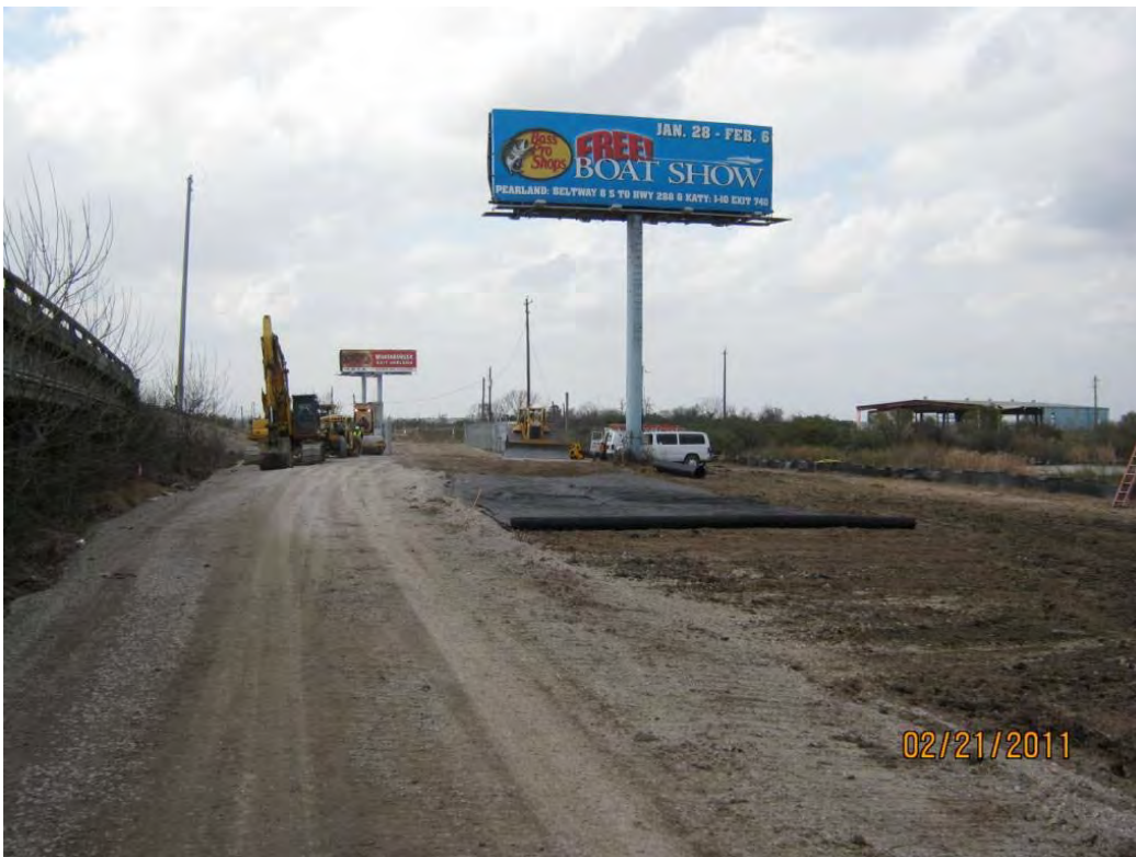
Photo 4 – Geotextile and CCRB placement for equipment laydown area inside main access gate at TxDOT ROW
