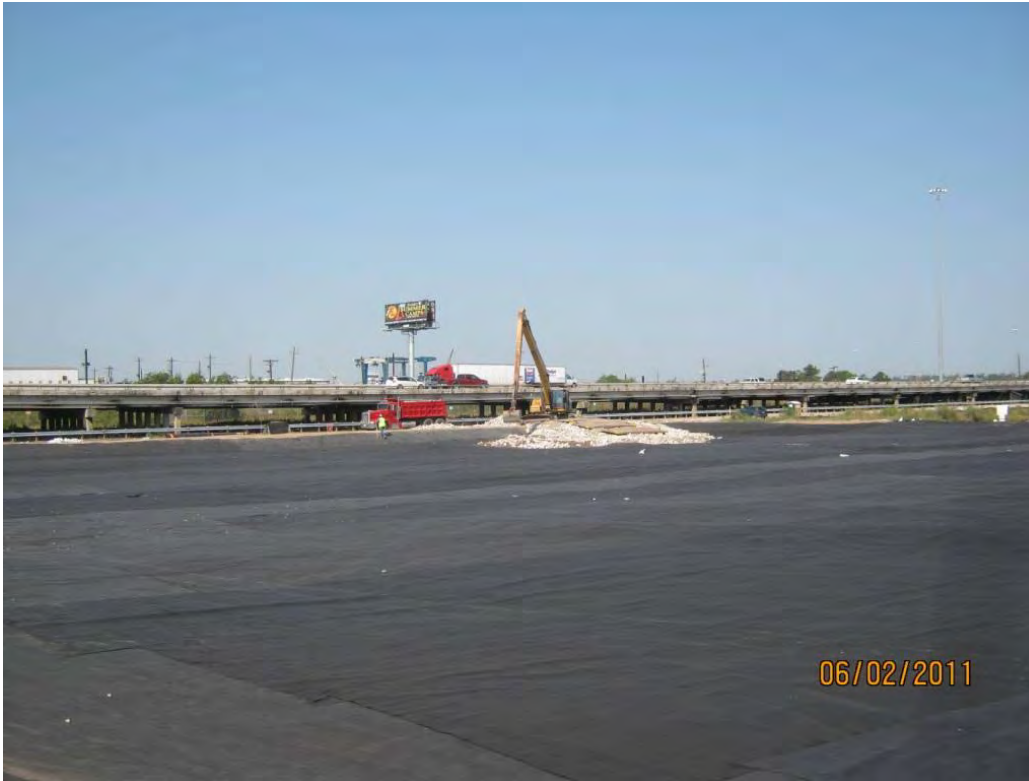
Photo 5 – Long-reach excavator placing Armor Cap B/C rock in the Western Cell.
