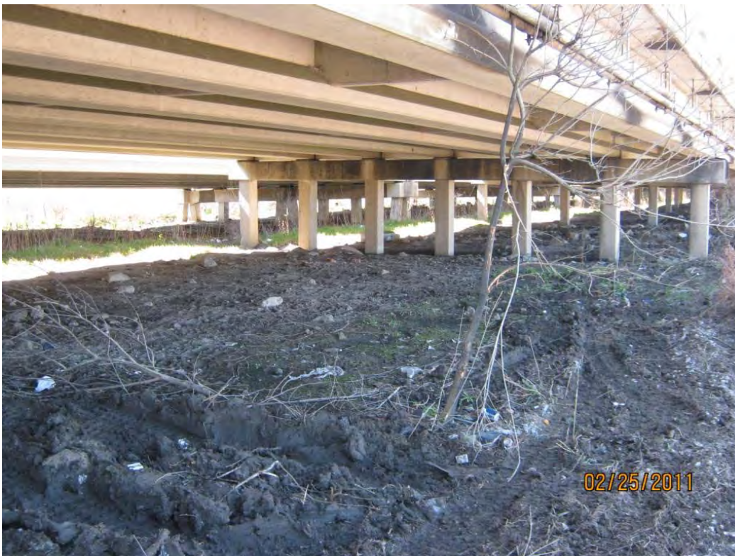
Photo 6 – Area under I-10 Bridge after debris removal using skidsteer
