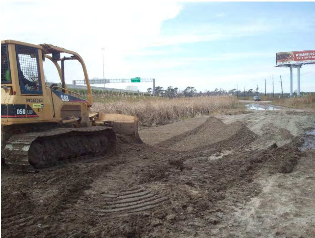
Photo 2 – Grading crushed concrete road base on TxDOT ROW west of main access gate
