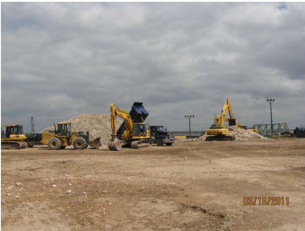
Photo 4 – Receiving Armor Cap A rock at the LaBarge Property (at left); Armor Cap D stockpile (at right).
