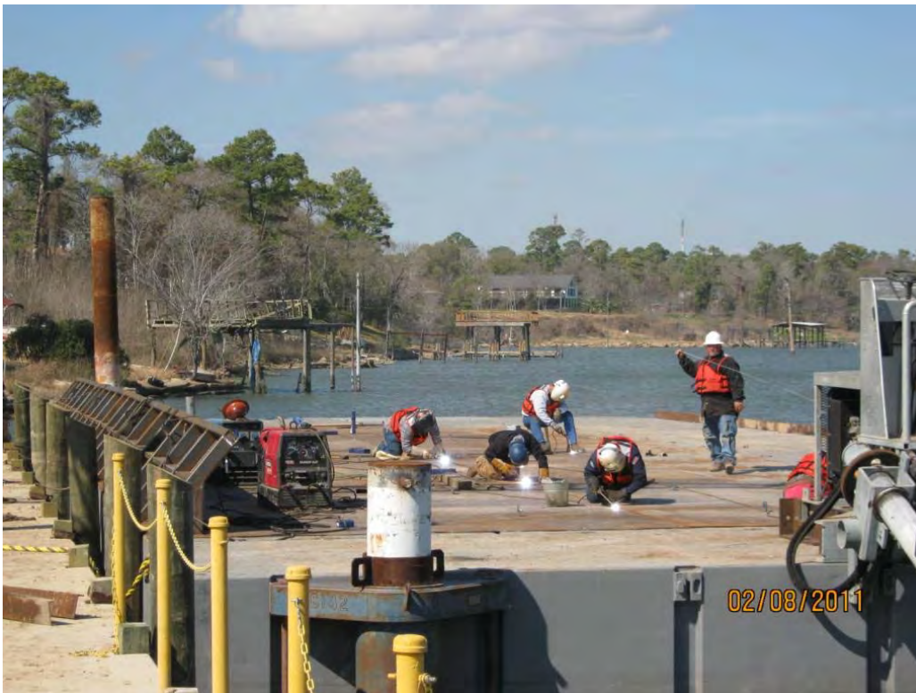
Photo 6 – Welding steel plates onto deck of aggregate transport barge
