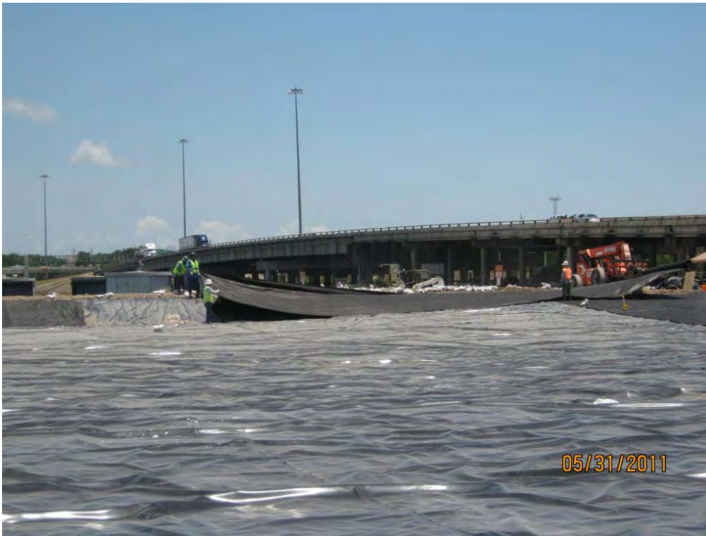
Photo 2 – Deploying 16-oz geotextile atop the LLDPE liner in the Western Cell.
