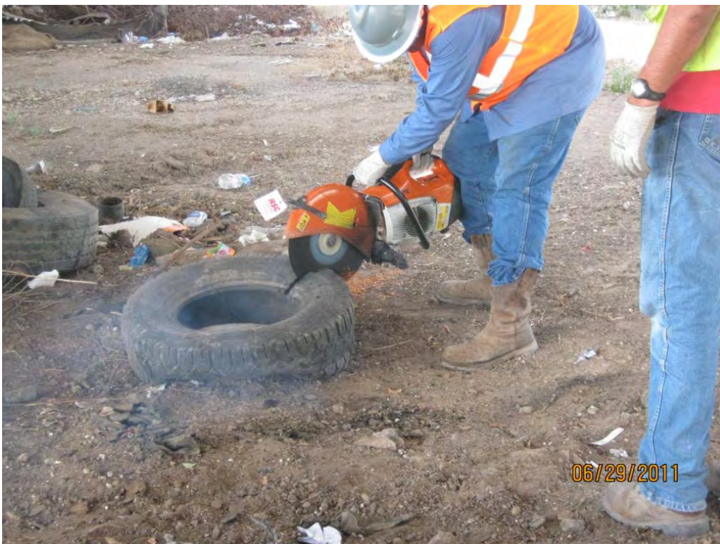
Photo 4 – Quartering tires on-site in preparation for future disposal of the tires at Coastal Plains RDF.
