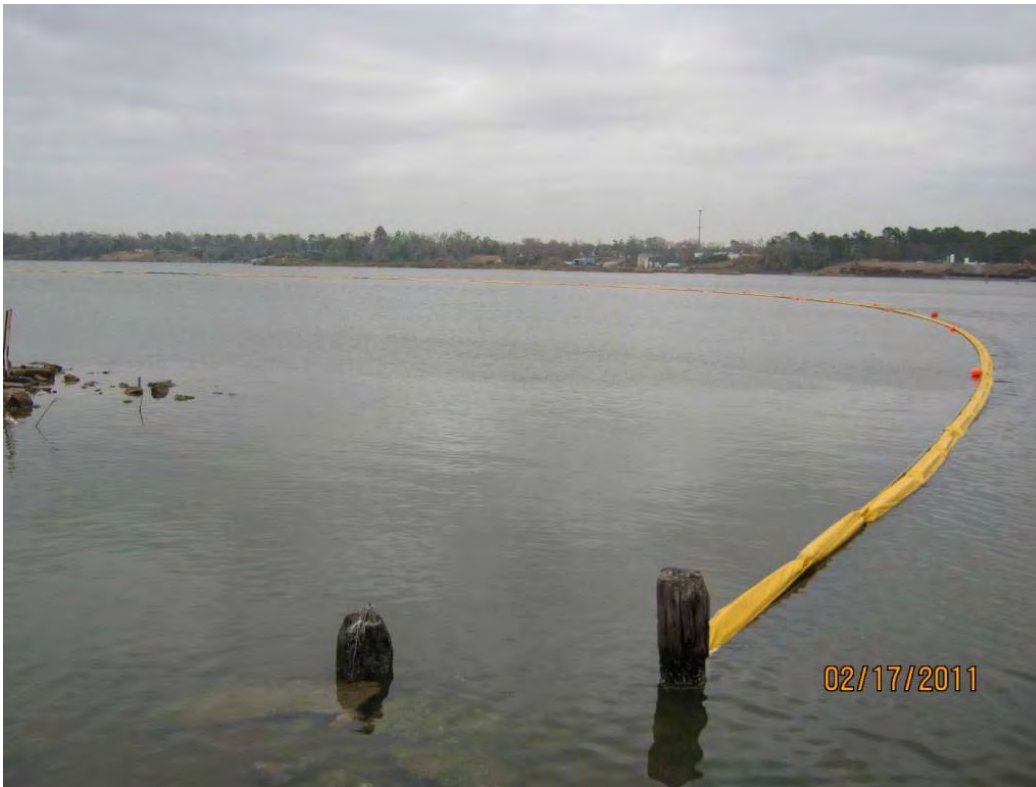
Photo 3 – Turbidity curtain deployed around perimeter of east cell
