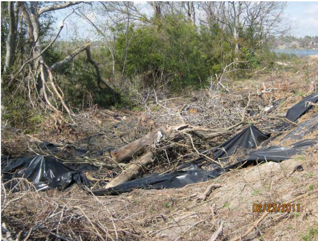
Photo 1 – Stockpiling vegetation cleared from the central berm onto plastic sheeting within west cell
