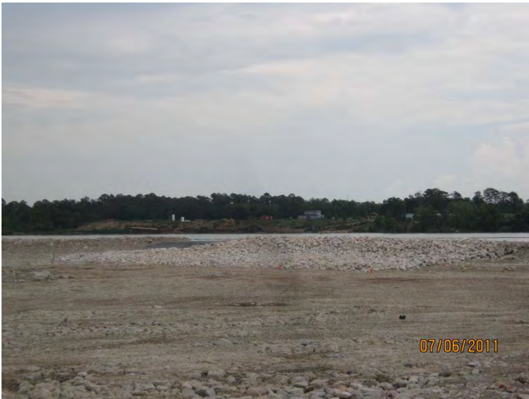
Photo 4 – Armor Cap D rock placed in the Western Cell.
