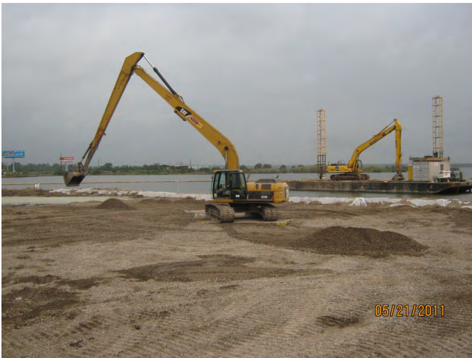
Photo 2 – Excavator placing CCRB adjacent to the northern berm in the Western Cell.
