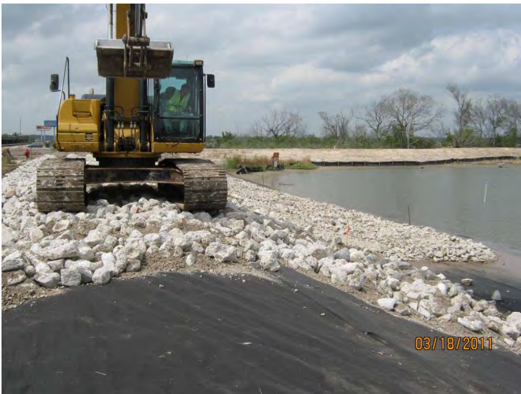
Photo 6 – Armor Cap B/C rock placed atop geotextile on the south berm of the east cell.
