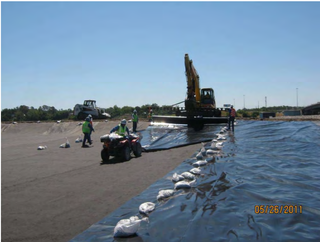
Photo 1 – Deploying LLDPE liner in the Western Cell.
