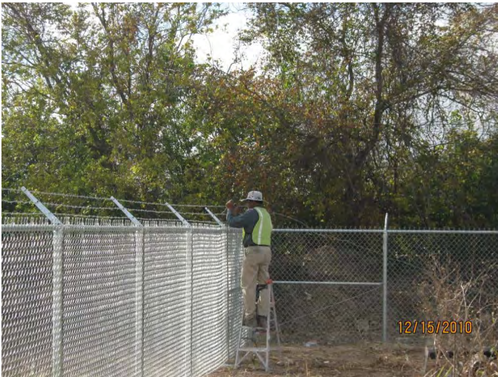
Photo 2 – Installing barbed wire atop 6-foot chain link fence along west edge of Big Star property.
