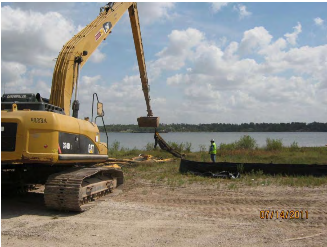
Photo 2 – Picking up a section of turbidity curtain for placement into a roll-off box.
