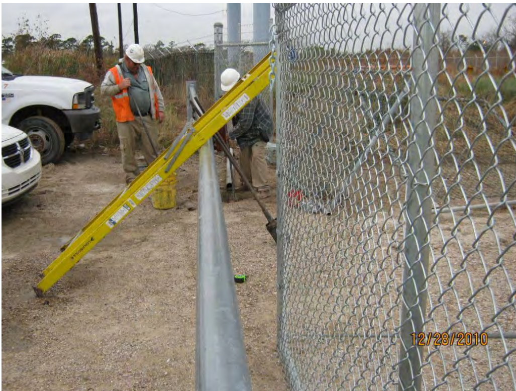
Photo 7 – Installing gate post for western gate entrance to Big Star property.
