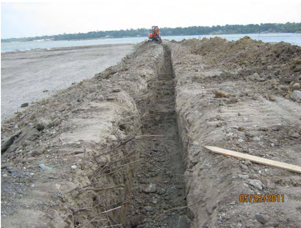
Photo 2 – Anchor trench excavated along the top of the central berm.
