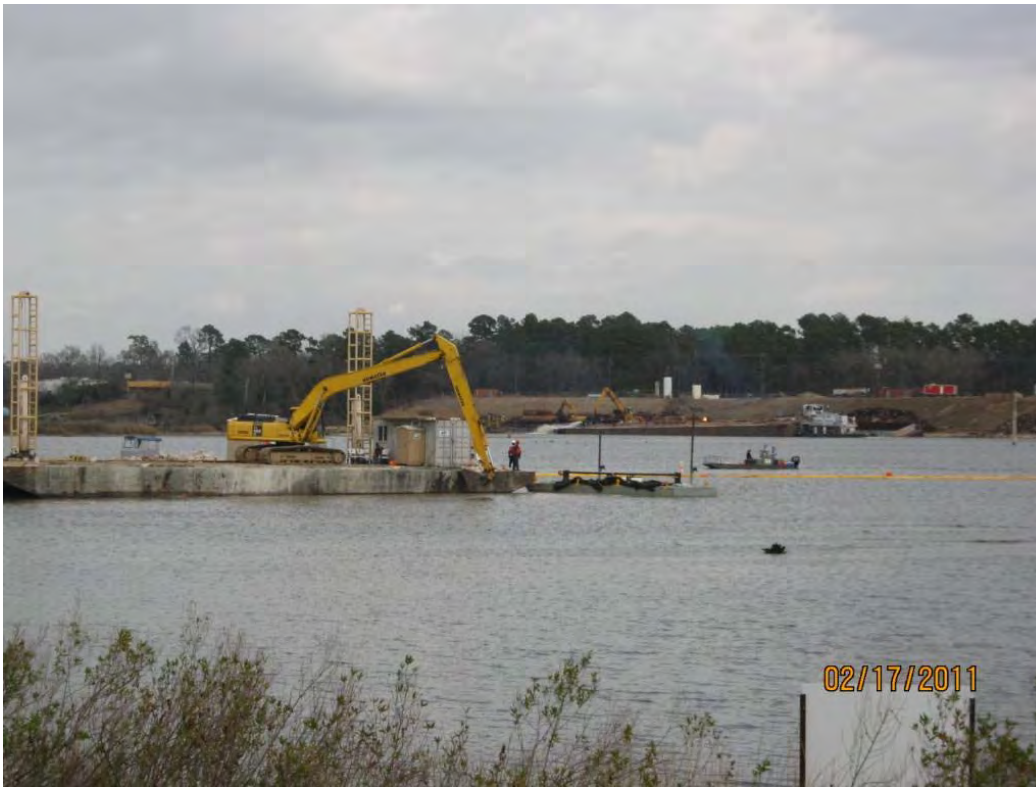
Photo 7 – Placing Armor Cap D rock in east cell (foreground), turbidity monitoring (smaller boat in background)
