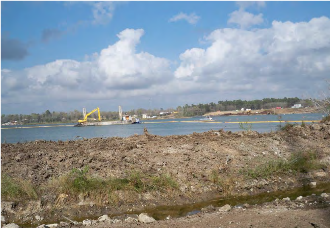
Photo 1 – Deploying geotextile and placing Armor Cap D rock in the east cell; repositioning the turbidity curtain.
