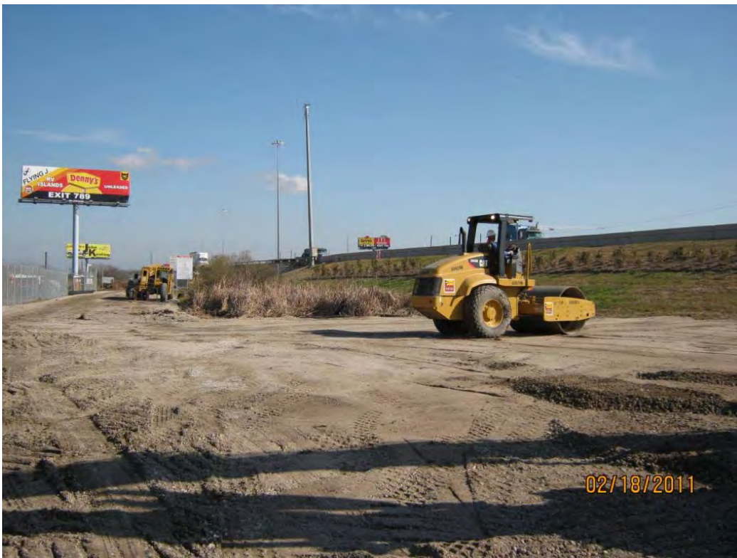
Photo 5 – Compacting crushed concrete road base for truck turnaround area outside main access gate
