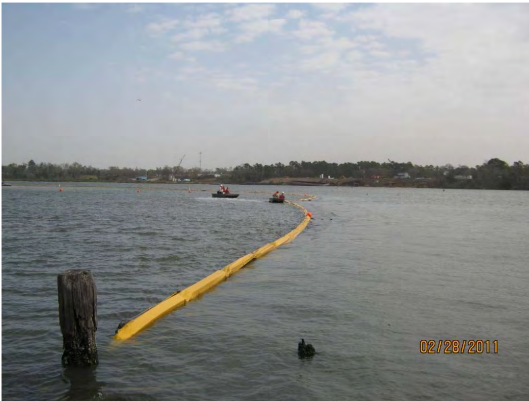
Photo 2 – Repairing breach to the turbidity curtain in the south half of the east cell
