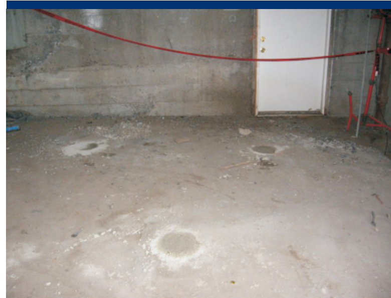
Photo 67 Holes in concrete floor were filled with quick-drying concrete upon completion of sampling.
