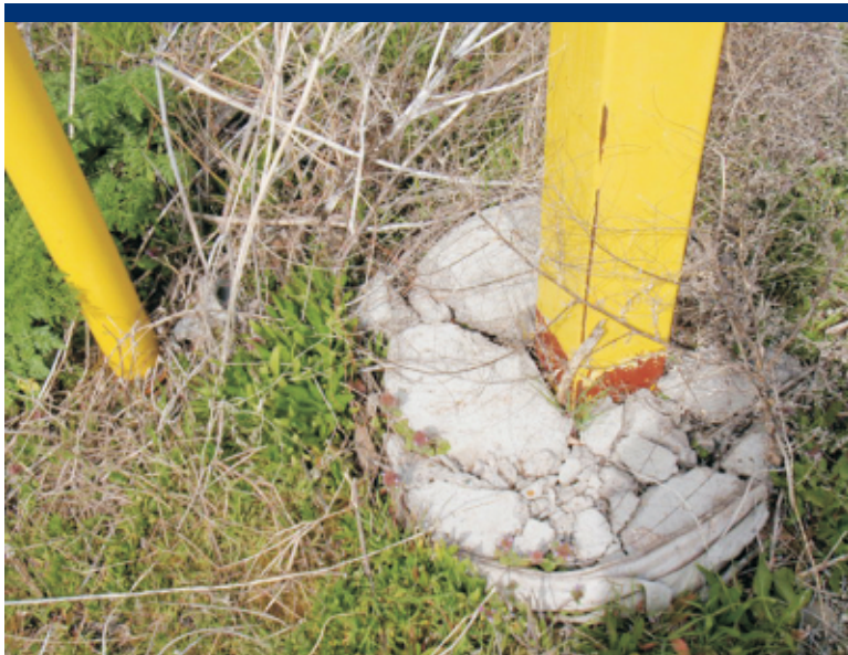
Photo 84 Closeup of damaged base at monitoring well MW02.
