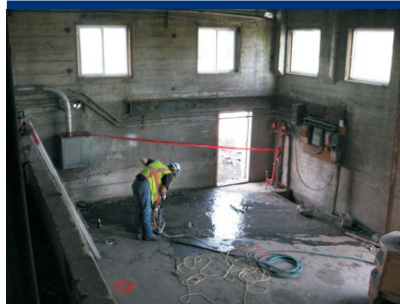
Photo 63 Coring through the concrete floor of the shop building.
