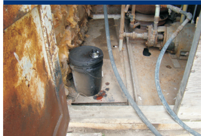
Photo 75 Interior of wellhouse near the process area with container of oily substance and stained flooring.
