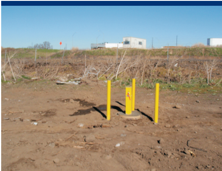
Photo 52 Installed monitoring well MW03.
