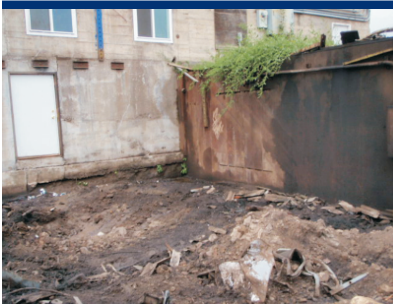
Photo 58 View of stained retaining wall and former location of baler and press; note the stained soil.
