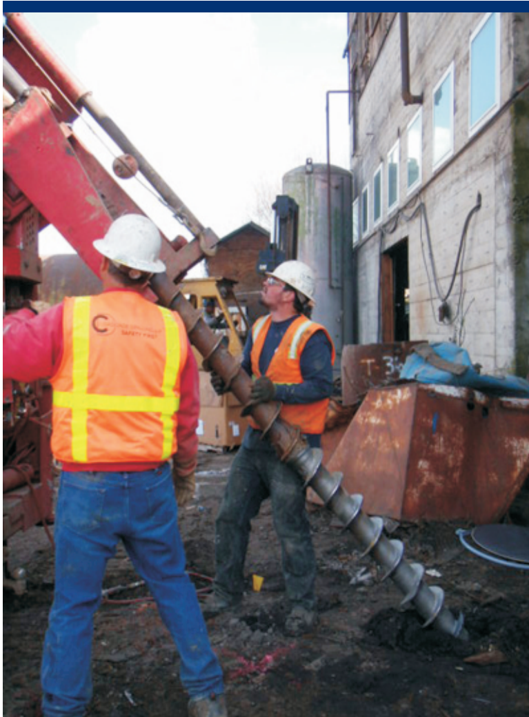
Photo 47 Installing investigative borehole SB02 near the baler at an angle.
