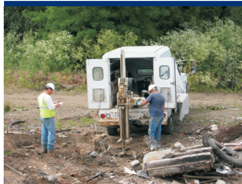
Photo 69 Installing a borehole in the process area.
