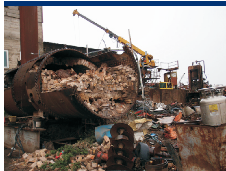
Photo 26 Partially demolished kiln; crane is operating in the background.
