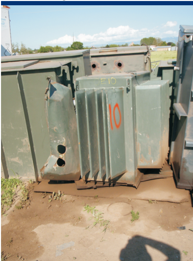
Photo 12 Leaking transformer and stained soil east of process area.
