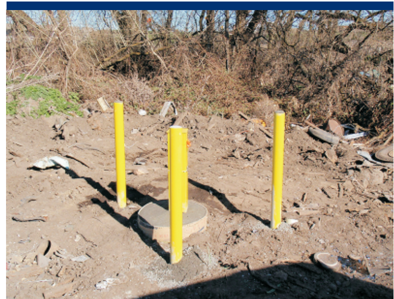
Photo 53 Installed monitoring well MW02 near the swale.
