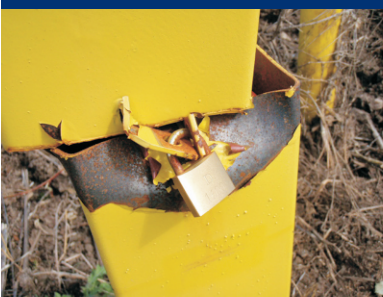
Photo 86 View of damaged riser and padlock at monitoring well MW04.
