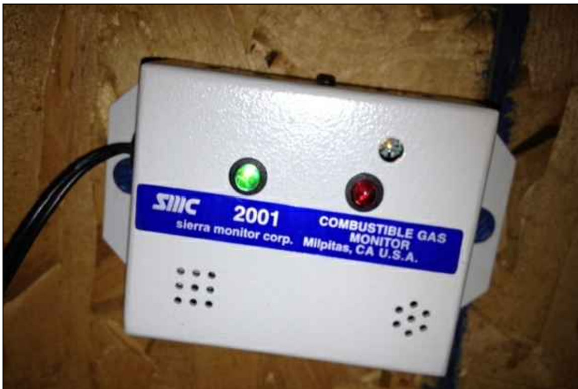
PHOTO 1: METHANE MONITOR CLOSE-UP IN SIM TRAINER, 2031 DRYDEN ROAD
