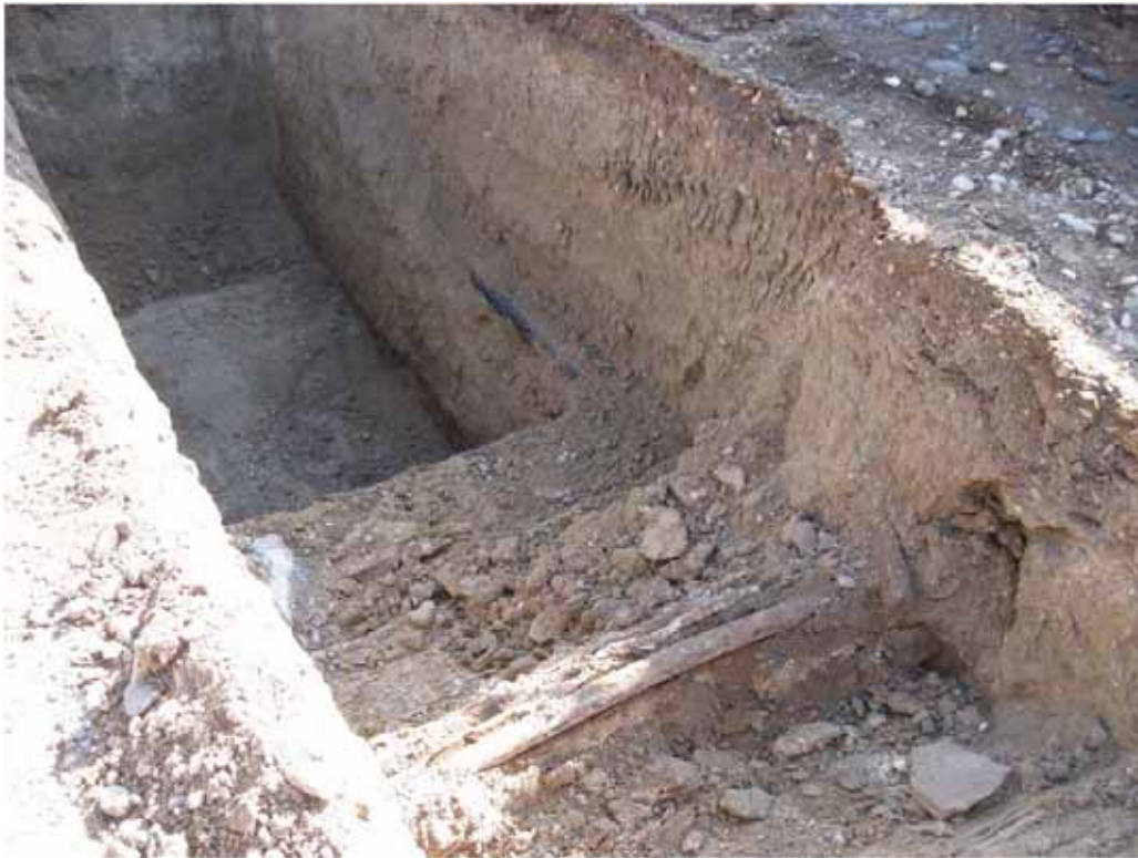
PHOTO 18 Test Pit 09: Subsurface piping through test pit
