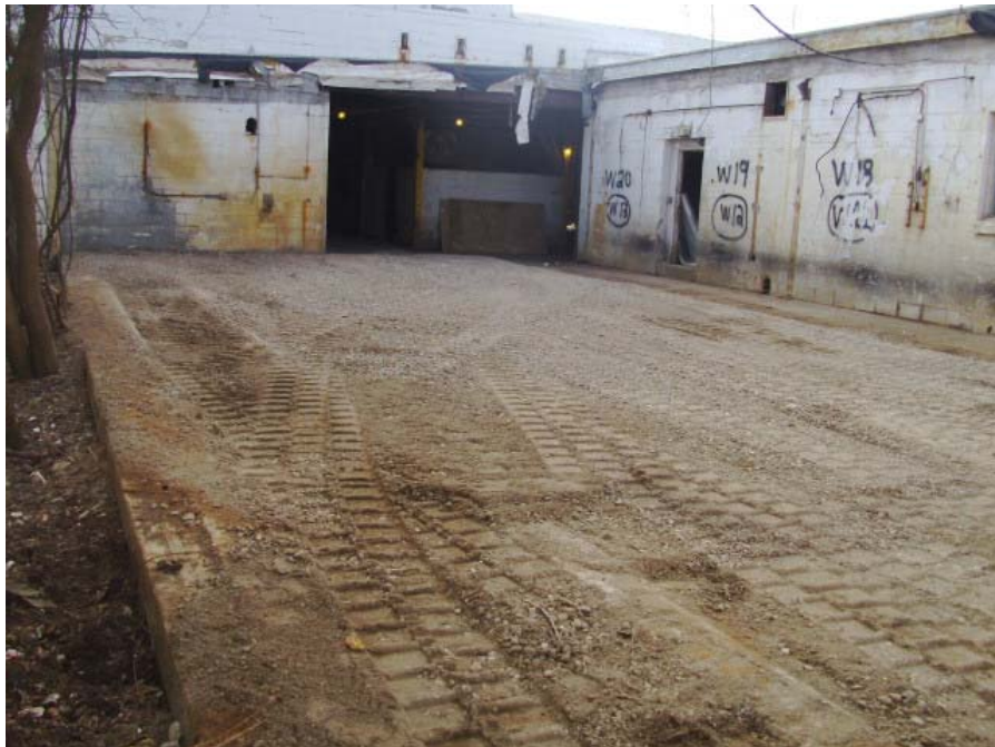
Site: Baycote Metals Finishing Site Photograph No.: 38 Direction: East Subject: Completed backfill of Area W
