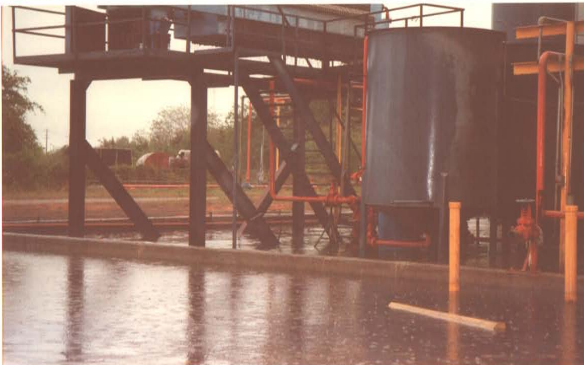
Picture: 6 of 47 Date: 4/7/2005 Time: 2:40 pm Direction: NA Agency: Georgia Hazardous Waste Management Branch Photographer: Eddie Williams Subject: Additional view of ponded rainwater on the outside of the plant's secondary containment.
