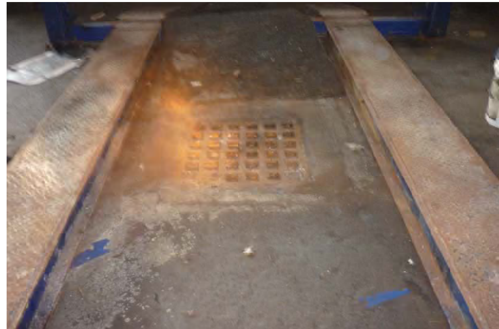
16 Catch basin style floor drain-main site bldg.jpg
