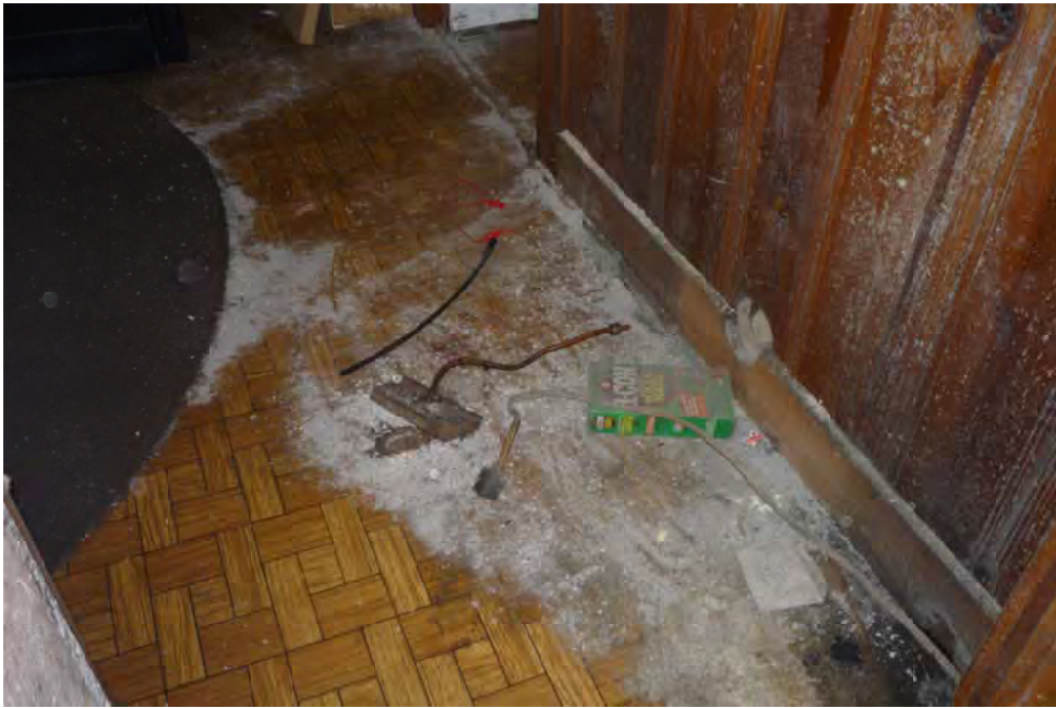
21 Potential mold growth & copper tubing-main site bldg.jpg
